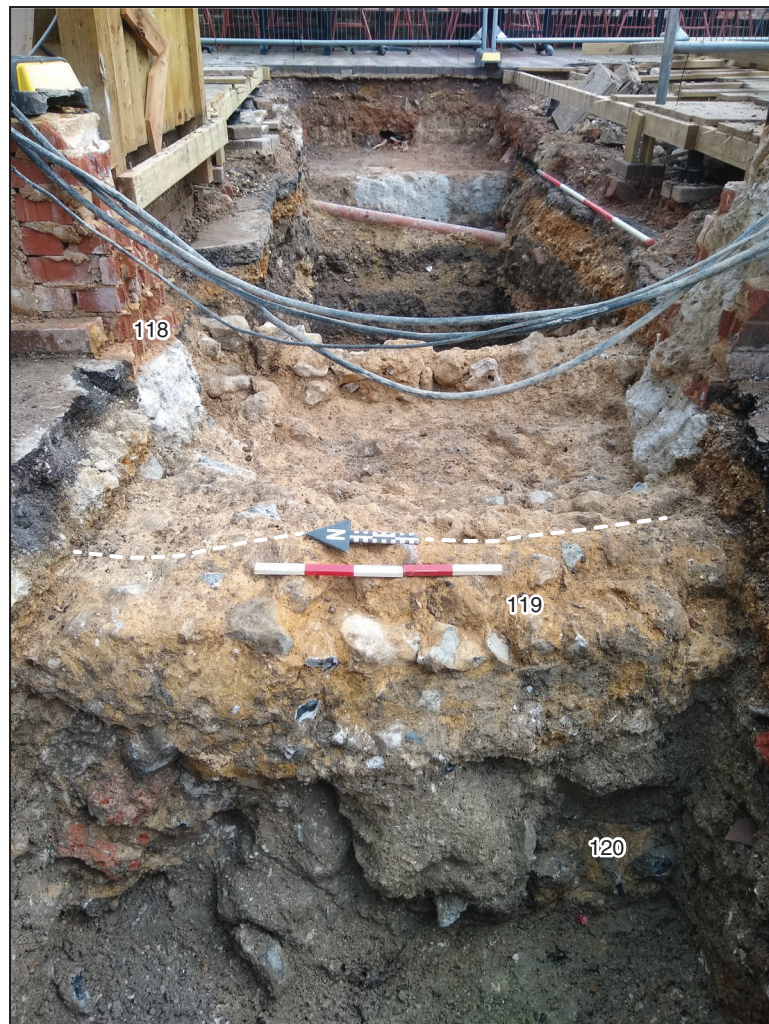
Elevations of walls 117, 119 and 120, looking east (0.5m scale)
