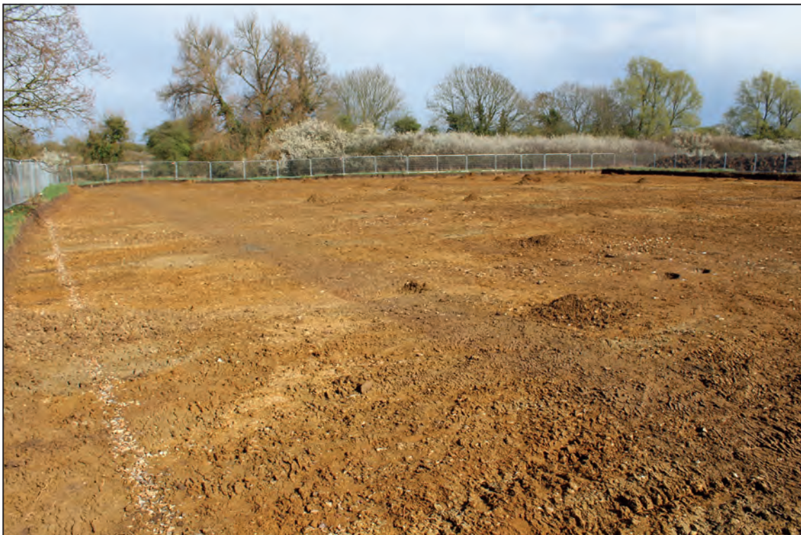
Excavation area, looking east
