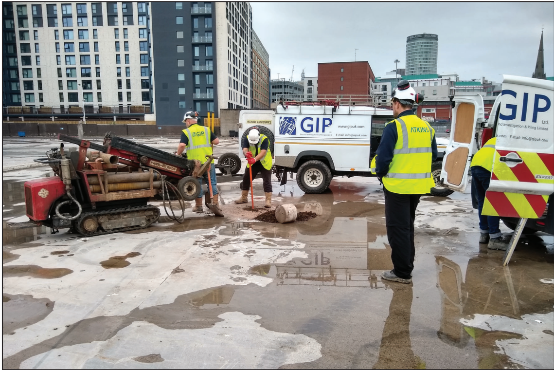
General view of borehole WS02, looking north
