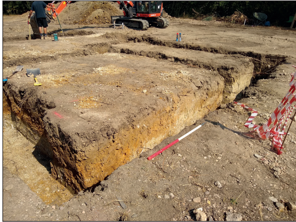
Plot 1, observed groundworks, looking north (1m scale)
