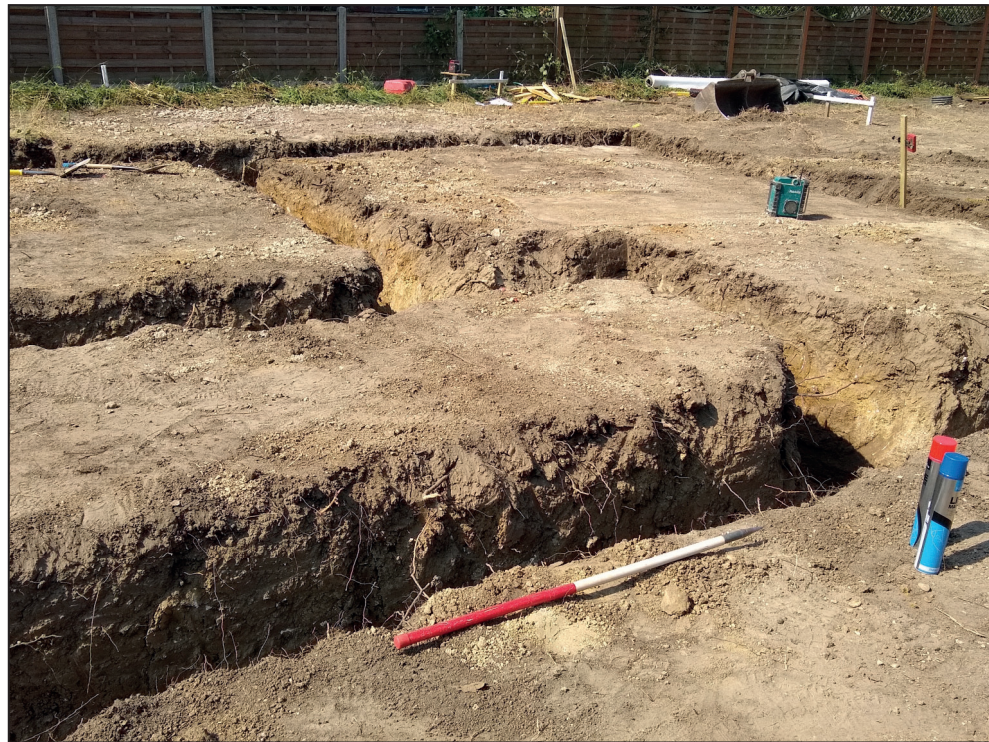
Plot 1, observed groundworks, looking west (1m scale)
