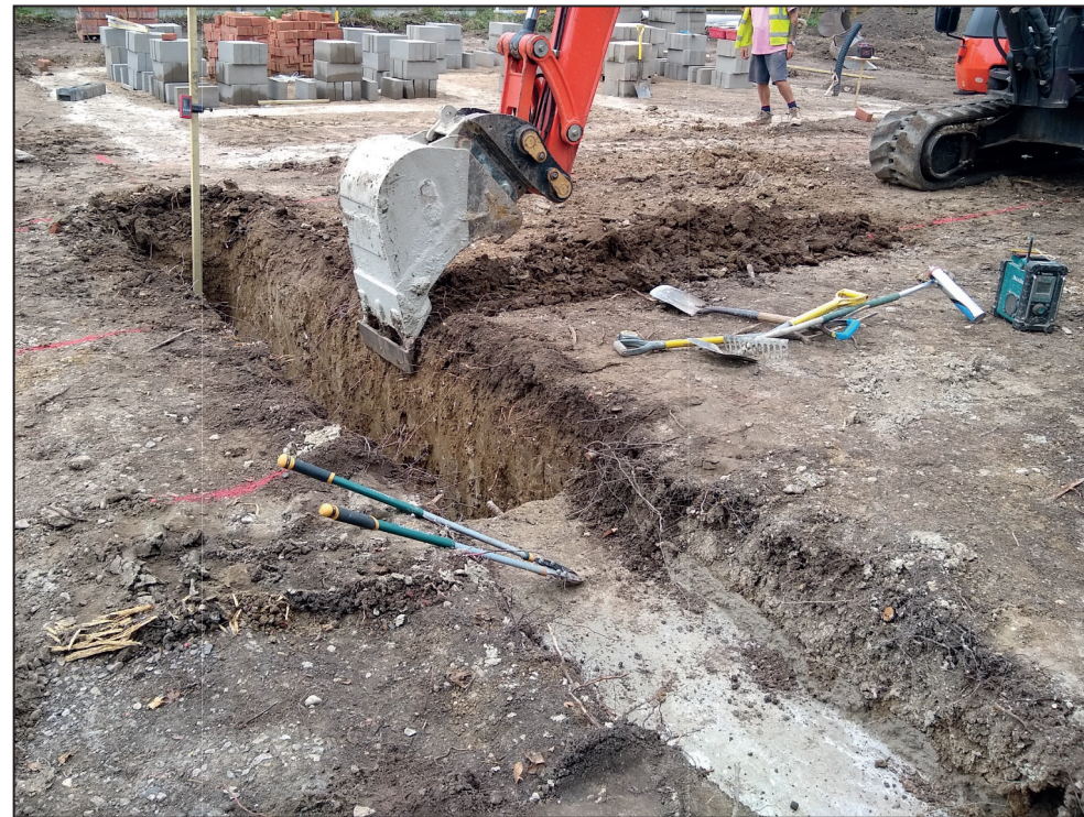
Plot 2, observed groundworks, looking west (1m scale)
