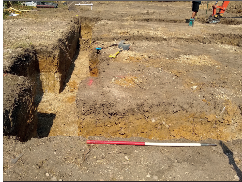
Plot 1, observed groundworks, looking north-west (1m scale)
