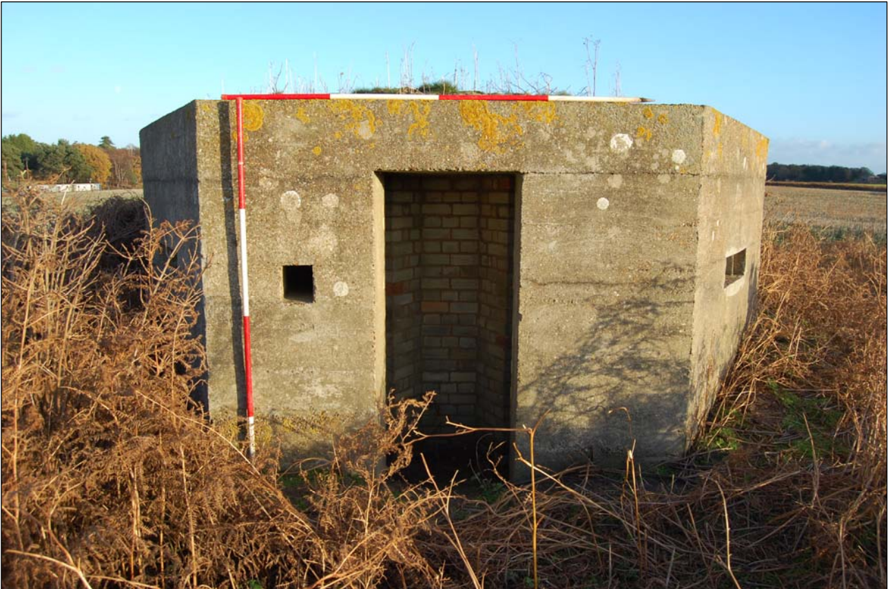
Plate 15. Type 22 pillbox, showing doorway and small loophole, facing east, 2x2m scales
