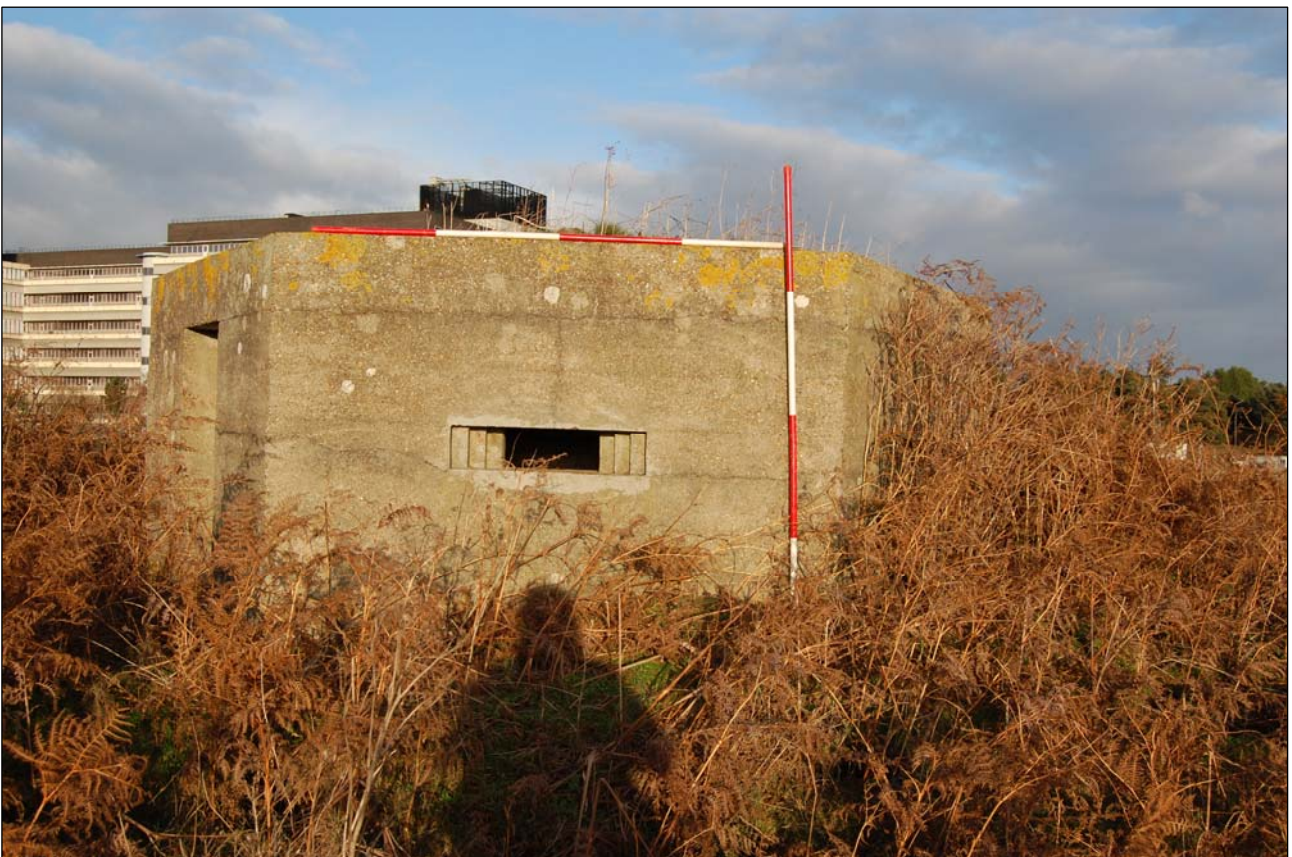
Plate 16. Type 22 pillbox, showing typical elevation, facing north-east, 2x2m scales
