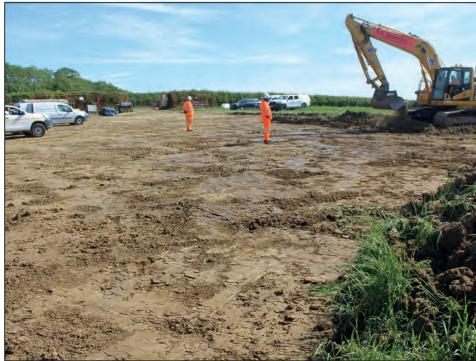
Working shot of watching brief Area 2, looking north-east
