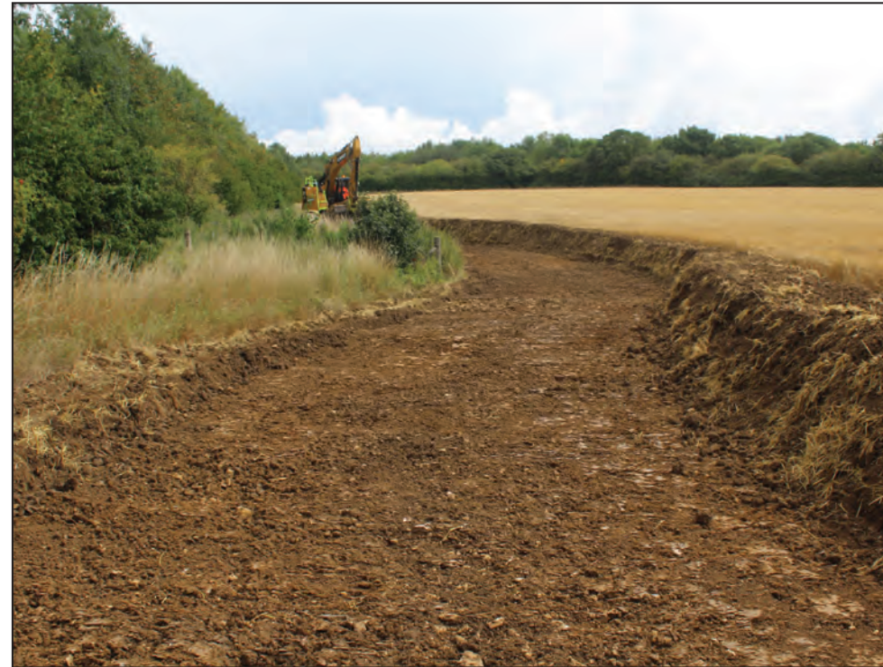
Working shot of northern watching brief Area 1, looking east
