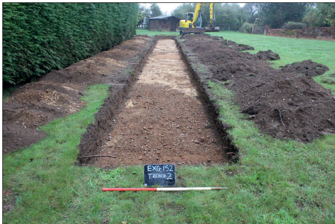
Trench 2, looking west south-west (1m scale)
