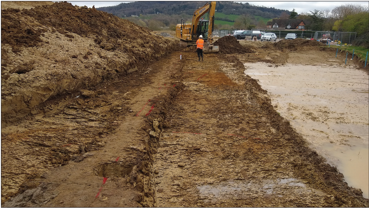
Area 2 ongoing stripping along service corridor
