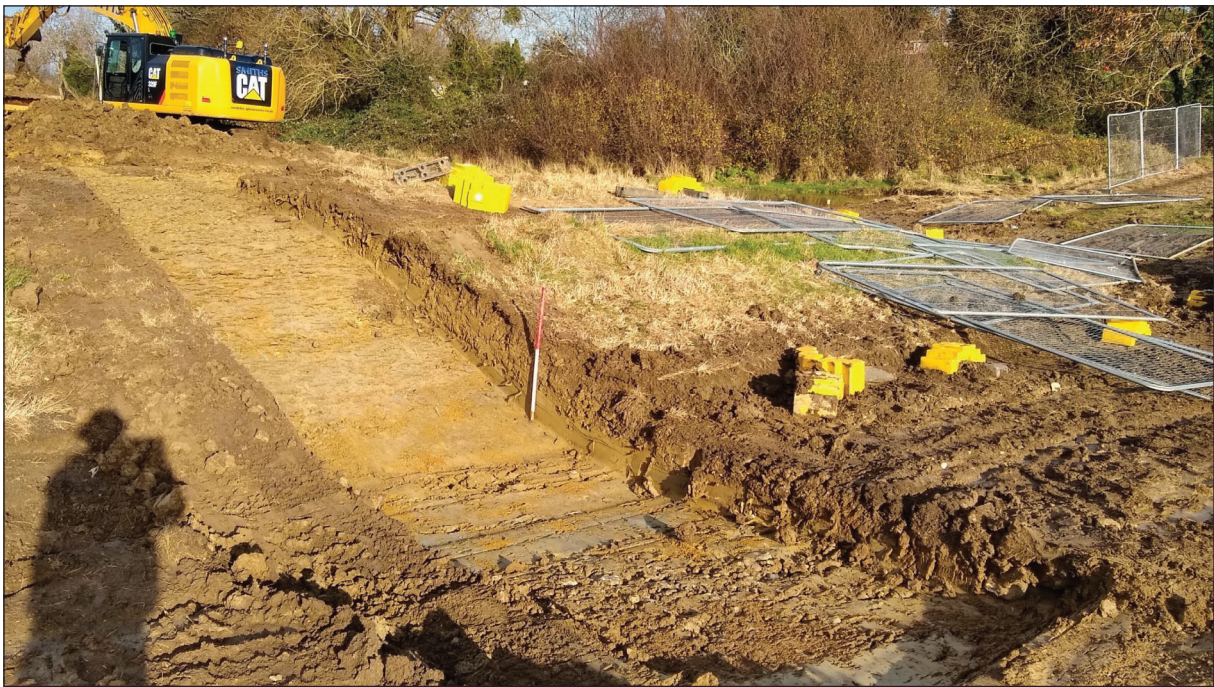
Area 3 oblique view of west-facing section of excavated trench across a geophysical anomaly/natural coombe
