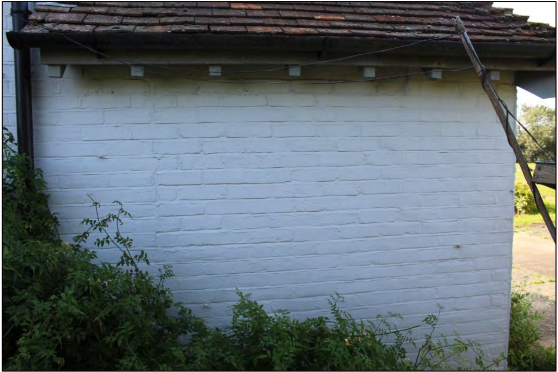
Photo 10: Northern elevation of single-storey projection
