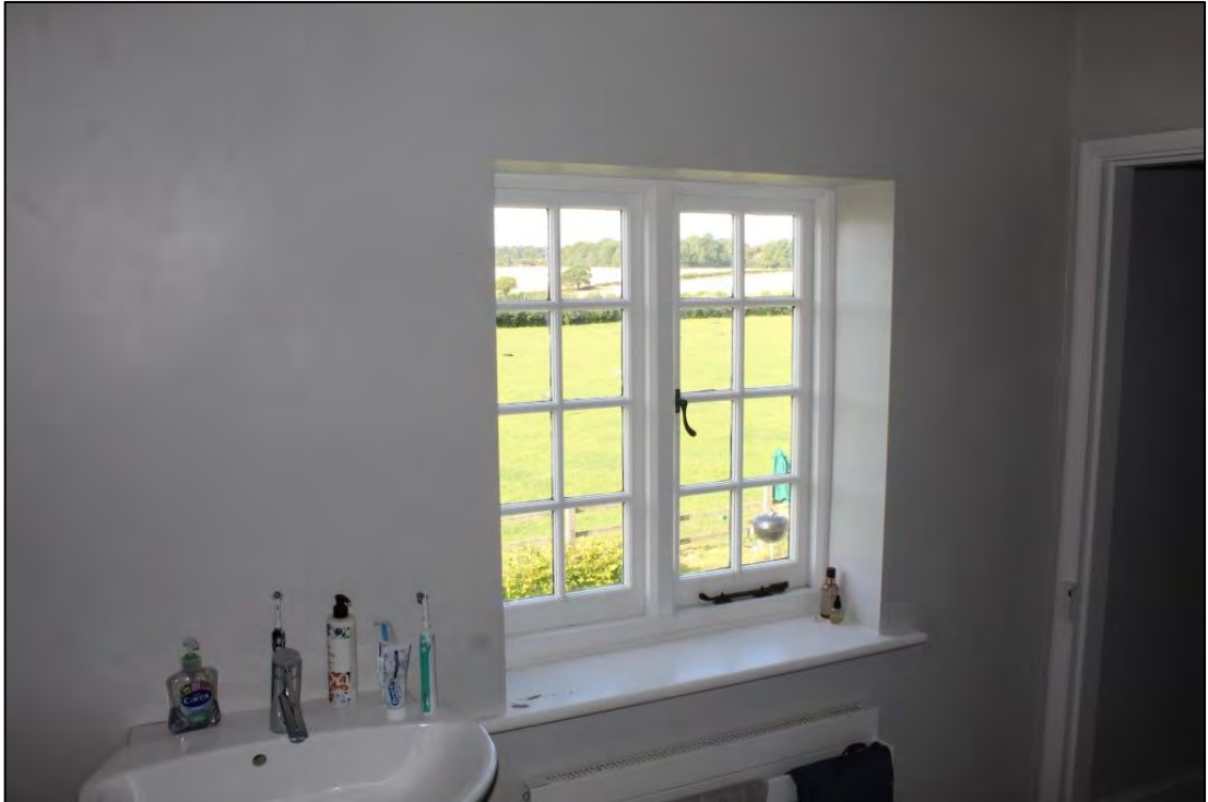
Photo 27: Overview of window within Room 10, looking west
