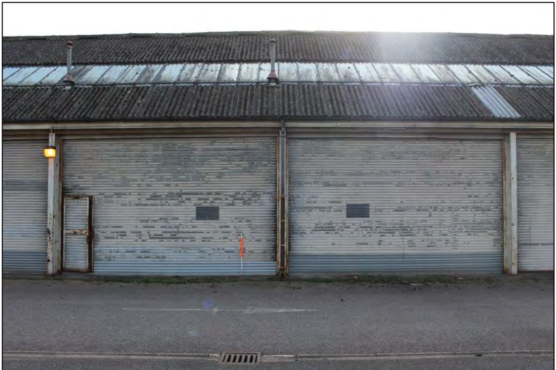
Photo 138: Building D, North elevation 2
