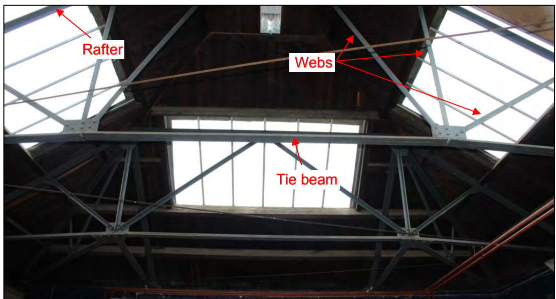
Photo 24: Example of 'fan' roof truss within Room B2
