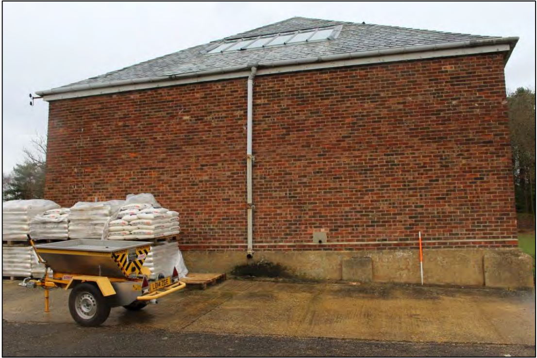
Photo 88: Building A, South elevation
