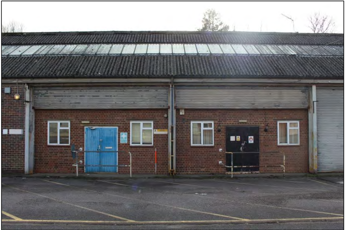
Photo 141: Building D, North elevation 5
