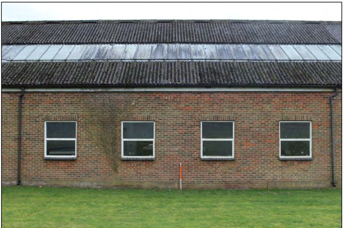
Photo 118: Building C, North elevation 2
