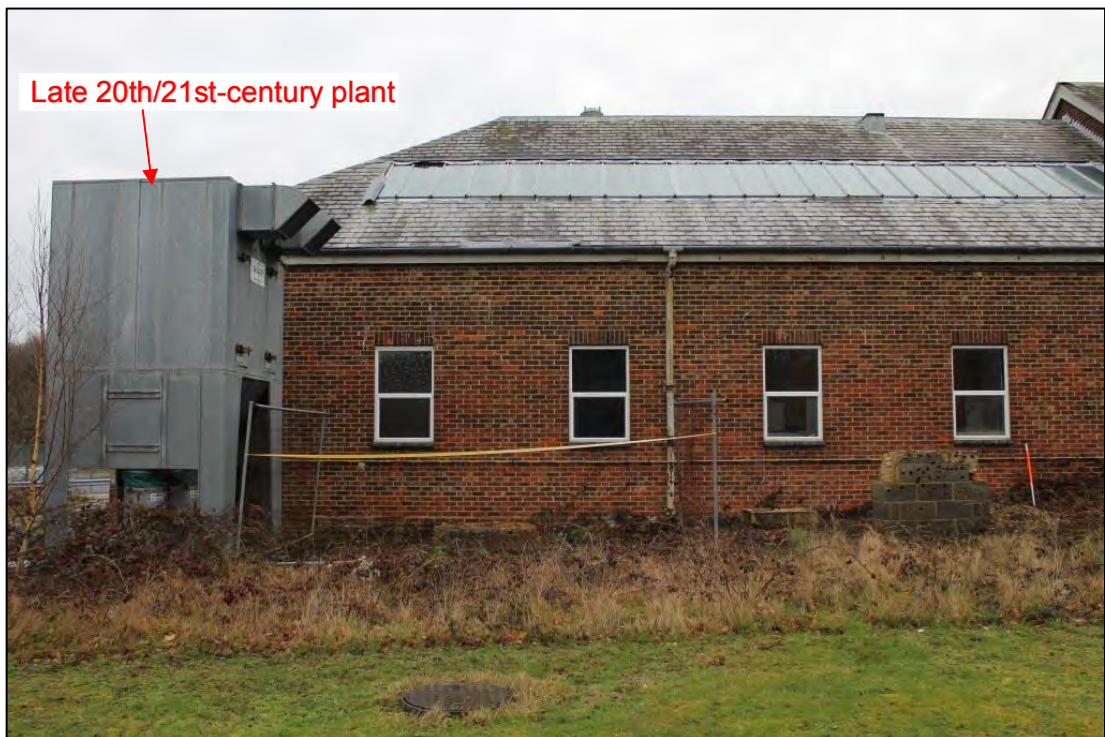
Photo 18: Eastern elevation of Building B showing late 20th/21st-century plant
