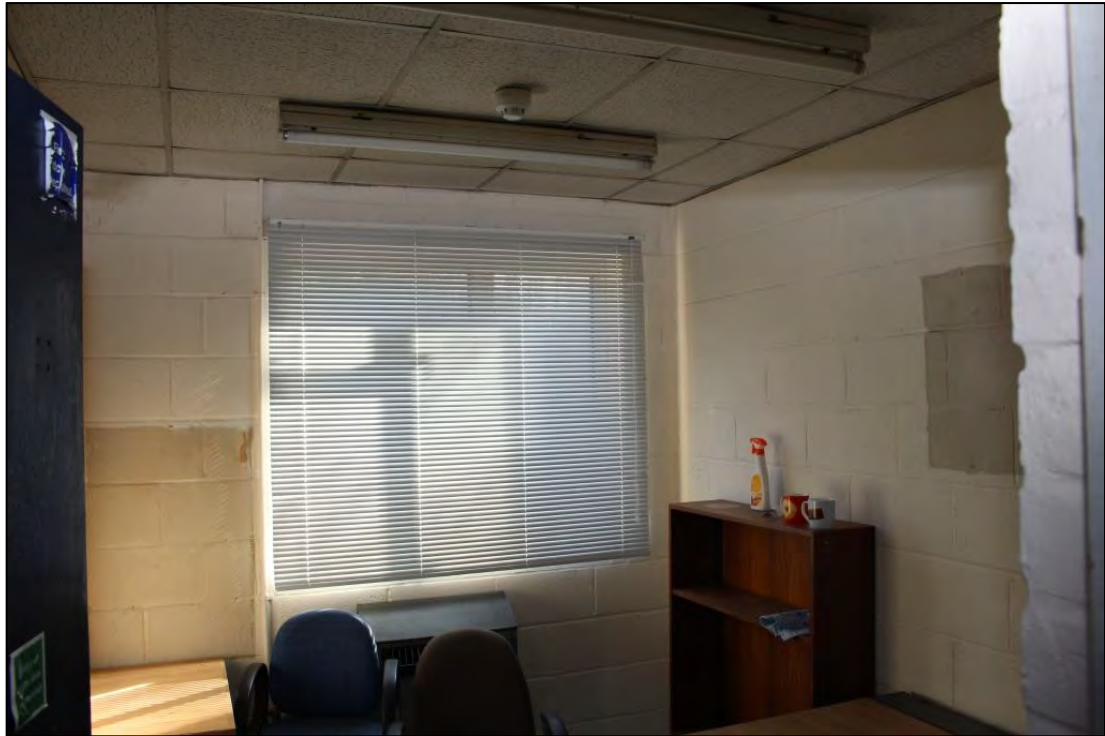
Photo 72: Overview of Room D4, looking east
