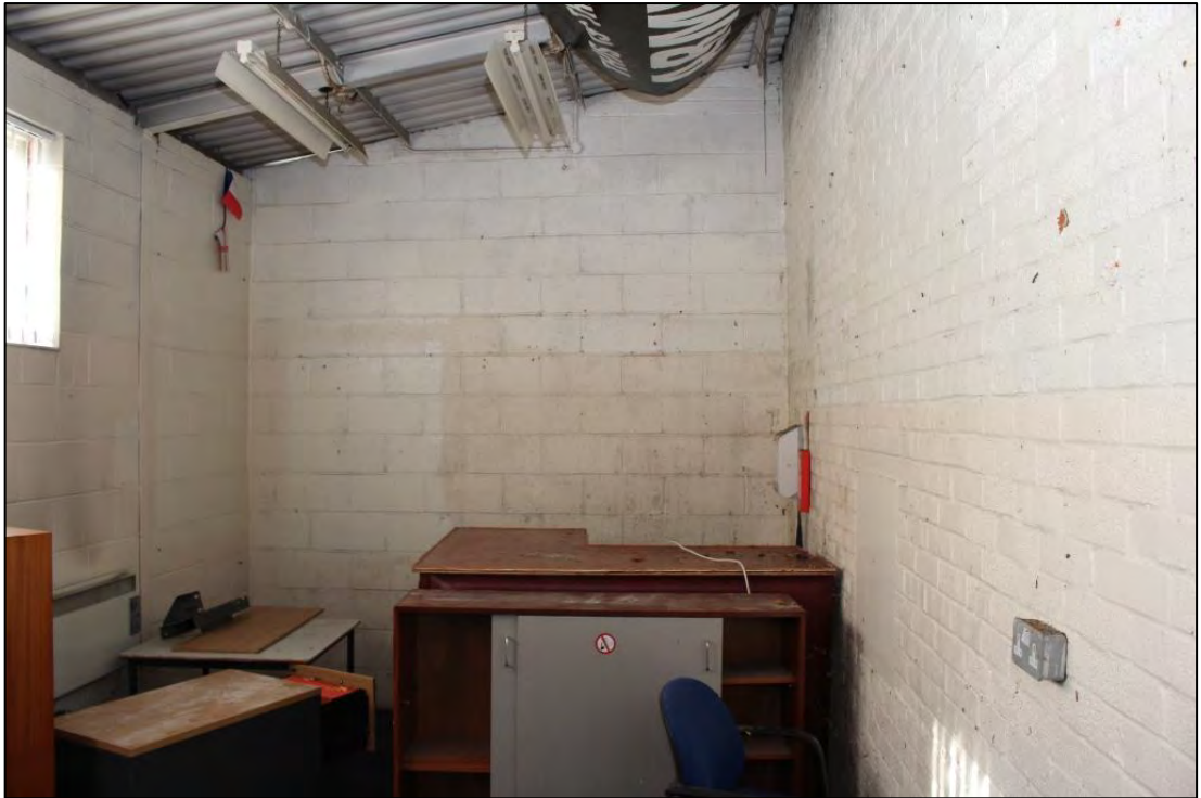
Photo 73, Overview of Room D7, looking west
