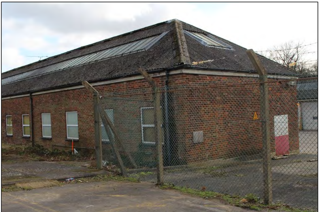
Photo 35: Northern and western elevations of Building C
