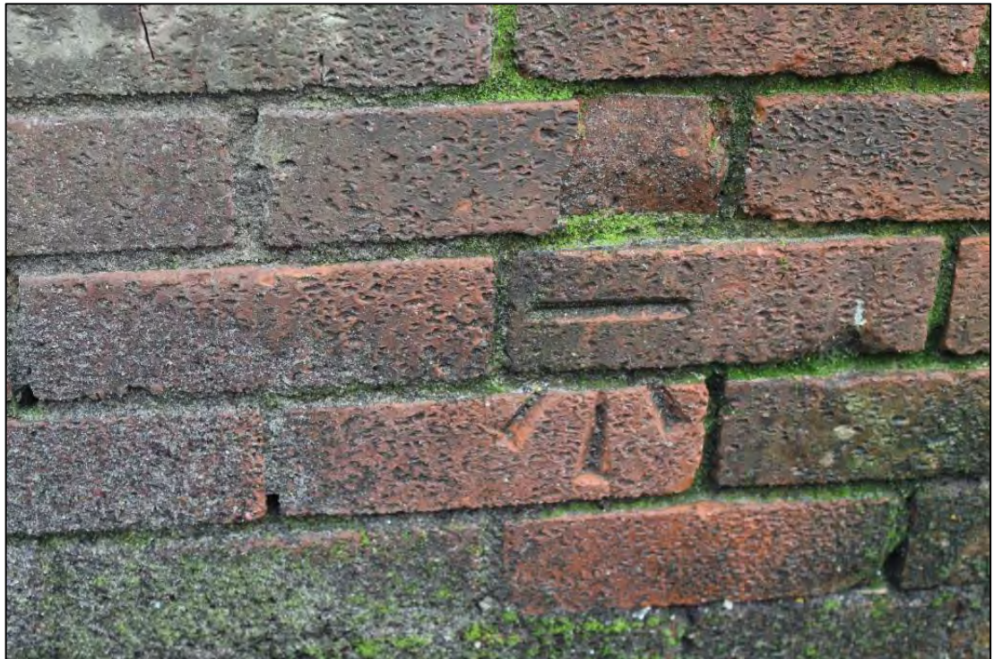
Photo 6: OS Benchmark Locator at western extent of Northern elevation
