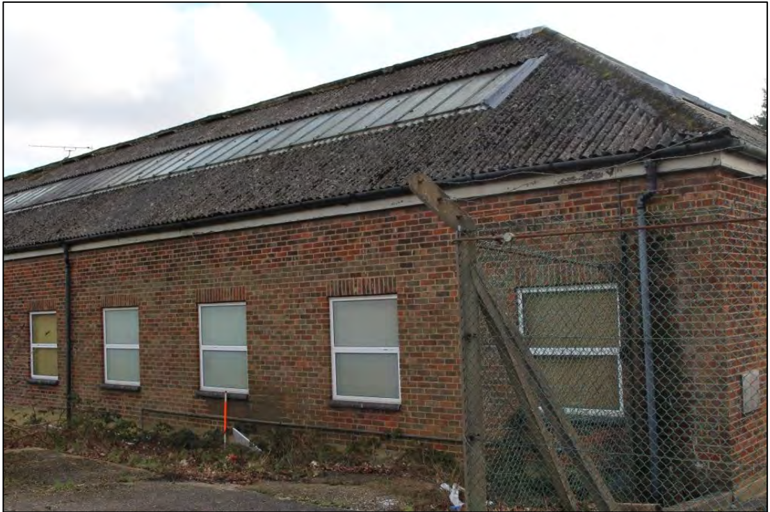
Photo 125: Building C, North elevation 9
