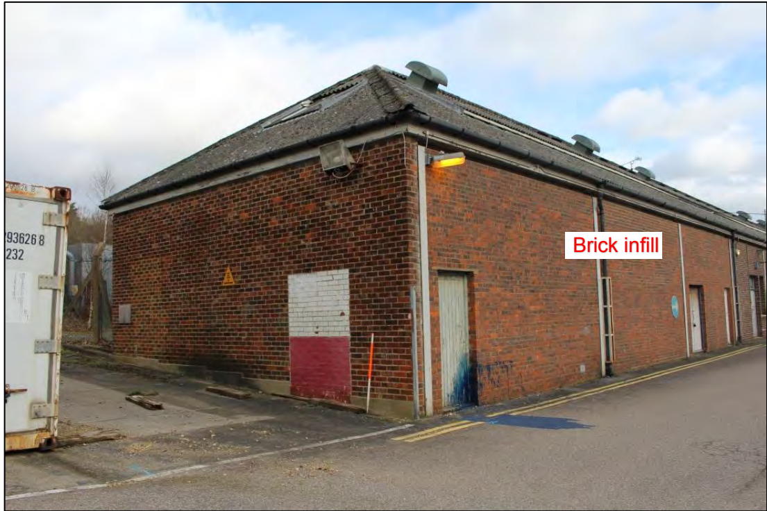
Photo 32: Western and southern elevations of Building C
