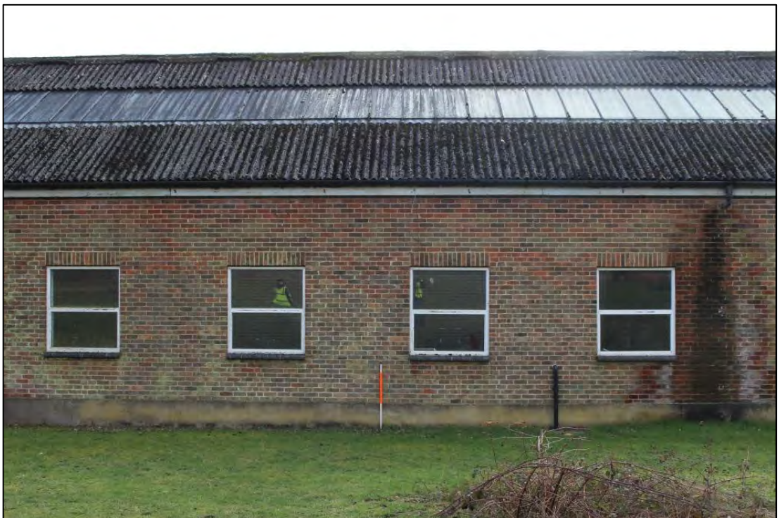
Photo 122: Building C, North elevation 6
