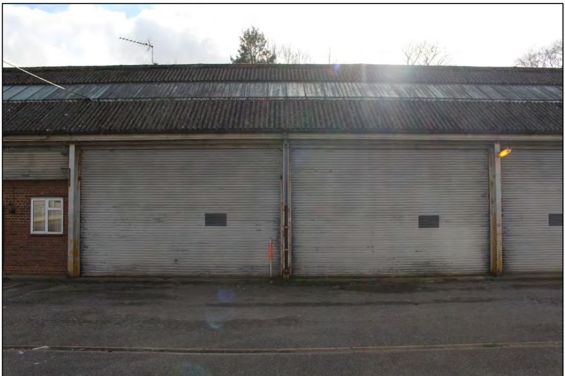
Photo 142: Building D, North elevation 6
