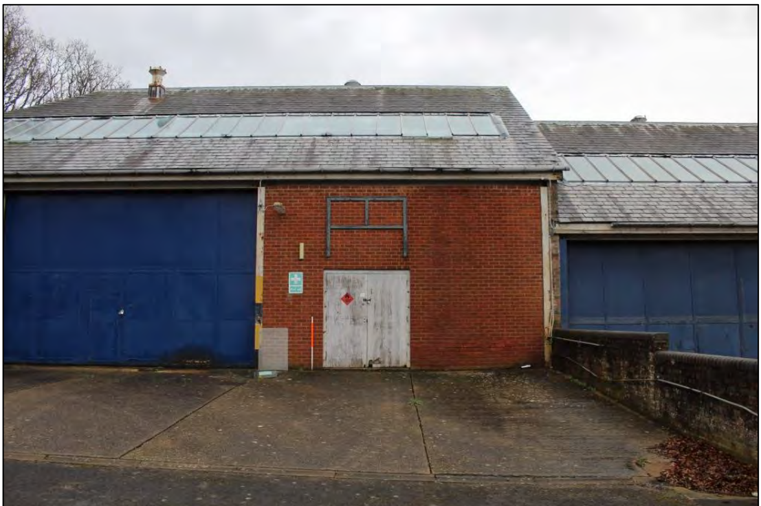
Photo 94: Building A, West elevation 2
