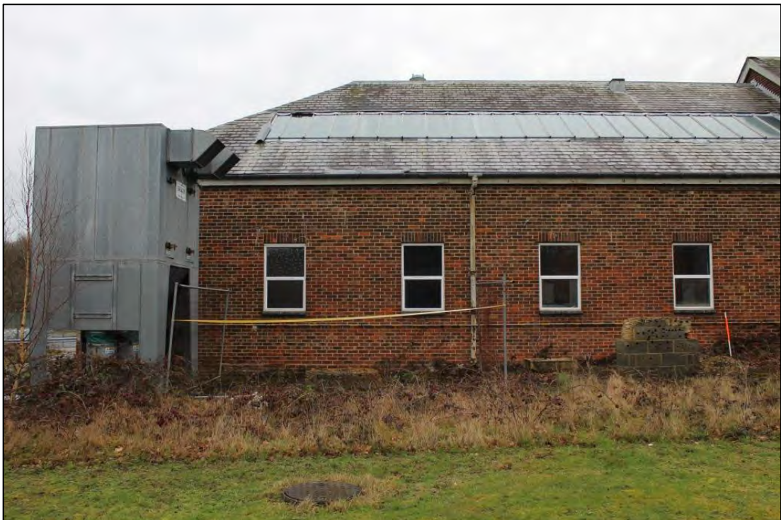
Photo 98: Building B, East elevation 1
