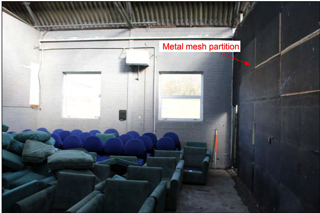
Photo 47: Overview of Room C12, looking north
