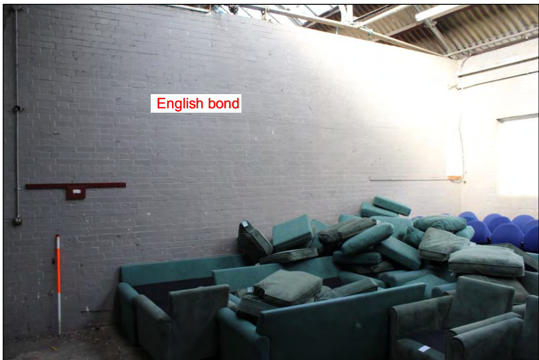
Photo 48: Western wall of Room C12
