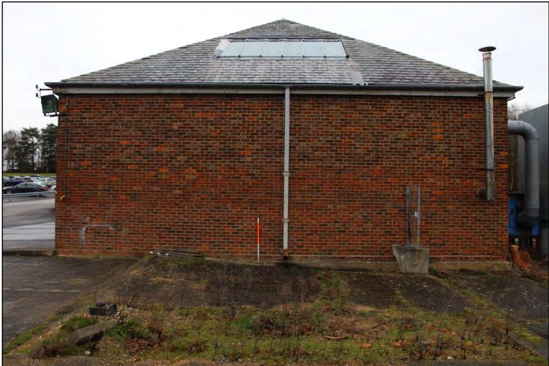
Photo 97: Building B, South elevation
