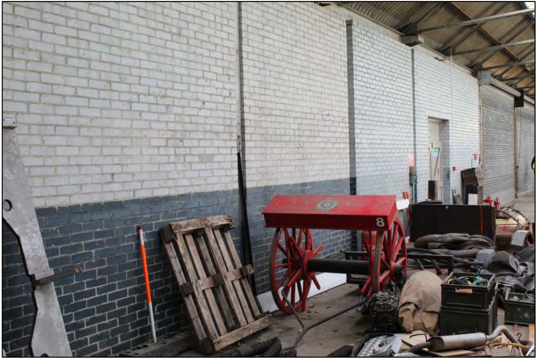
Photo 53: Overview of southern wall of Room C14
