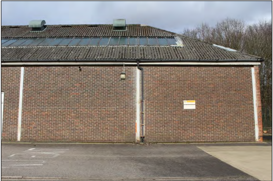
Photo 115: Building C, South elevation 9
