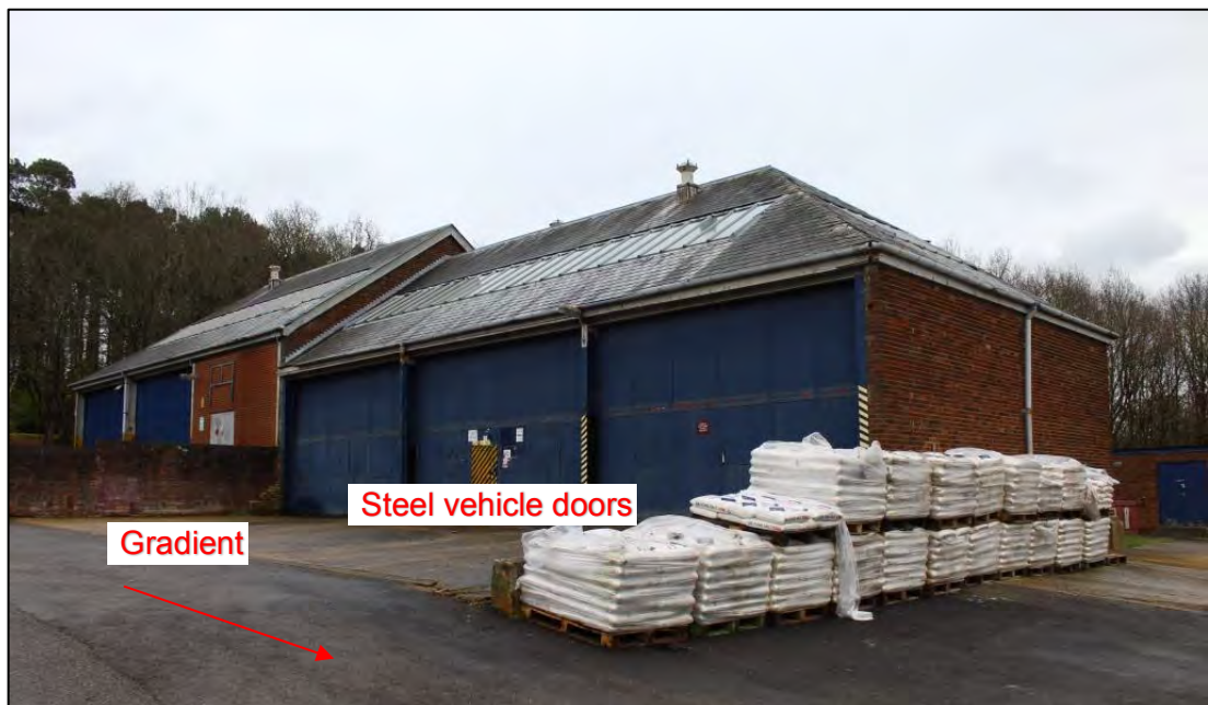
Photo 1: Overview of Building A, western elevation
