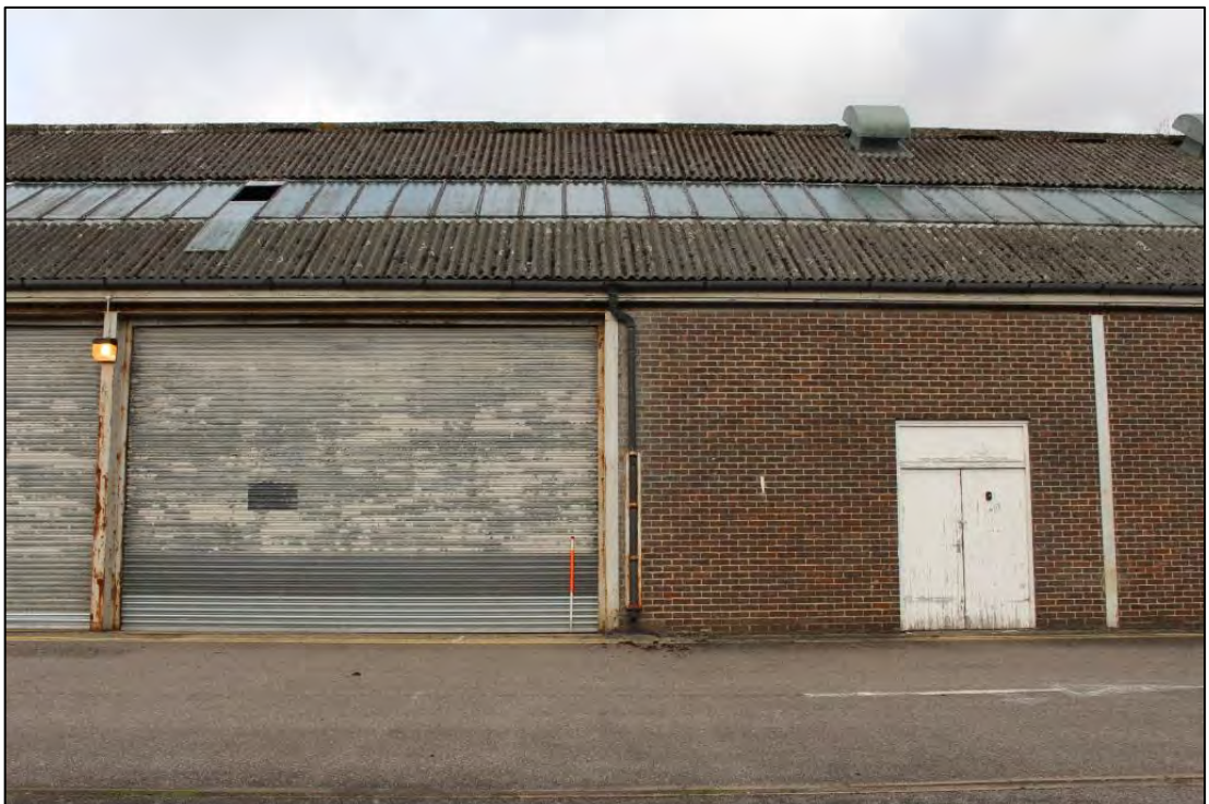
Photo 114: Building C, South elevation 8
