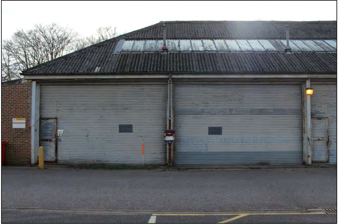
Photo 137: Building D, North elevation 1
