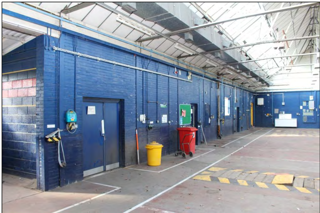
Photo 68: Overview of Room D1, looking south-west
