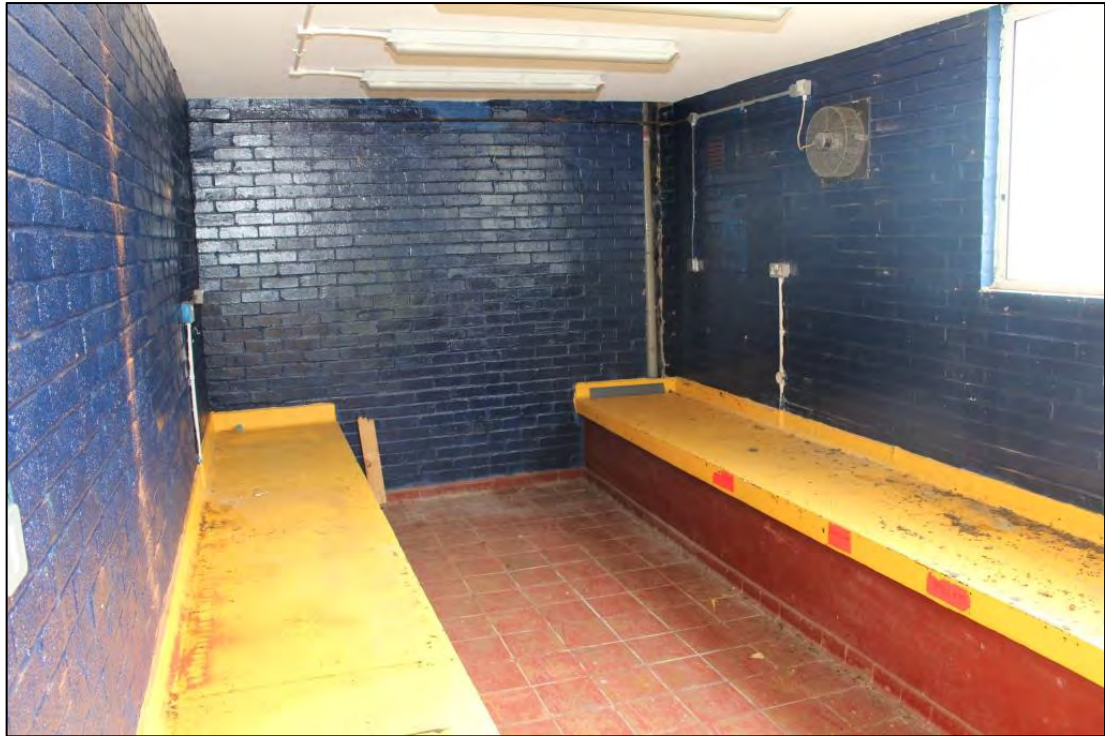
Photo 76: Overview of Room D10, looking east
