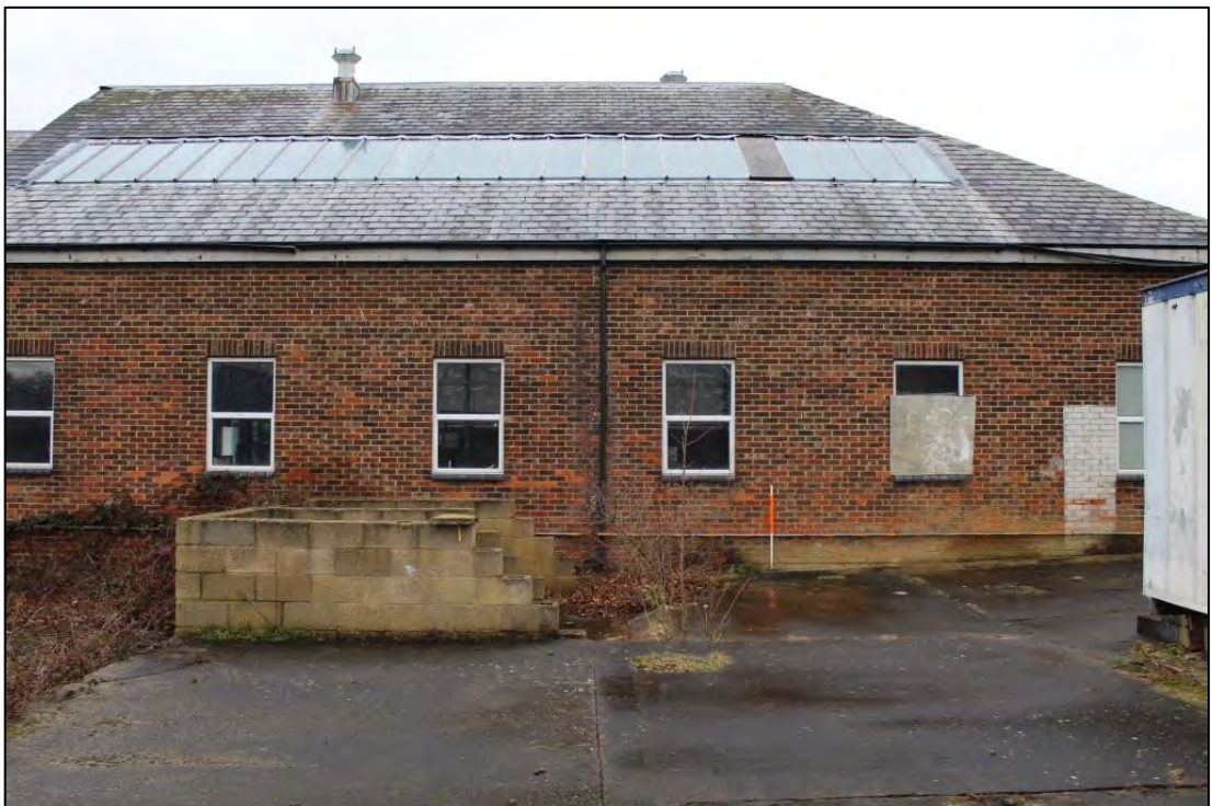
Photo 100: Building B, East elevation 3
