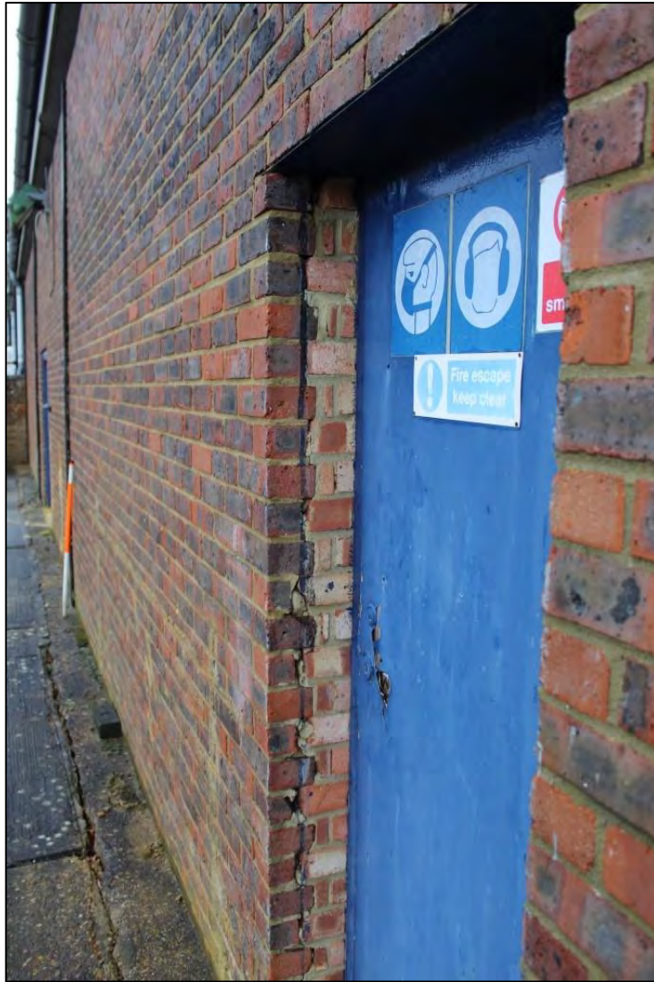
Photo 30: Detail of door reveal in western elevation of Building B
