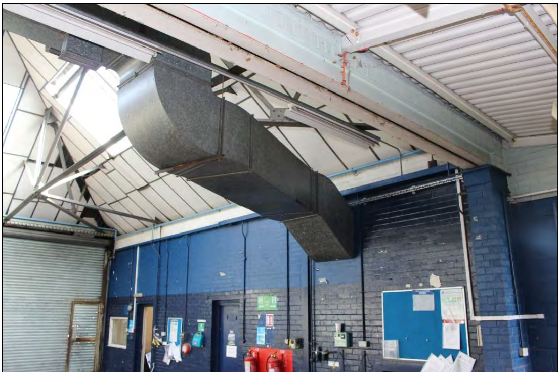
Photo 70: Detail of extraction plant in Room D1, looking north-east
