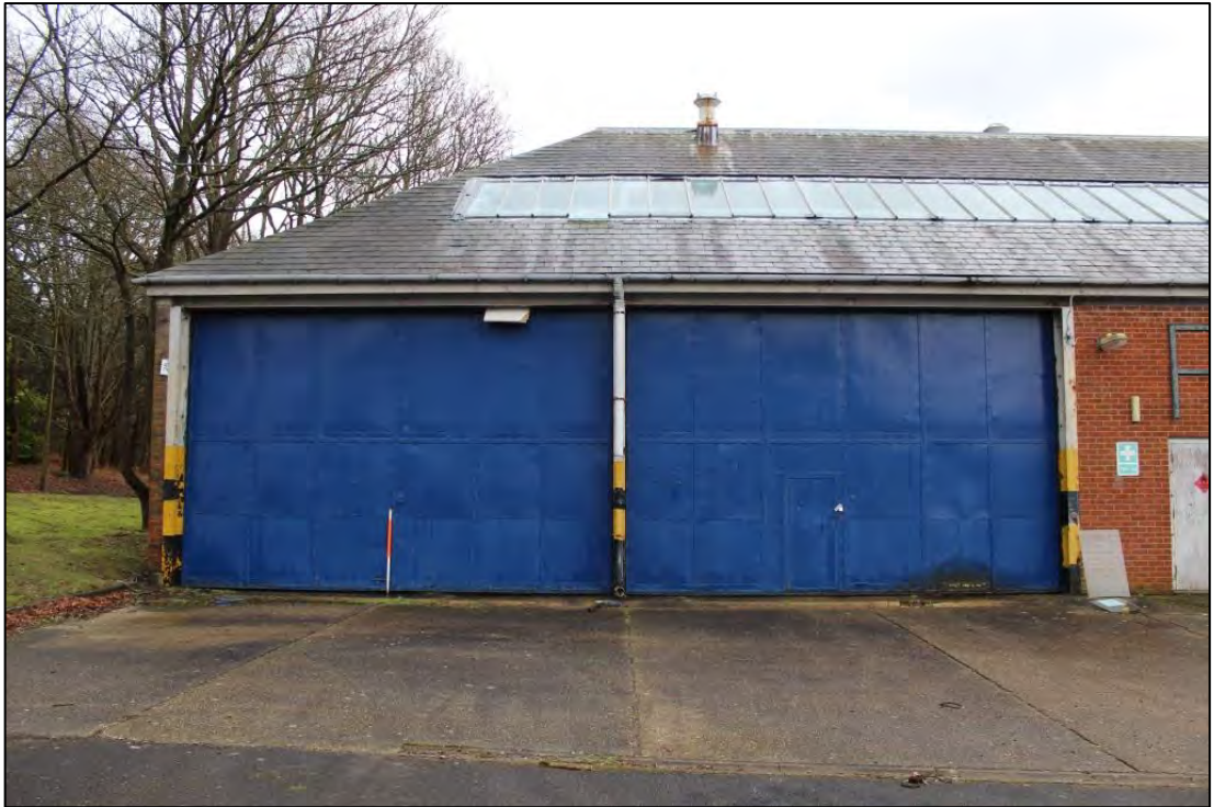
Photo 93: Building A, West elevation 1
