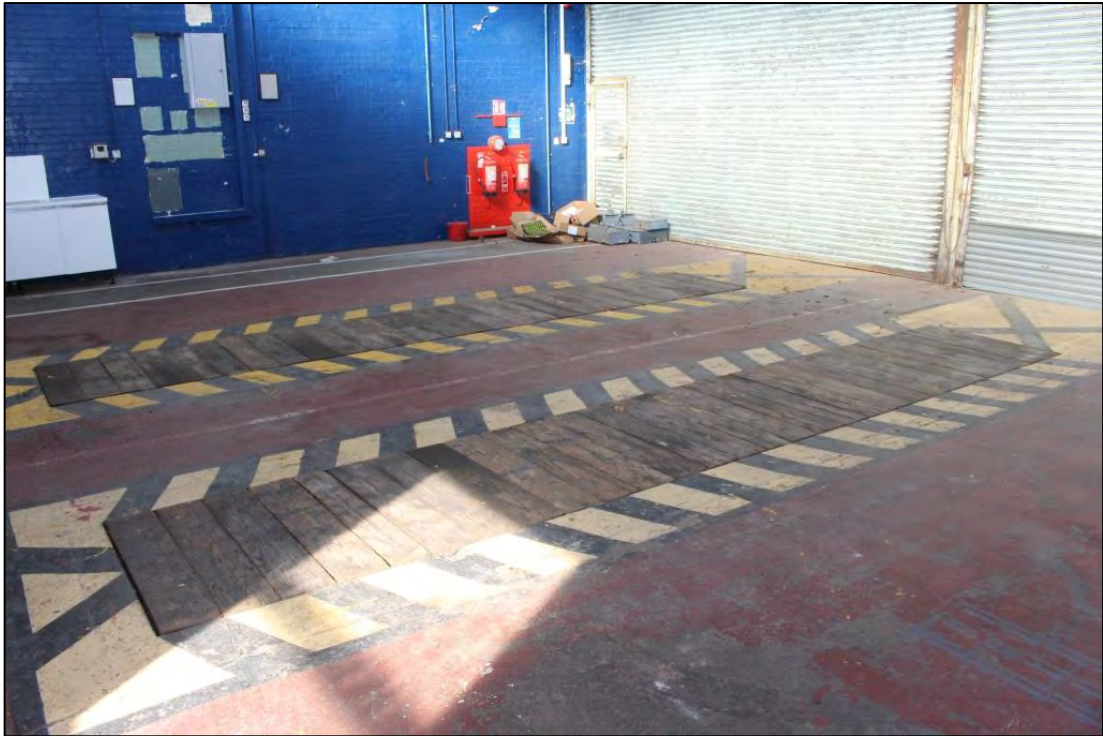
Photo 69: Overview of vehicle inspection pits in Room D1, looking north-west
