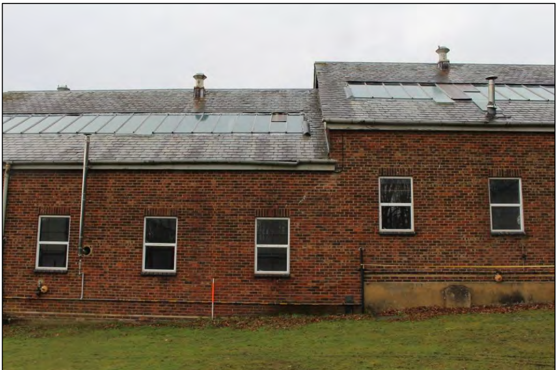
Photo 90: Building A, East elevation 2
