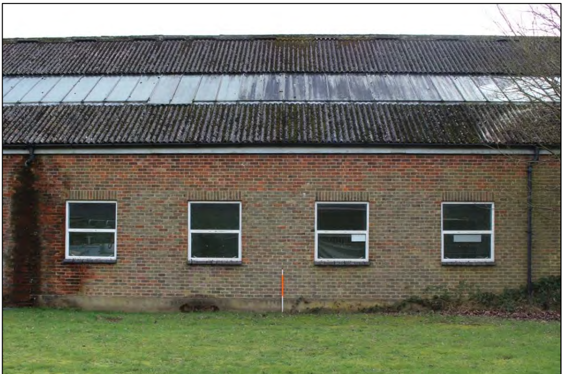
Photo 38: Overview of fenestration arrangement to northern elevation of Building C
