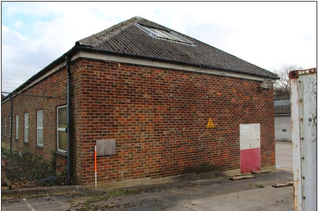
Photo 106: Building C, West elevation
