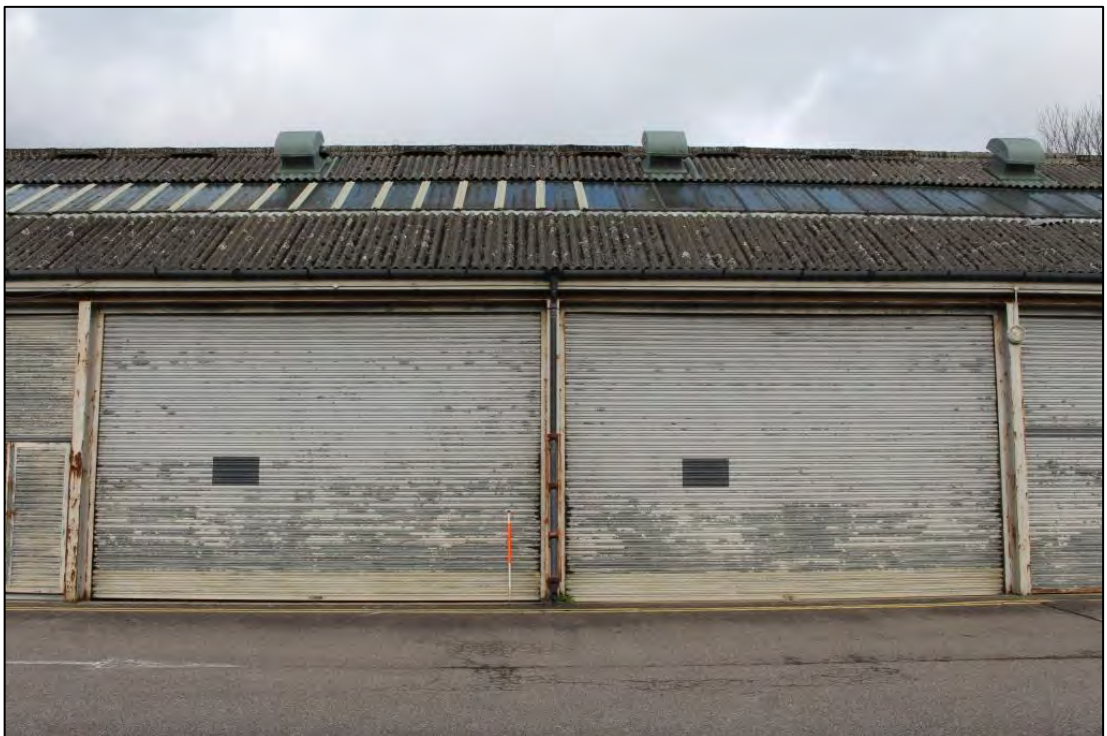
Photo 110: Building C, South elevation 4
