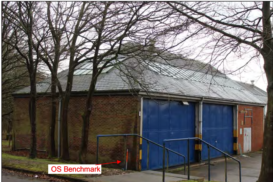
Photo 7: Northern and western elevation of Building A
