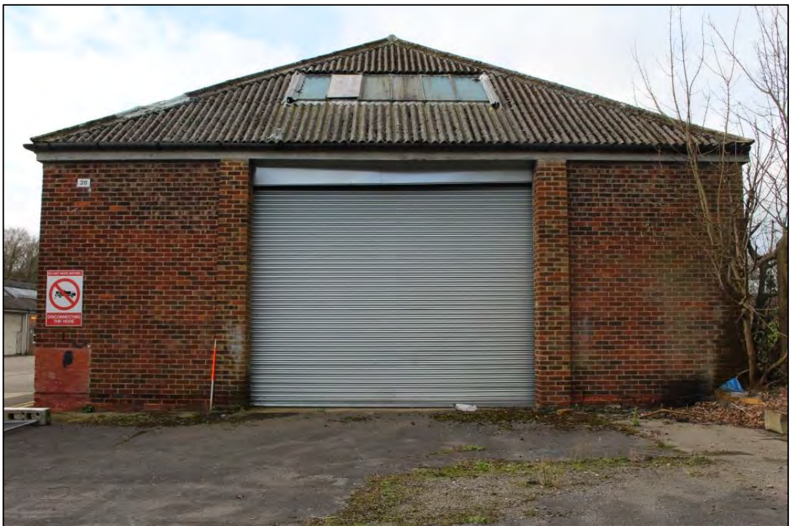
Photo 116: Building C, East elevation
