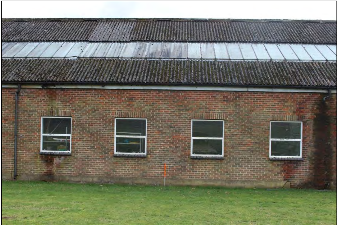
Photo 119: Building C, North elevation 3
