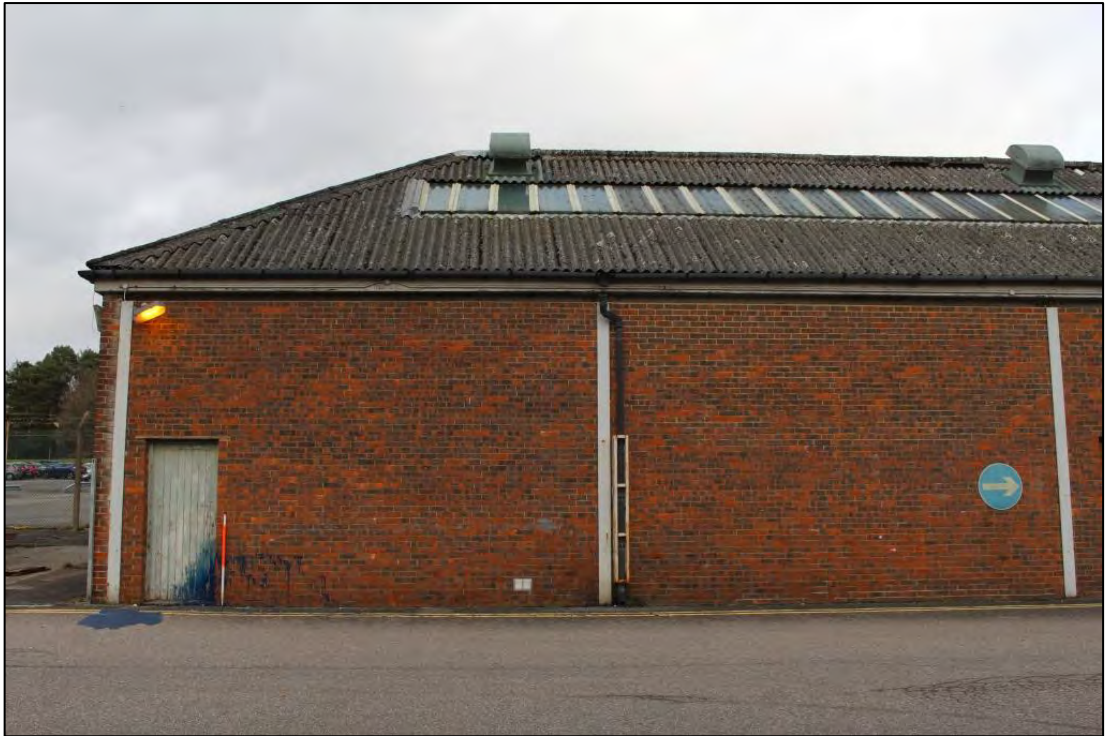
Photo 107: Building C, South elevation 1
