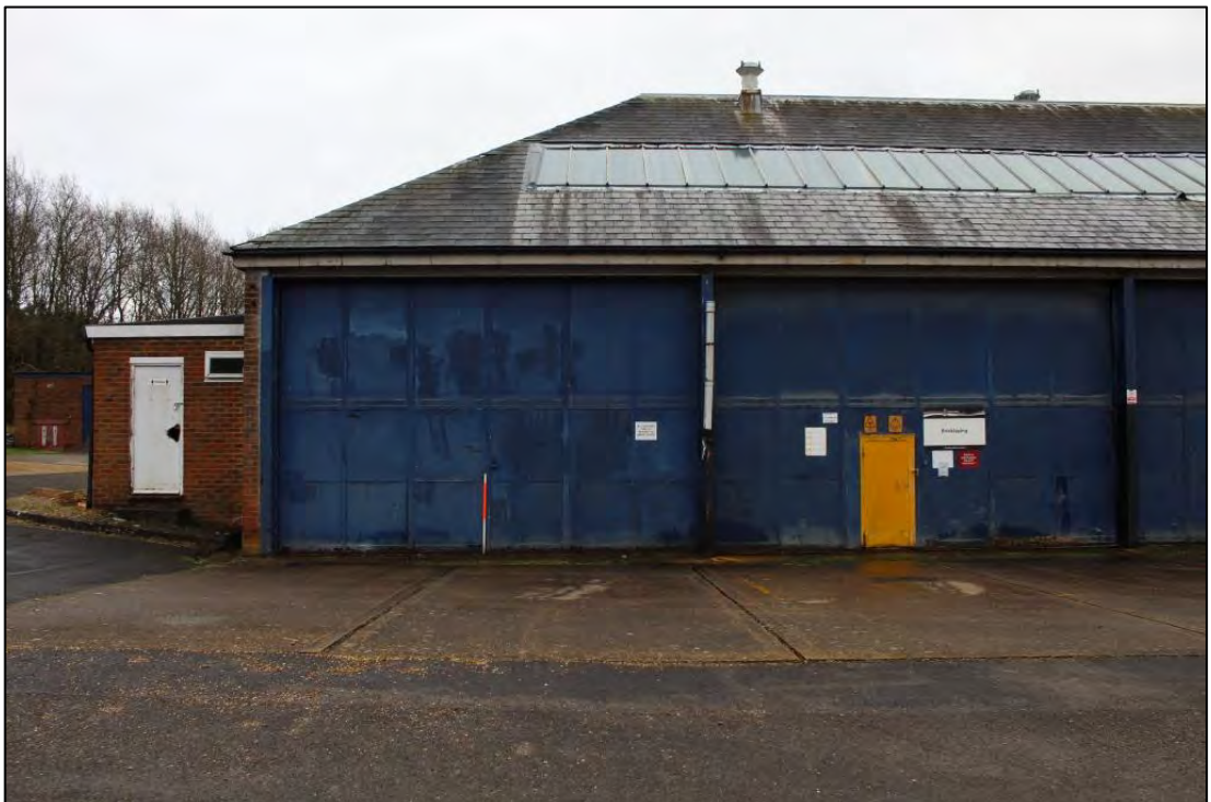
Photo 102: Building B, West elevation 1
