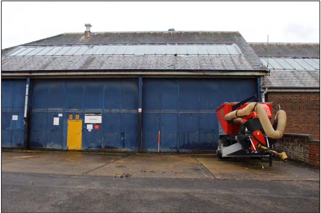
Photo 103: Building B, West elevation 2
