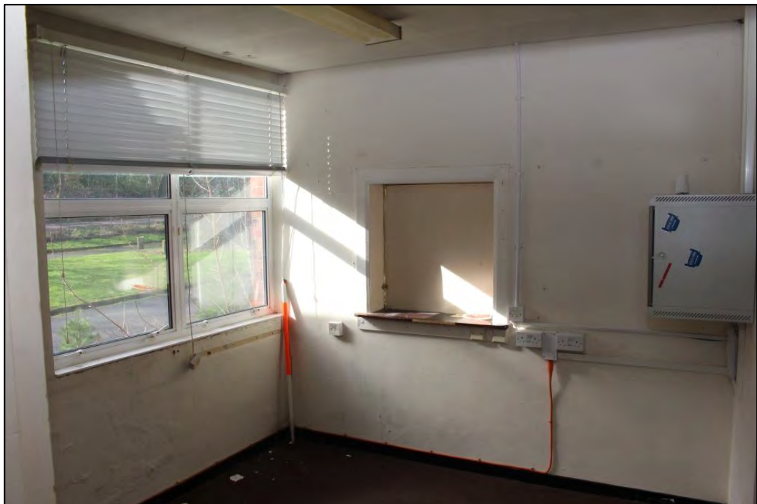
Photo 78: Overview of Room D18, incorporating blocked hatch to Room 24, looking west
