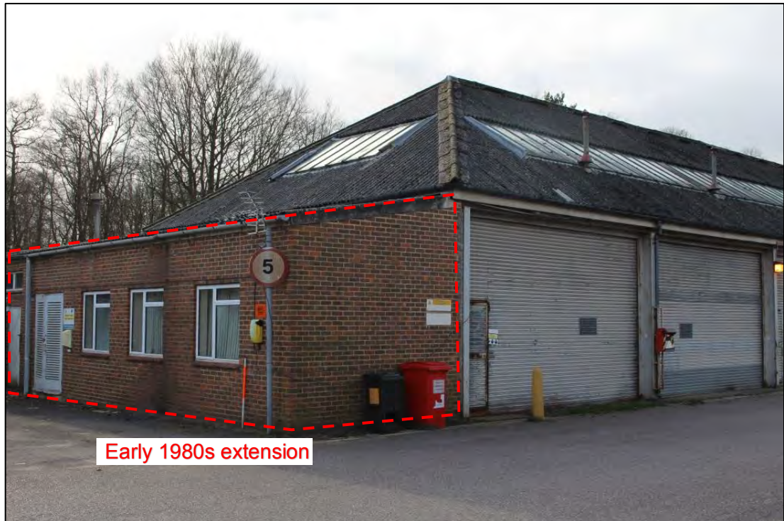
Photo 61: Eastern and northern elevations of Building D
