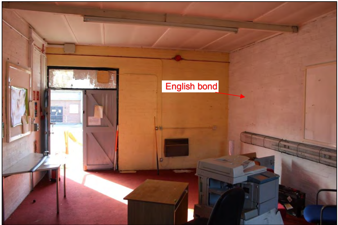
Photo 44: Overview of Room C4, looking south
