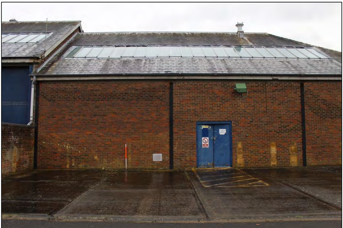
Photo 104: Building B, West elevation 3
