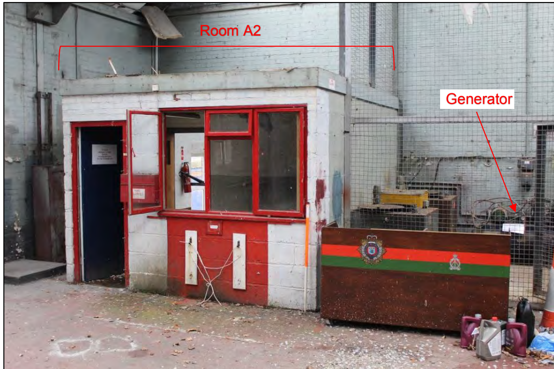
Photo 11: Overview of Room A2, looking south-east
