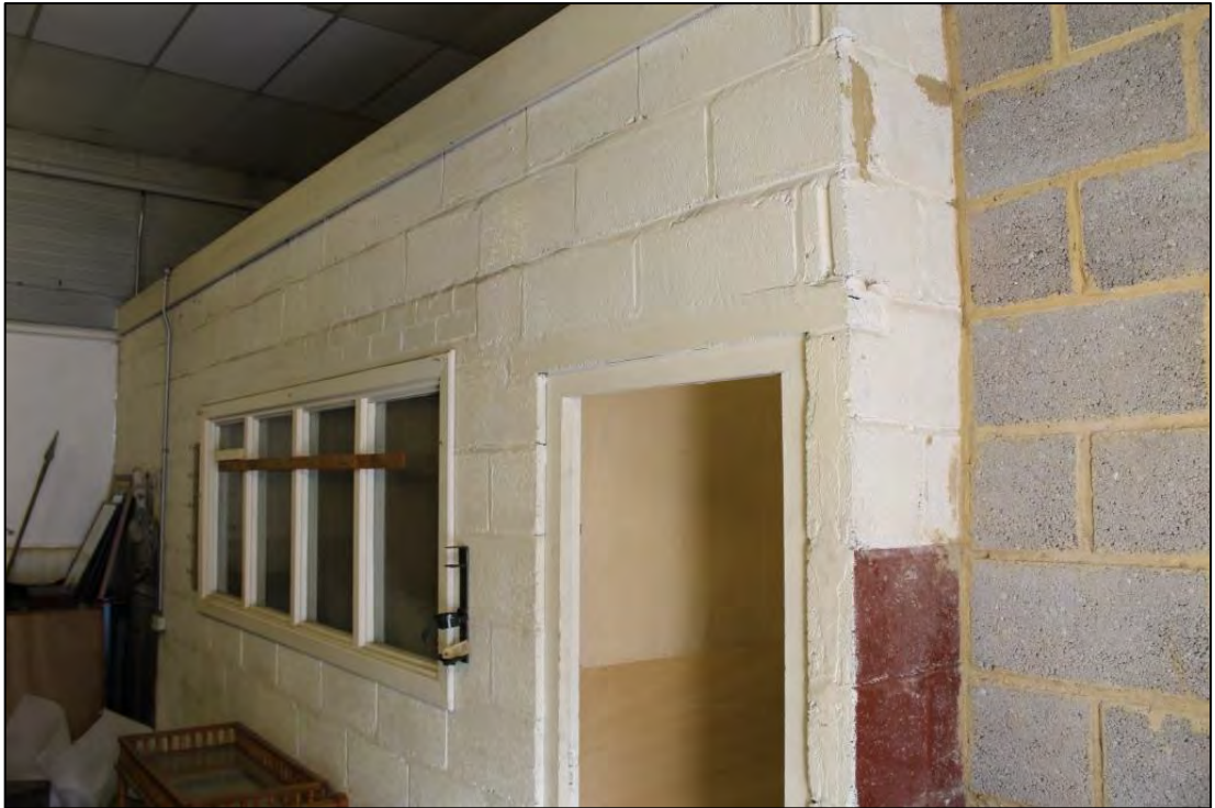
Photo 41: Overview of access to Room C2, looking north-east
