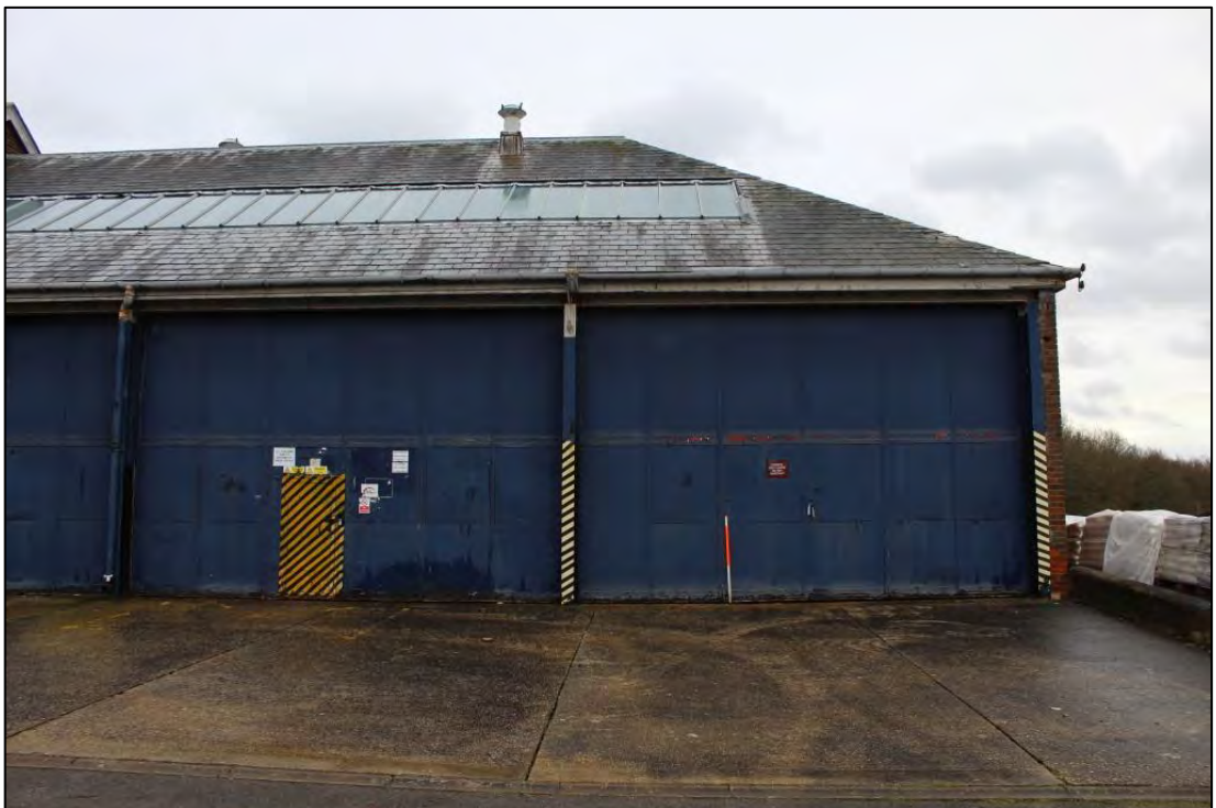
Photo 96: Building A, West elevation 4
