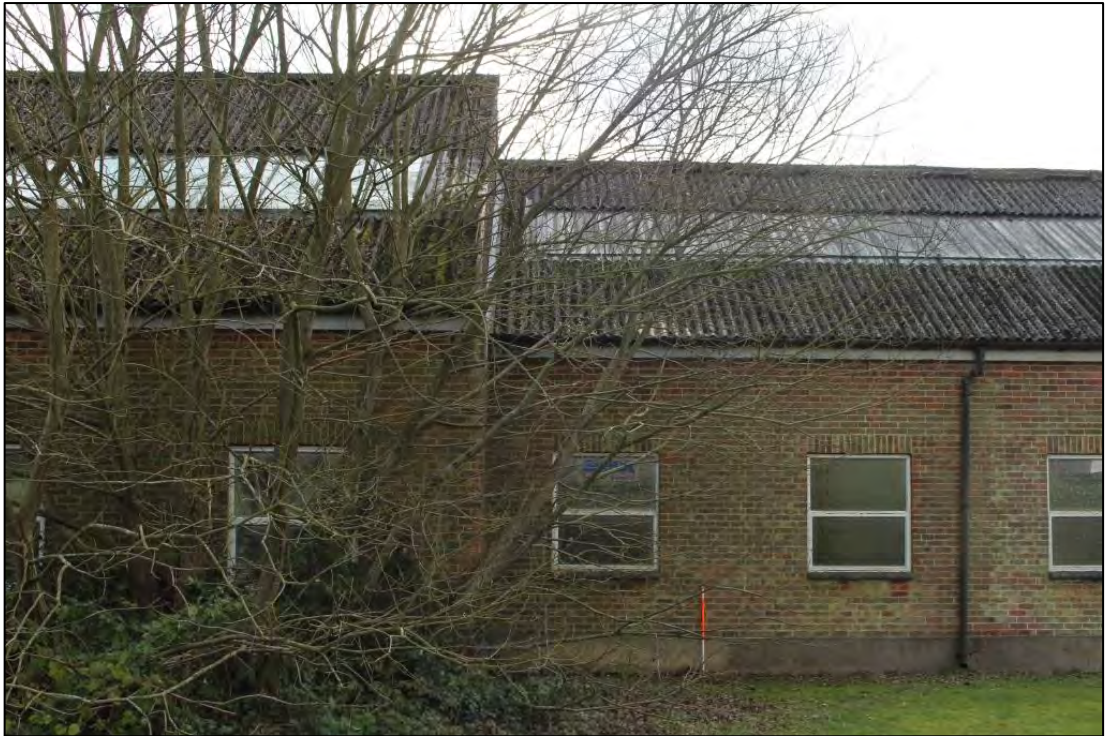
Photo 121: Building C, North elevation 5
