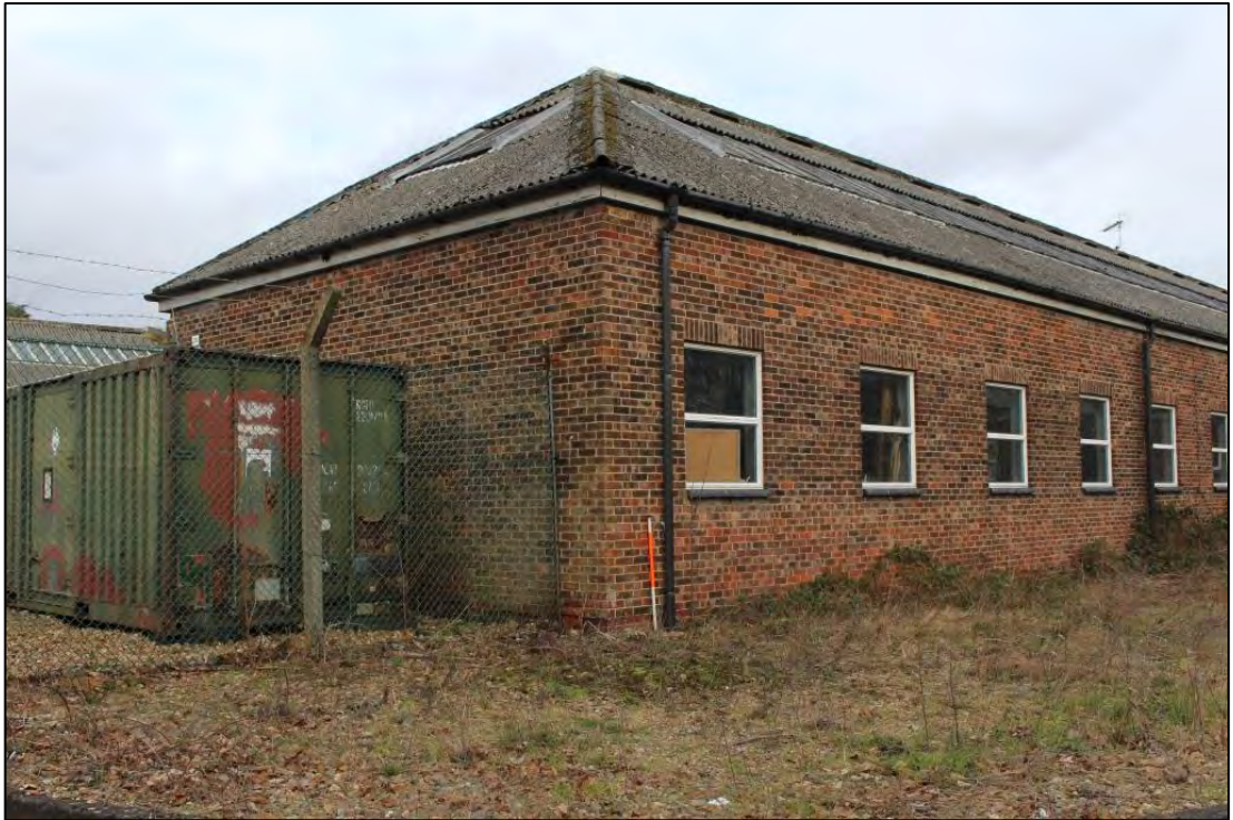
Photo 59: Western and southern elevations of Building D
