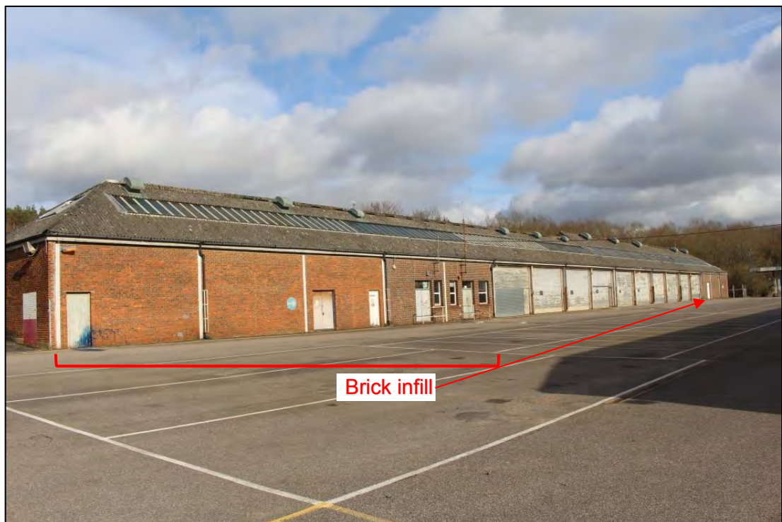
Photo 31: Overview of Building C, looking north-east
