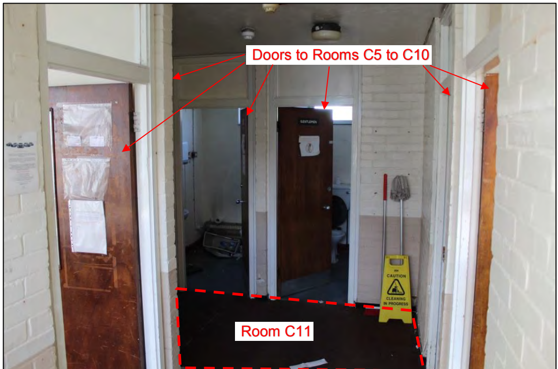
Photo 45: Overview of Room C11, looking north
