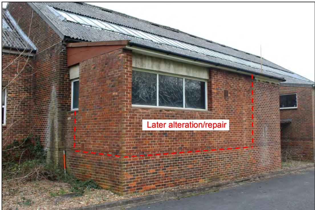
Photo 63: Overview of extension to southern elevation, looking north-east
