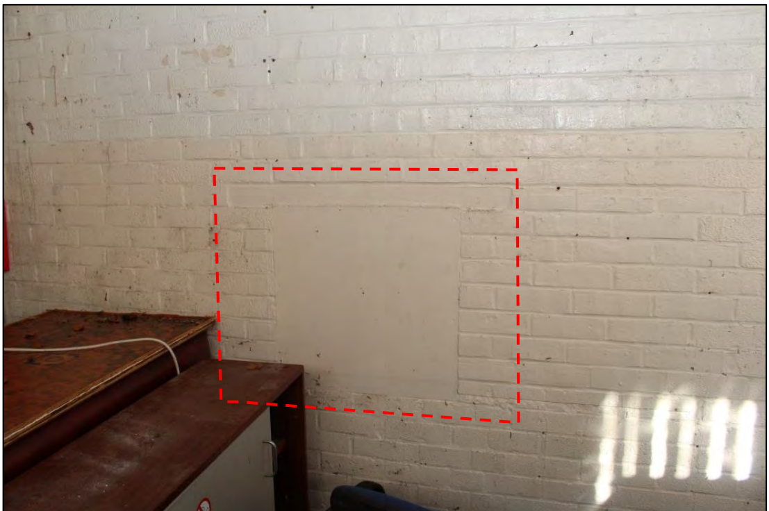
Photo 74: Detail of blocked aperture in Room D7, looking north
