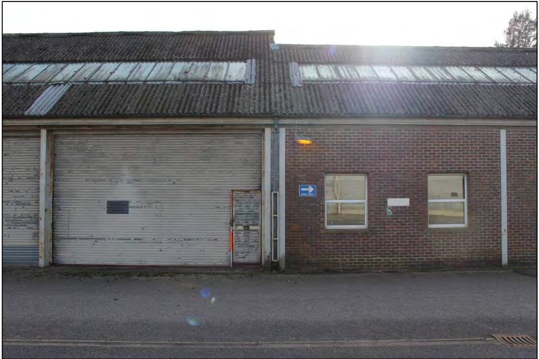
Photo 139: Building D, North elevation 3
