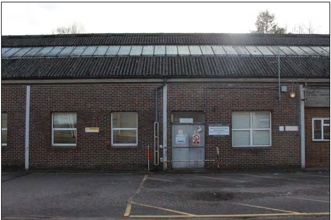
Photo 140: Building D, North elevation 4
