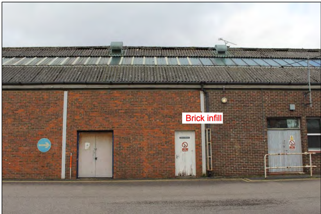
Photo 36: Detail of infilled bays within southern elevation of Building C
