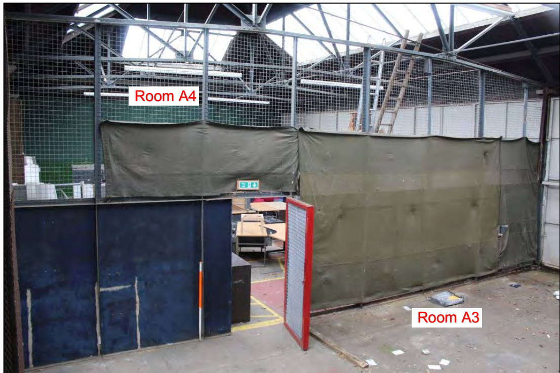
Photo 14: Metal mesh partition between Rooms A3 and A4, looking south-west
