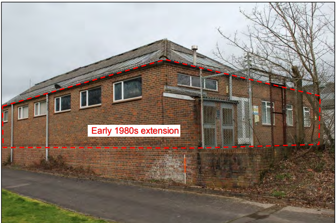
Photo 60: Southern and eastern elevations of Building D
