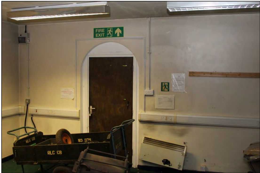
Photo 84: Arch-headed door to eastern extent of Room 30, looking east
