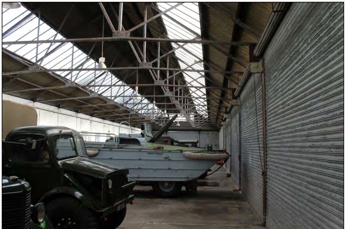
Photo 52: Overview of Room C14, looking east
