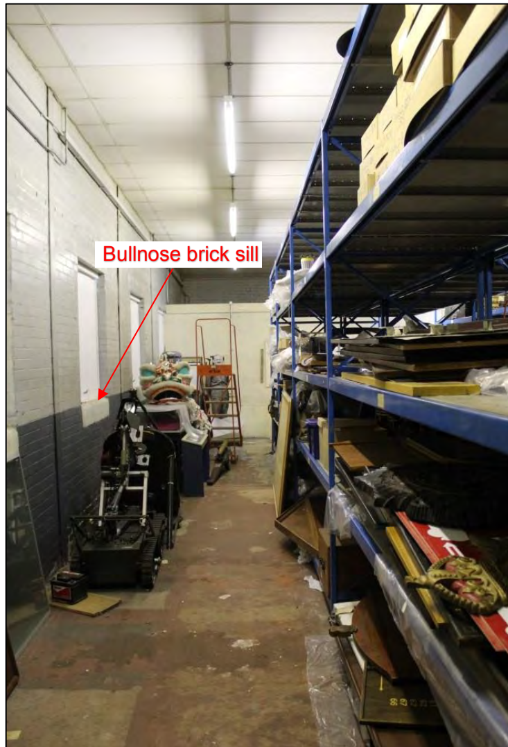
Photo 39: Overview of Room C1, looking east
