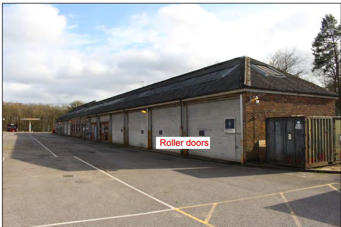
Photo 58: Overview of Building D, looking south-east
