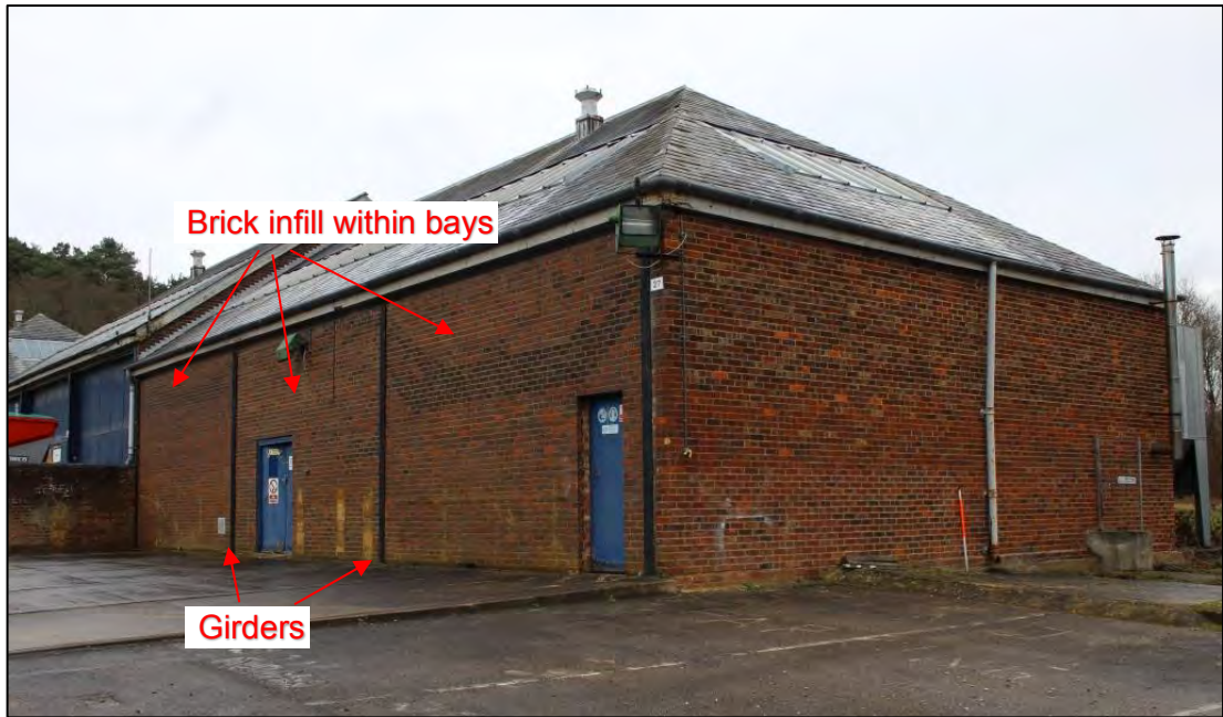
Photo 17: Western and southern elevations of Building B, looking north-east
