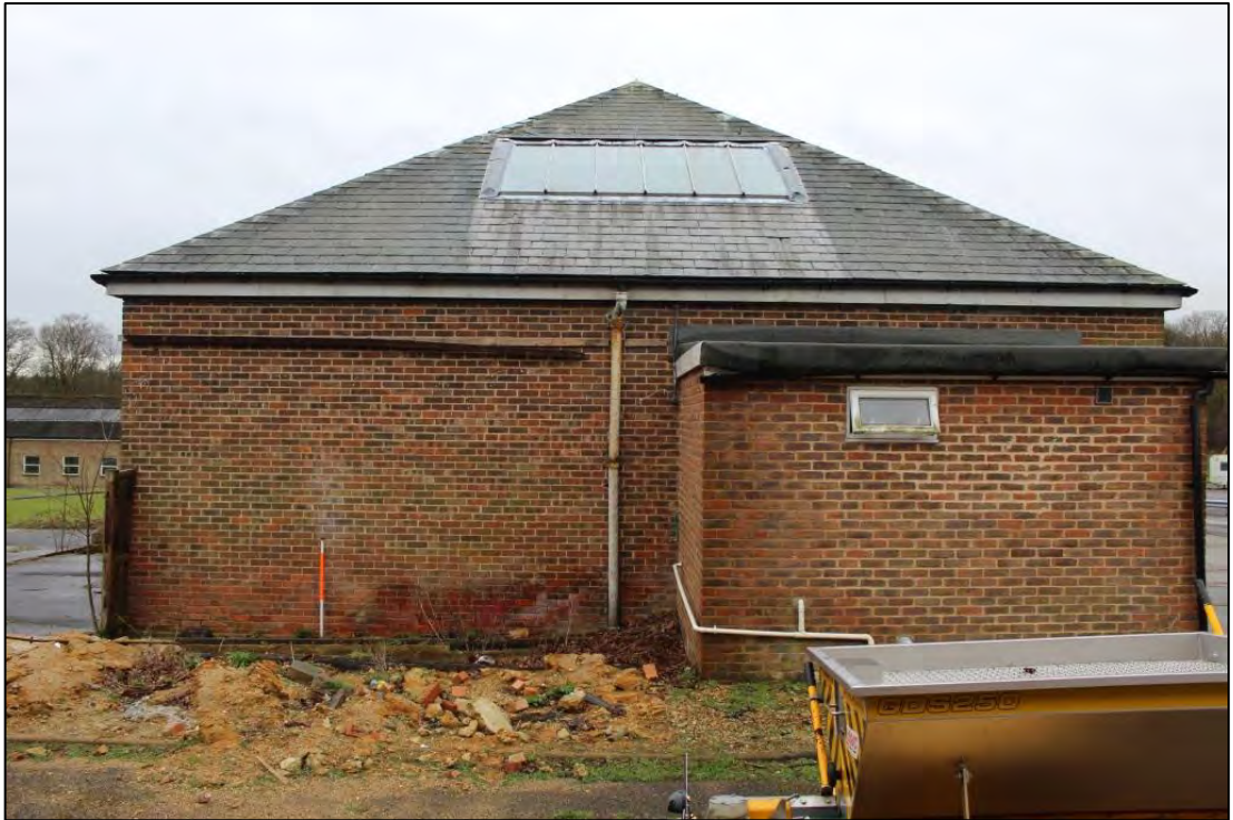
Photo 101: Building B, North elevation
