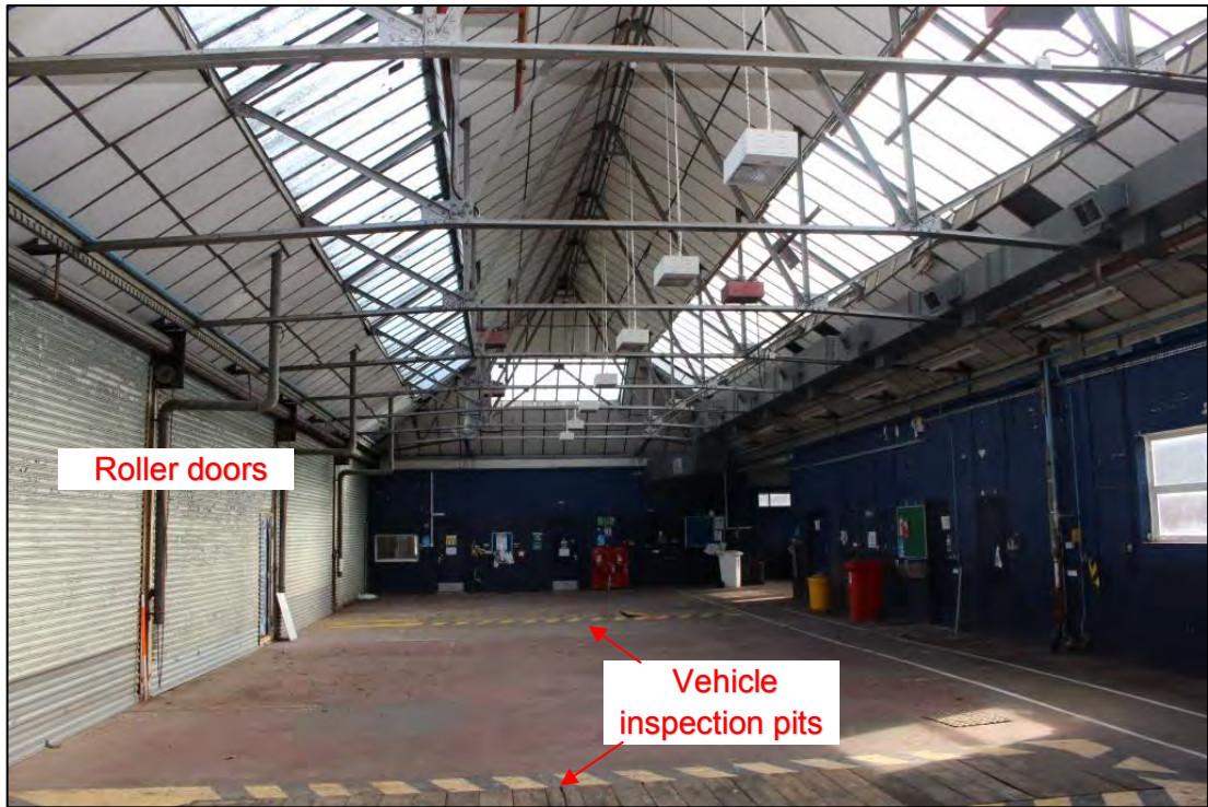
Photo 67: Overview of Room D1, looking east
