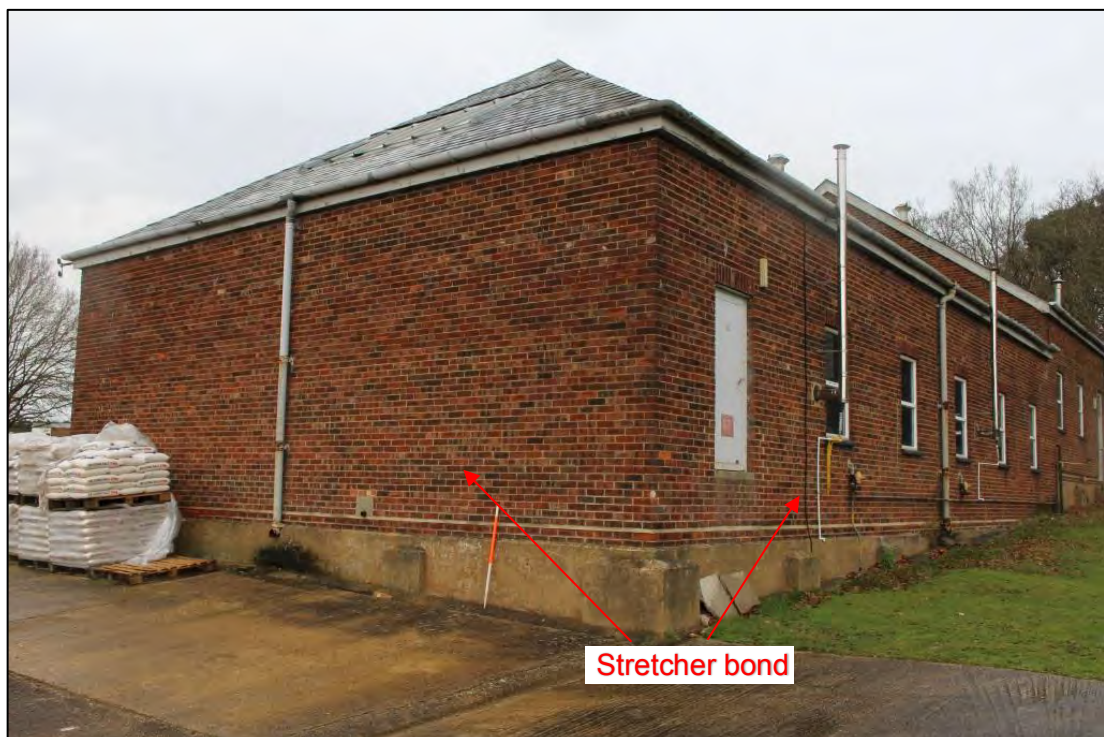
Photo 4: Southern and eastern elevations of Building A
