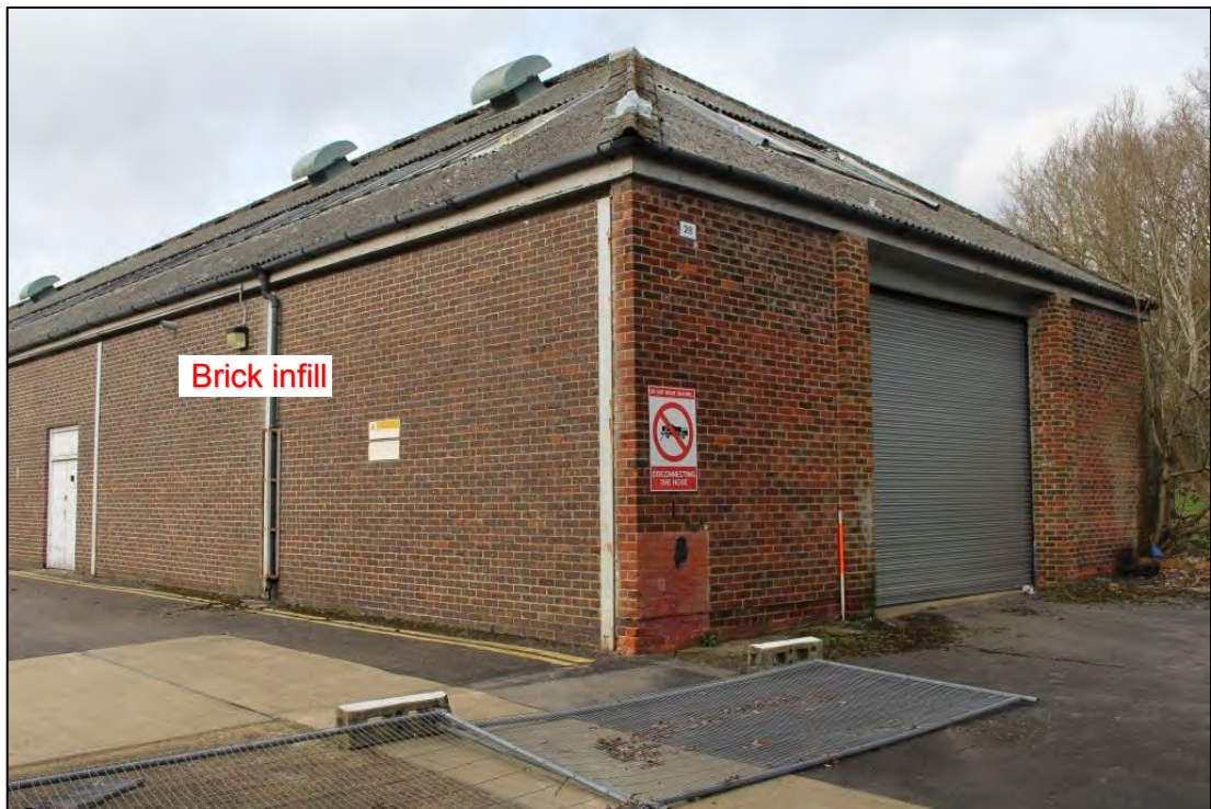
Photo 33: Eastern and southern elevations of Building C
