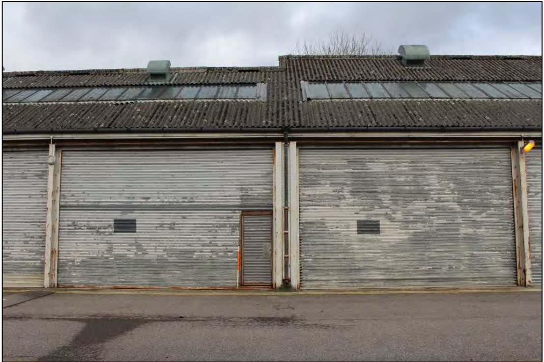
Photo 111: Building C, South elevation 5
