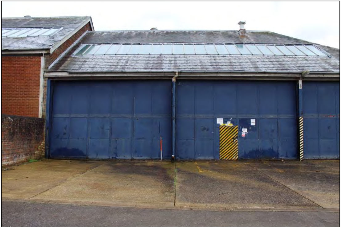
Photo 95: Building A, West Elevation 3
