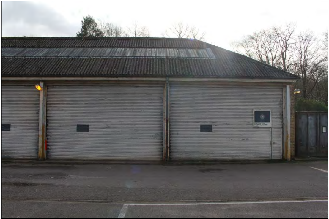
Photo 143: Building D, North elevation 7
