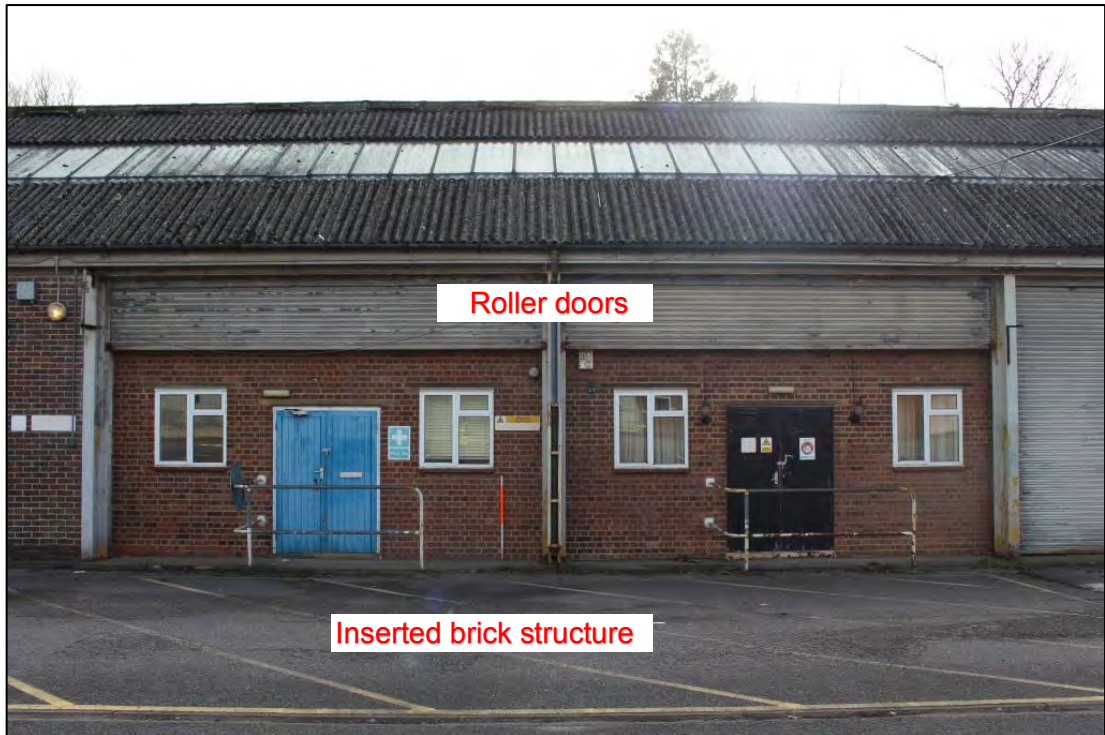
Photo 66: Overview of brick structure within Building D
