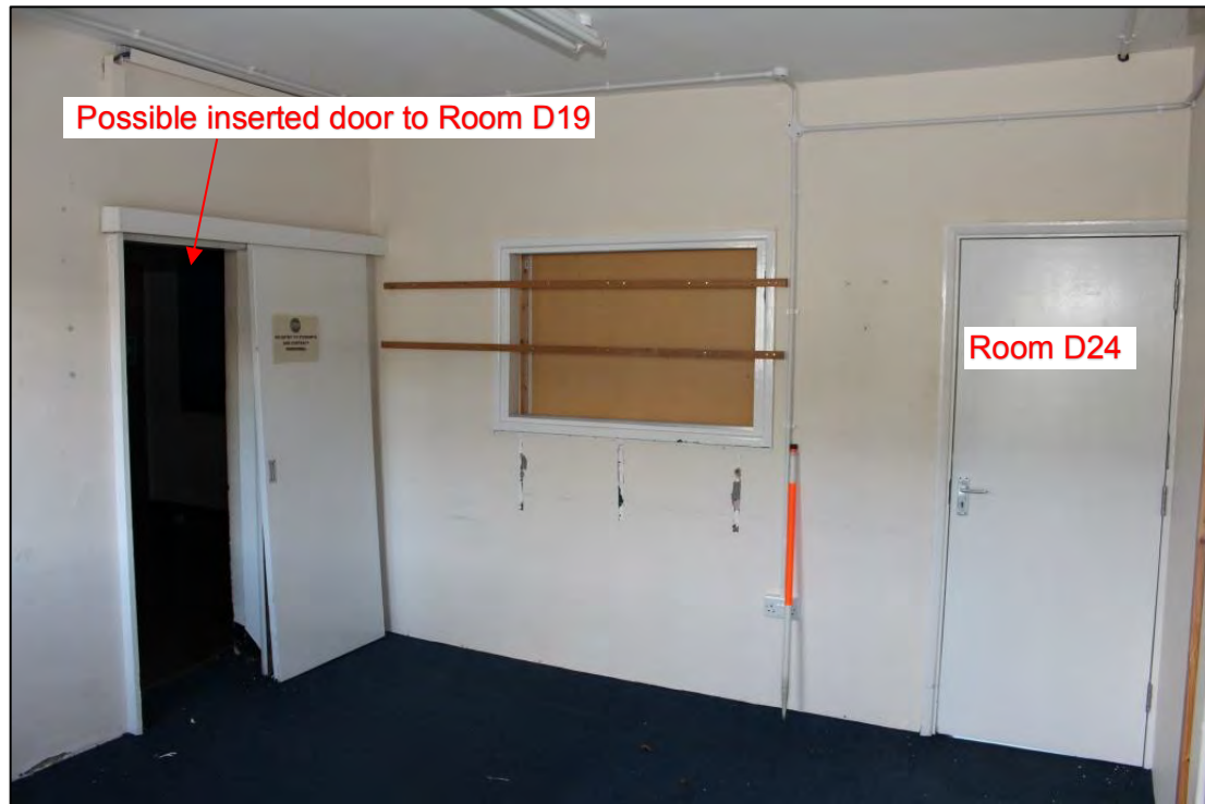
Photo 81: Overview of Room D25, looking south.
