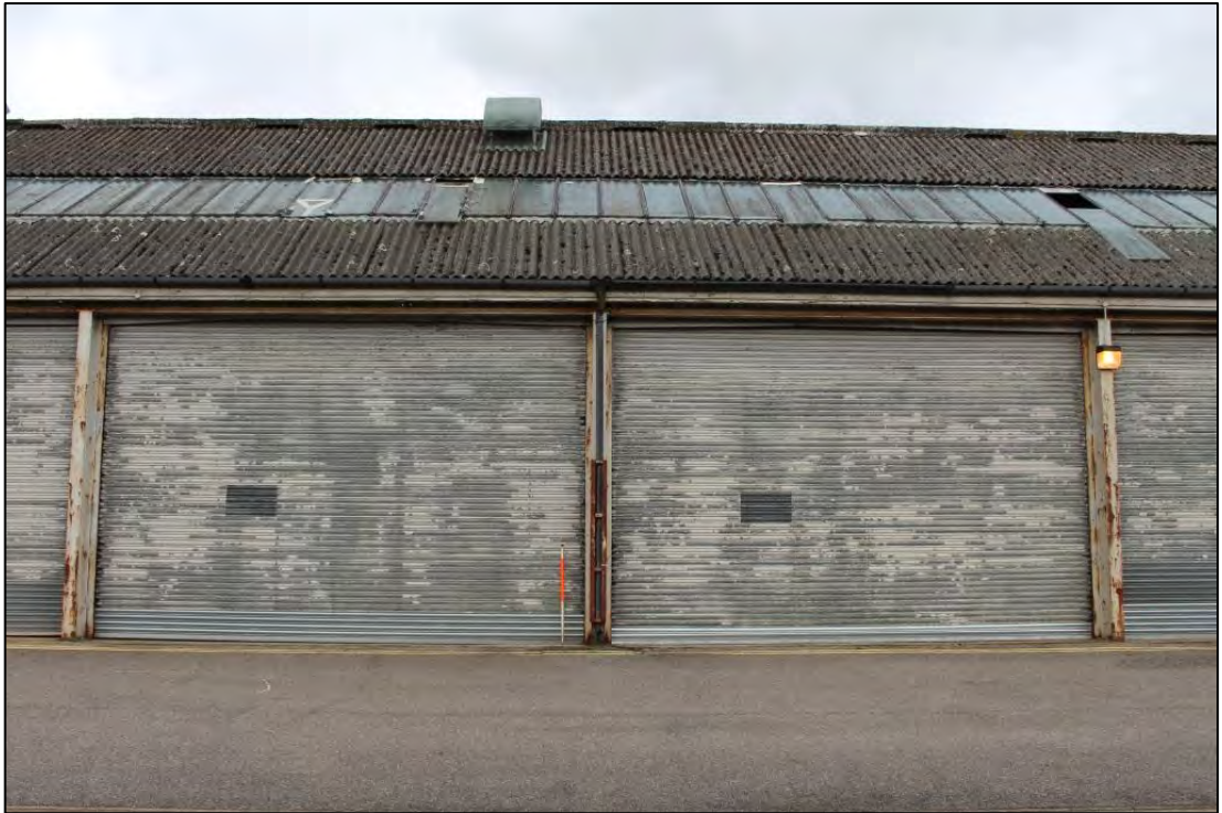
Photo 113: Building C, South elevation 7
