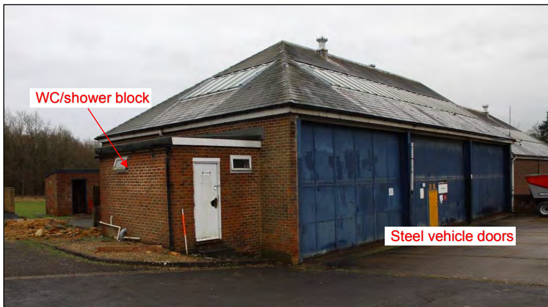
Photo 16: Northern and western elevations of Building B, looking south-east
