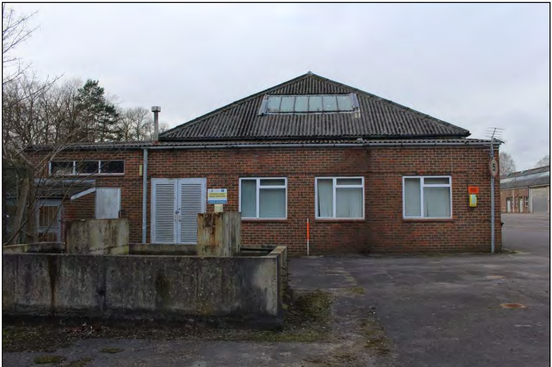
Photo 136: Building D, East elevation
