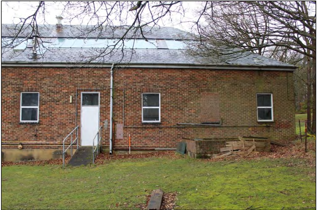
Photo 91: Building A, East elevation 3
