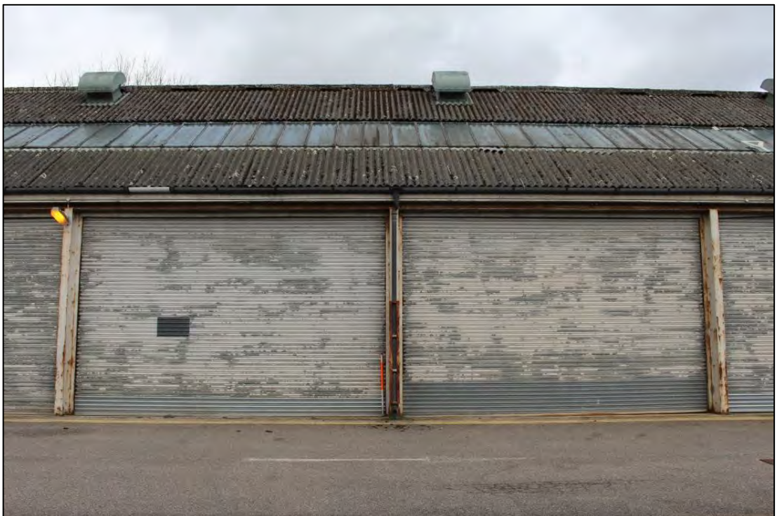
Photo 112: Building C, South Elevation 6
