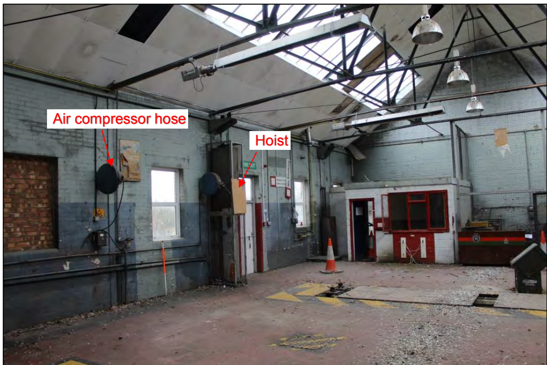
Photo 9: Overview of Room 8, looking south-east
