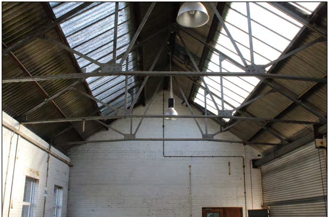
Photo 49: Overview of Room C13, looking east
