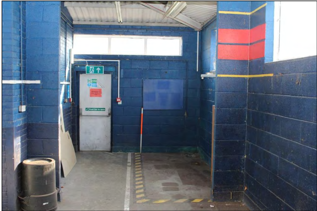
Photo 71: Overview of south-eastern extent of Room D1, looking east
