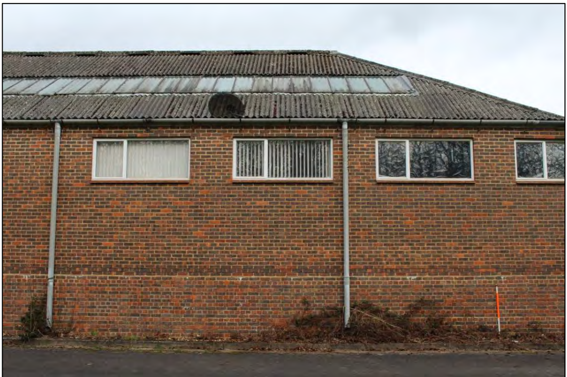
Photo 134: Building D, South elevation 8
