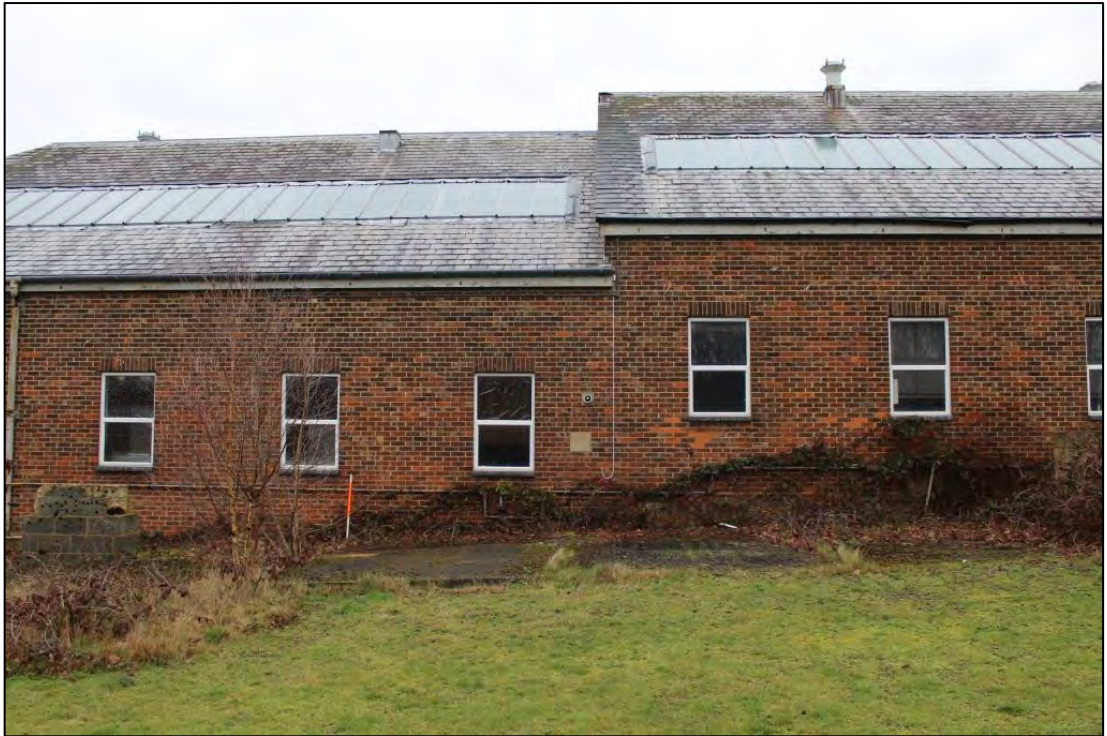
Photo 99: Building B, East elevation 2
