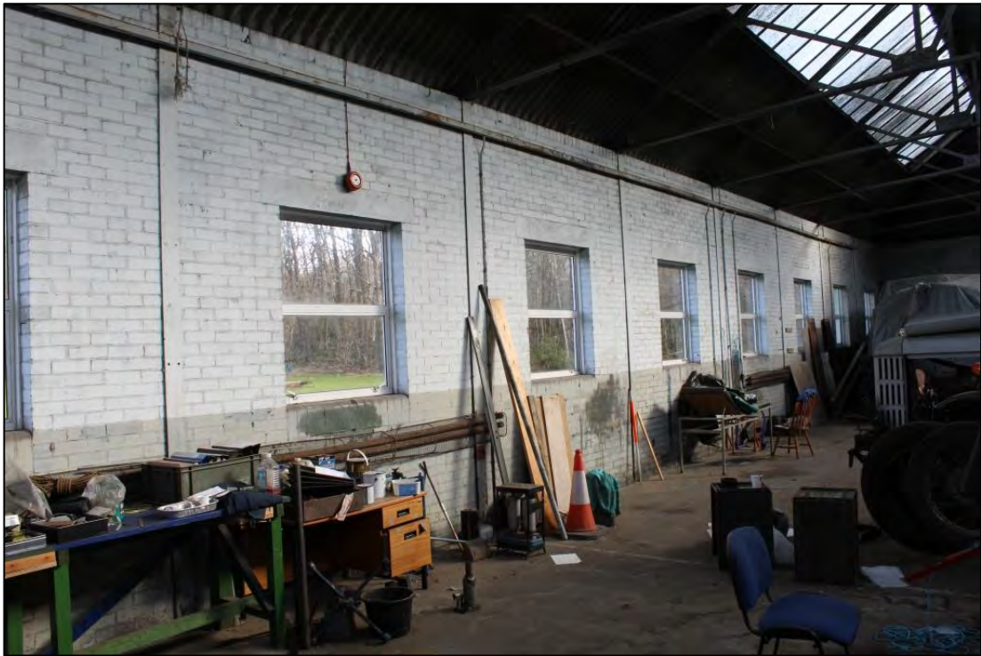
Photo 55: Window arrangement within northern wall of Room C14, looking north-east
