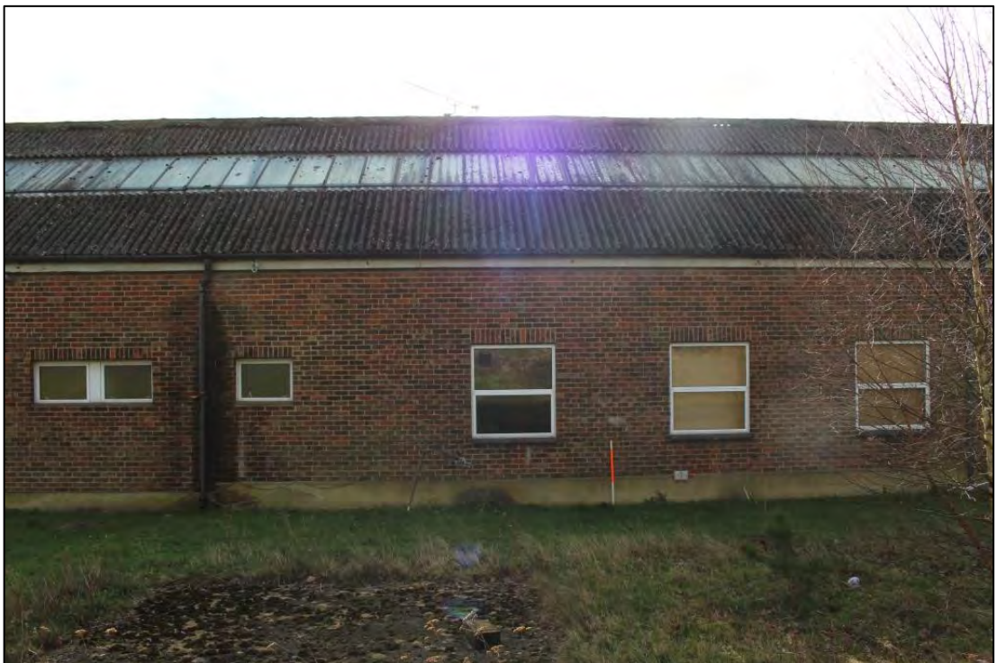
Photo 124: Building C, North elevation 8
