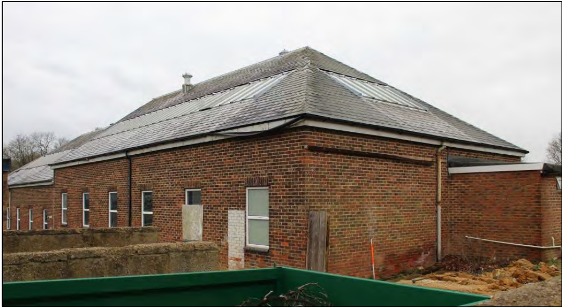
Photo 19: Western and northern elevation of Building B
