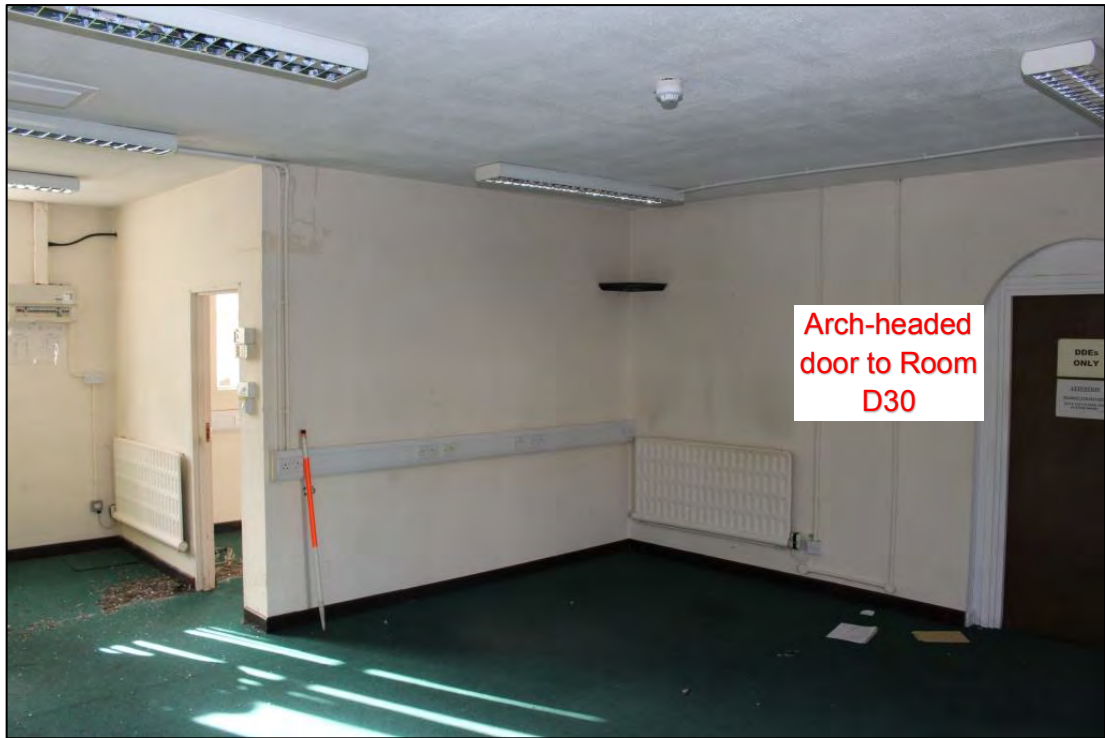
Photo 82: Overview of Room D27, looking south-west
