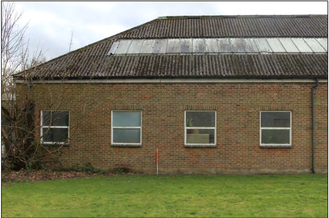
Photo 117: Building C, North elevation 1
