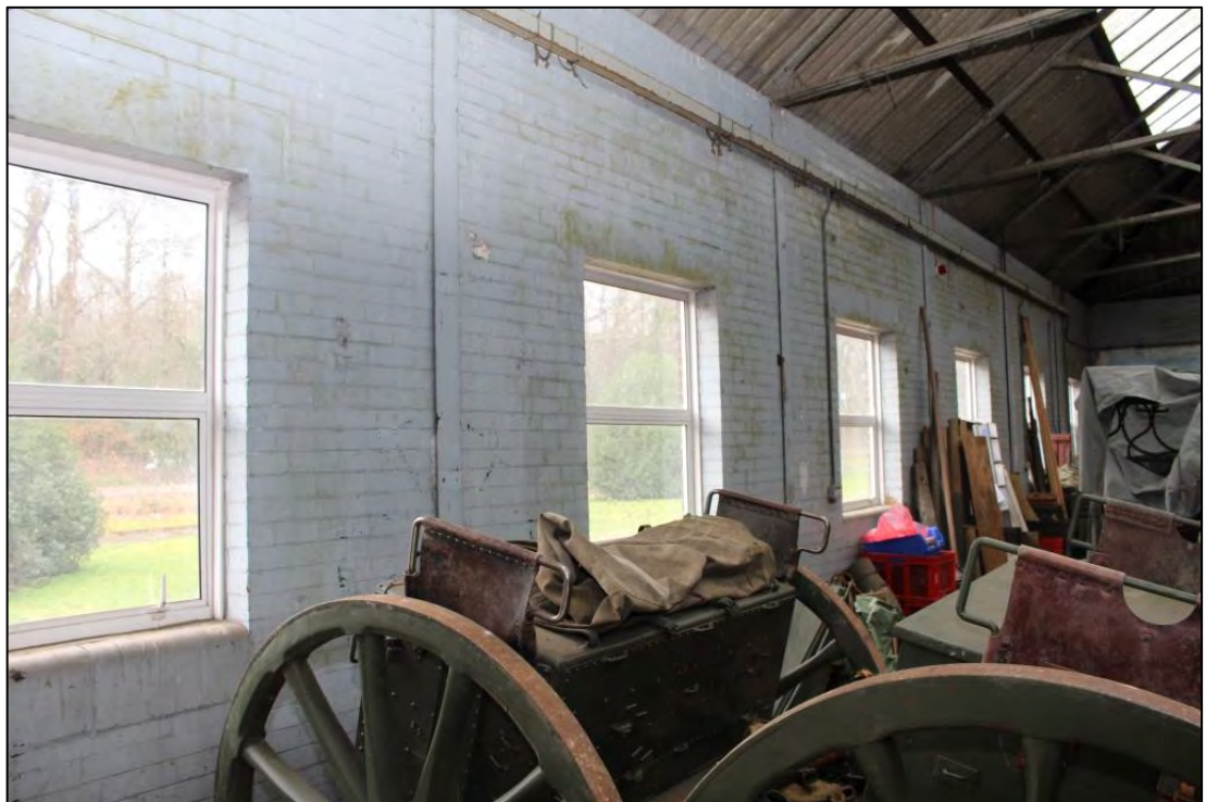
Photo 86: Overview of southern wall of Room D31, looking south-west
