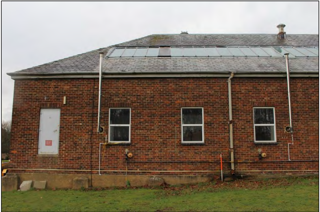
Photo 89: Building A, East elevation 1
