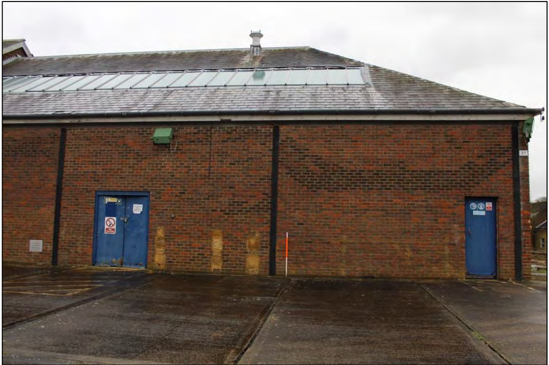
Photo 105: Building B, West elevation 4
