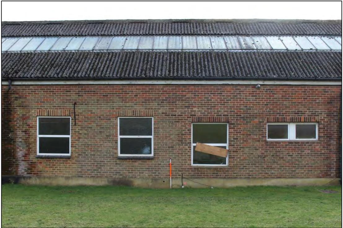
Photo 123: Building C, North elevation 7
