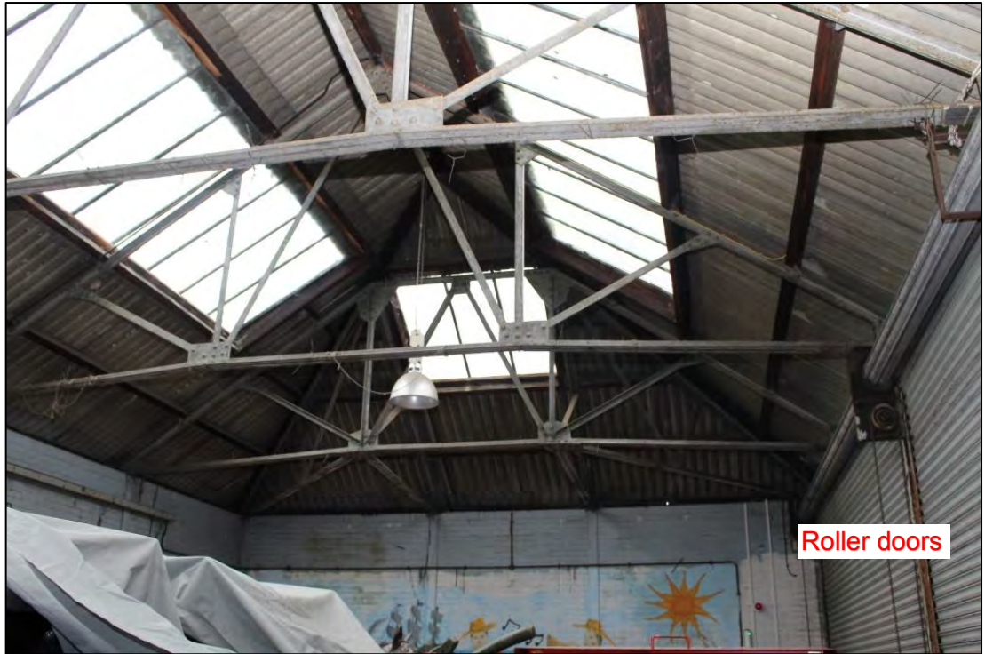
Photo 85: Overview of Room D31, looking west
