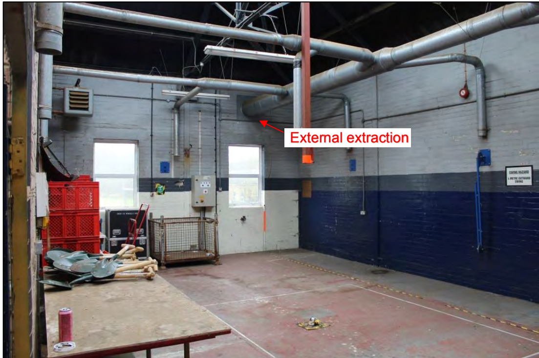
Photo 29: Overview of Room B8, looking south-east
