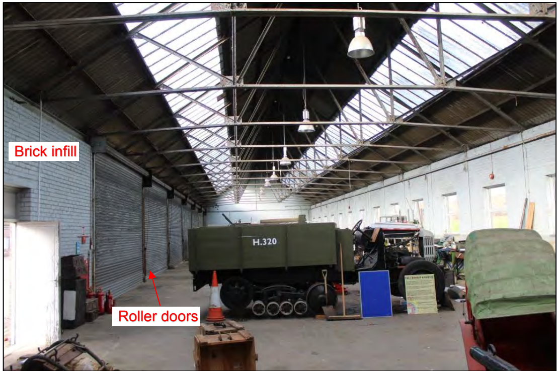
Photo 51: Overview of Room C14, looking west
