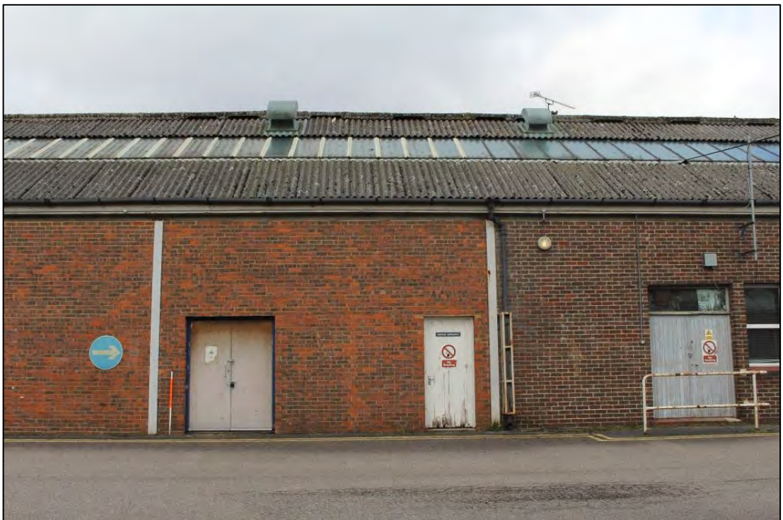
Photo 108: Building C, South elevation 2
