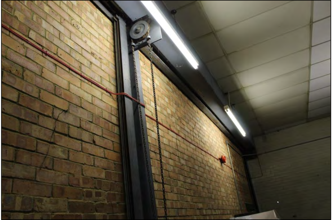
Photo 40: Pulley mechanism and brick infill within southern wall of Room C1
