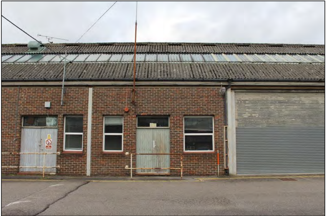
Photo 109: Building C, South elevation 3
