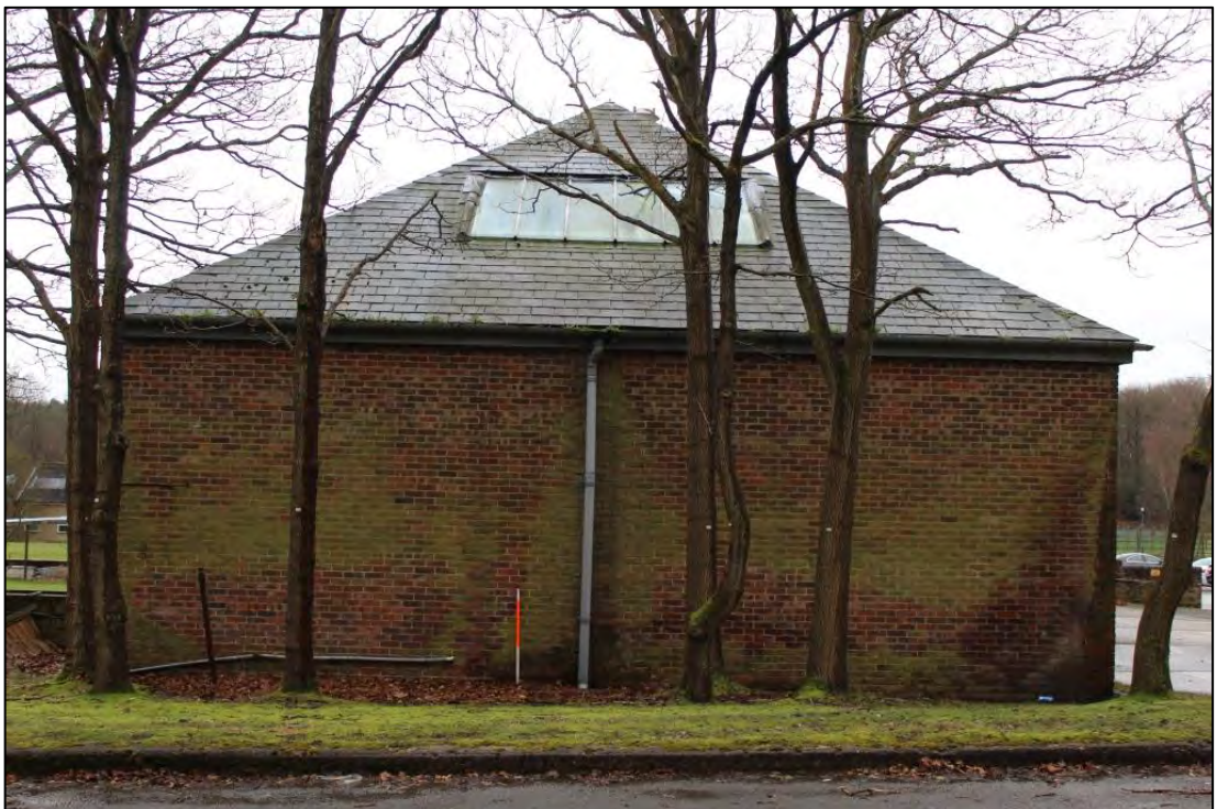
Photo 92: Building A, North elevation
