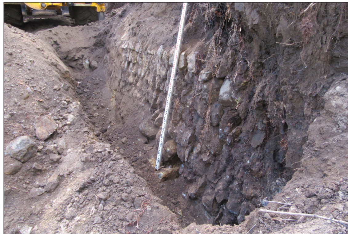
Wall 1802, looking north-east
