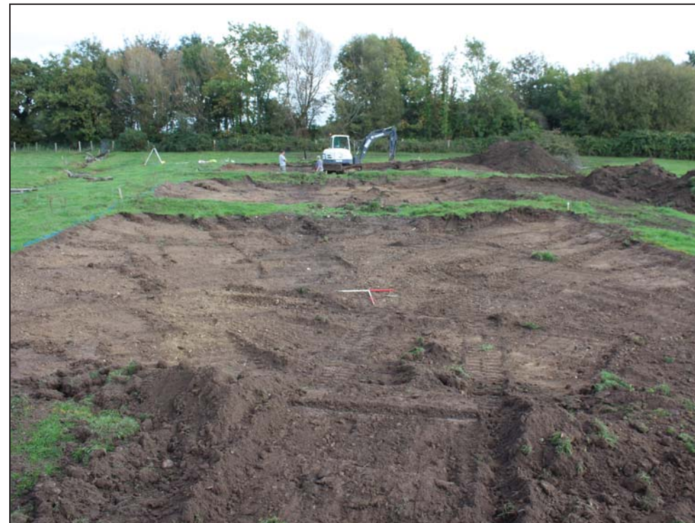
Basal channel 'drain' (103) of water meadow earthwork, looking south-west (1m scales)
