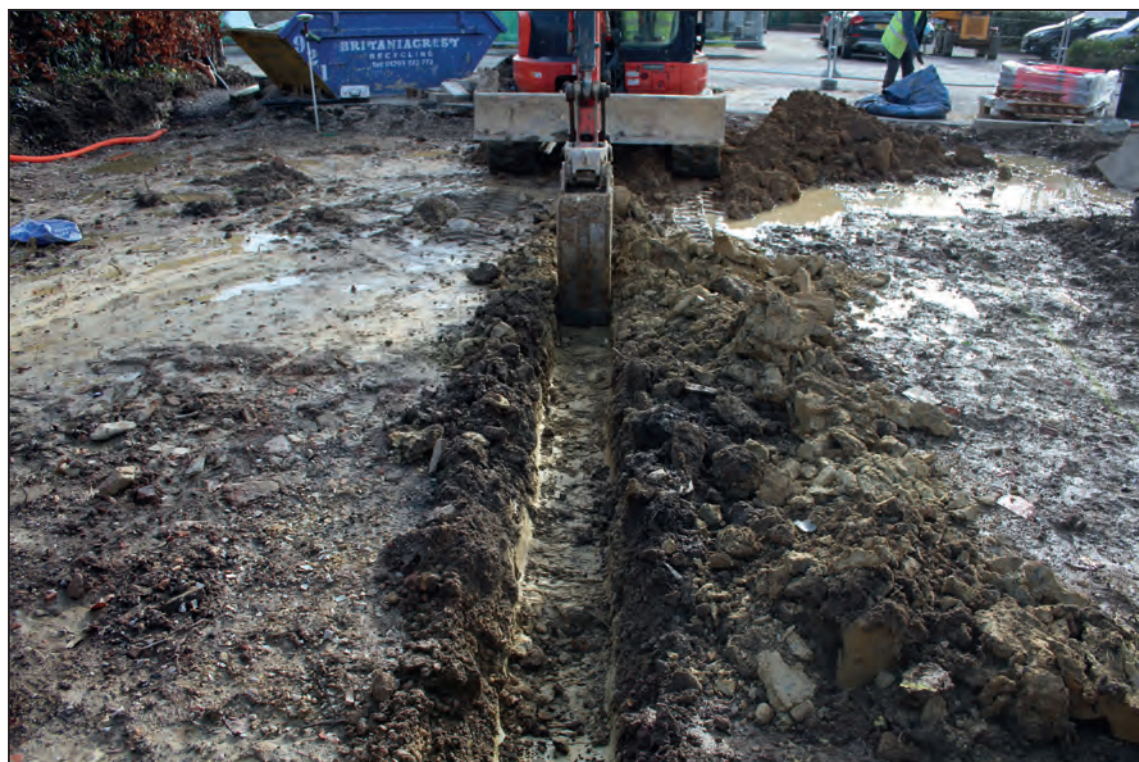
Trench 3 working shot
