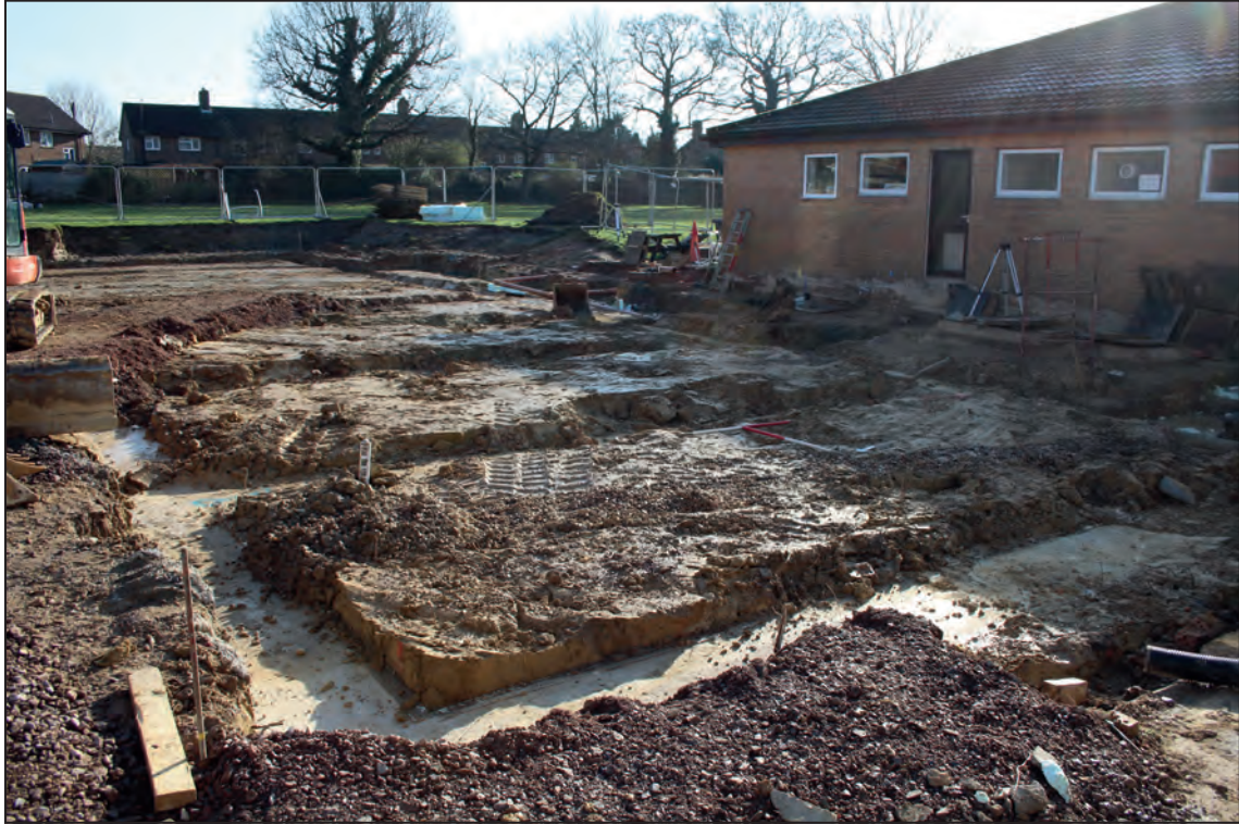
Trench 2 working shot, looking south-east (1m scales)
