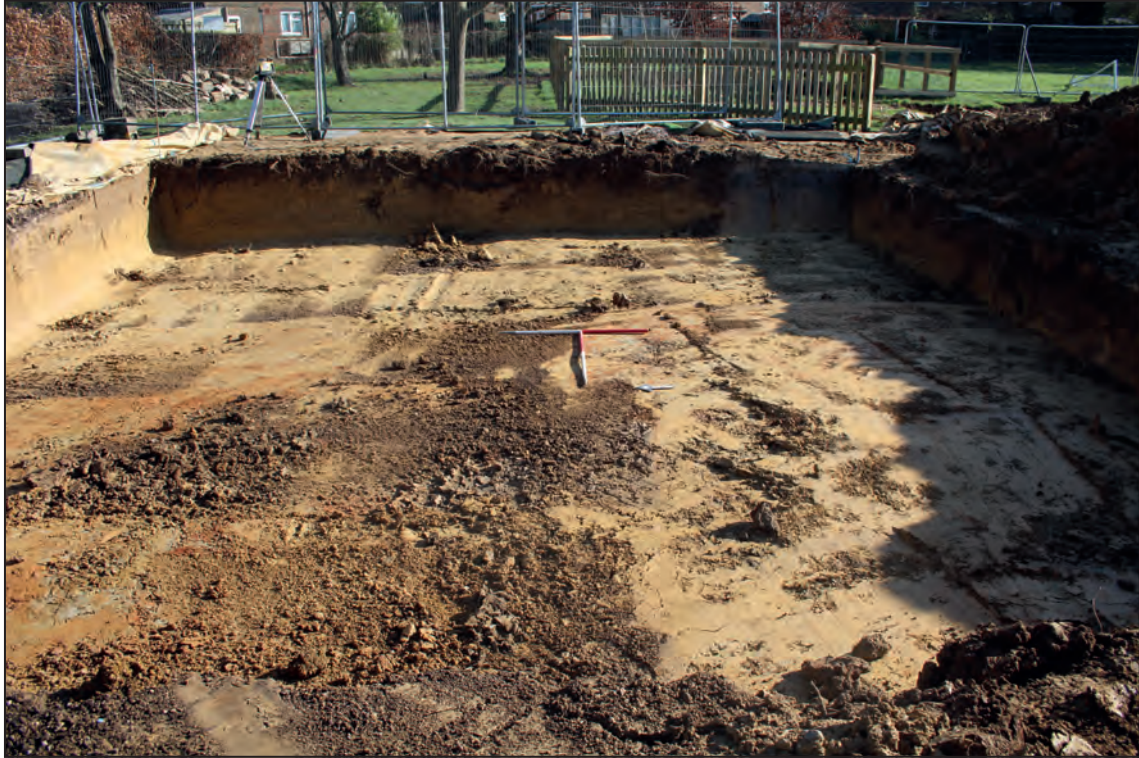
Trench 4 post-excavation, looking east (1m scales)
