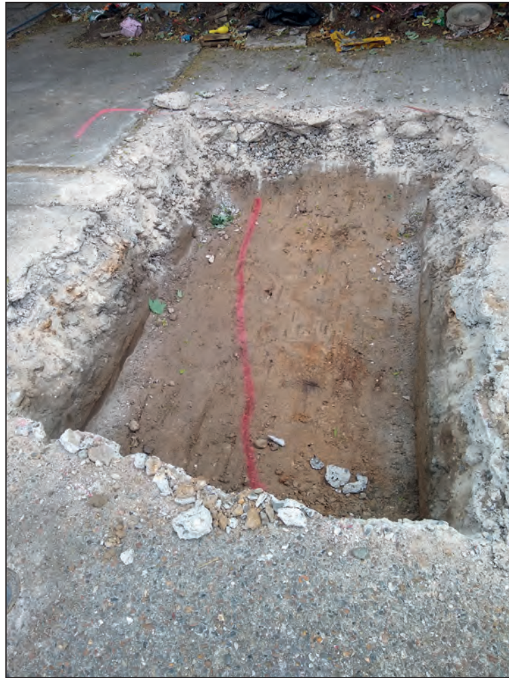
Trench 2A pre-excavation, looking south
