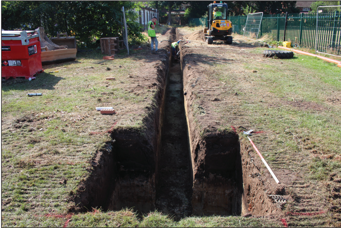
Trench 1, post-excavation, looking south-east (1m scale)
