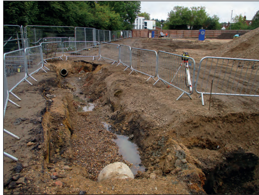
Pipe replacement: Trench 4
