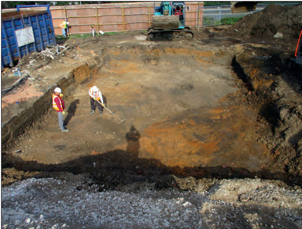
Attenuation tank in Trench 3, looking north
