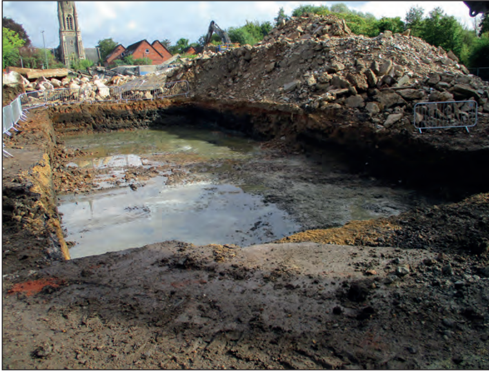
Attenuation tank in Trench 1, looking east
