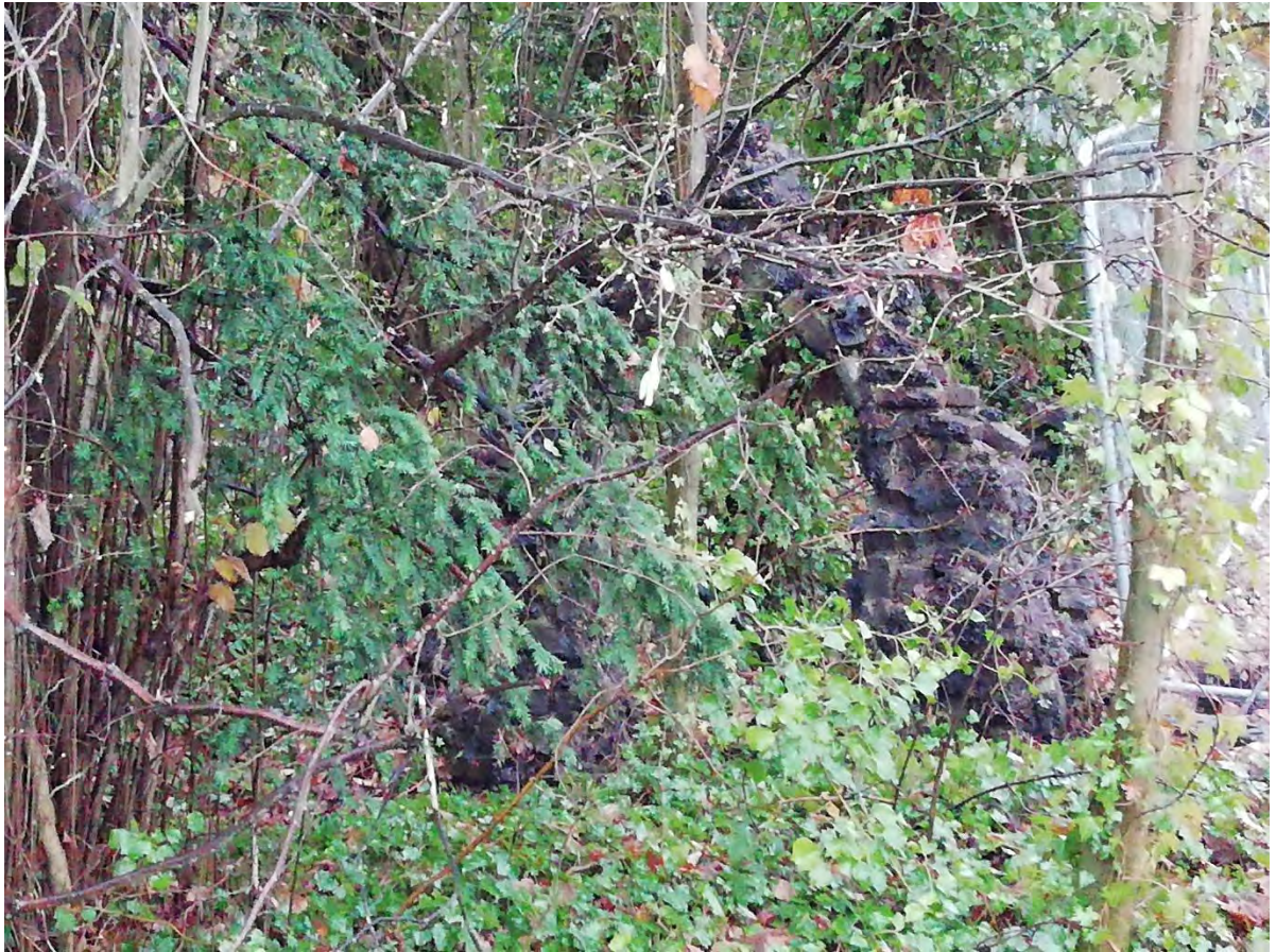
Plate 1: Surviving part of former brick / stone arch
