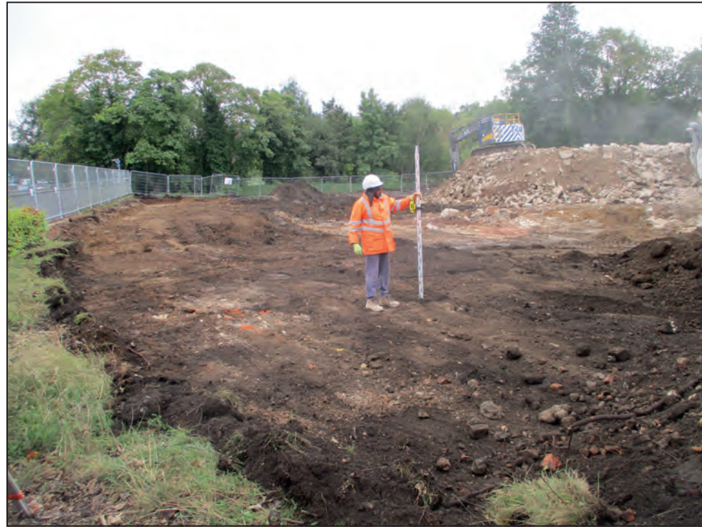
Ground reduction for piling mat: Trench 2, looking south-east
