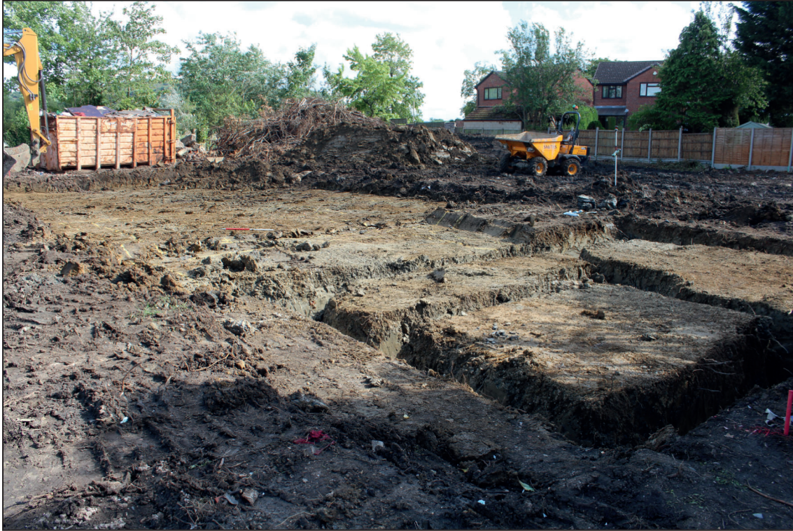
Trench 1 after ground reduction, looking south-east (1m scale)
