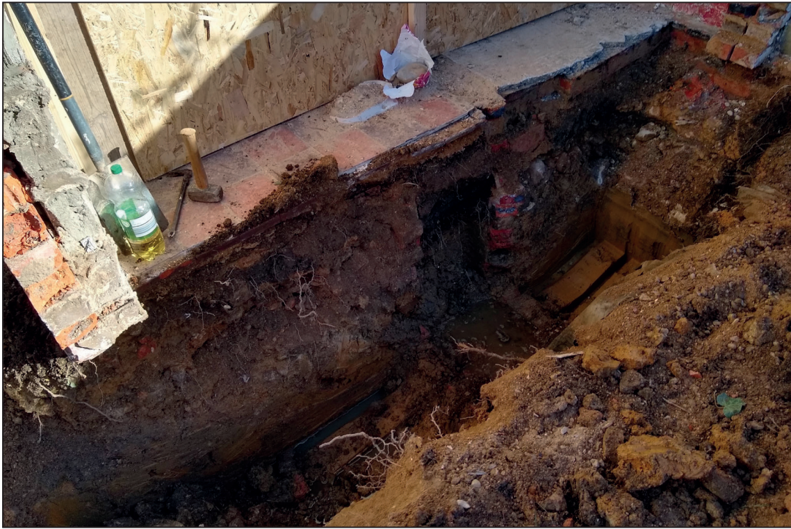
Trench mid-excavation showing piped access to water tank, looking north-west
