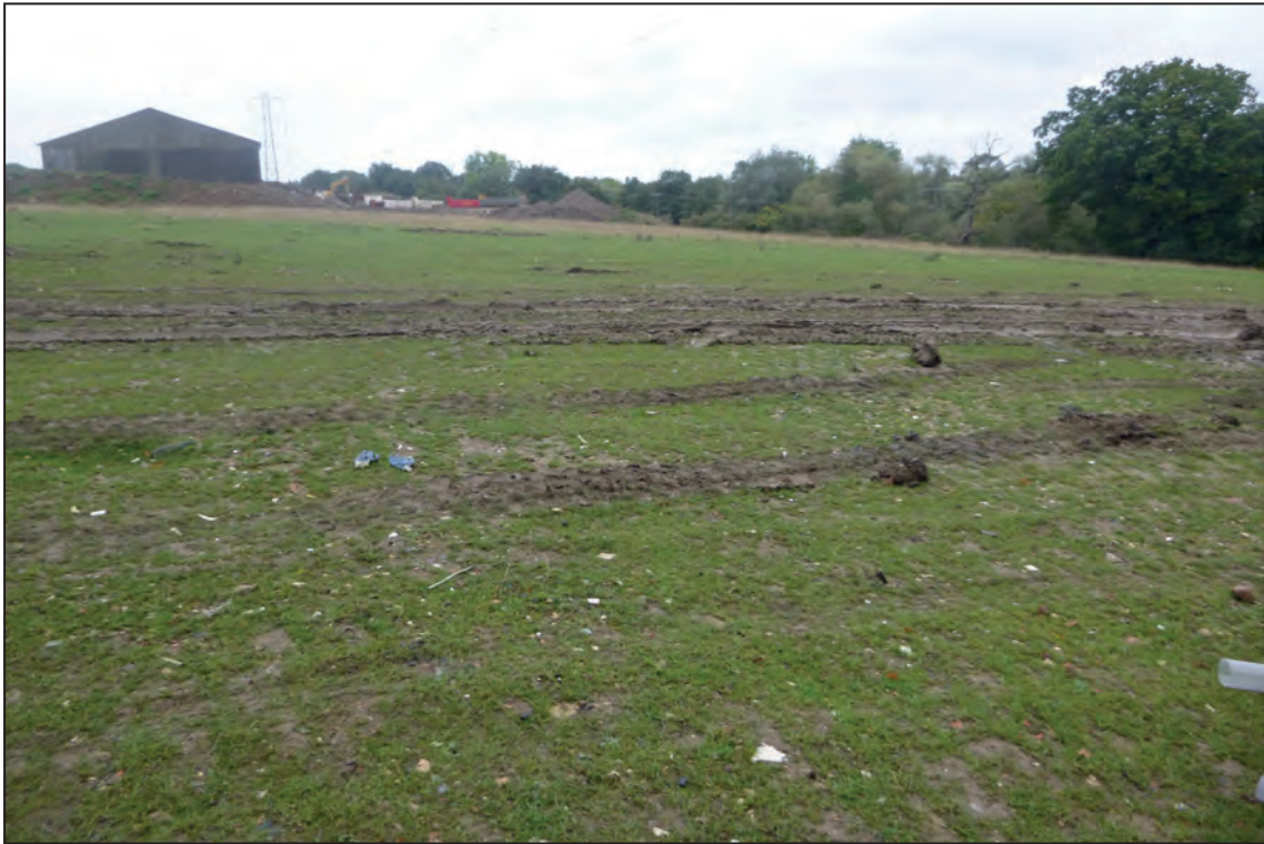
Site, looking south towards skip yard
