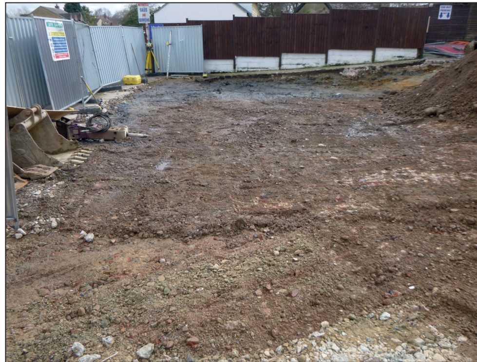
Excavated area, looking south
