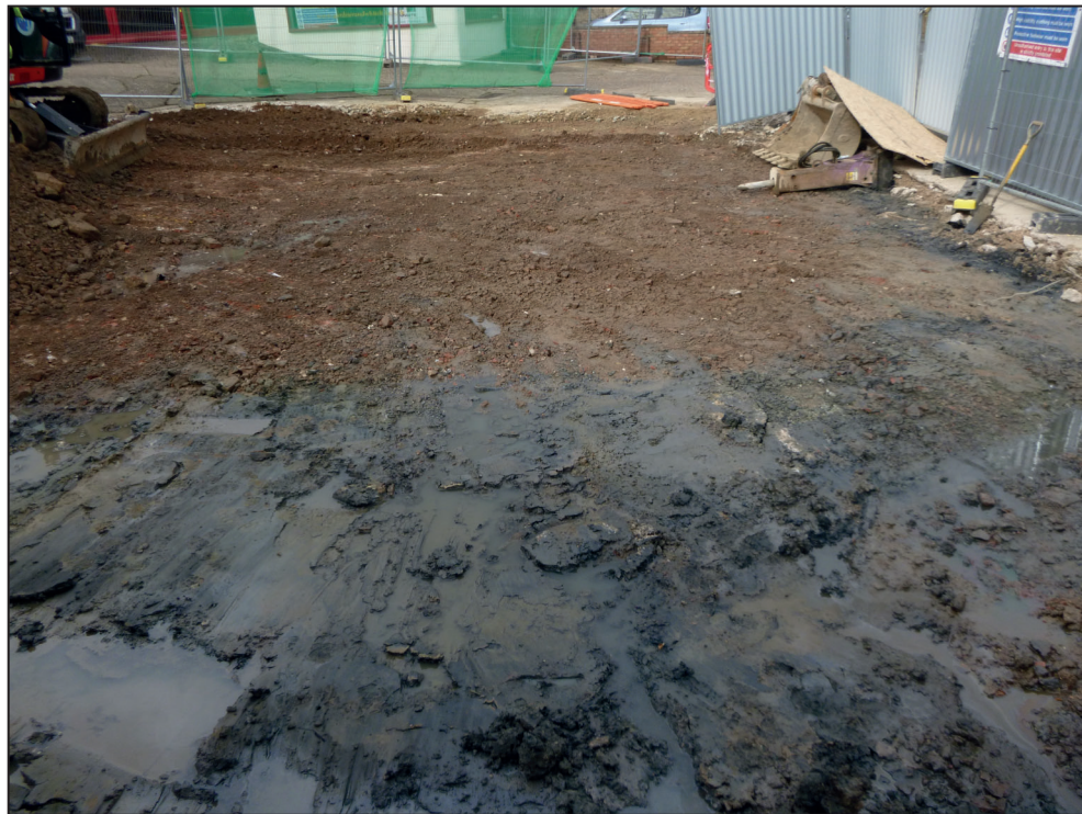
Excavated area, looking north
