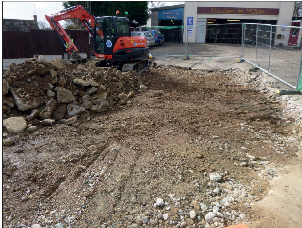
Removal of concrete
