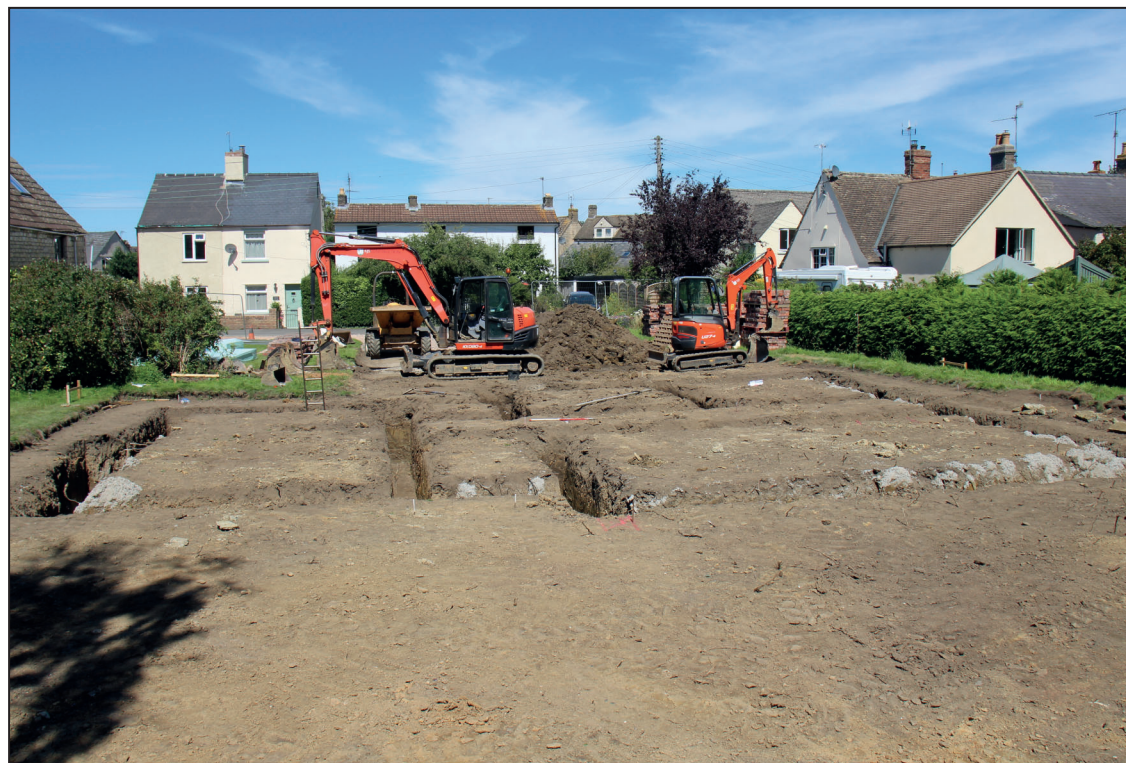
Trench 5, looking north (1m scale)
