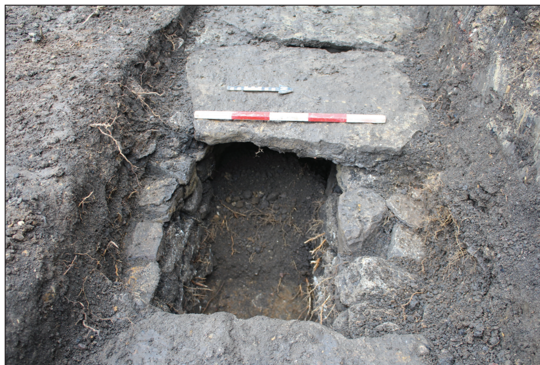
Culvert 117, looking west (0.5m scale)
