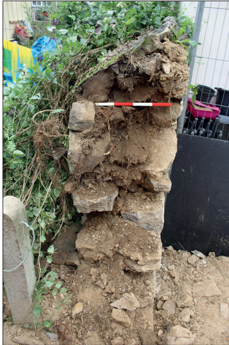
Wall 900 section, looking north-east (0.4m scale)
