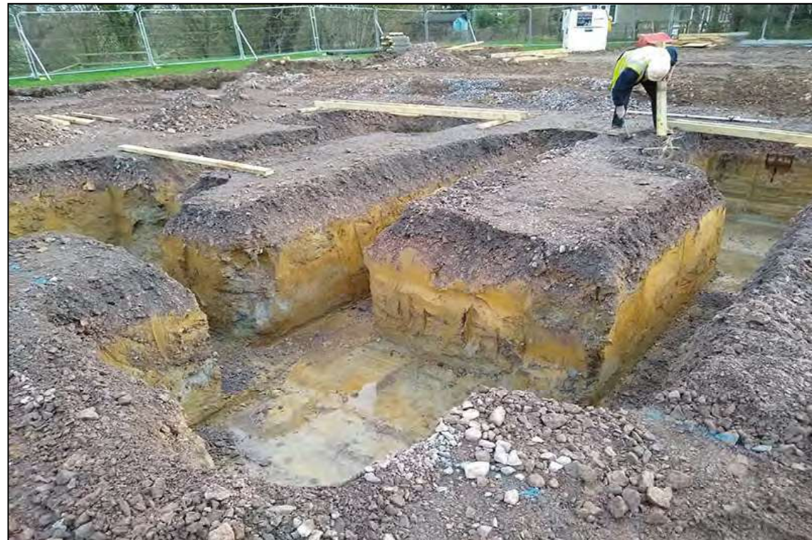
Trench 13, looking north-east
