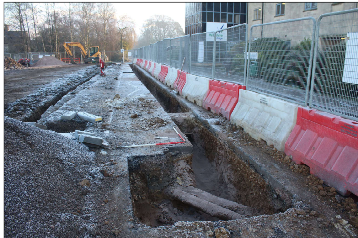
Trench 11, looking east (1m scales)
