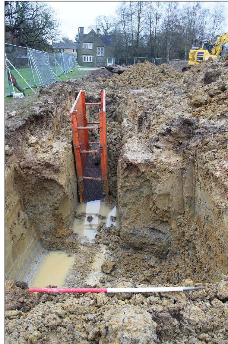
Trench 2, looking east (1m scale)
