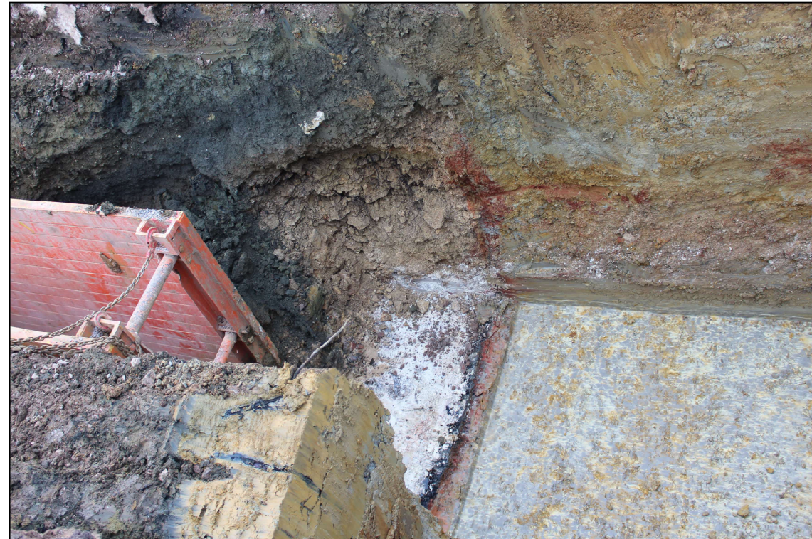
Southern extent of soakaway 306
