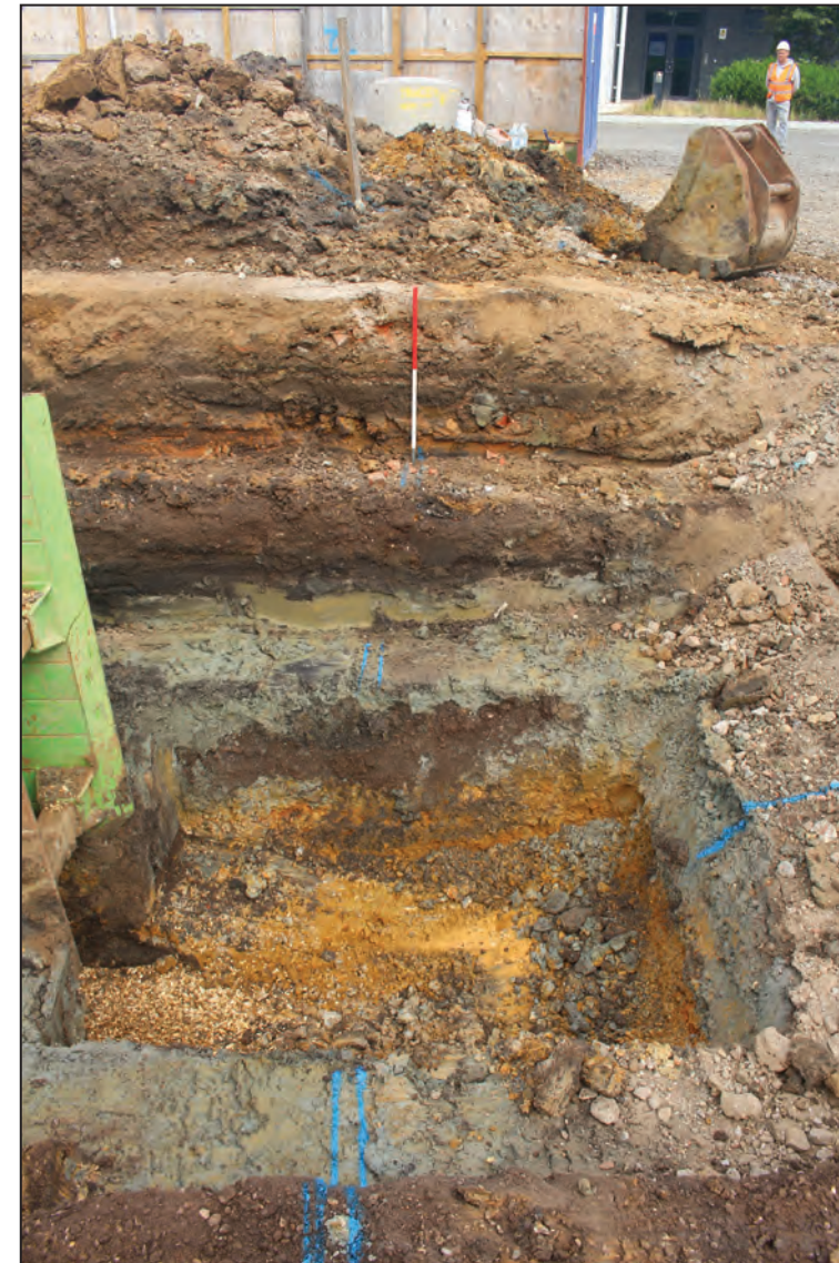
Trench 4, looking north-west (1m scale)
