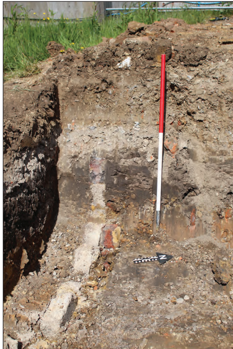
Structure 108, looking north-west (1m scale)
