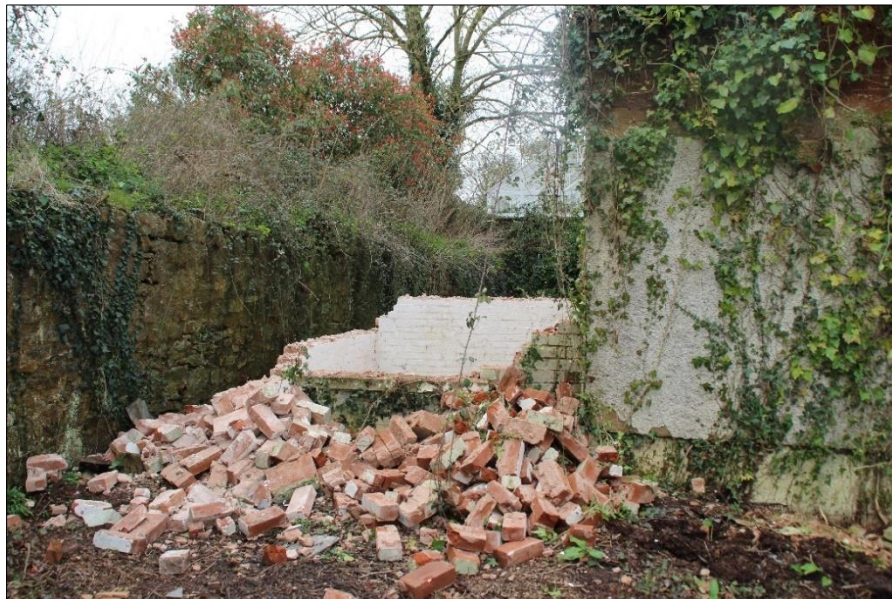
Fig.48 View of brick dairy extension, looking west
