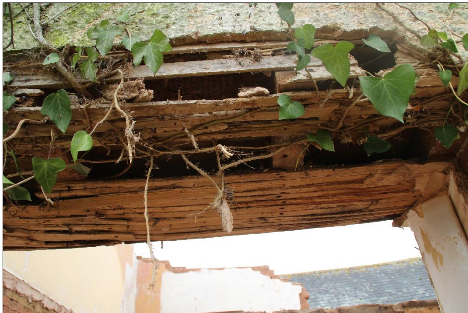
Fig.45 View of lintel over window in eastern elevation
