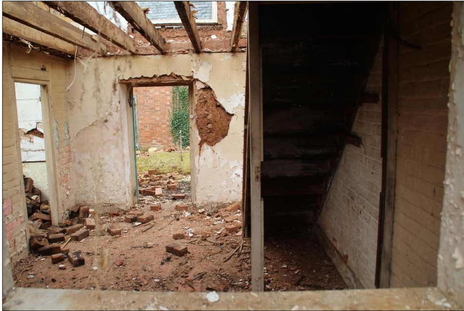
Fig. 50 View of the rear entrance hall with staircase to right
