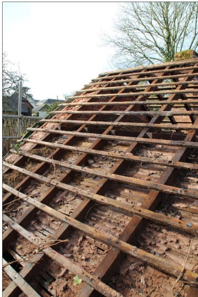
Fig.24 Lathe and torching on eastern roof slope
