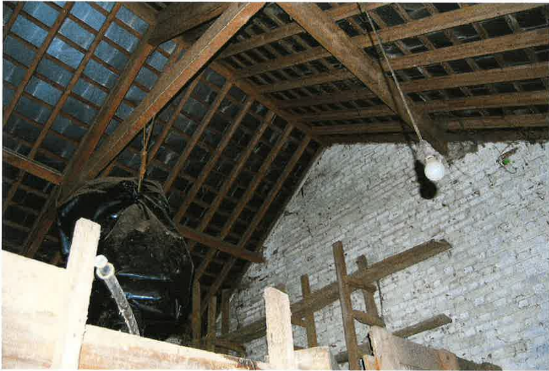
Pl.30: The roof structure and loft in the Cart Shed (Building C).
