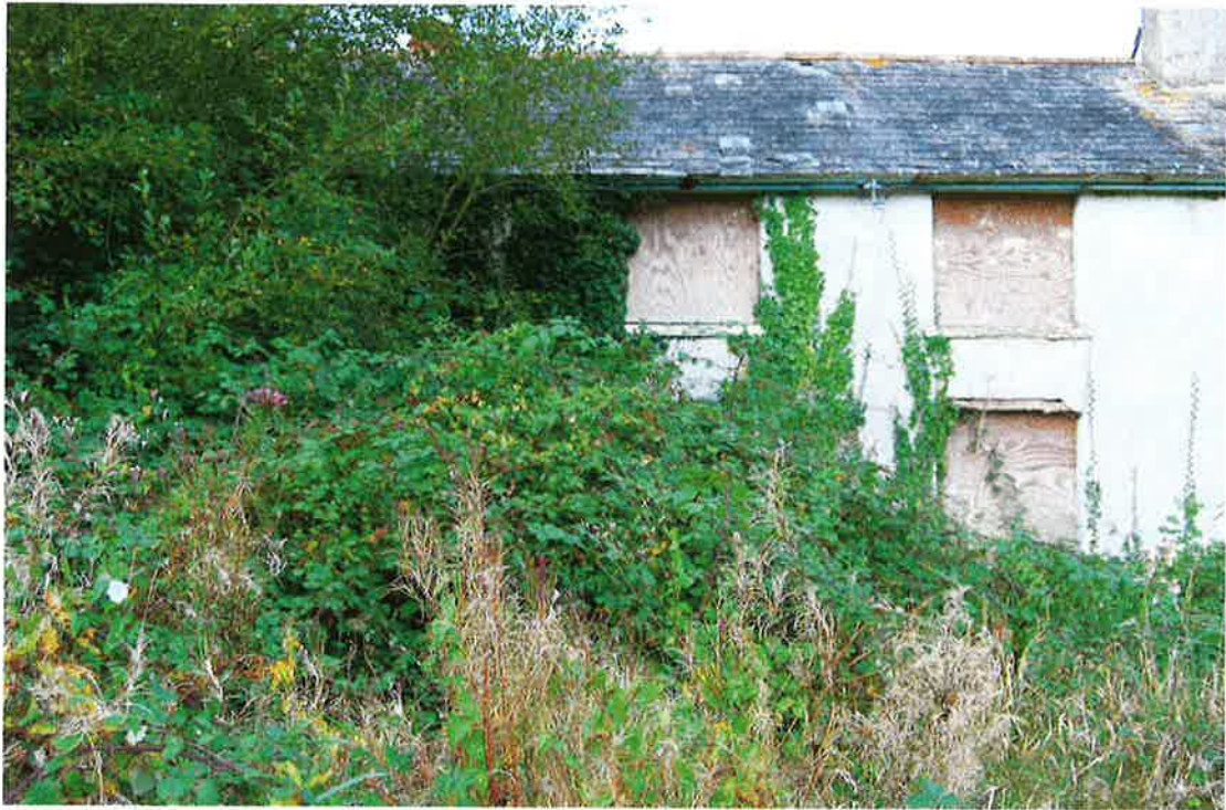
Pl.13: The east elevation of the southern portion of the farmhouse.
