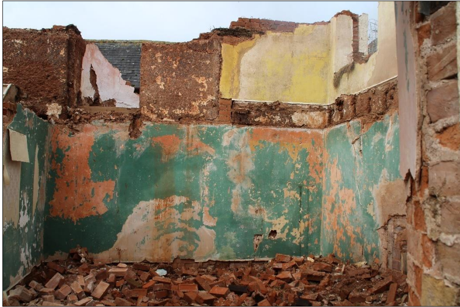
Fig.41 View of the sitting room looking west
