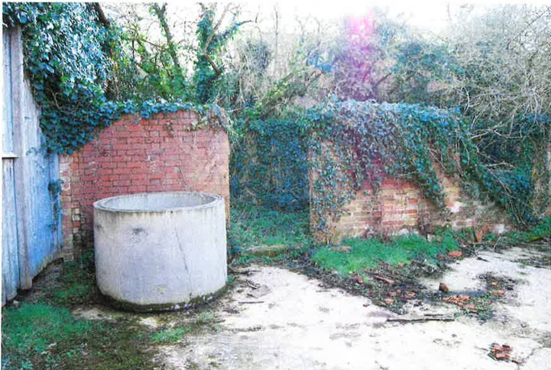
Pl.31: The ruined West Linhay (Building D) from the north.
