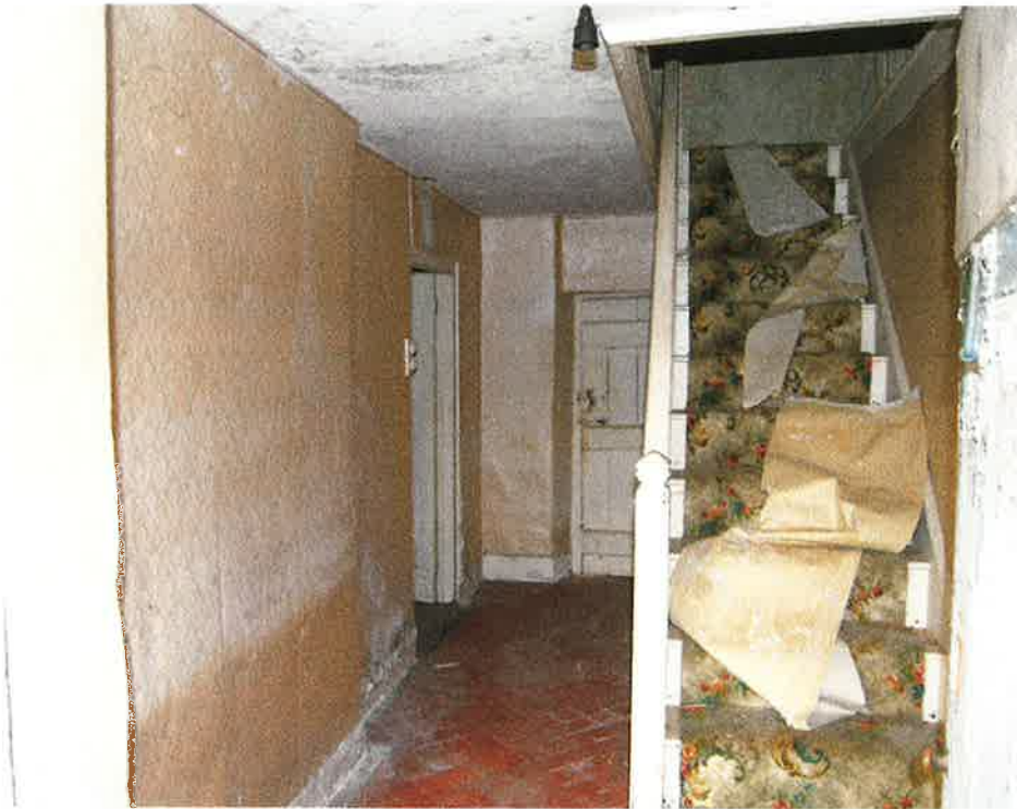
Pl.8: The entrance hall, looking west.
