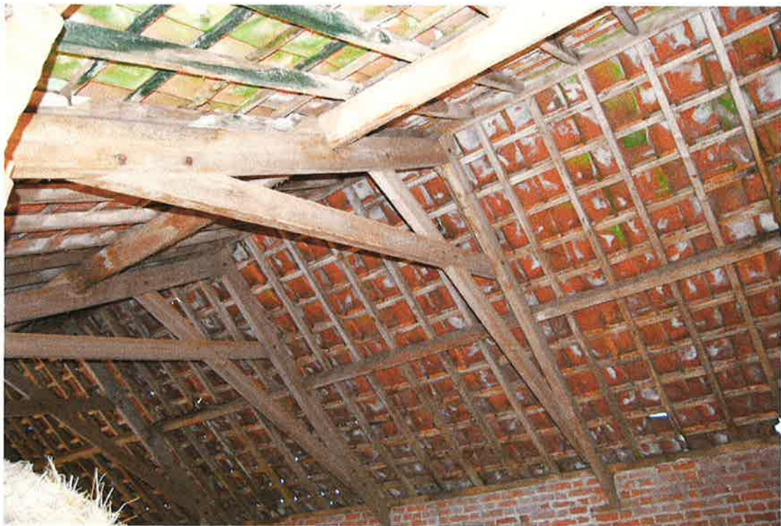
Pl.42: The unusual scissor-braced roof trusses in the North-West Range (Building H).
