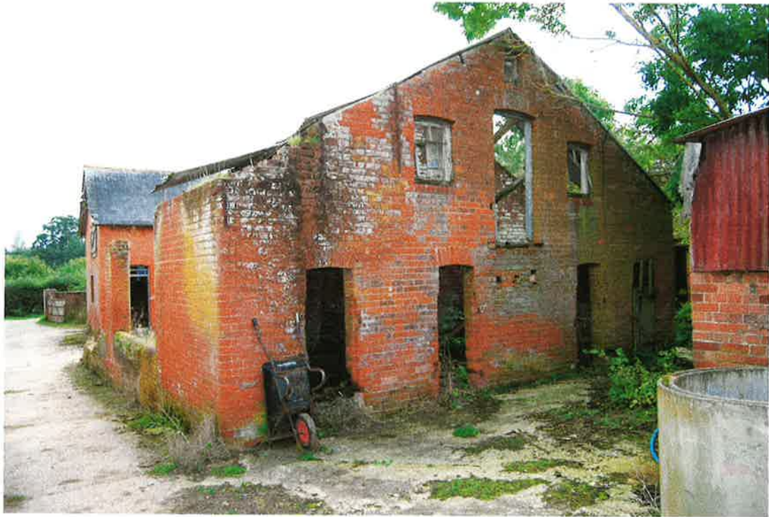
Pl.35: The Piggery Complex (Building G) from the north-west.
