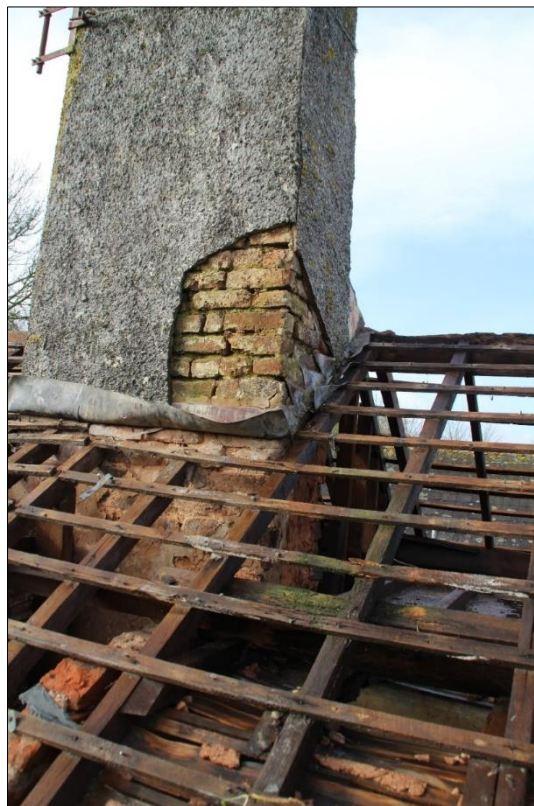
Fig.21 View of large central chimney stack with pale bricks
