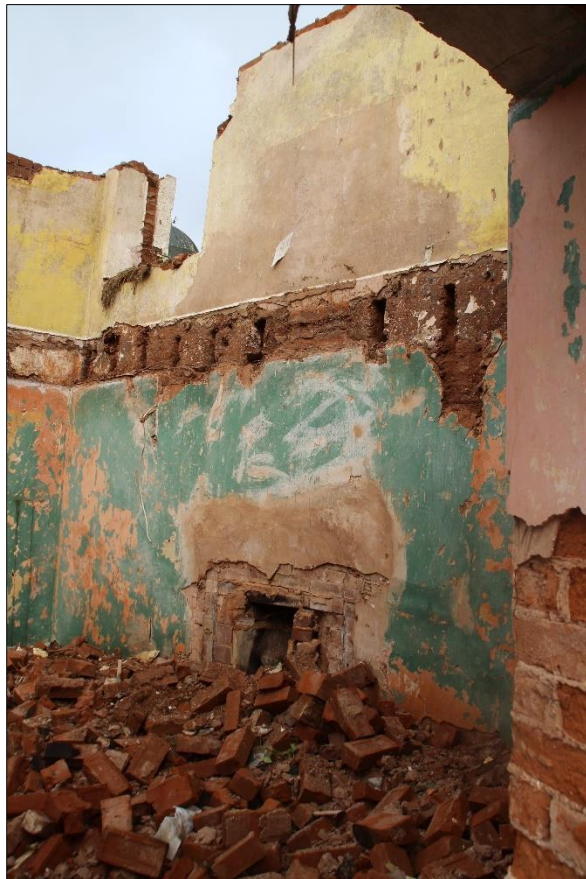
Fig.42 View of the sitting room fireplace, looking north-west
