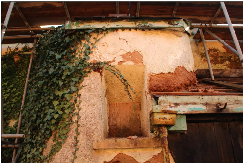
Fig.12 View of the turret window and joint with the lean-to roof
