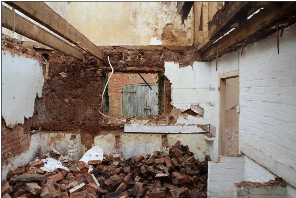
Fig.46 View of the dairy, looking west
