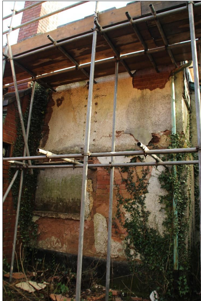
Fig.15 The northern section of the eastern elevation
