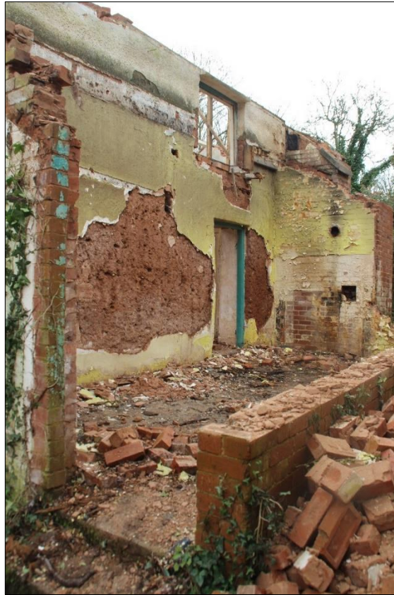
Fig.53 View of the demolished kitchen extension
