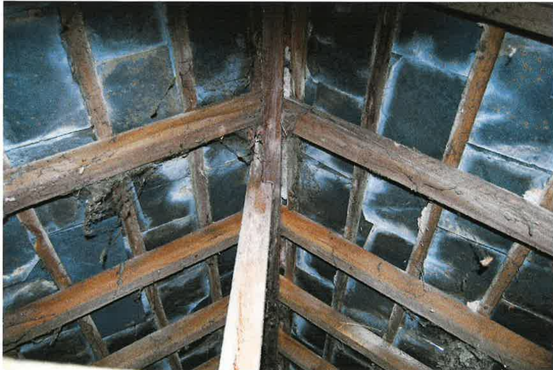
Pl.15: Part of the simple roof structure.
