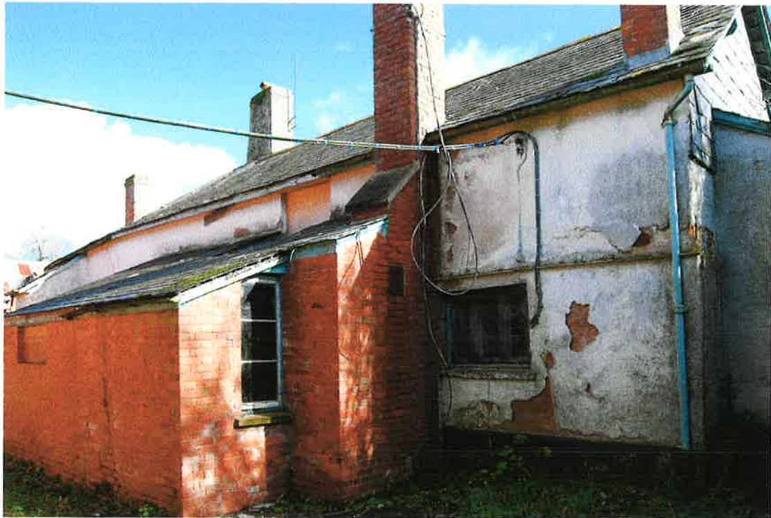
Pl.14: The farmhouse from the south-west, with the kitchen extension to the left and the dairy extension on the extreme right. Note kink in roof.
