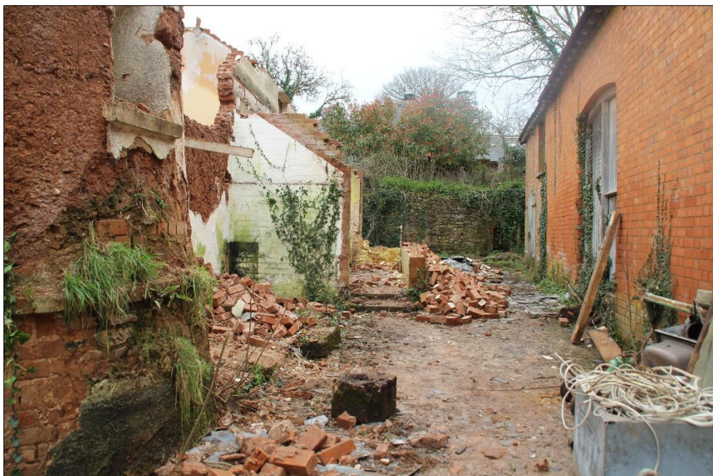
Fig.56 A general view of the western elevation, looking south
