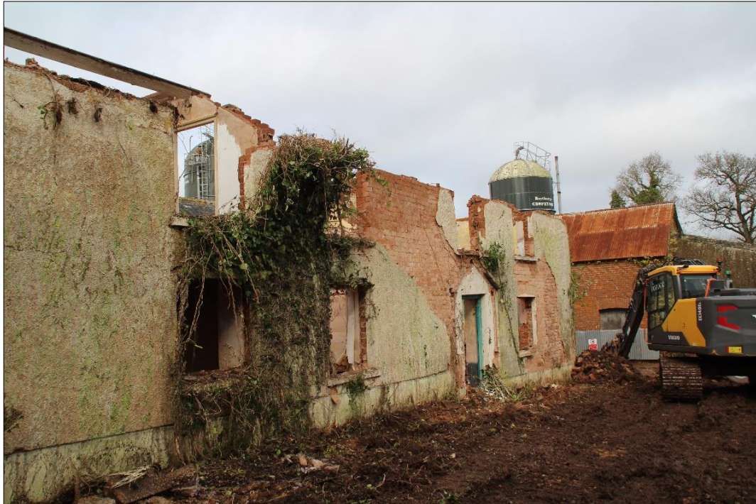
Fig.38 The eastern elevation of the building looking north
