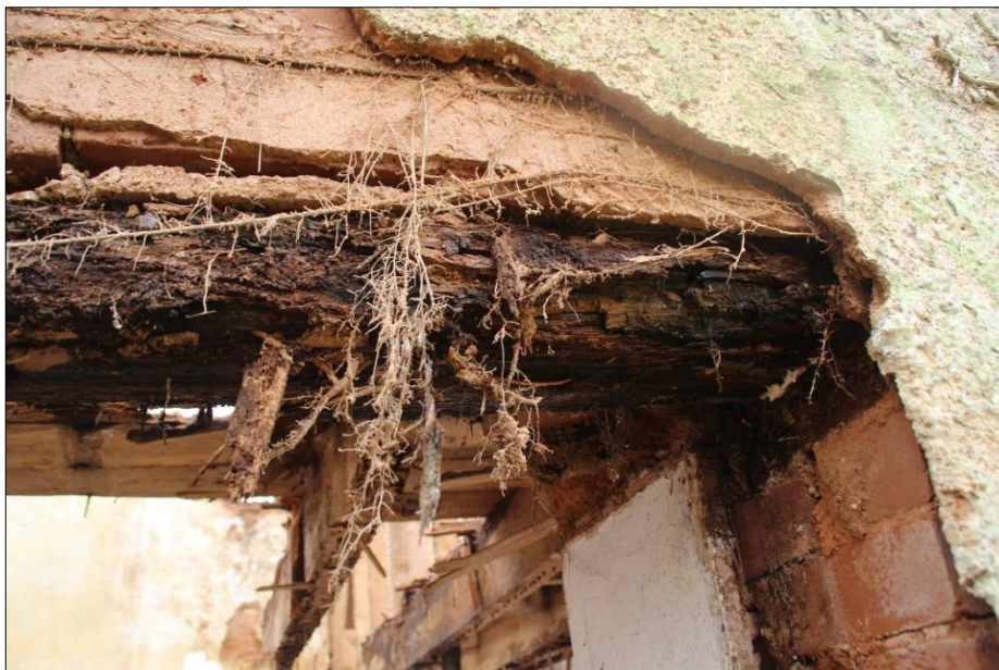
Fig.47 View of timber lintel over window to dairy
