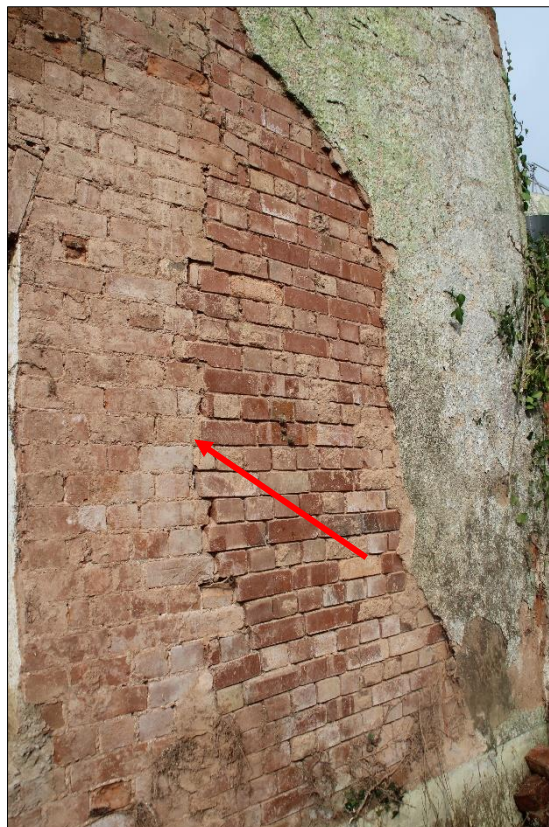
Fig.39 Detail showing modern brick (left hand side) and handmade bricks (shown with arrow)
