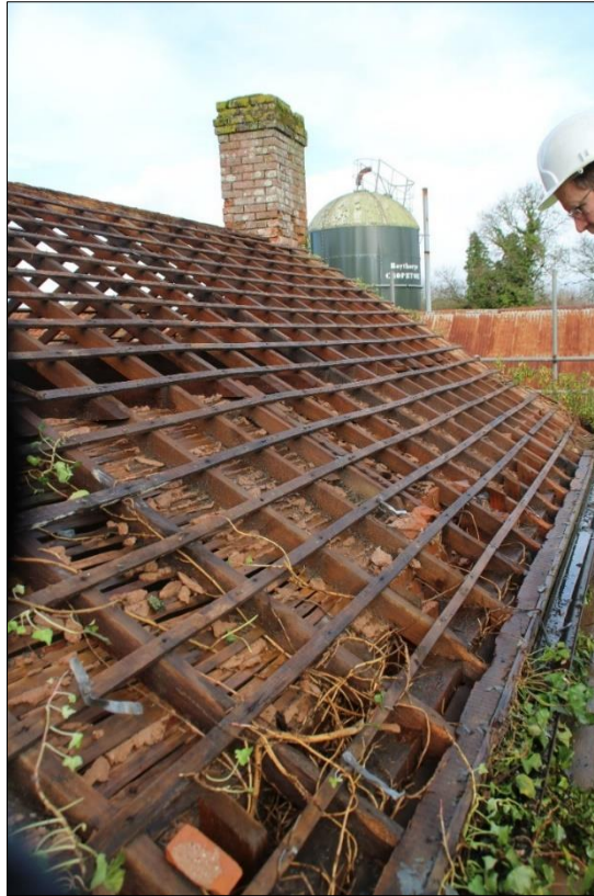
Fig.20 View of lathes and torching, eastern roofslope
