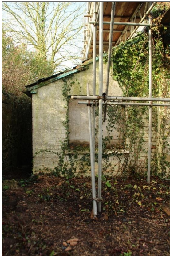
Fig.8 Dairy extension, image taken looking west
