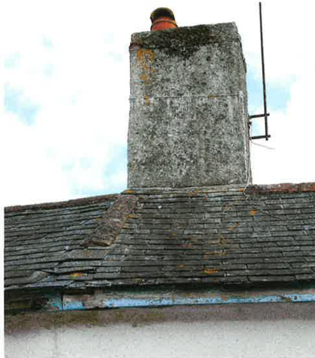
Pl.7: Detail of the main chimney from the west, also showing the 'kink' in the roof structure between the two main sections of the farmhouse.
