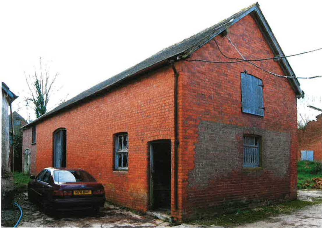
Pl.23: The Barn from the north-east; note the different brickwork in the lower part of the gable wall, probably part of an earlier building.
