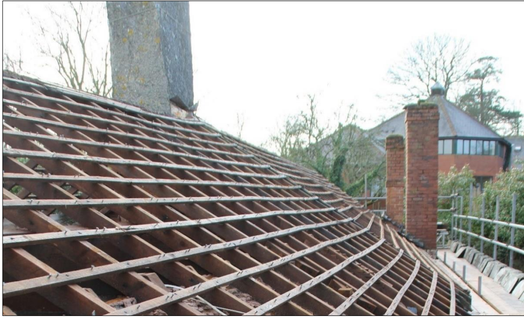
Fig.26 View of two chimney stacks on western roof slope
