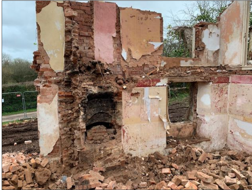
Fig.60 View of bread oven within eastern elevation and large chimney stack
