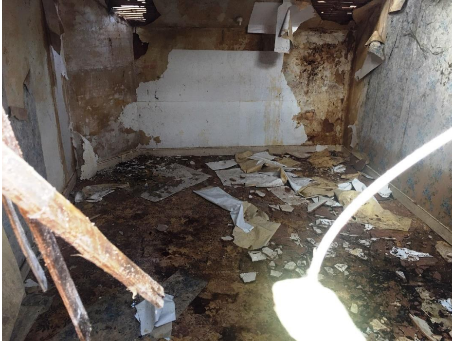
Fig.31 South bedroom viewed from scaffolding platform showing corner chimney breast
