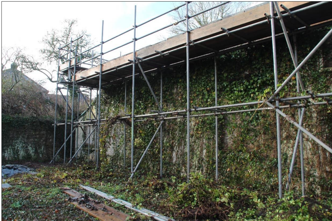
Fig.6 Eastern elevation of the Building, image taken looking south-west
