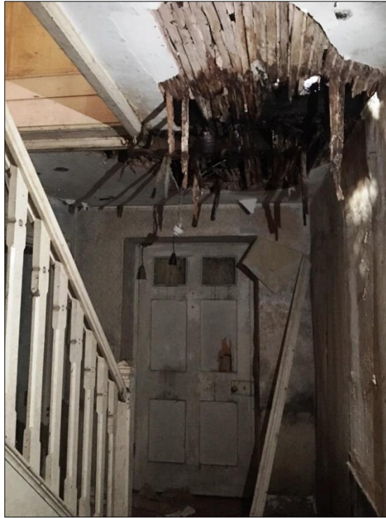
Fig.34 Lathe ceiling in the main entrance hall
