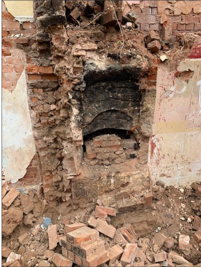
Fig.59 Bread oven discovered in large chimney stack
