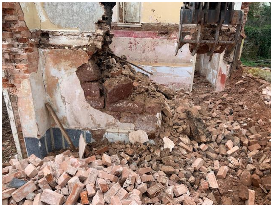
Fig.58 View of stone walling within fabric
