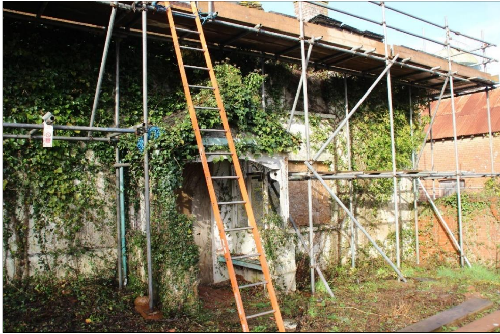
Fig.7 Eastern elevation of the Building, image taken looking north west
