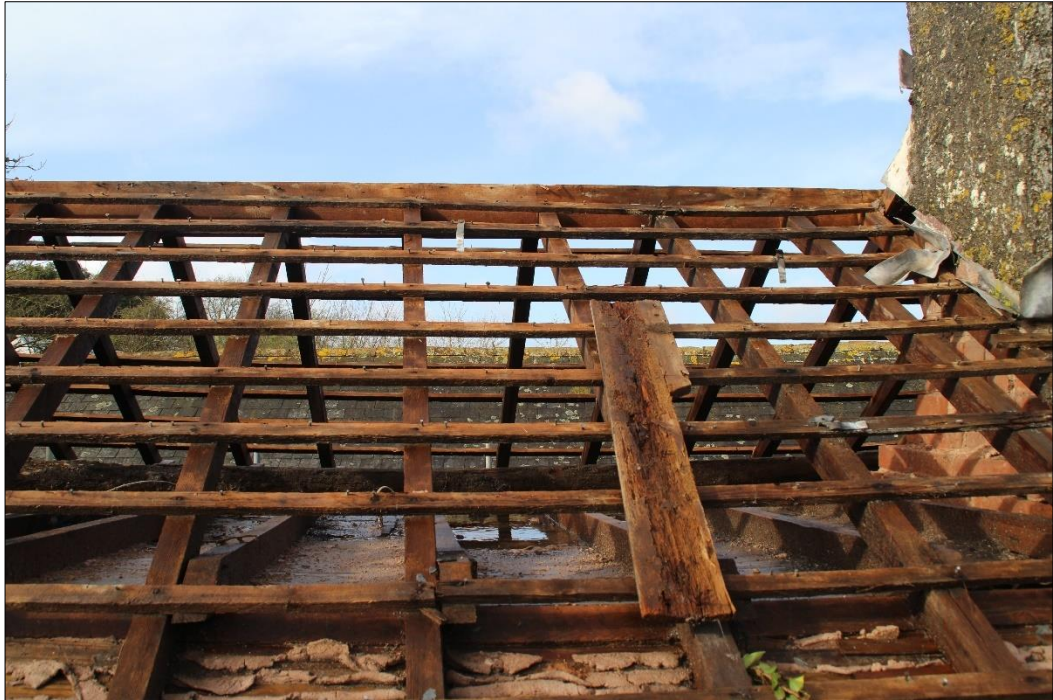
Fig.23 Eastern roof slope on the southern part of the building
