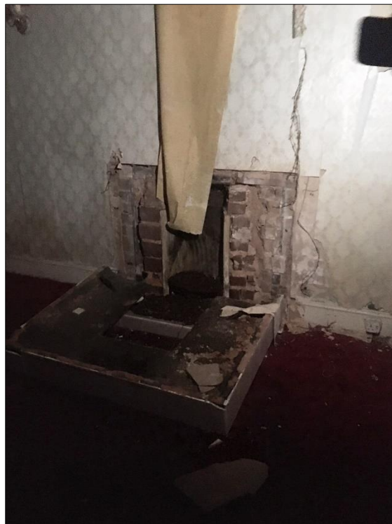
Fig.35 Brick fireplace in the sitting room (northern elevation)
