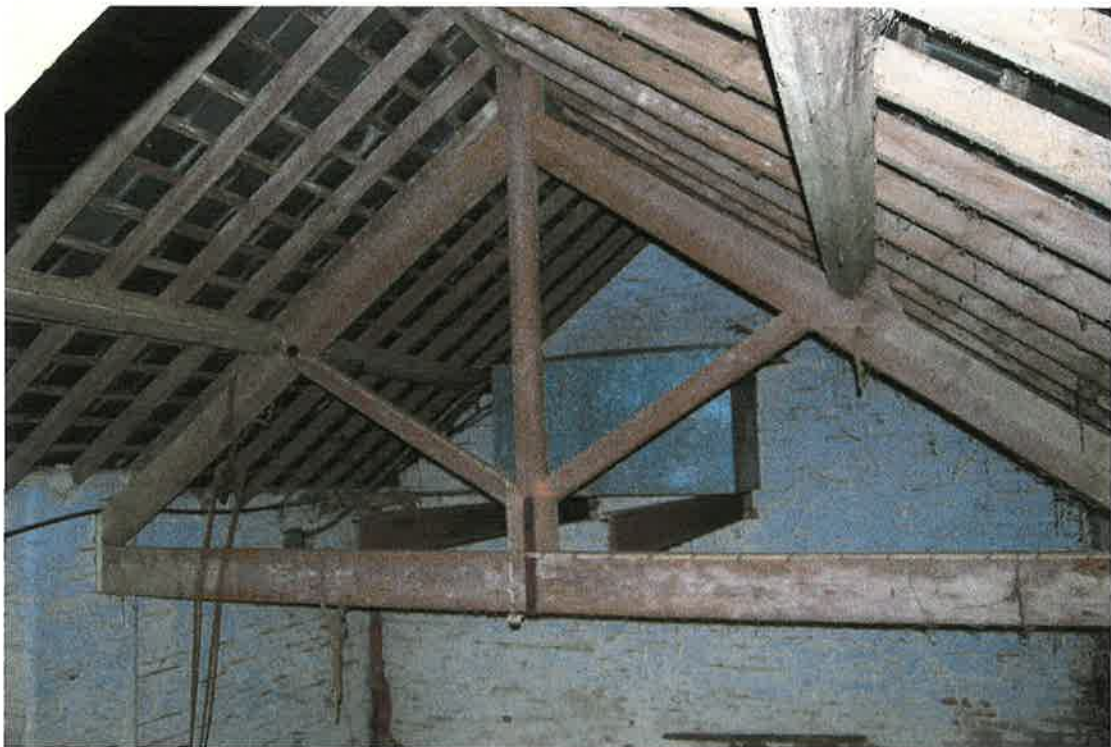
Pl.26: The southern truss of the Barn Range, from the north.
