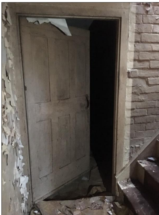
Fig.29 Doorway to living room showing brick spine wall
