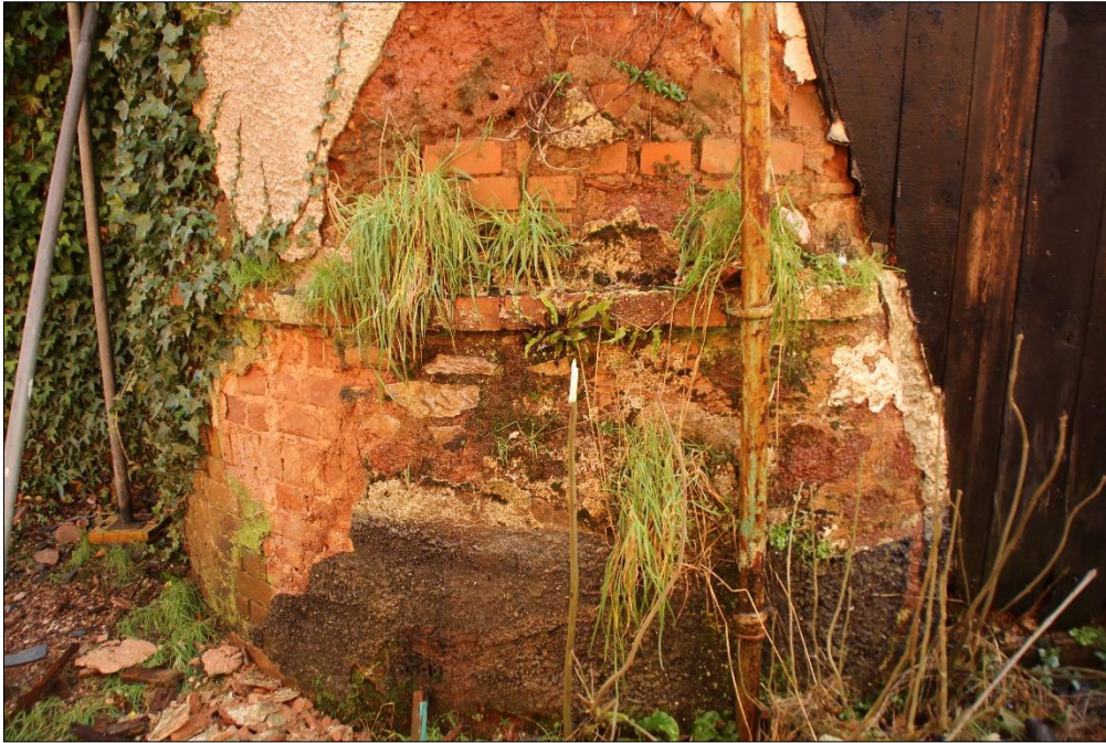
Fig.11 View of the turret on the west elevation showing mixed materials
