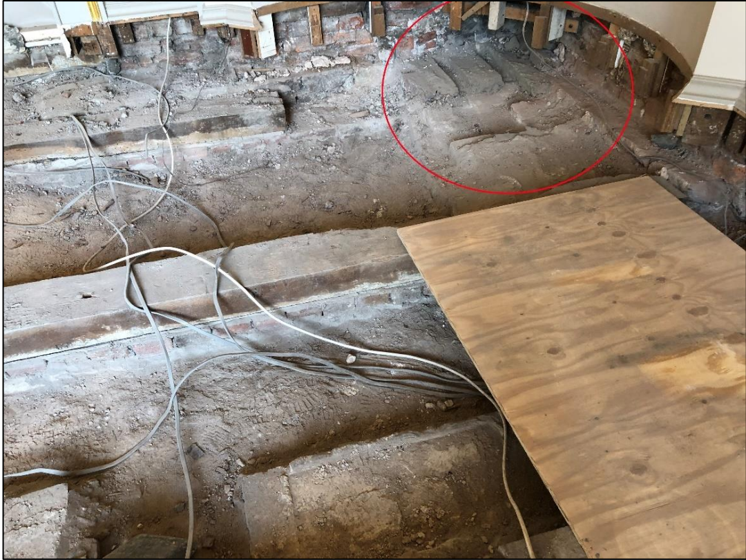
Photo 12 Detail showing the infill in the north-east corner
