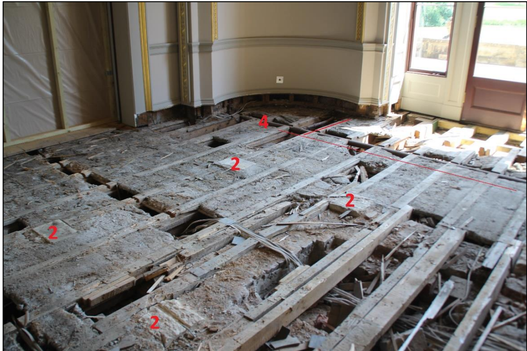
Photo 7 View of the south-east corner of the room
