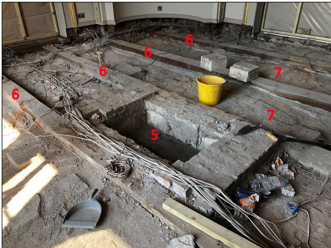
Photo 11 View of the western half of the room looking north-west
