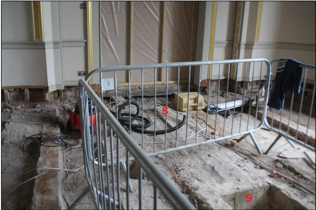
Photo 13 View of the central eastern section of the room
