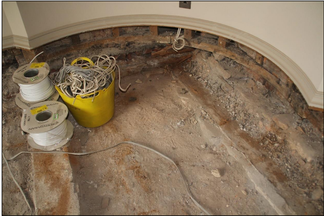
Photo 19 Detail of the north-east corner showing illustrating niche joinery and interface with brick piers running across the room
