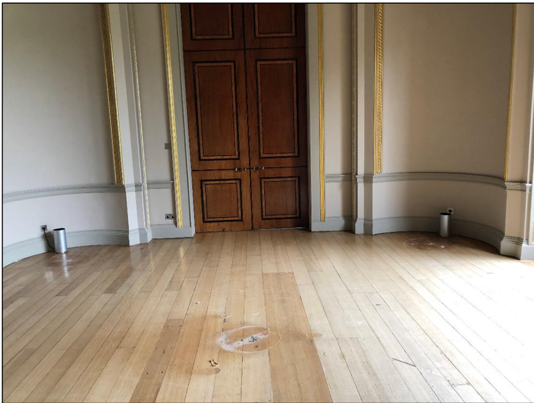
Fig.5 Image of the room looking east towards the drawing room
