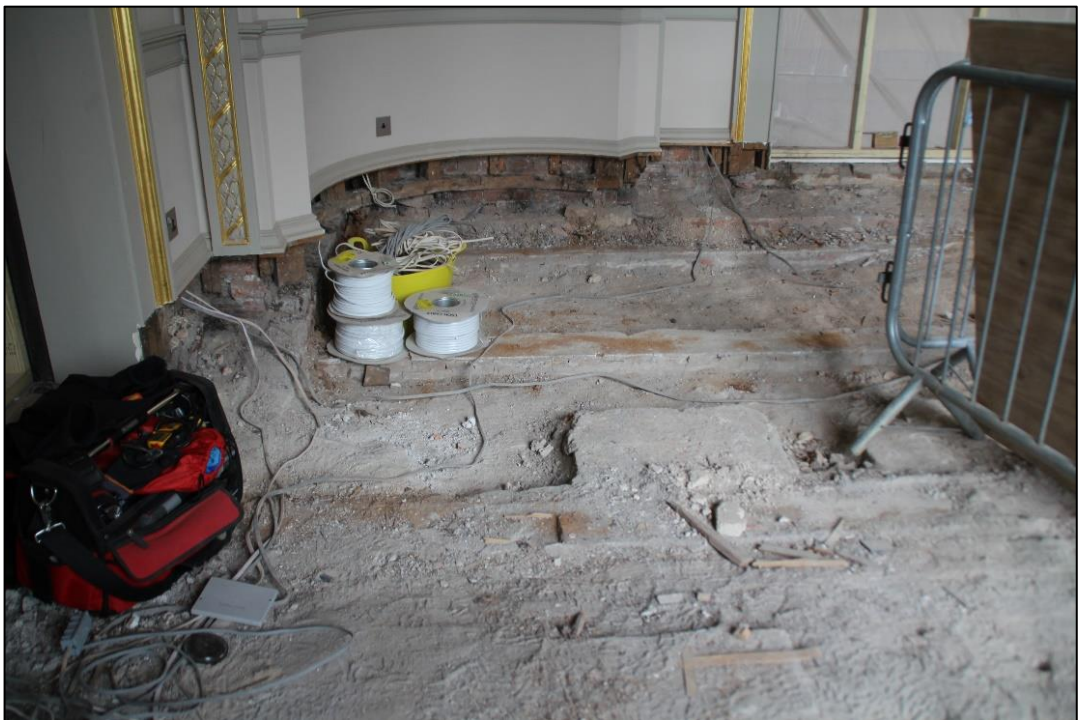
Photo 16 View of the north-west corner
