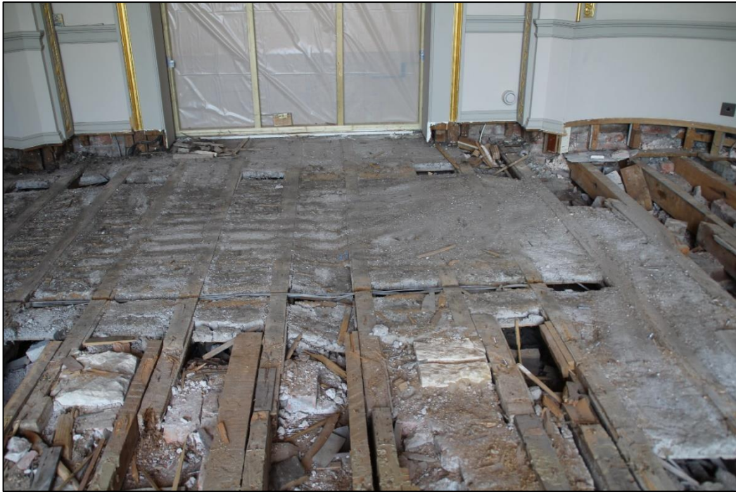
Photo 2 View of central northern portion of room
