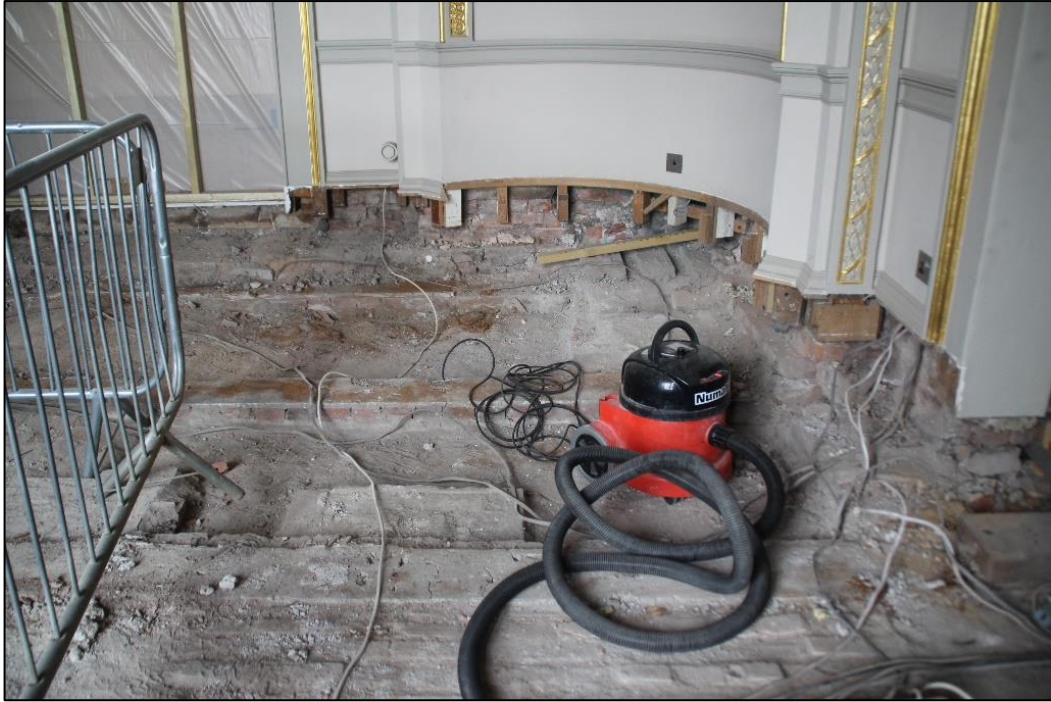
Photo 17 View of the north-east corner
