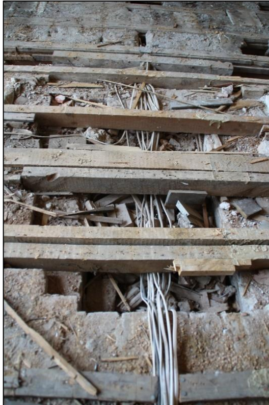
Photo 4 View of central stove void as found following removal of floorboards
