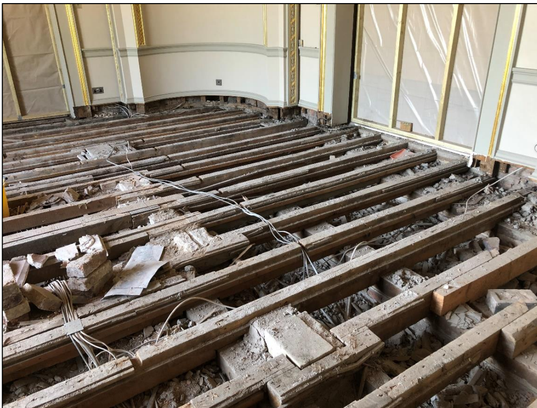
Photo 10 View of the northern half of the room looking west
