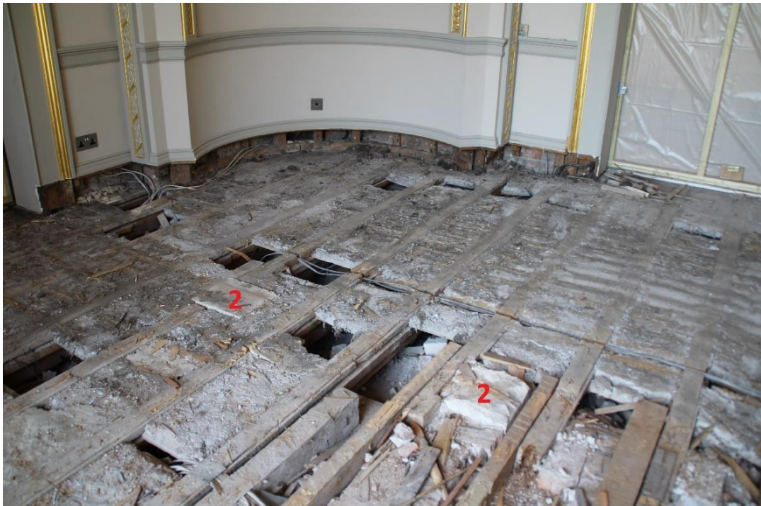
Photo 3 View of north-west corner of room
