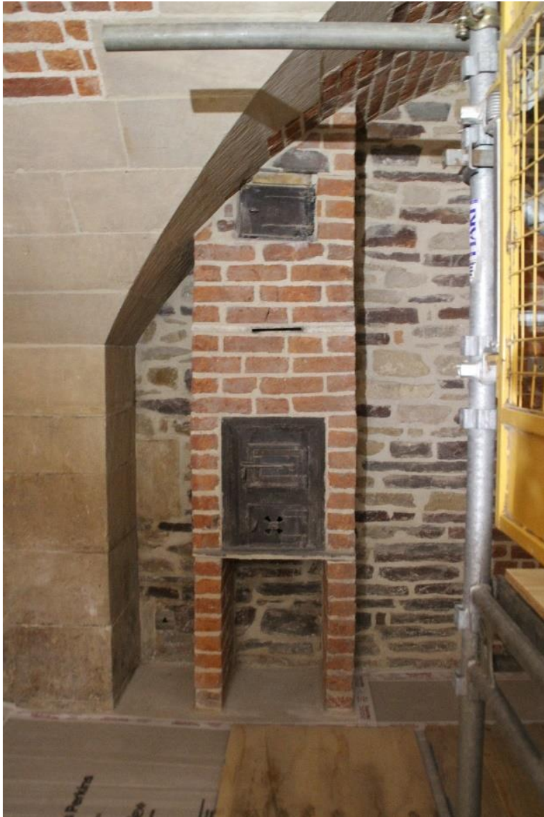
Fig.10 View of the small chimney and inset stove within the north-east corner
