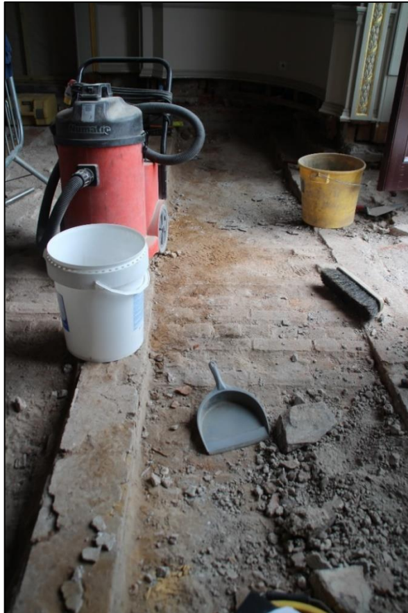
Photo 14 Detail showing apex of the barrel being uncovered
