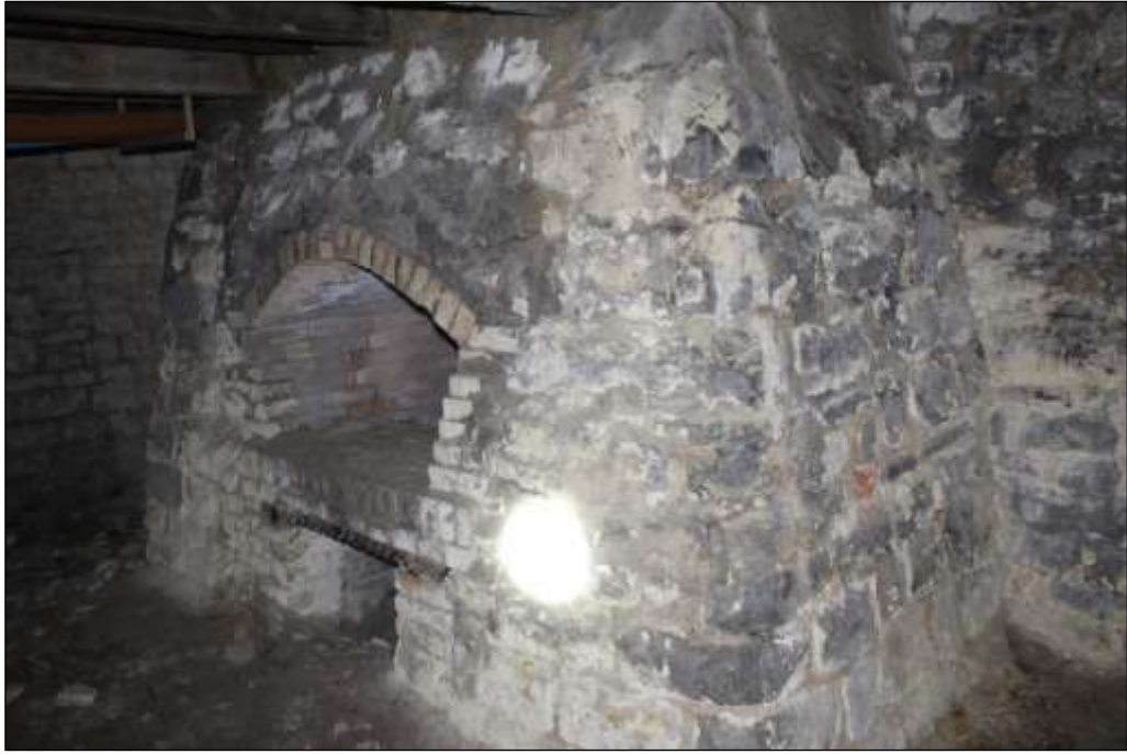
Fig.57 View of furnace structure on kiln interior side
