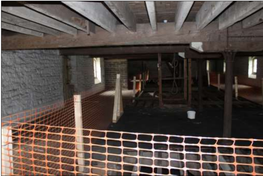
Fig.32 Upper growing floor viewed from east end
