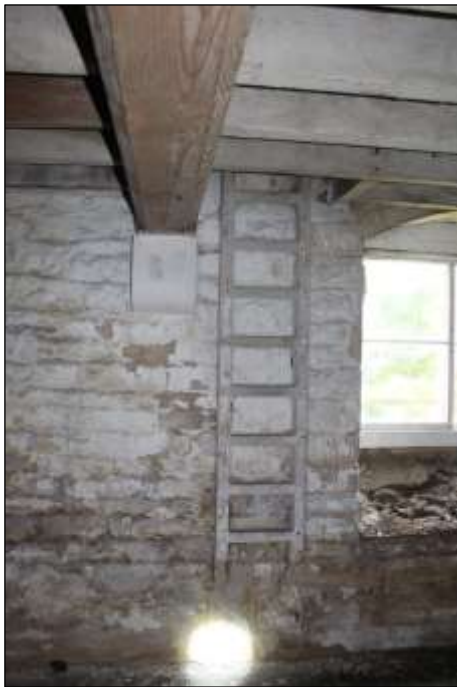
Fig.30 Ladder in lower ground floor leading from hatch (above)
