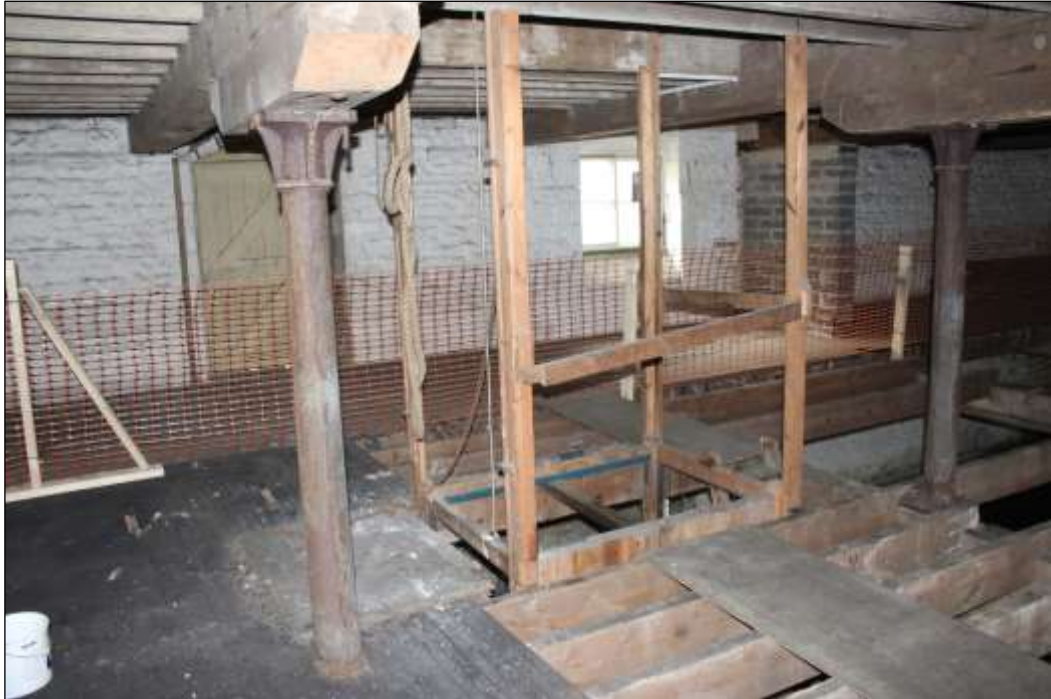
Fig.34 View of hoist structure, upper growing floor
