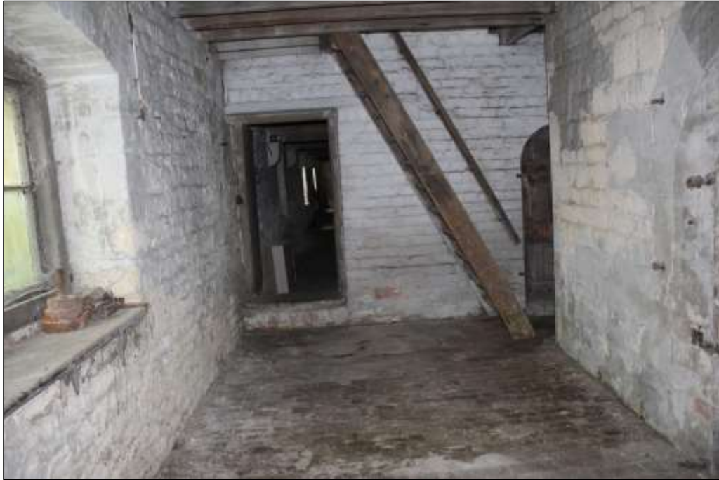
Fig.55 View of furnace anteroom, view to the east
