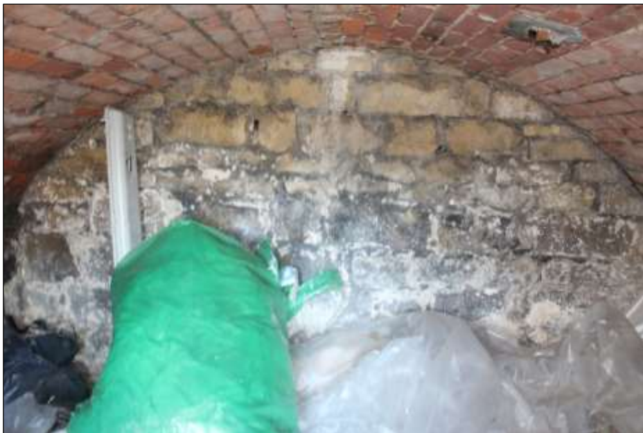
Fig.25 Interior of small vault under the steep, Maltings 1
