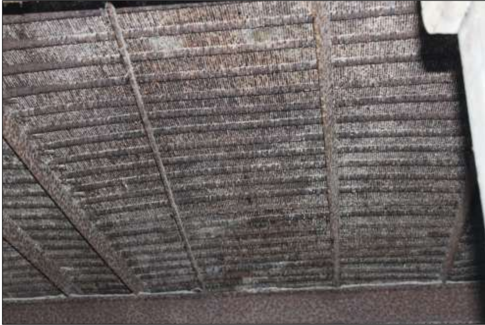
Fig.80 Detail of surviving mesh floor in kiln of Maltings 1
