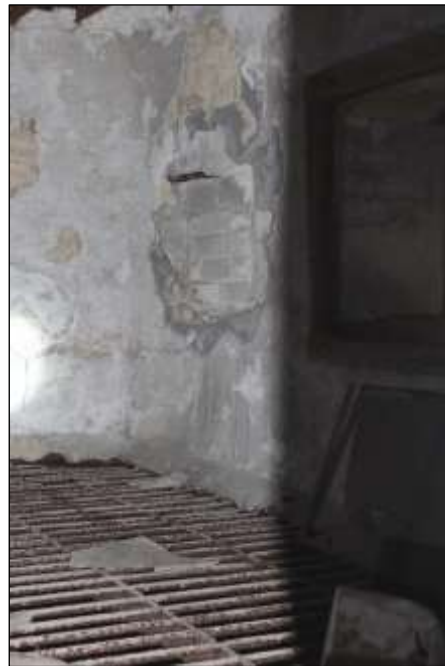
Fig.81 detail of metal lower drying floor of kiln in Maltings 2, this would have had a mesh covering when in use
