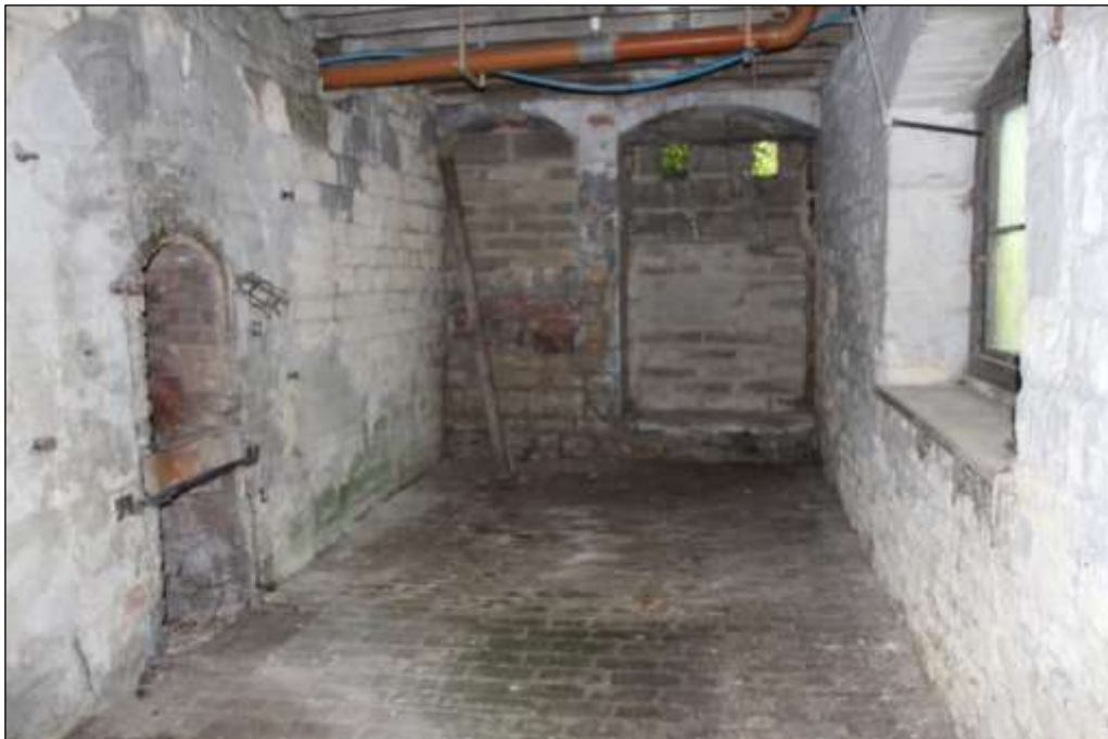
Fig.52 Kiln furnace anteroom, lower ground floor view to the west
