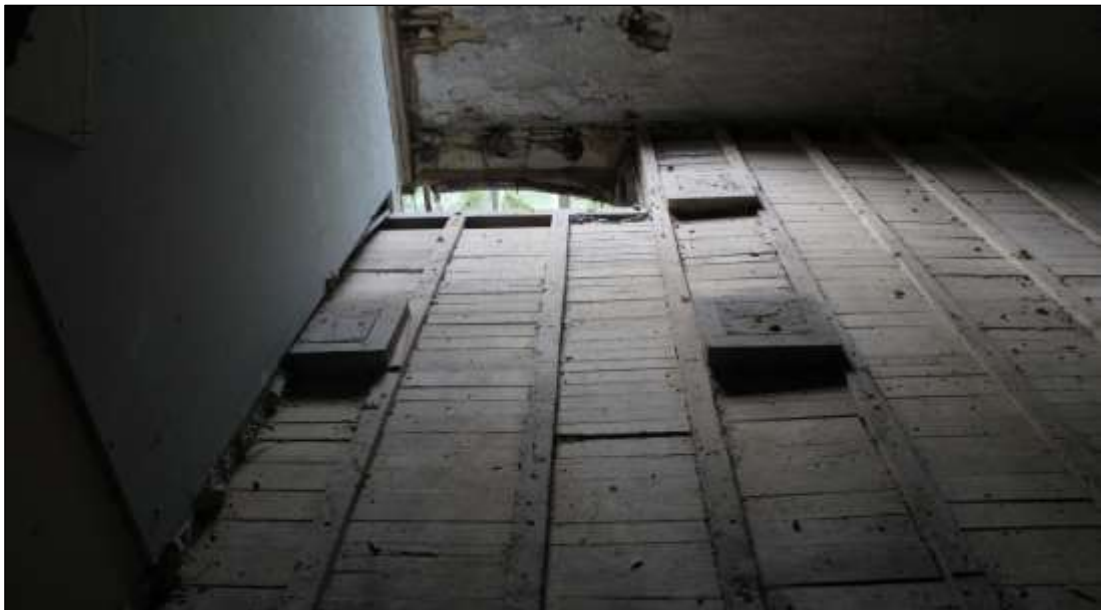
Fig.77 Detail of hatches revealed where asphalt has been removed
