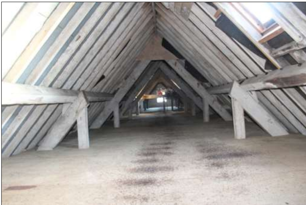
Fig.42 The upper drying floor (attic space), Maltings 1
