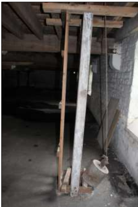
Fig.23 Detail of hoist counterweight, lower growing floor, Maltings 1
