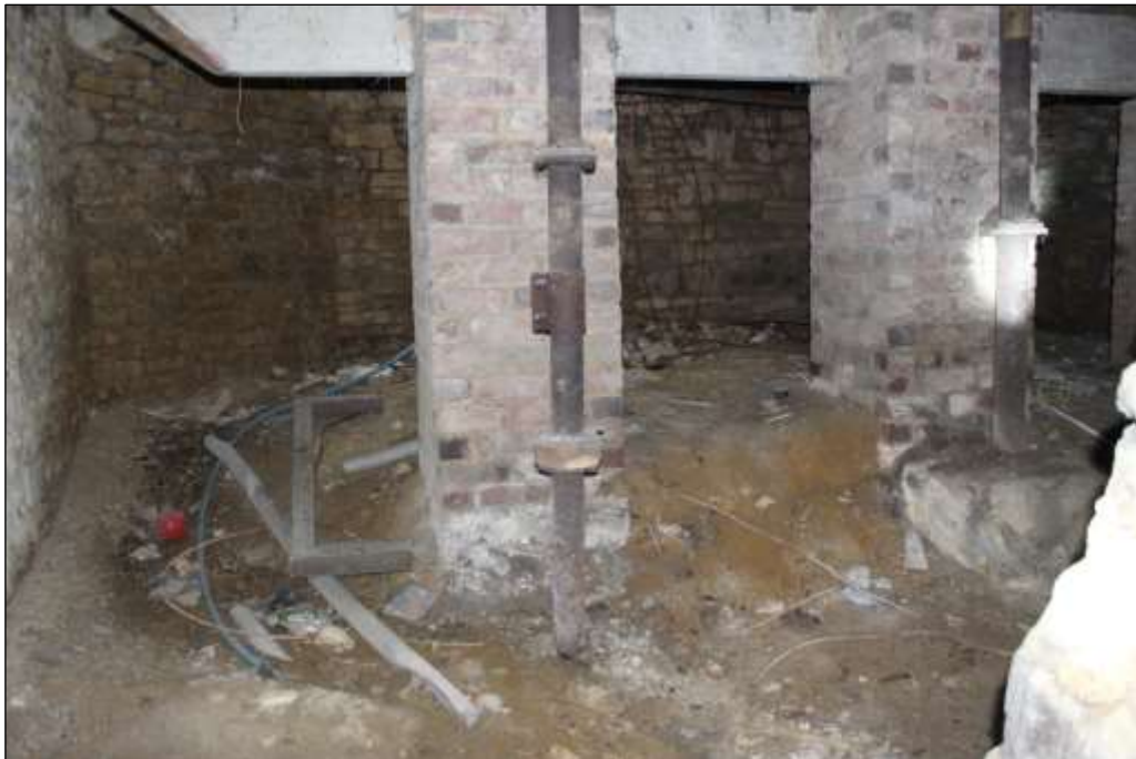
Fig.56 View of the interior of the kiln at lower ground floor
