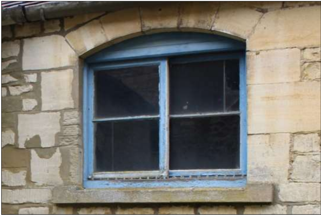
Fig.10 View of a typical window, Maltings 1
