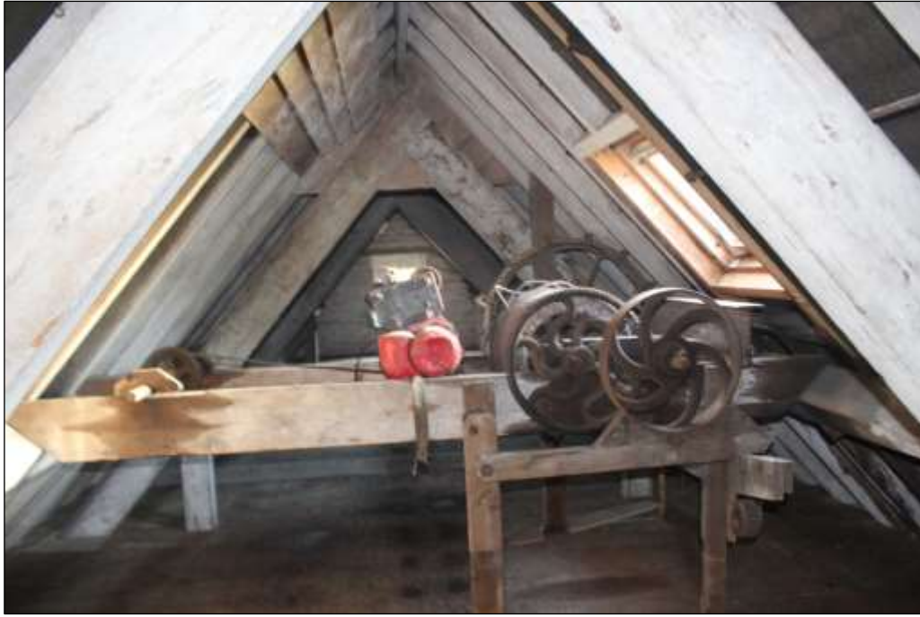
Fig.42a Detail of hoisting machinery winder, Maltings 1 attic
