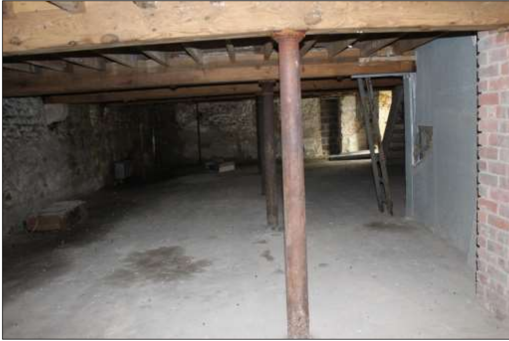
Fig.67 The lower growing floor (lower ground floor) of Maltings 2, view to the west
