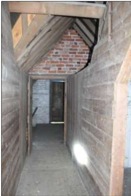
Fig.39 View to the south of the upper floor of the cross-wing
