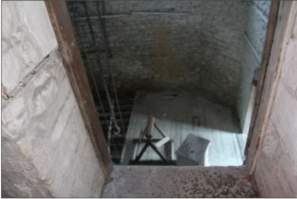
Fig.44 Doorway over kiln void, once accessing the upper kiln drying floor
