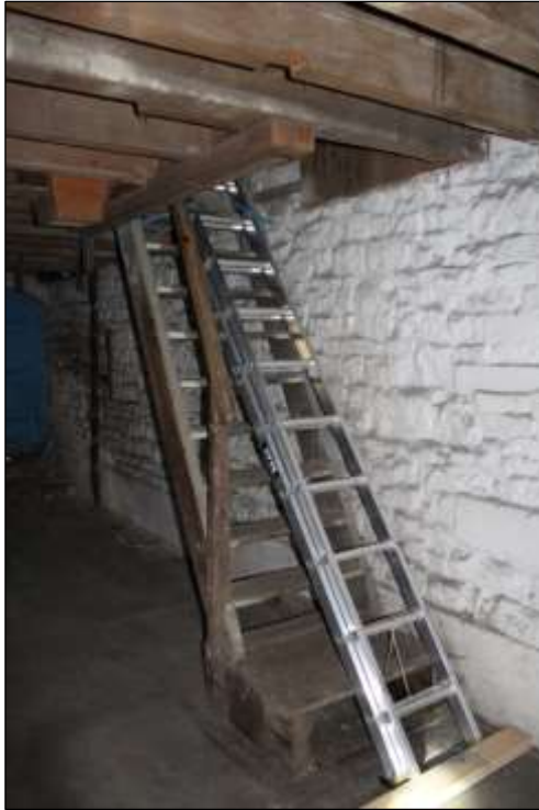
Fig.35 Ladder to lower storage floor (first floor)
