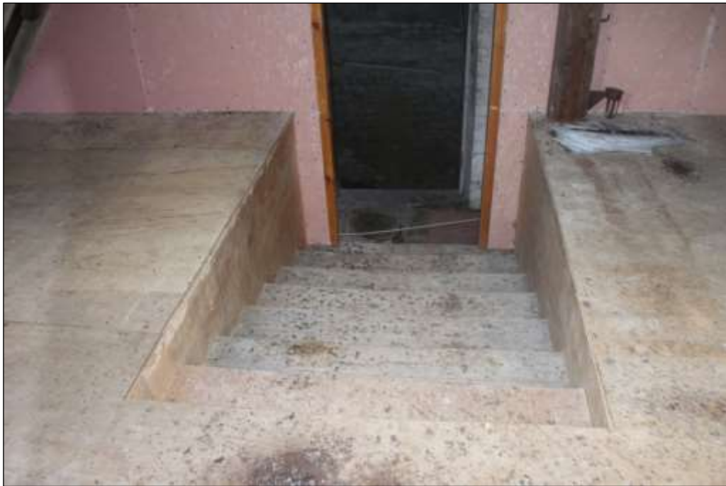
Fig.43 Shallow staircase to entrance of attic, with doorway to kiln void seen beyond
