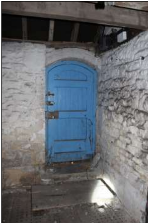
Fig.36 Doorway to southern (courtyard) elevation
