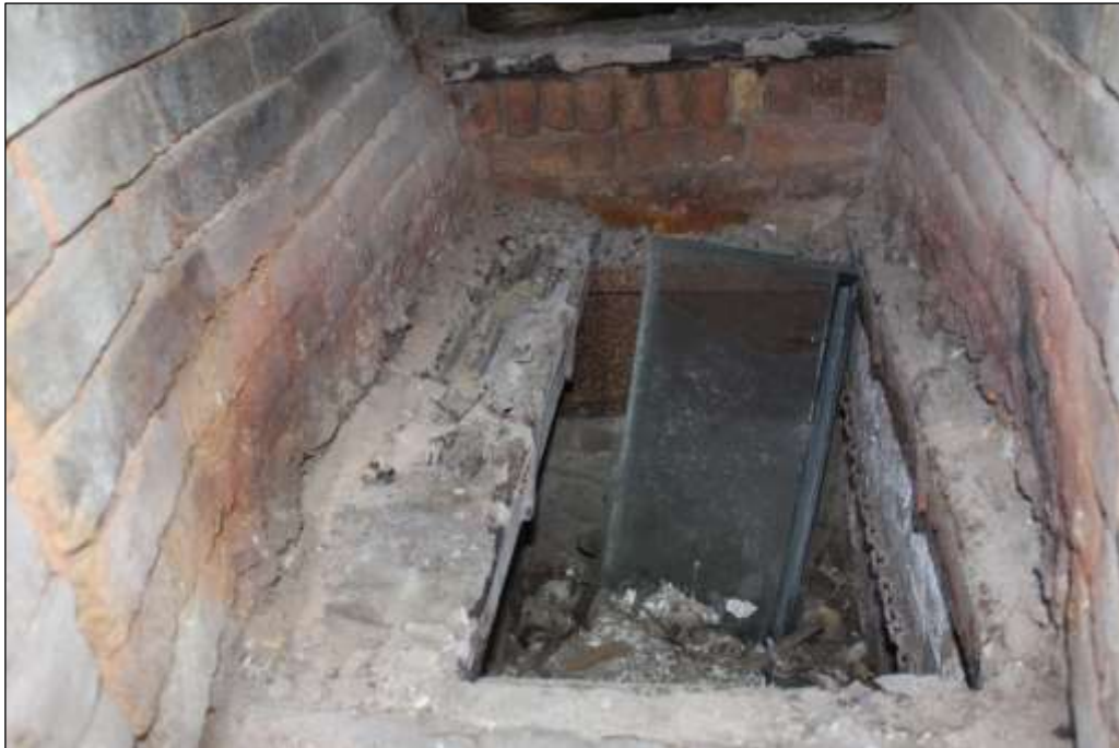
Fig.54 View inside furnace
