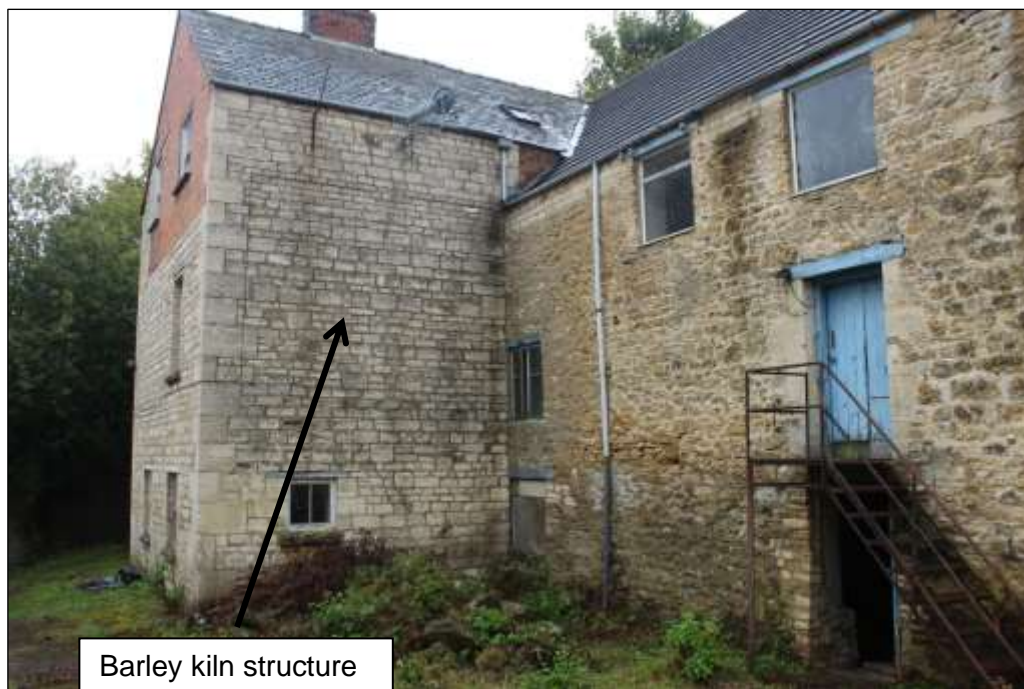
Fig.64 View of north-facing elevation of Maltings , image take towards the east
