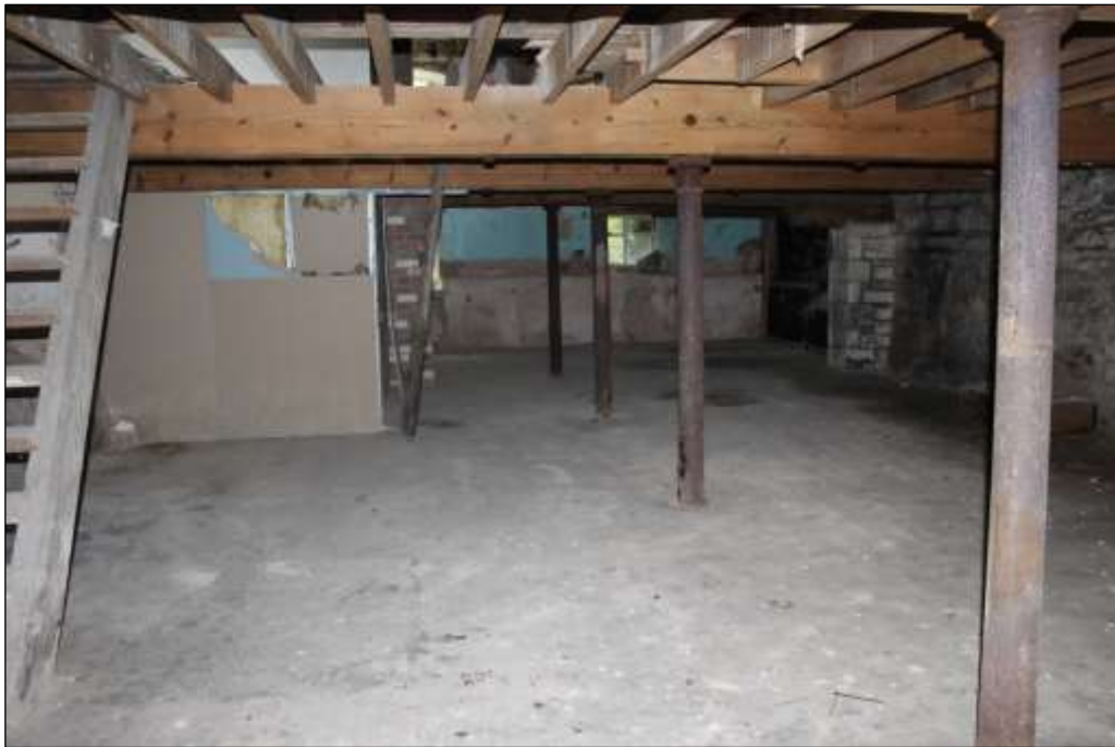
Fig.68 The lower growing floor of Maltings 2, view to the east, showing modern insertion of dividing walls
