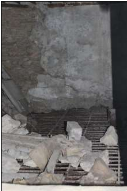
Fig.81 detail of metal lower drying floor of kiln in Maltings 2, this would have had a mesh covering when in use
