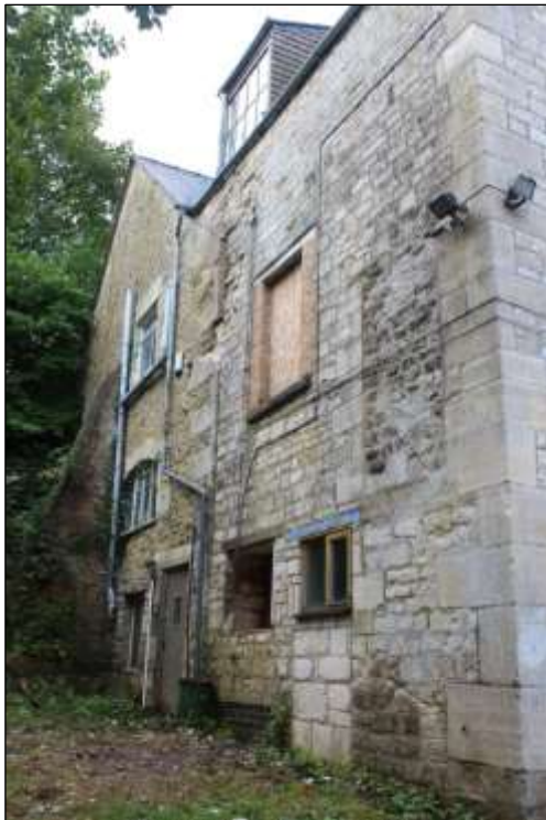
Fig.66 View of east elevation of Maltings 2
