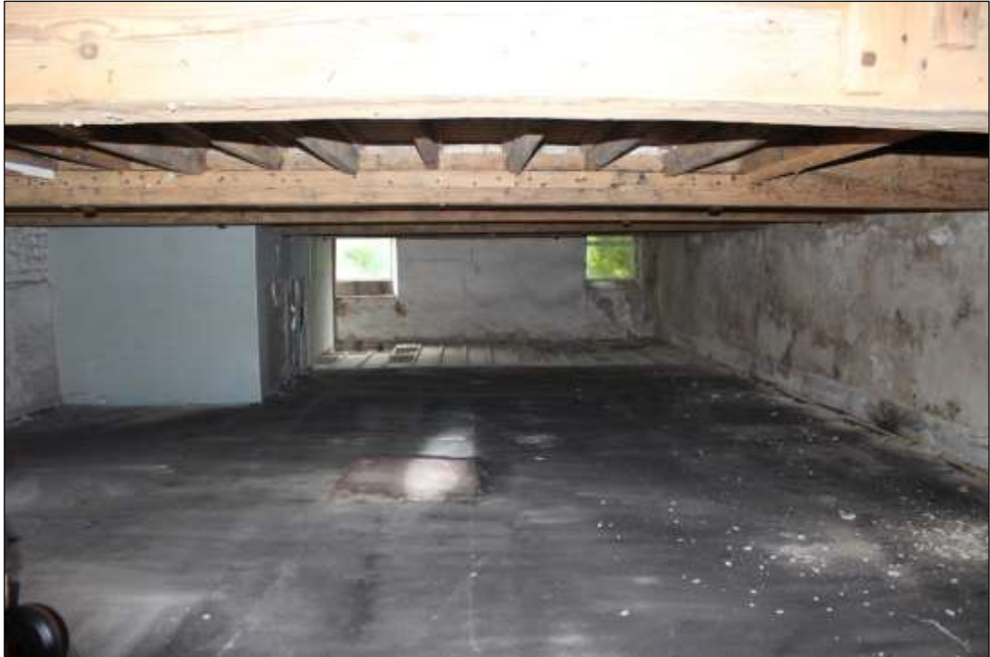
Fig.76 Upper storage floor (2nd floor) Maltings 2
