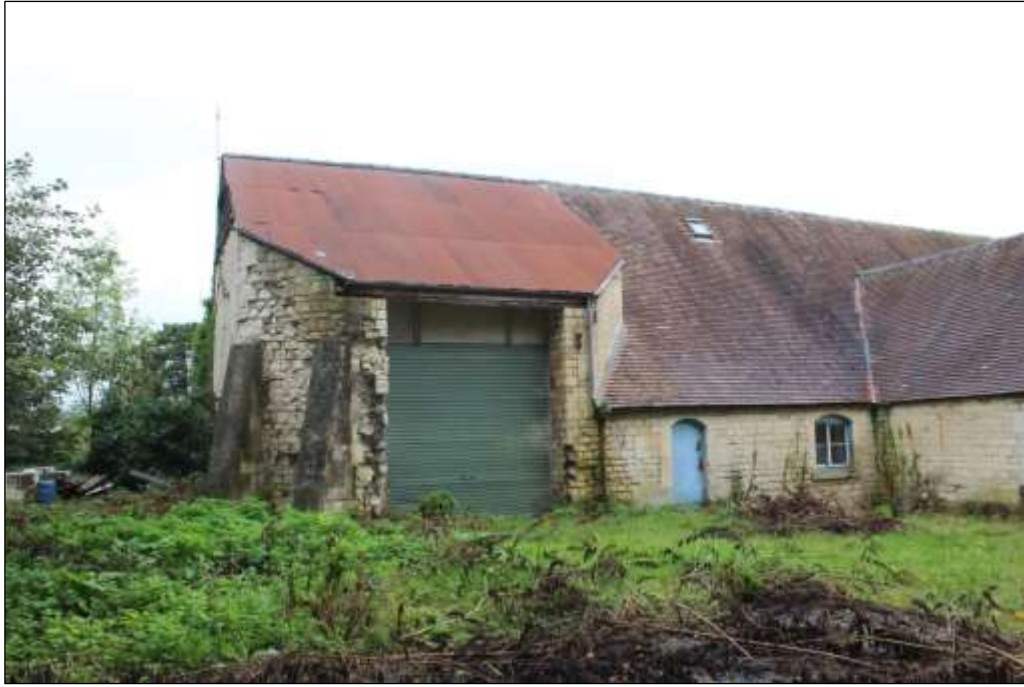
Fig.11 View towards the north of the kiln of Maltings 1
