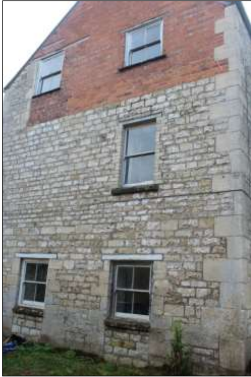
Fig. 65 View of barley kiln, north-facing elevation, on Maltings 2
