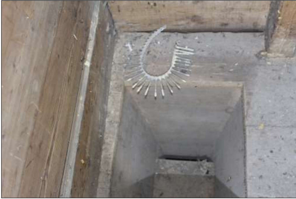
Fig.40 Funnel hatch in the lower storage floor (first floor)
