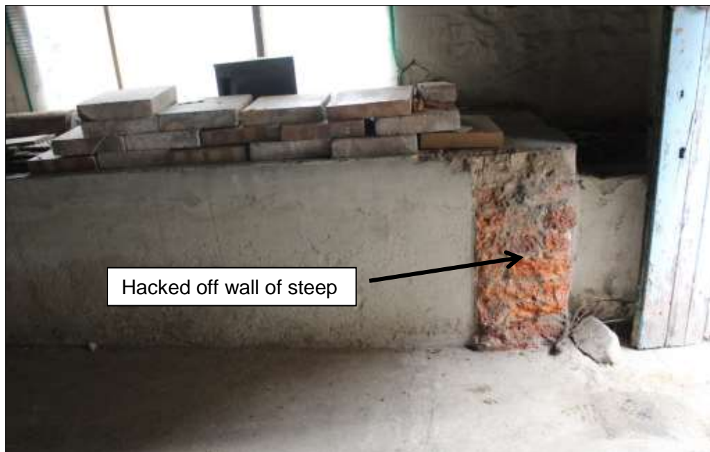
Fig.26 Hacked end of the steep which would have formed a rectangular 'bath'
