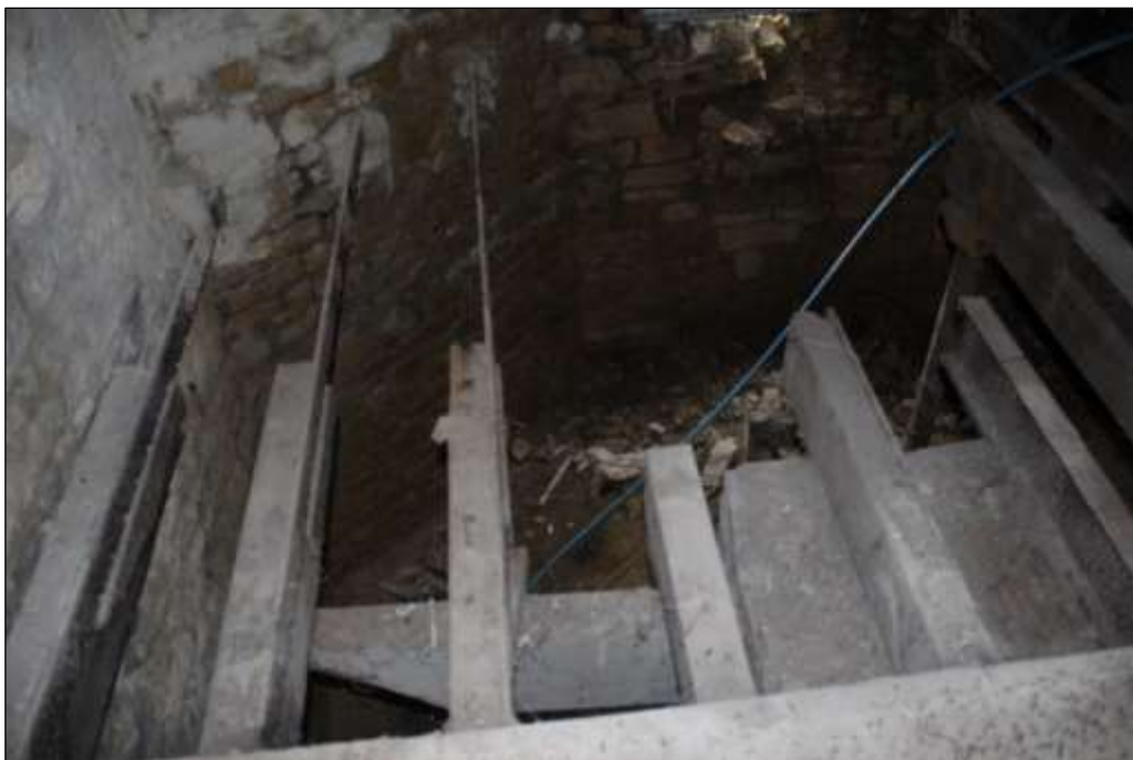
Fig.51 View of lower ground space of kiln from ground floor
