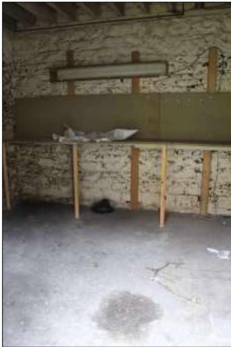
Fig.60 Internal view of crosswing building looking north
