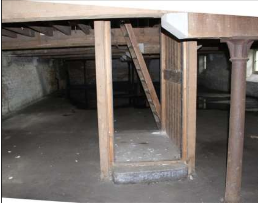
Fig.22 image of hoist equipment and hatch on lower growing floor of Maltings 1
