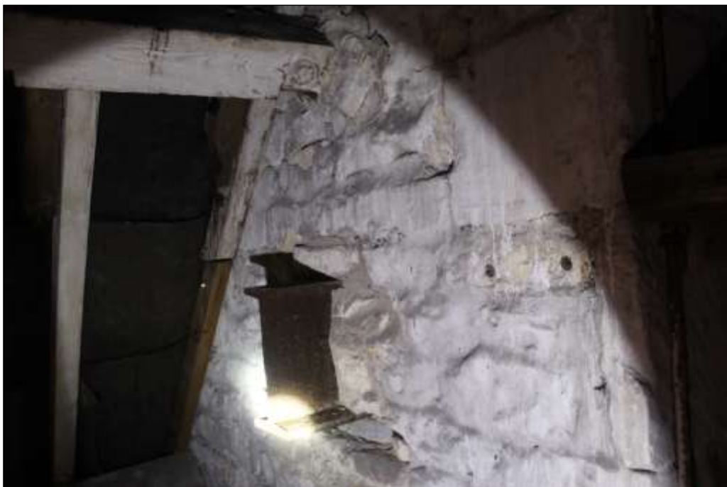
Fig.41 View of kiln end wall, showing various insertions and additions
