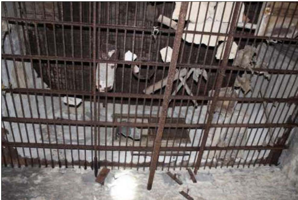
Fig.85 Looking upwards into the body of the kiln, showing the metal floor and wire mesh floor above
