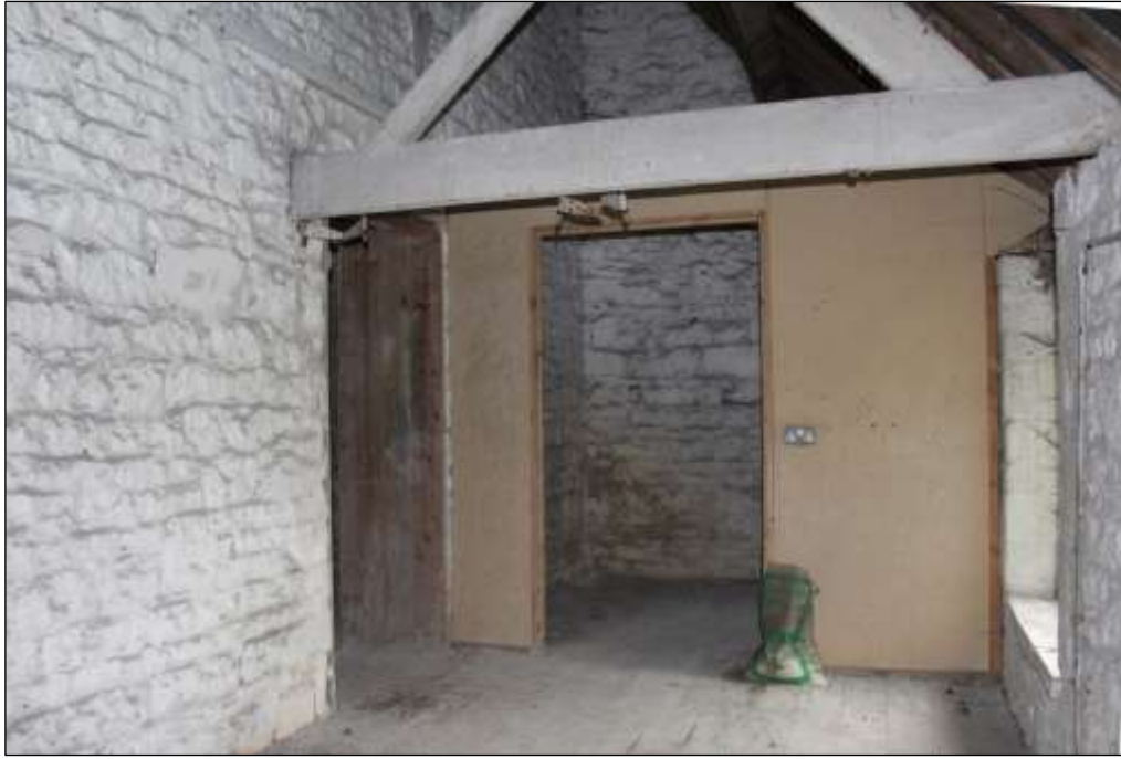
Fig.46 Kiln anteroom, ground floor, with modern partition and toilet behind
