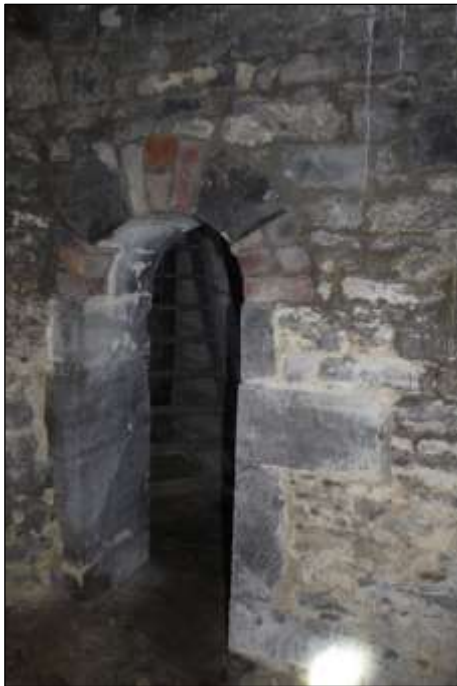
Fig.58 View of side entrance to interior of the kiln
