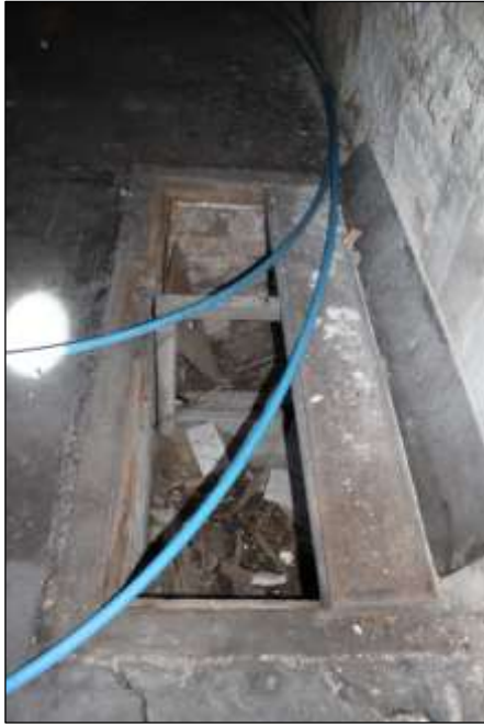
Fig.24 Floor hatch with bricked out hole, lower growing floor Maltings 1
