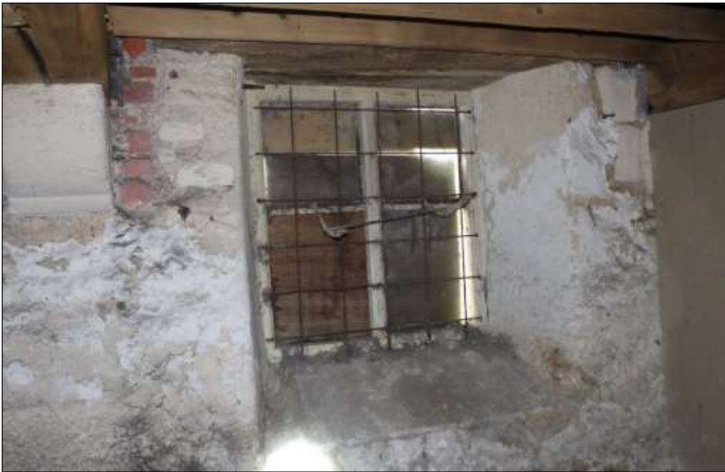
Fig.70 Detail of window also showing brick infill around the stone corbel
