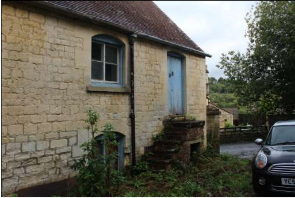
Fig.15 View to the east of the eastern section of Maltings 1
