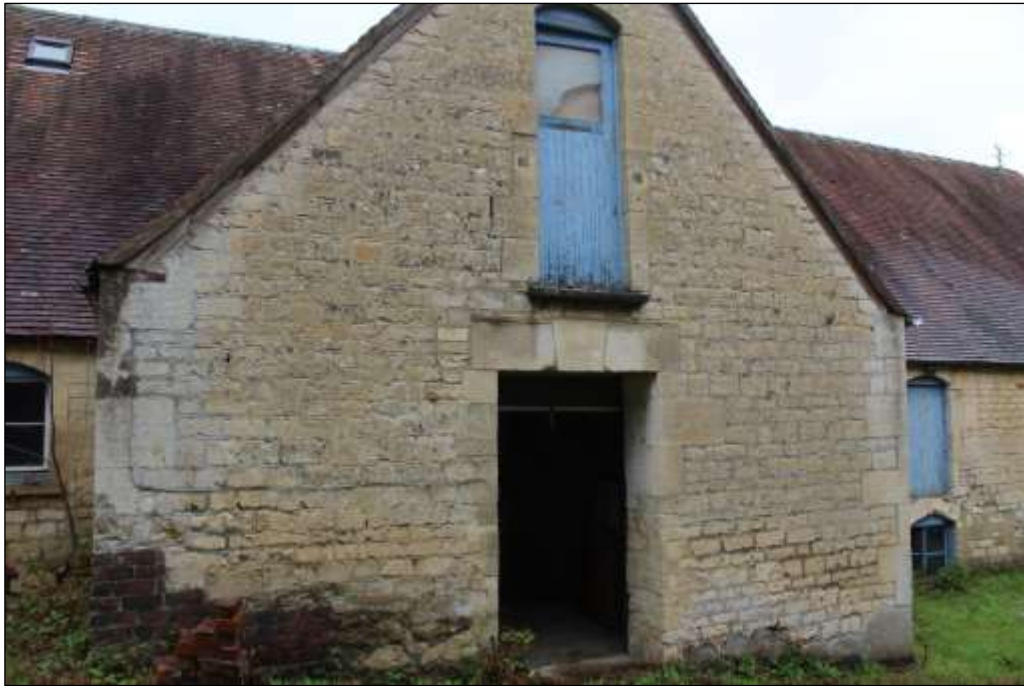
Fig.13 View of the cross-wing of Maltings 1, image taken looking north
