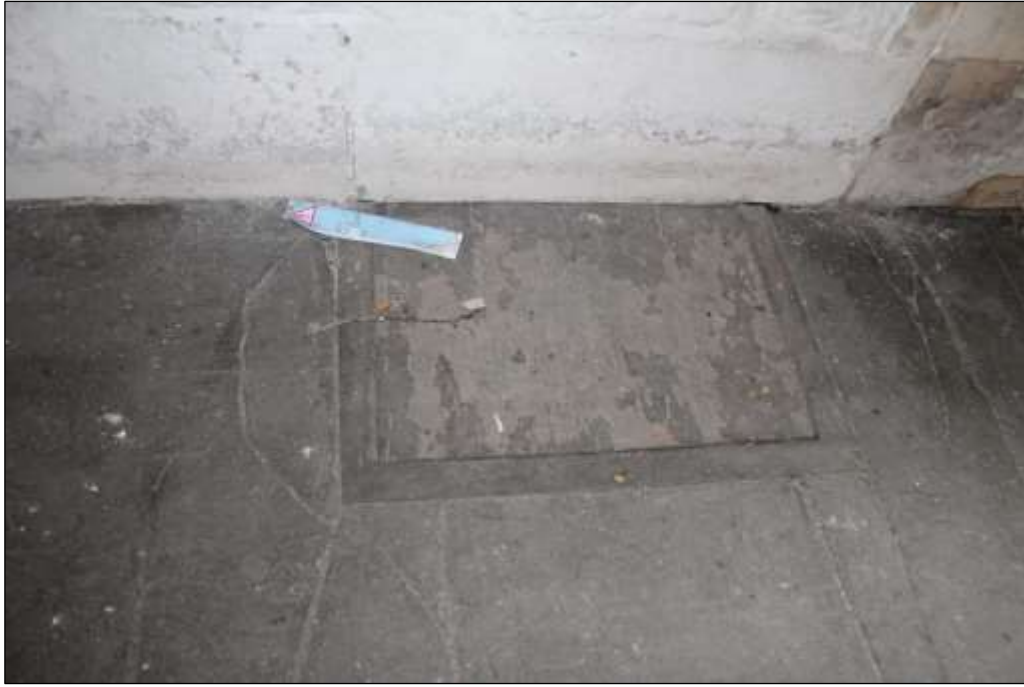
Fig.31 Hatch onto lower ground floor ladder, located in upper growing floor
