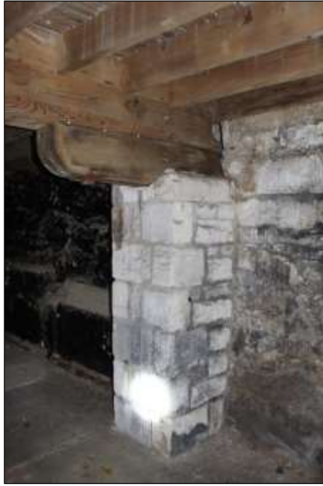
Fig.69 Stone pillar with wooden pad to support beam
