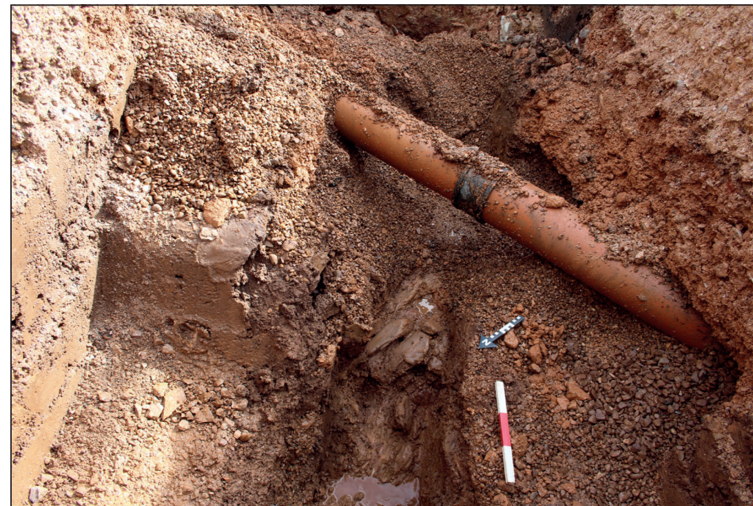
Feature 212 and modern service pipe, looking south-west (0.3m scale)
