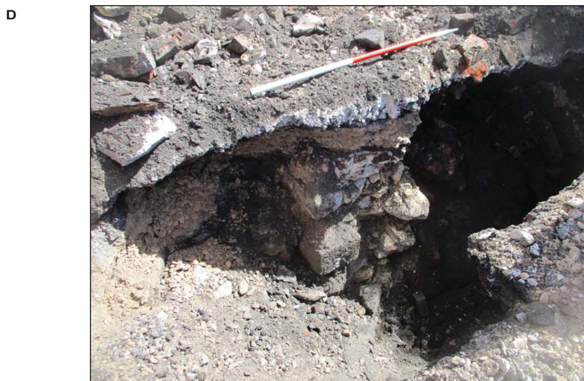
Wall 304, facing east (1m scale)
