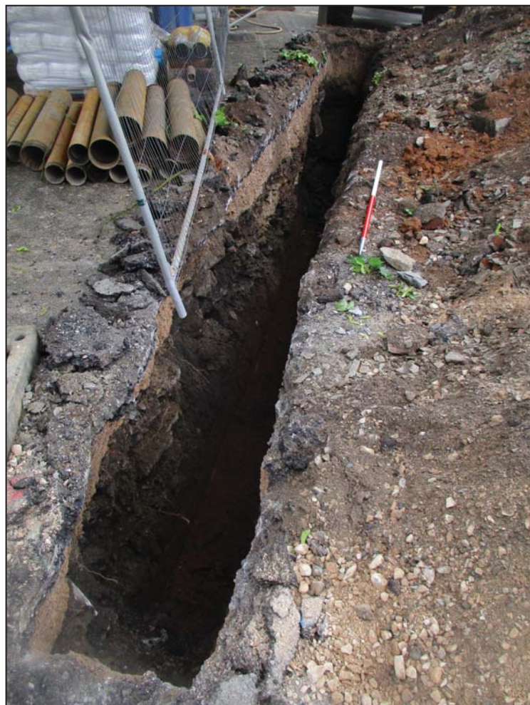
Trench 1 overview, facing north-west (1m scale)
