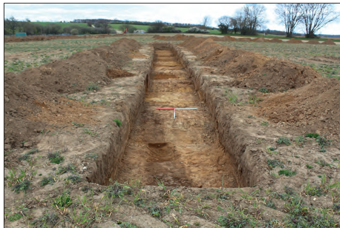
Trench 17, looking north (1m scales)
