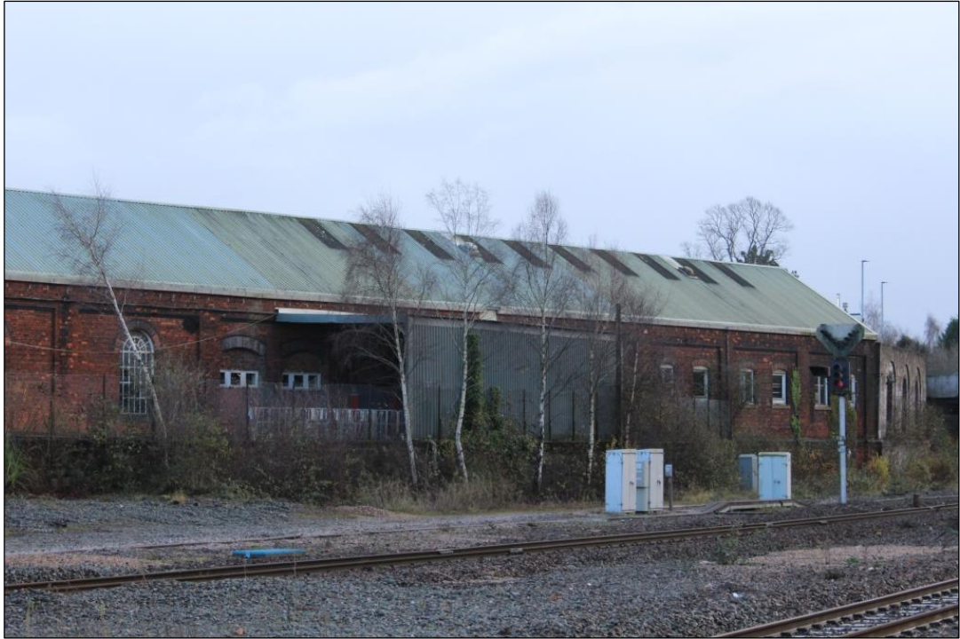
Photograph 15 View of the canopy off centre to the south on the west elevation
