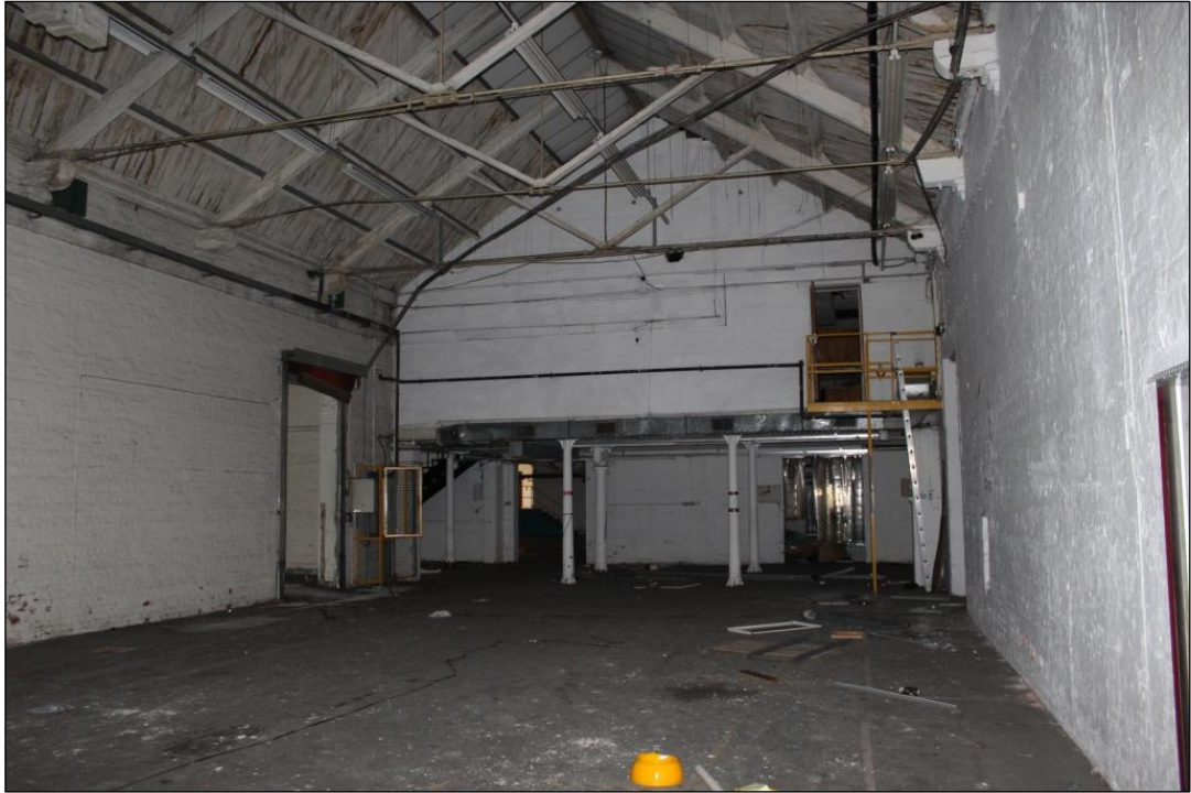
Photograph 21 Mezzanine in room 3 supported on pillars
