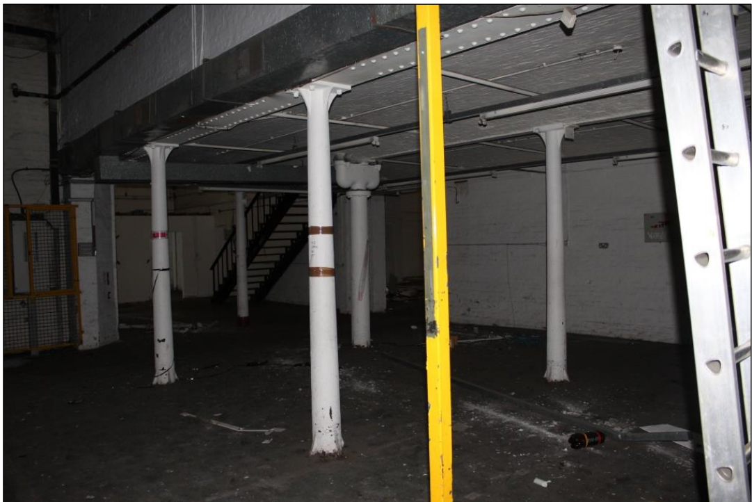
Photograph 22 Detailed view of the pillars supporting the mezzanine
