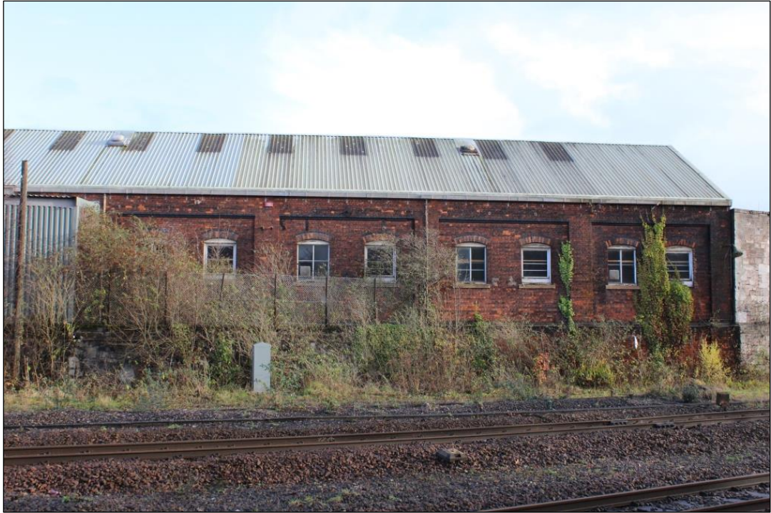
Photograph 17 View of the southern part of the west elevation
