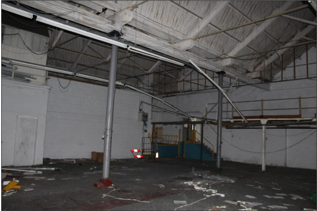
Photograph 23 General view of room 4 looking to the south-east
