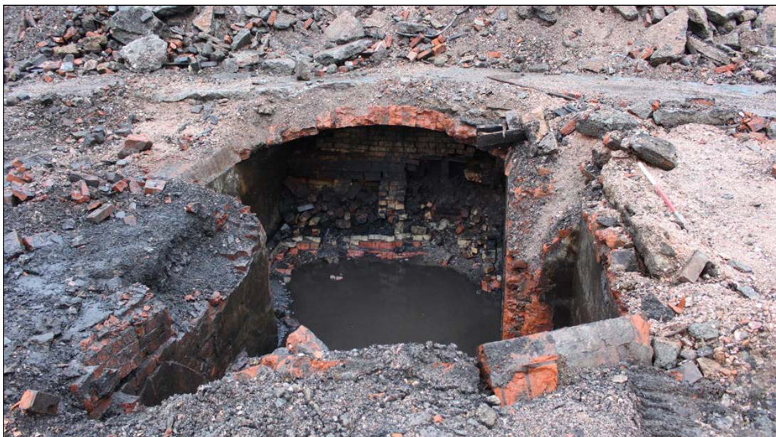
Photograph 28 Basement 105 with furnaces in the background, facing north
