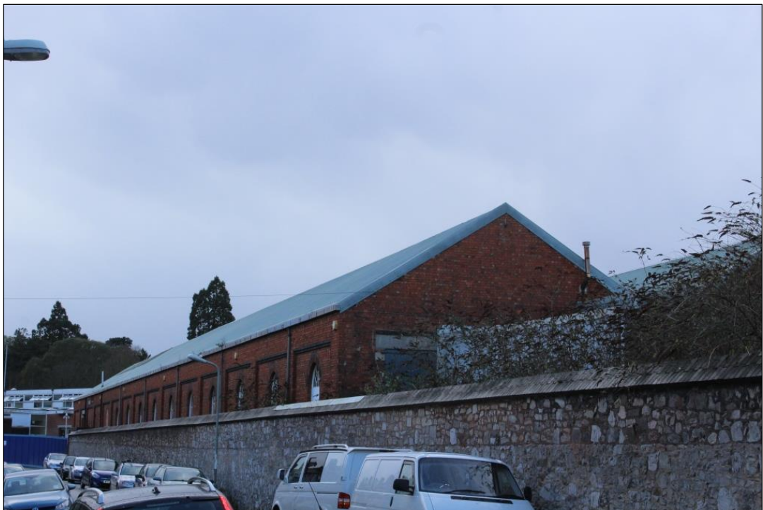
Photograph 6 General view of the east elevation with the stone boundary wall
