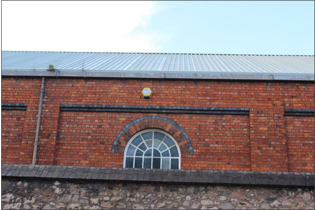
Photograph 7 Sample of the recessed walling with an arched window
