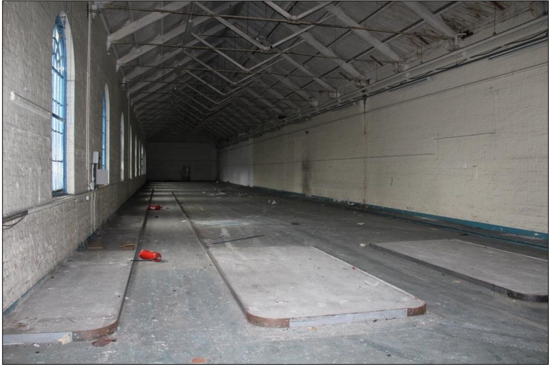
Photograph 20 General view of the room 2 looking to the south-west
