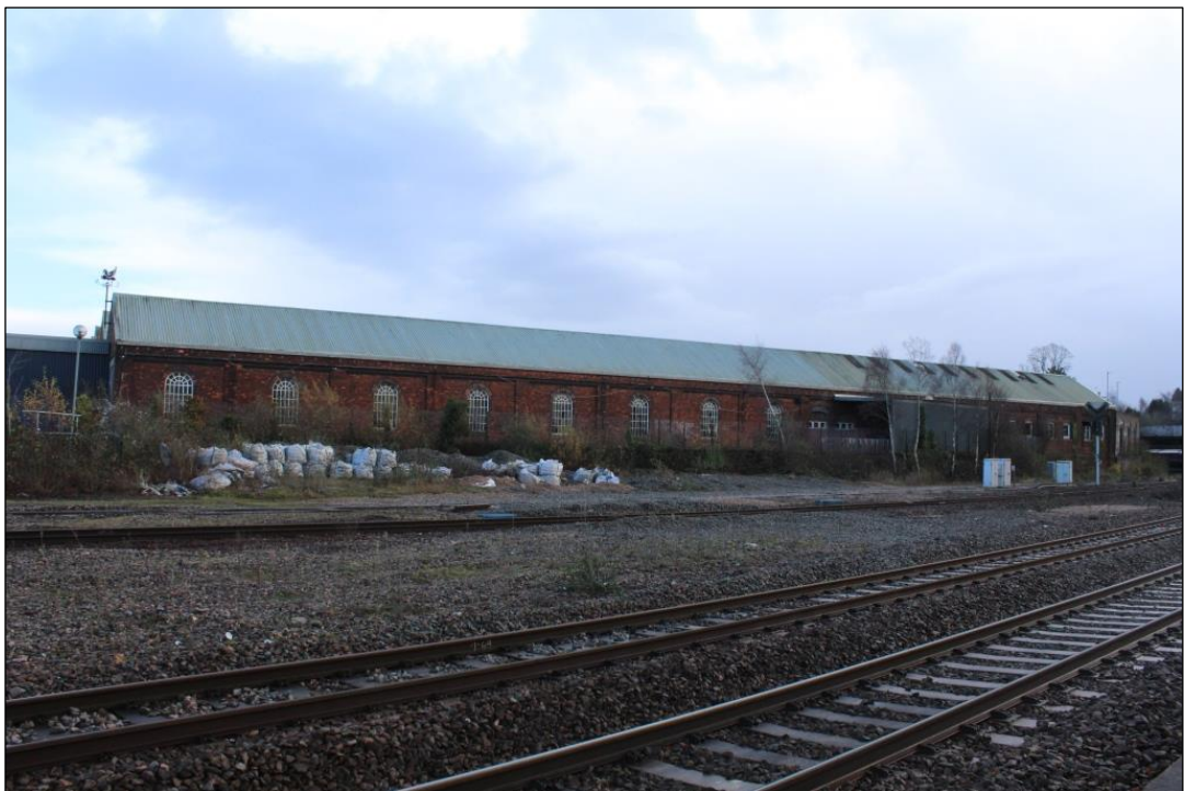
Photograph 14 General view of the west elevation taken from the Station car park
