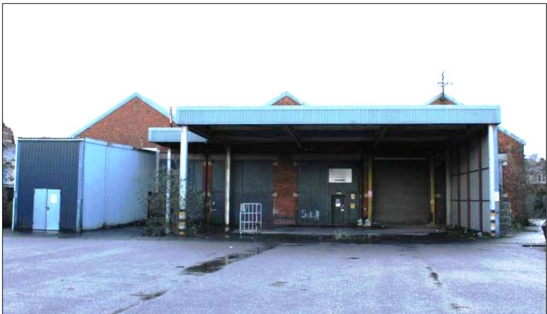
Photograph 1 General view of the north Elevation
