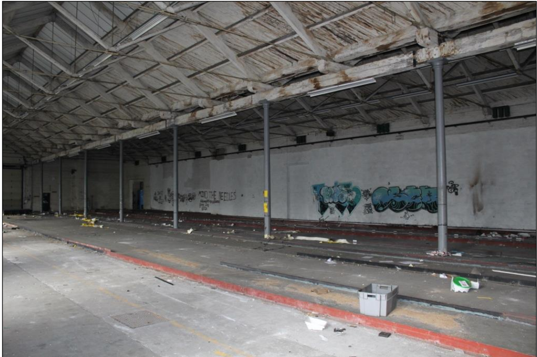
Photograph 19 General view of the room 1 looking to the north-east
