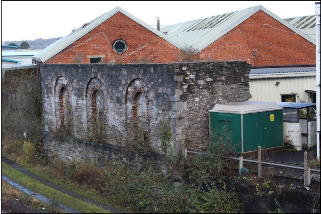
Photograph 10 View of the south elevation from the adjacent railway bridge showing the three gables and remnants of the former roof of the adjacent structure (Building B) and circular window in the western gable
