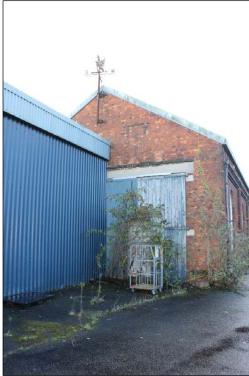
Photograph 4 Western edge of the north elevation with the overlapping of the later canopy and Pegasus weather vane
