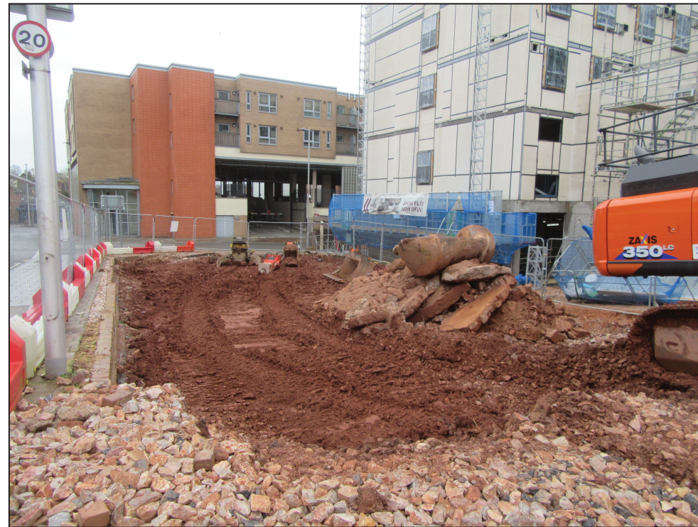
Area 2 western end, looking south
