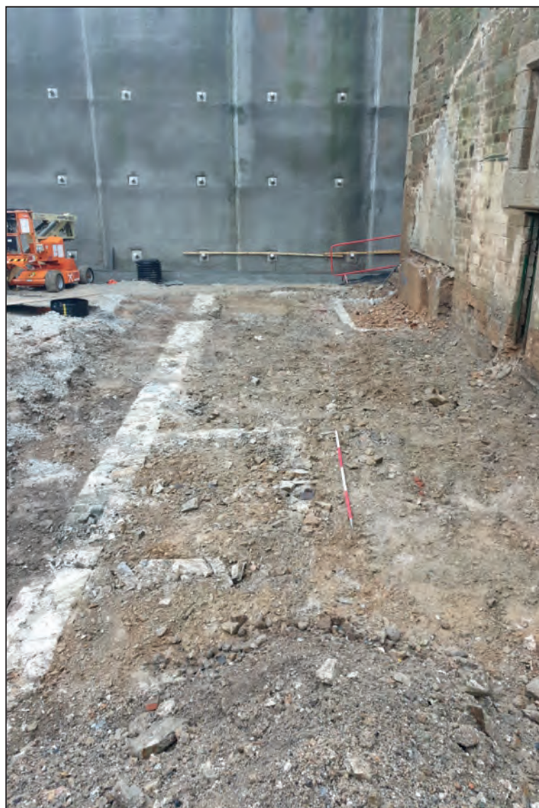
Trench 142b, showing wall 14206, looking north-west (2m scale)
