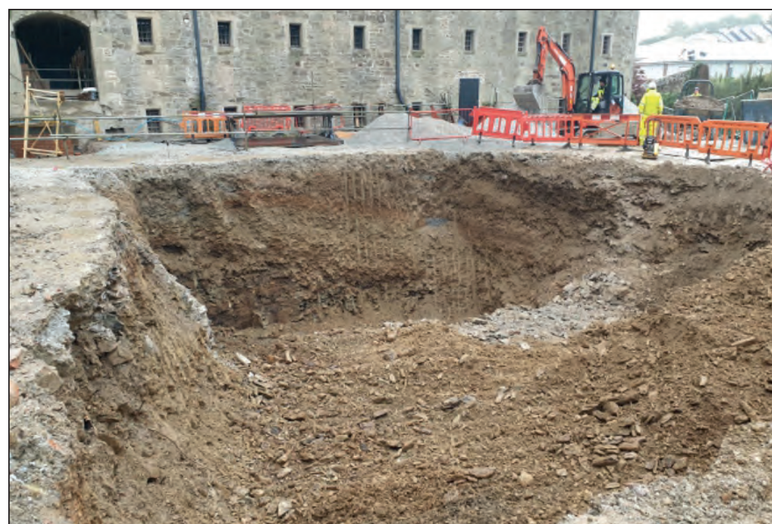
Trench 140, looking east
