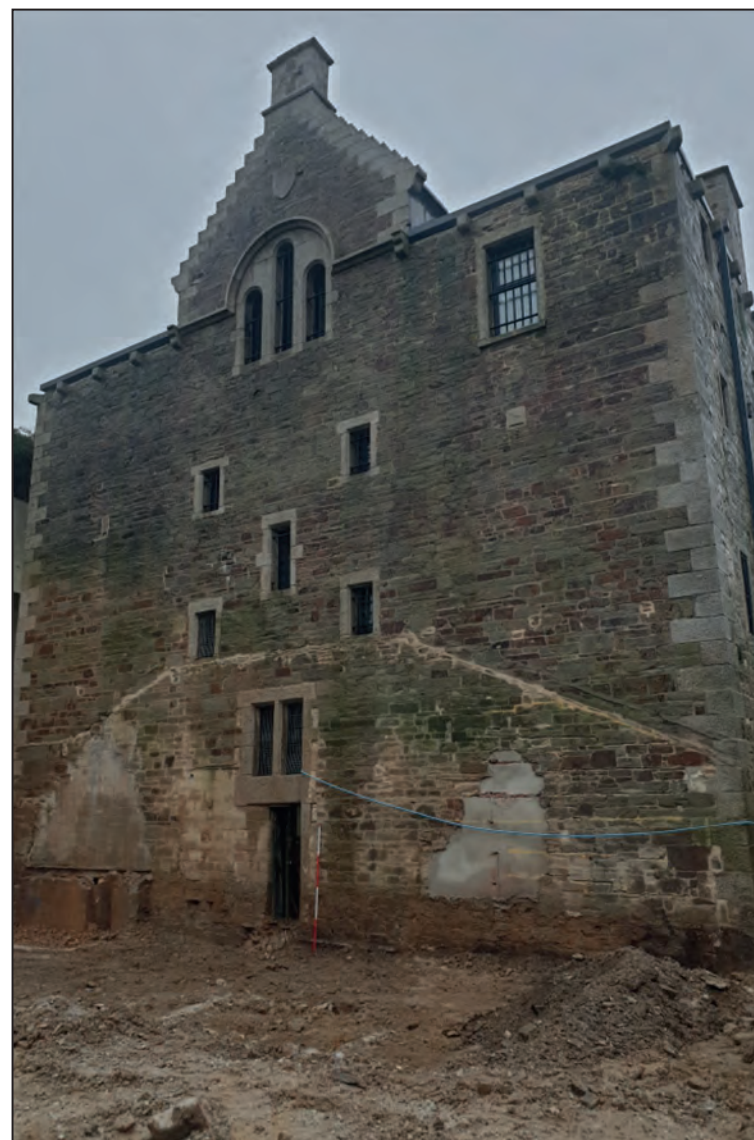
Trench 142b, showing former laundry building, looking north-east (2m scale)
