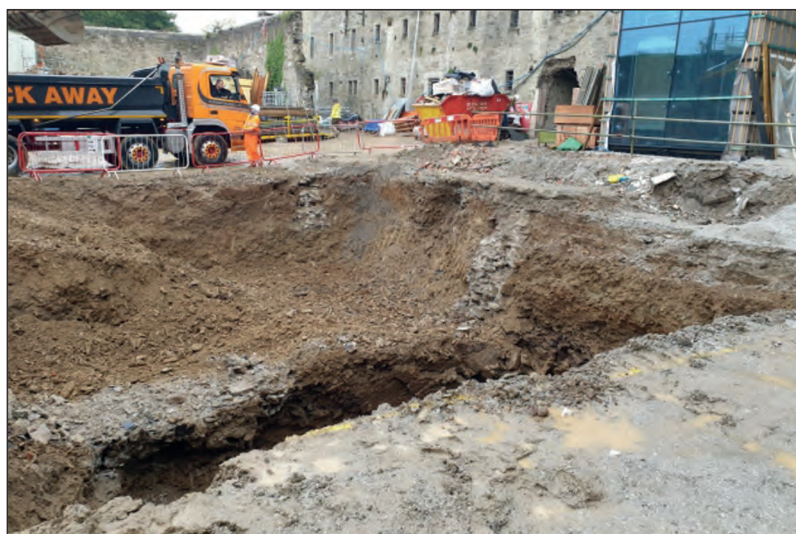
Trench 140 showing wall 14007 (centre) and 140009 (left), looking west
