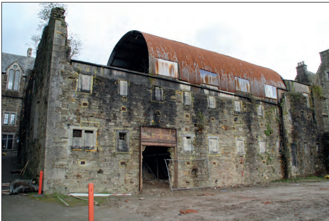
South elevation of the Hospital Block, looking north-east
