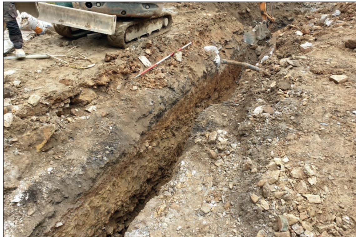
Trench 142a, looking south-east (2m scale)
