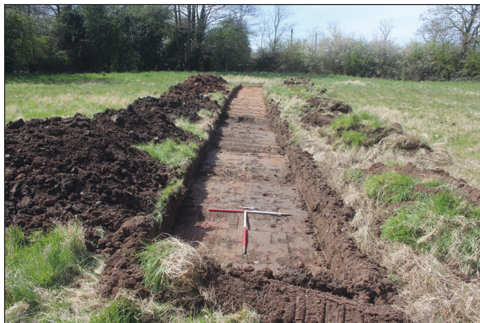
Trench 4, looking west (1m scales)
