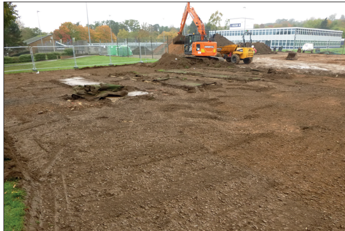
Area 53 initial ground reduction, looking south-east
