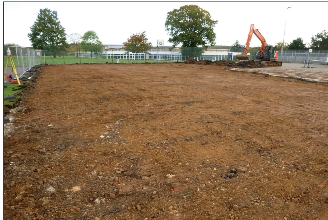
Area 52 initial ground reduction, looking east
