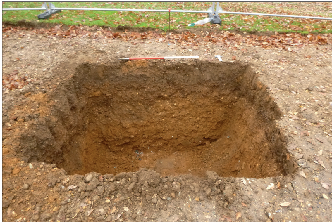
Trench 46 foundation pad, looking north (1m scale)
