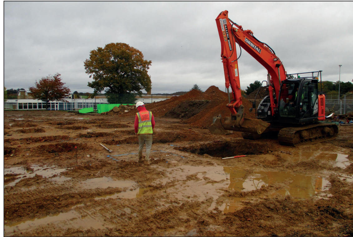
Excavation of foundation pads, looking east
