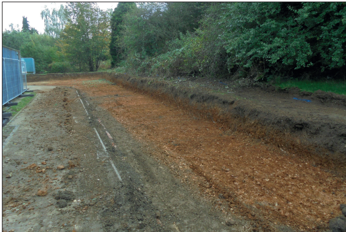
Area 1 haul road, looking south-east
