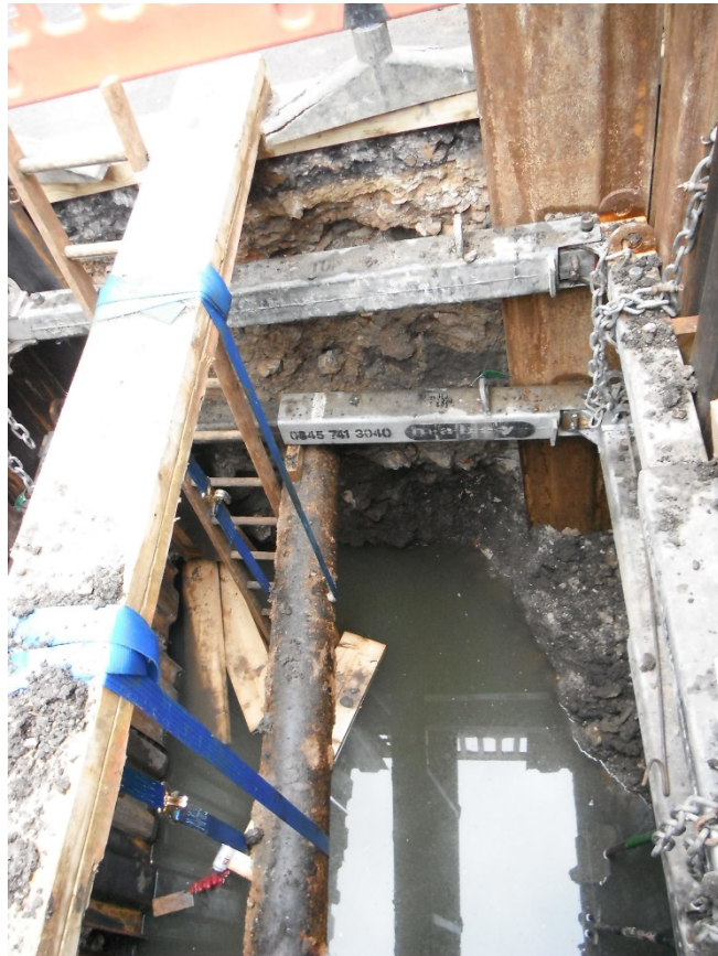
Photo 1: The trench, showing modern deposits including the compacted limestone rubble
