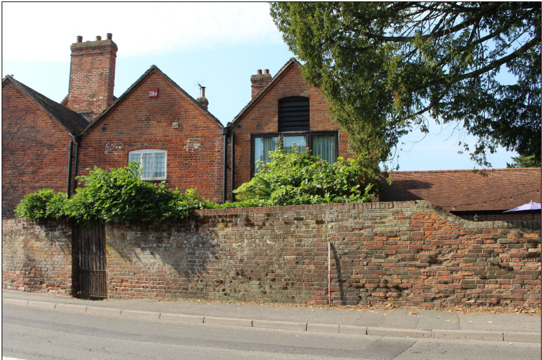
Photo 34: Sections 3 to 6 of the eastern elevation.
