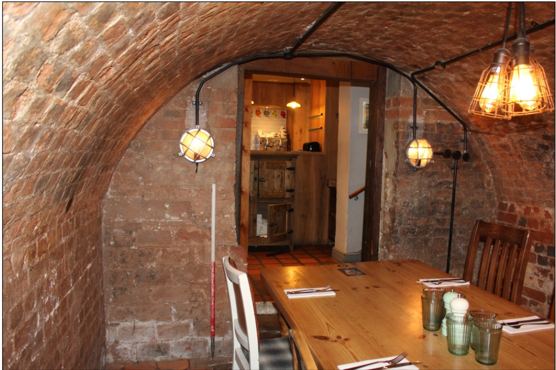
Photo 13: The view south towards the beam from within the cellar vault.
