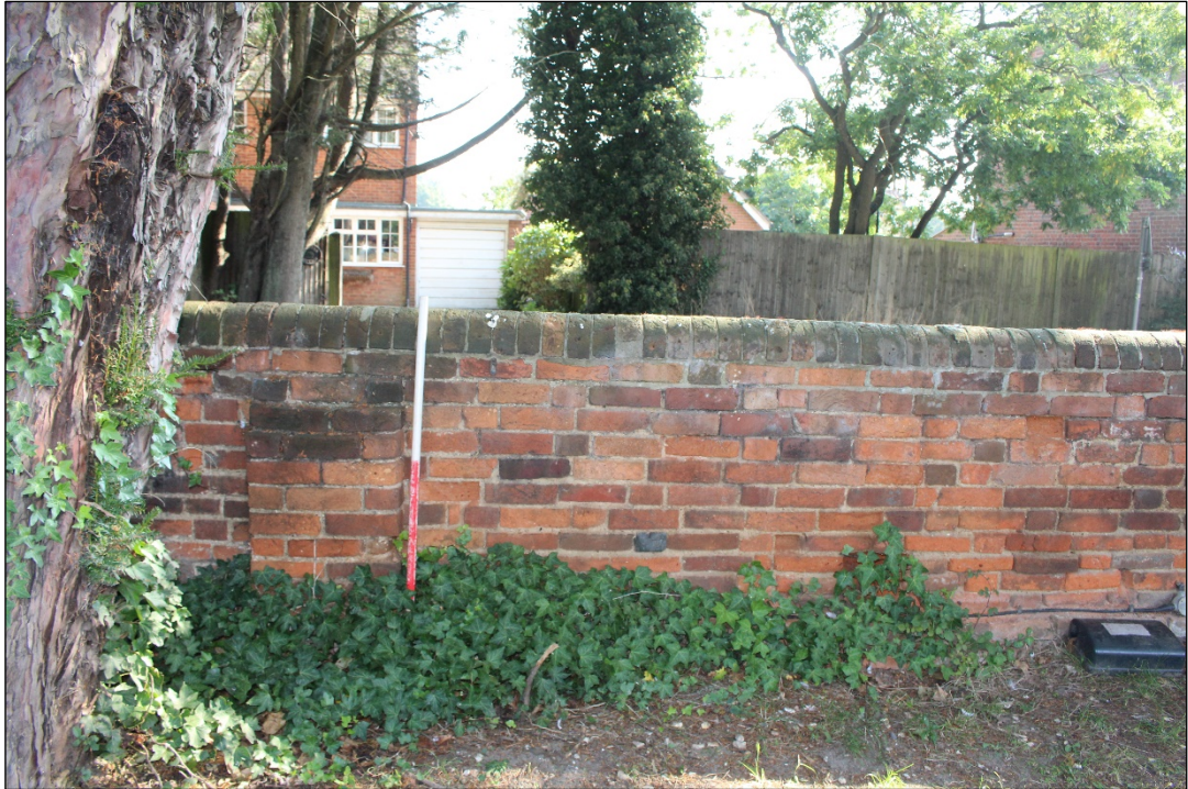
Photo 41: The northern extent of the boundary wall from the west.
