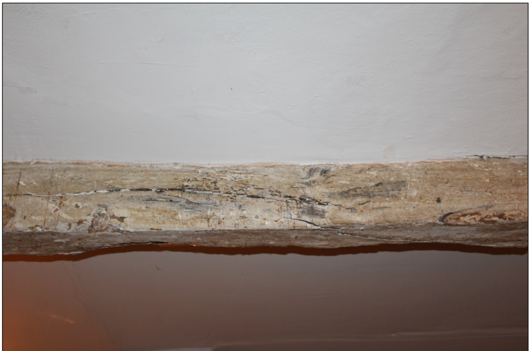
Photo 16: The eastern extent of a central part of the timber beam.
