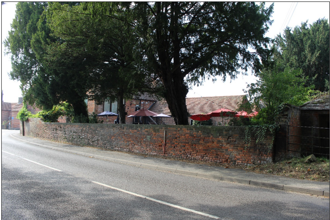
Photo 24: The eastern elevation of the boundary wall from the north-east.
