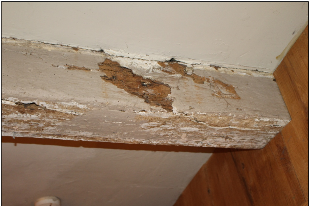
Photo 21: The southern extent of the timber beam from the north-west.
