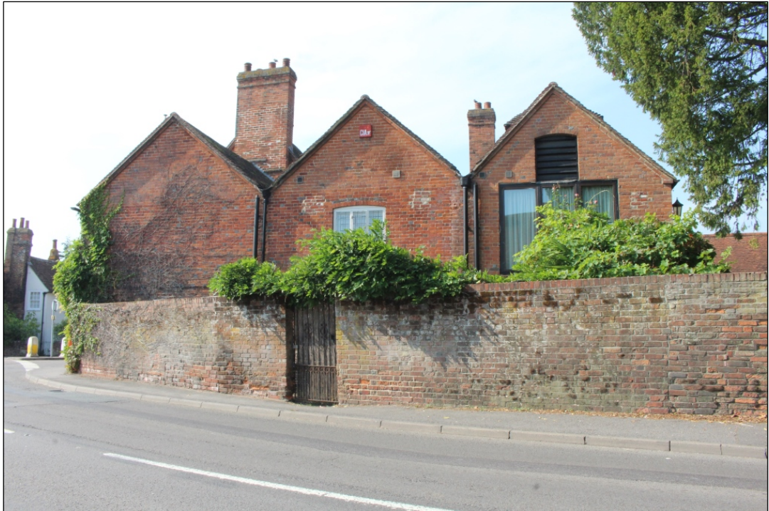
Photo 3: The eastern elevation of The Hinds Head.
