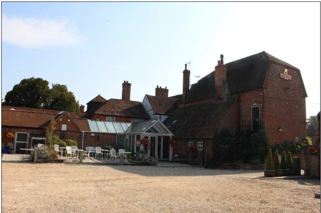
Photo 4: The northern elevation from the north-west.
