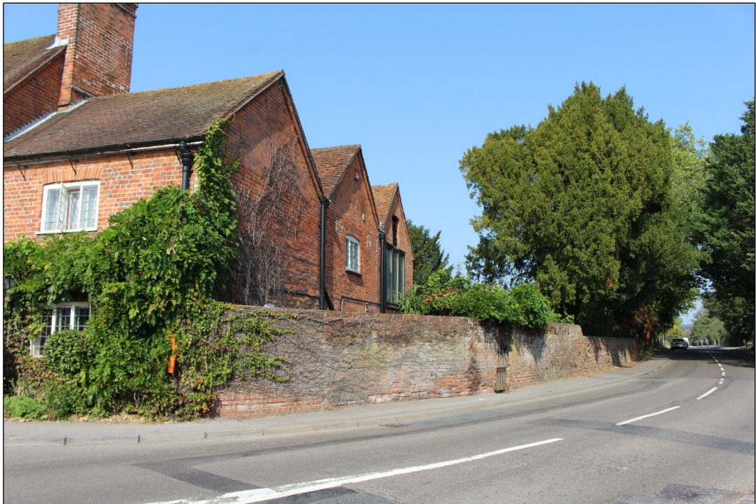
Photo 22: The eastern elevation of the boundary wall from the south-east.
