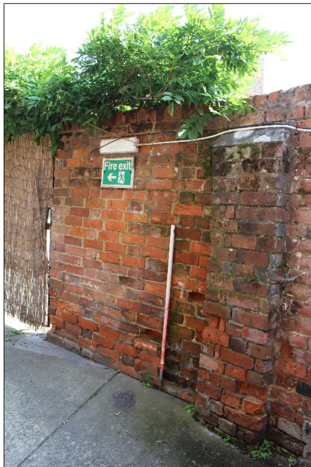
Photo 29: Section 3 of the western elevation from the south-west.
