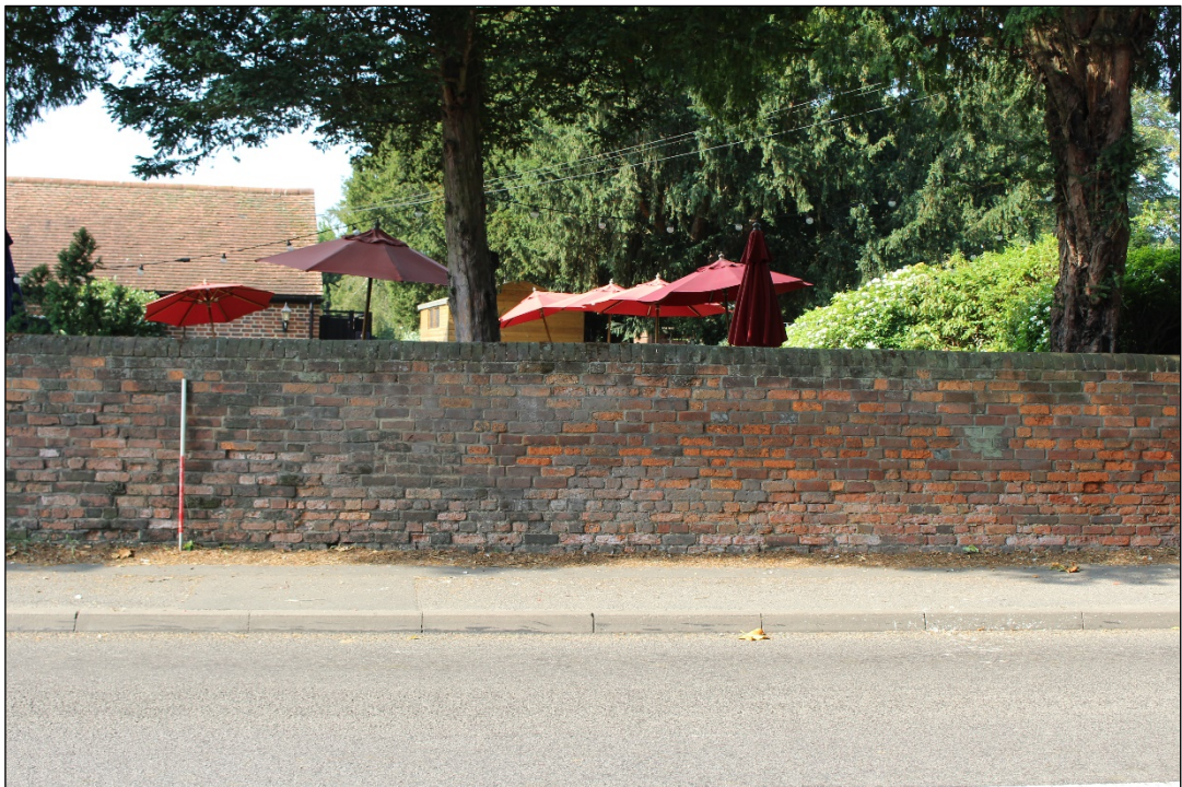
Photo 38: The central part of the eastern elevation of Section 7.
