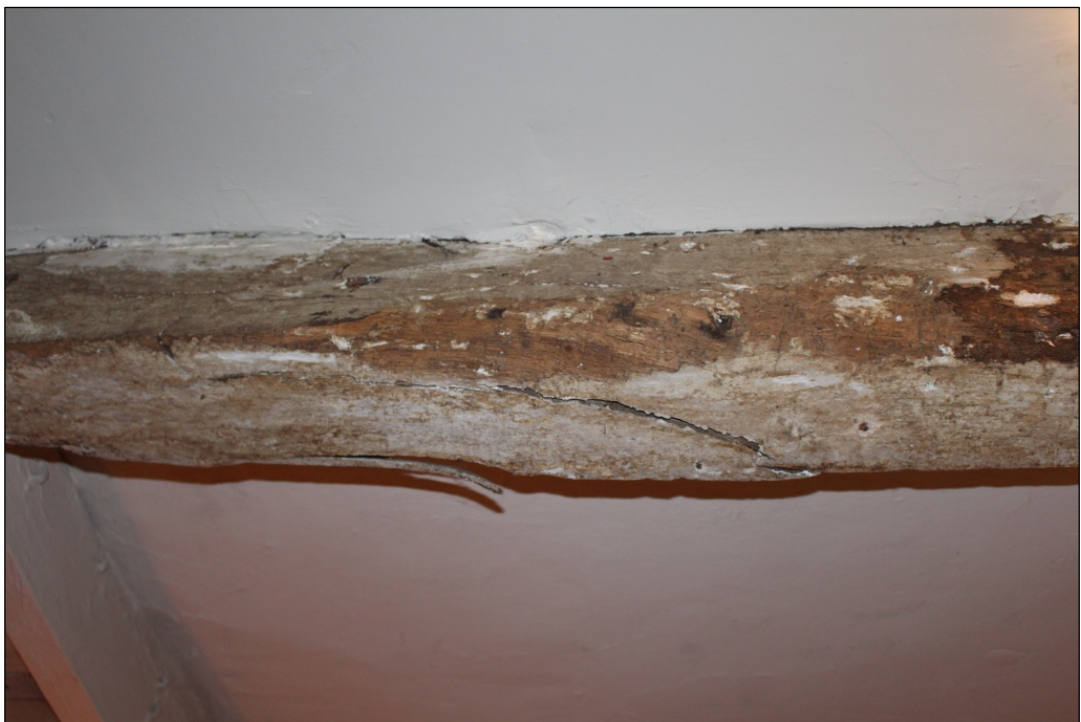
Photo 18: Detail of the timber beam from the west.
