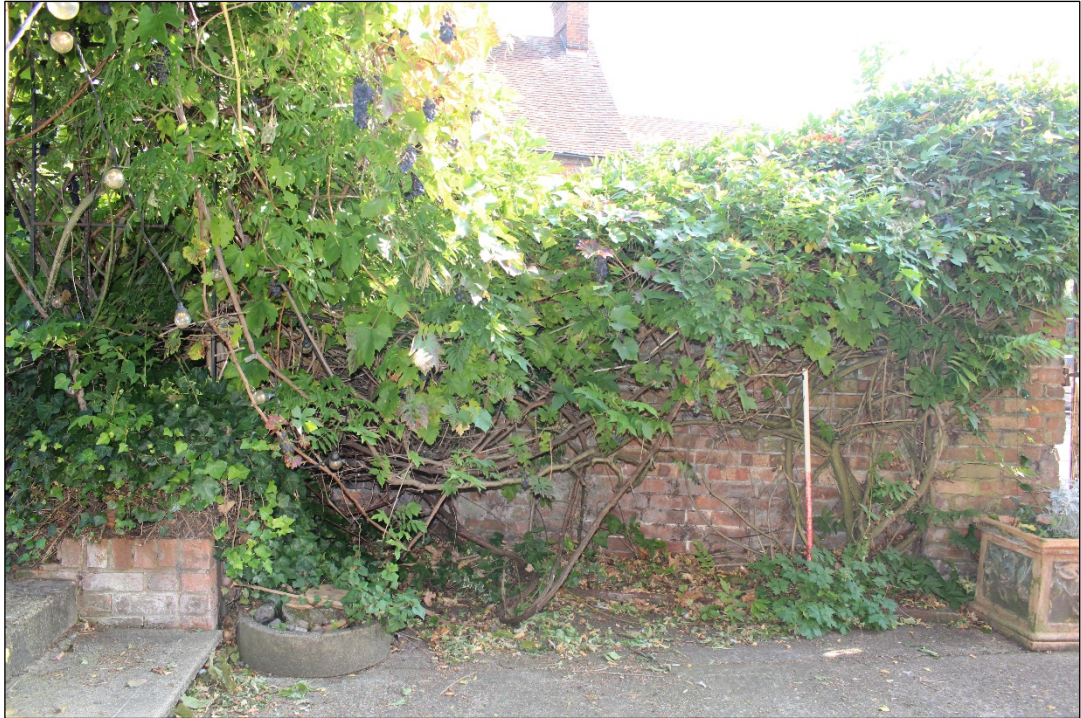
Photo 31: Section 4 of the western elevation from the west.
