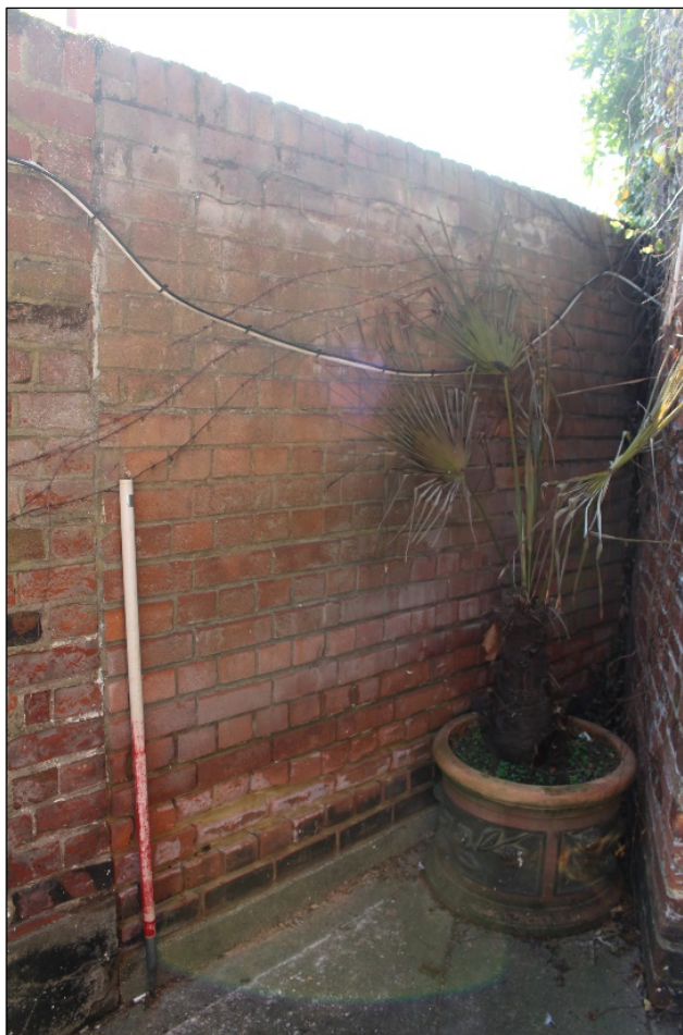
Photo 26: Section 1 of the western elevation from the north-west.
