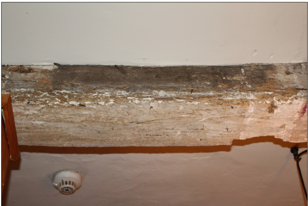
Photo 19: The southern half of the timber beam from the west.
