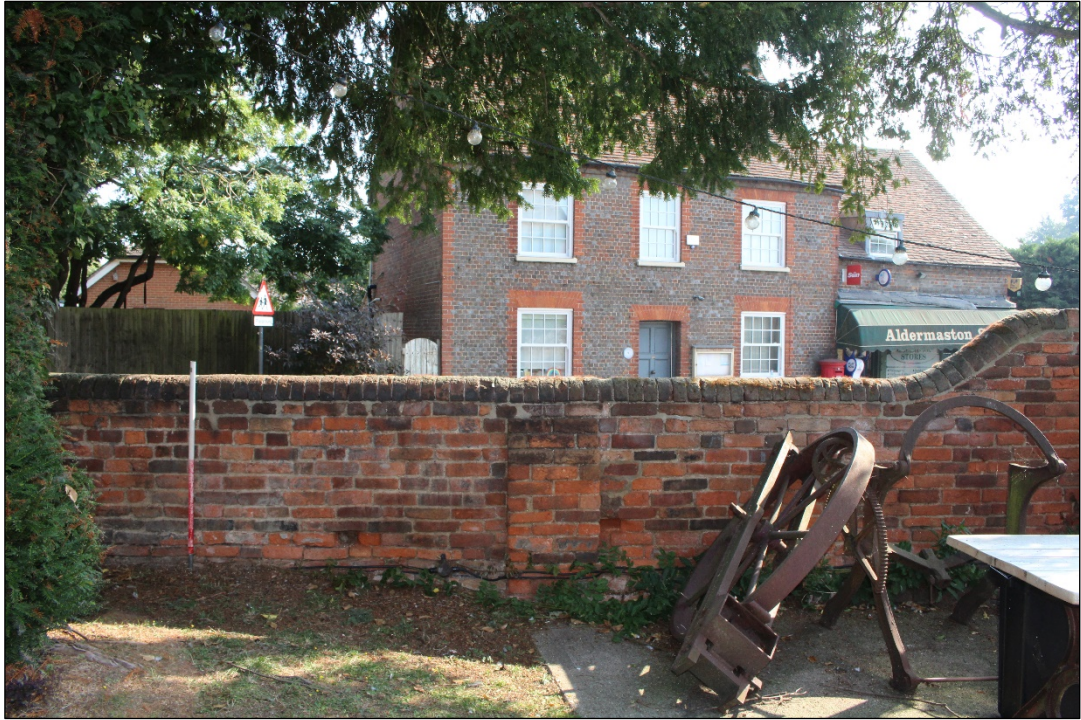
Photo 43: The southern extent of Section 7 where it increases in height to 1.6 metres within Section 6.
