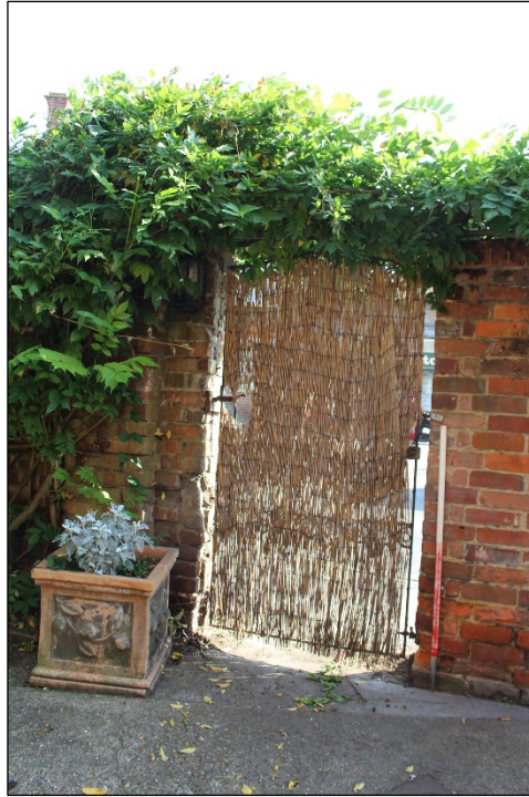
Photo 30: Door opening between Sections 3 and 4 of the western elevation.
