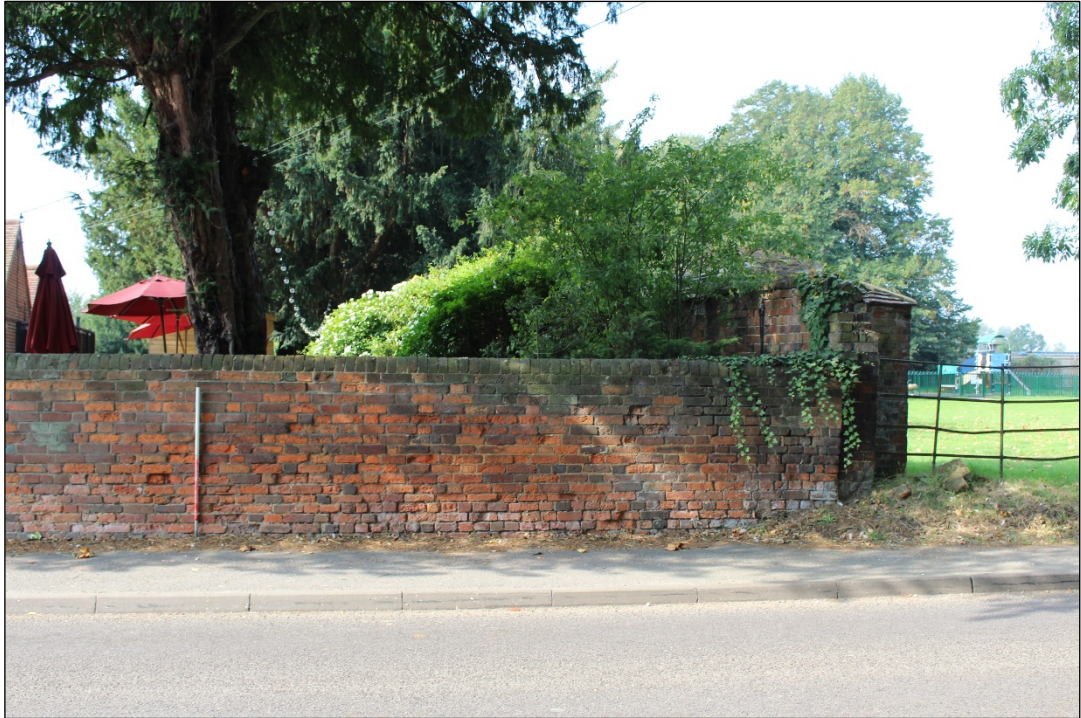
Photo 39: The northern extent of the eastern elevation of Section 7.
