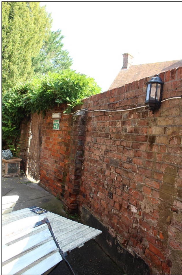
Photo 27: Sections 2 and 3 of the western elevation from the south-west.
