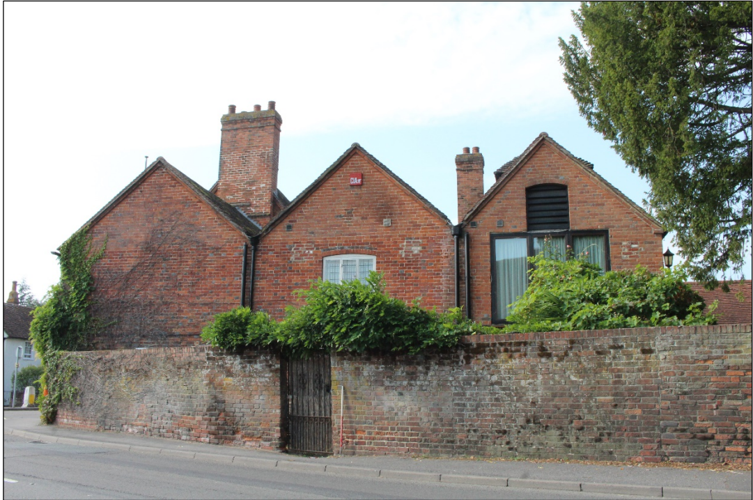
Photo 23: The eastern elevation from the east.
