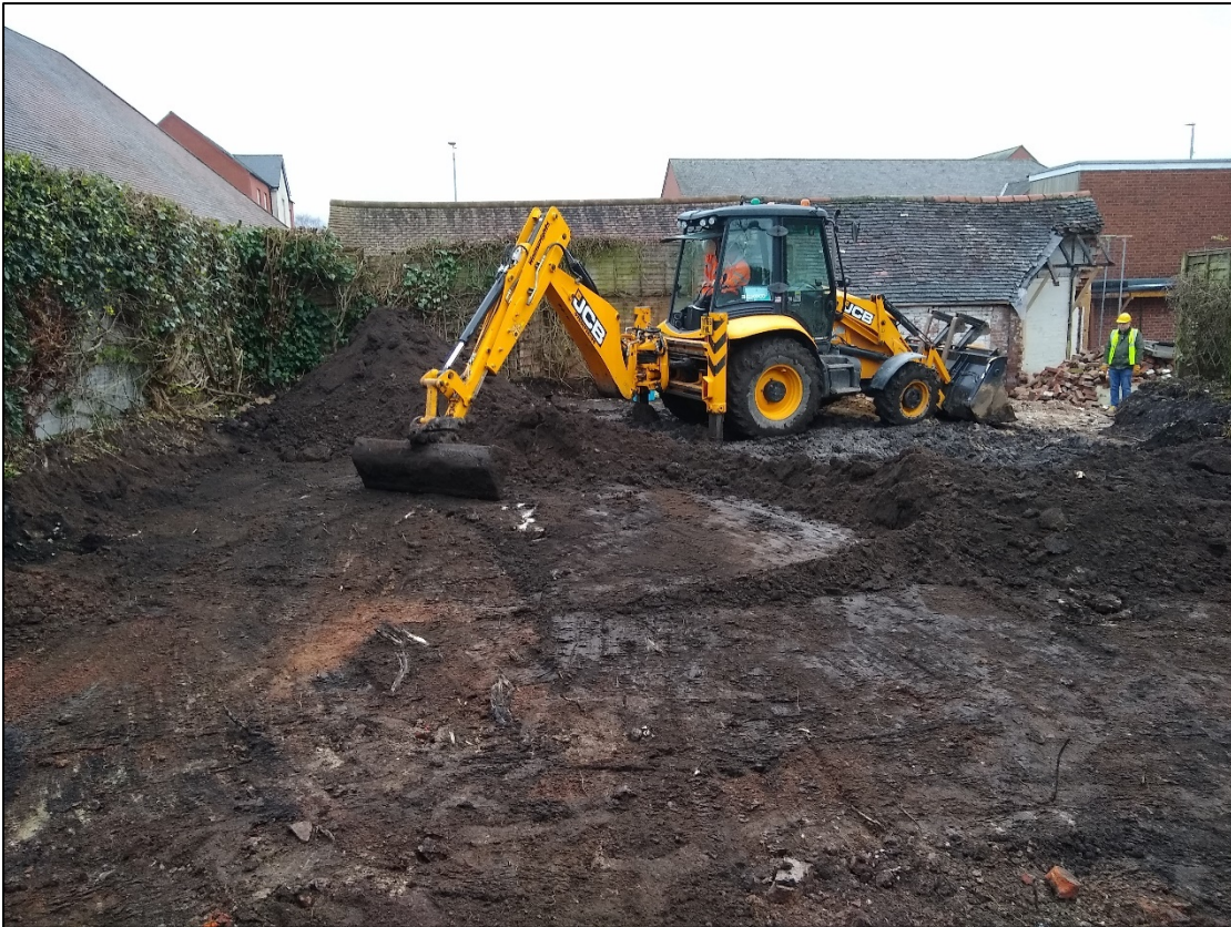
Fig. 4: rear car park area – ground reduction in progress (looking east)
