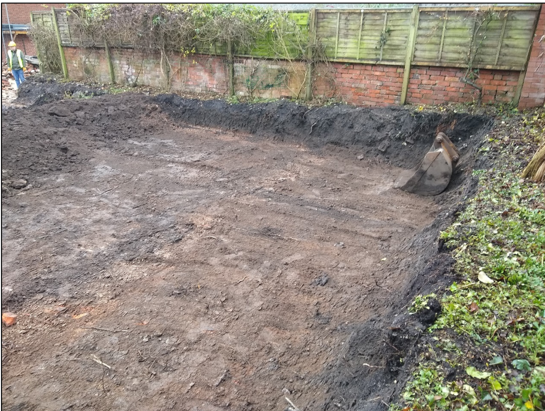
Fig. 5: rear car park area following reduction of ground levels (looking west)
