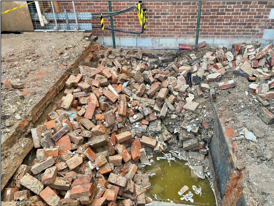
Fig. 2: rear extension area showing sub-basement
