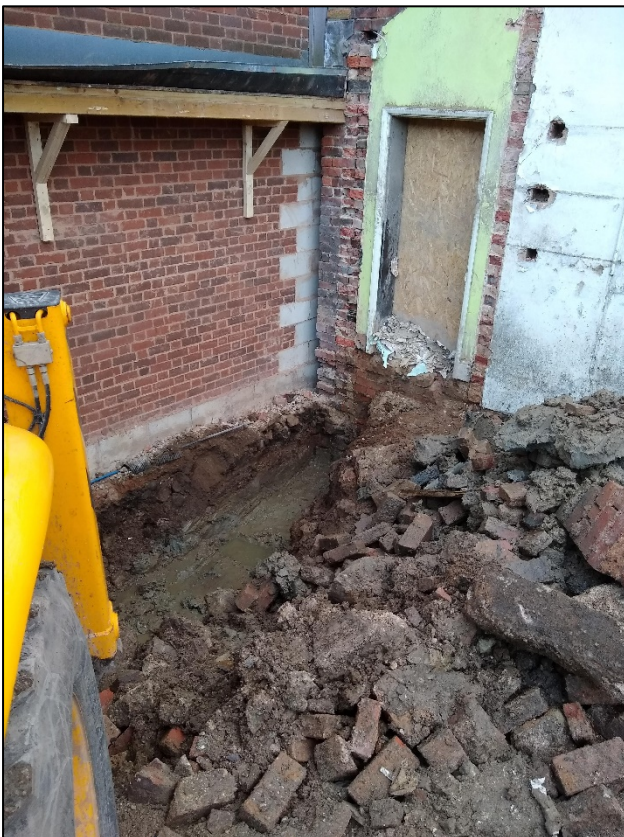
Fig. 3: rear extension area showing foundation trench with natural clay substrate exposed
