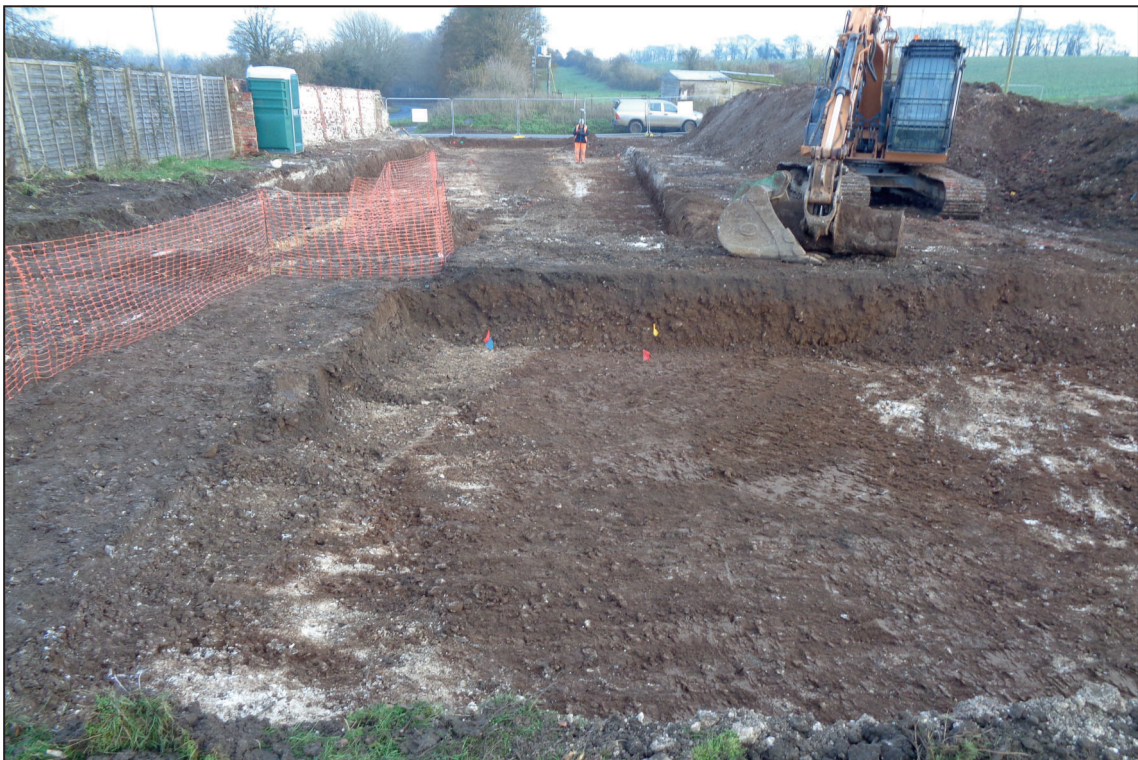
Area 2, looking east
