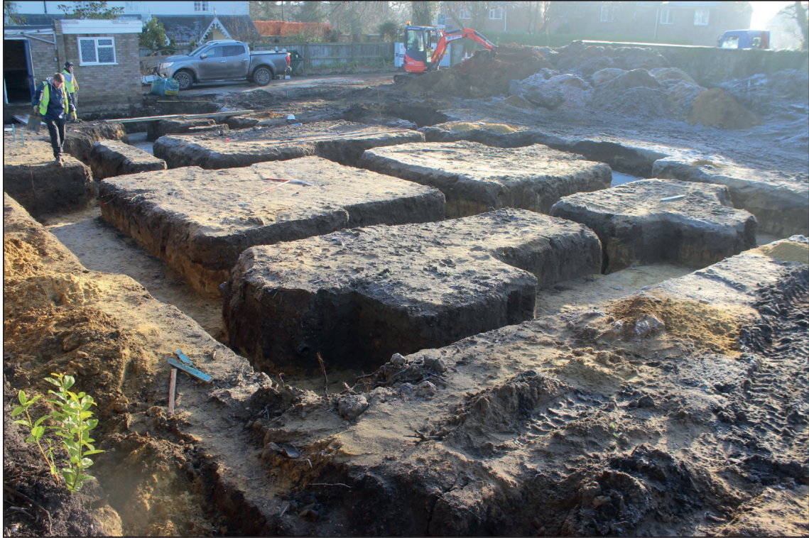
Area 1: excavated foundation trenches, looking south-east (1m scales)
