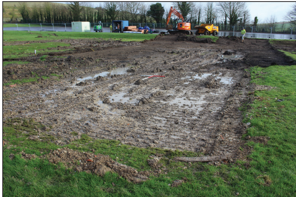
Foundation deposit 104, looking east (1m scales)
