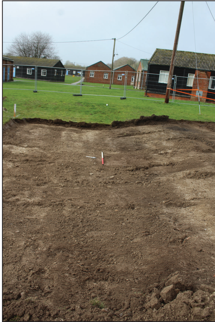
Foundation cut 106, looking west (1m scale)
