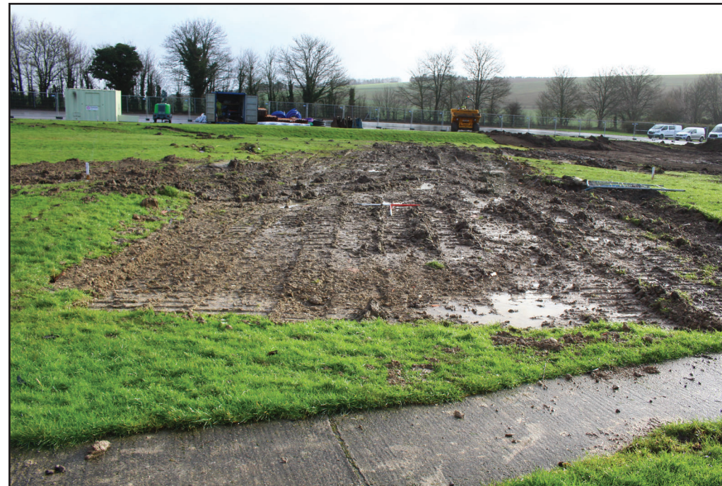
Foundation deposit 105, looking south-east (1m scales)
