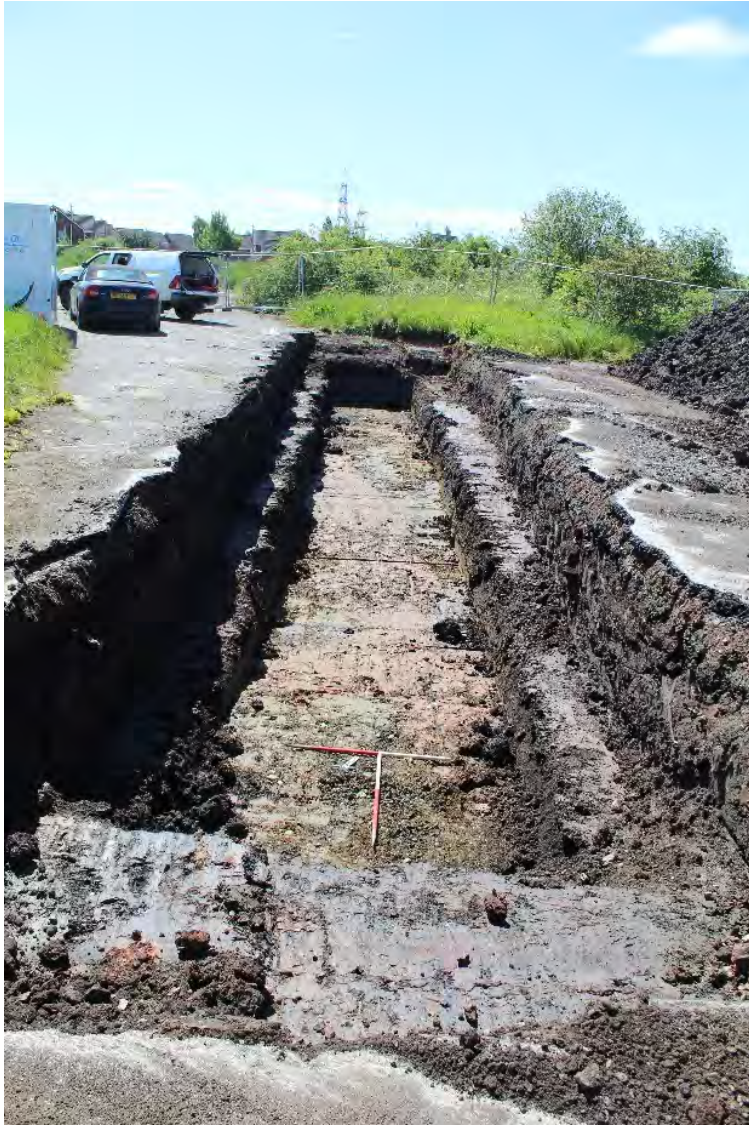
Fig 17. Trench 30, looking SE.
