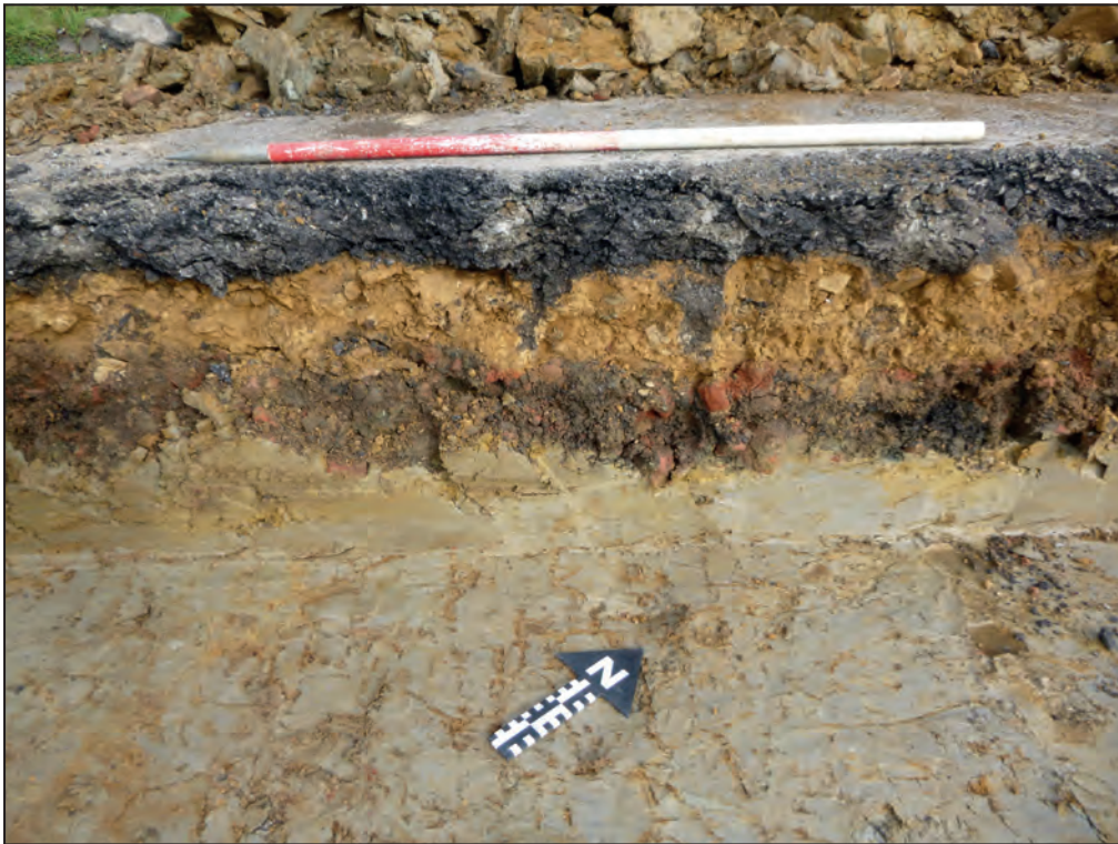
Trench 4 section, looking north-west (1m scale)
