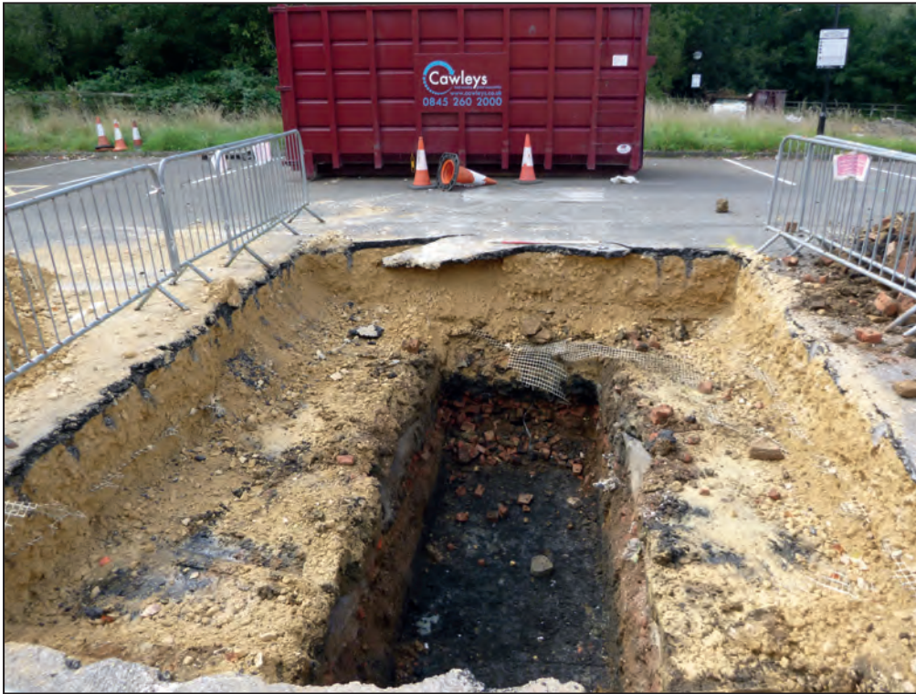
Overall trench 2, looking north-west (1m scale)
