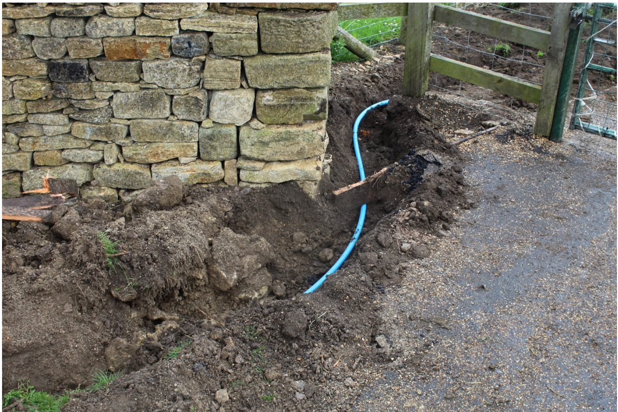
Fig. 8 Photograph, pipe installation around reinstated wall looking northeast.
