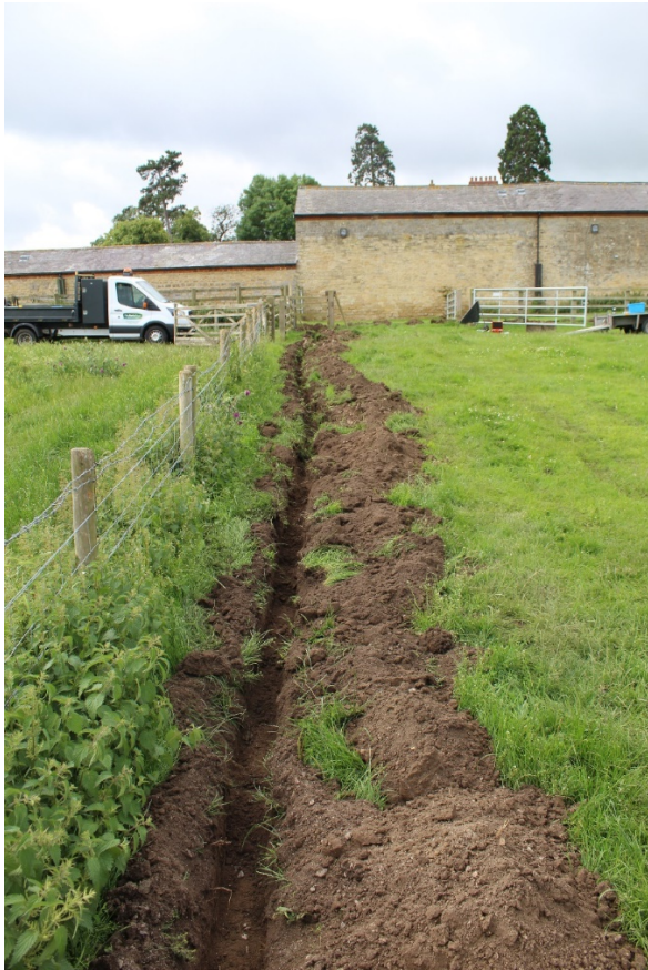
Fig. 3 Photograph, pipe trench looking south towards farm buildings.
