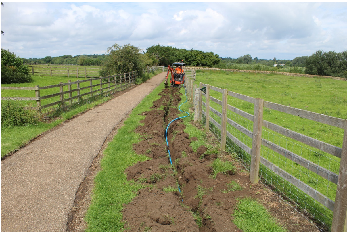
Fig. 4 Photograph, working shot of trench excavation looking west.
