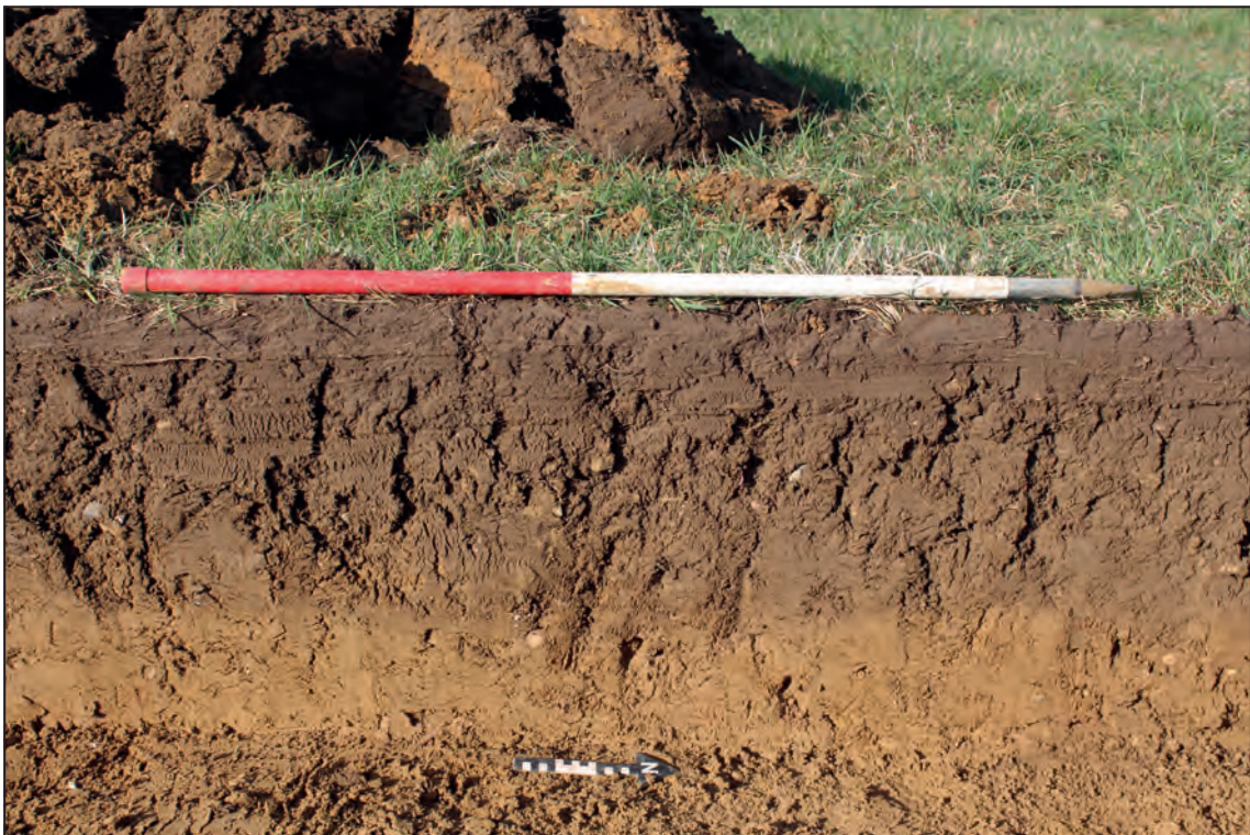
Trench 5 representative section, looking west (1m scale)
