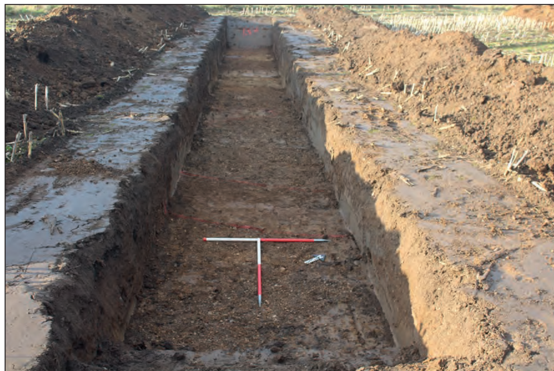
Trench 137, looking north-west (1m scales)
