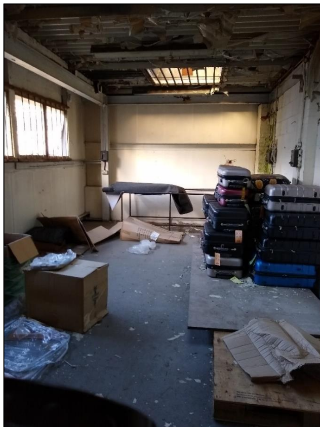
Photo 96 View of rear room in Building 8 first floor
