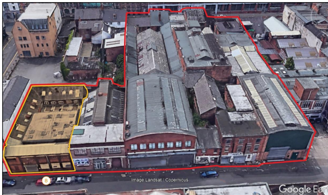
Fig.26 Aerial view of Building 8
