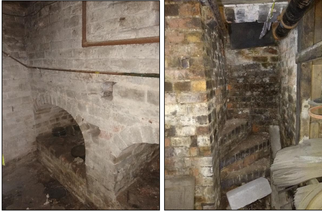
Photo 57 (left) furnace ovens seen in basement of No.29
