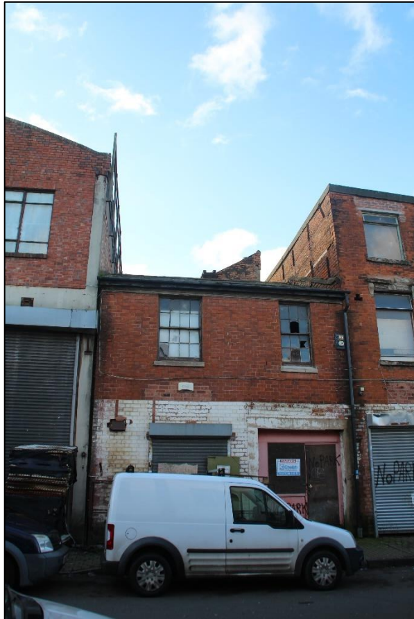
Photo 98 View of No.54A Barr Street
