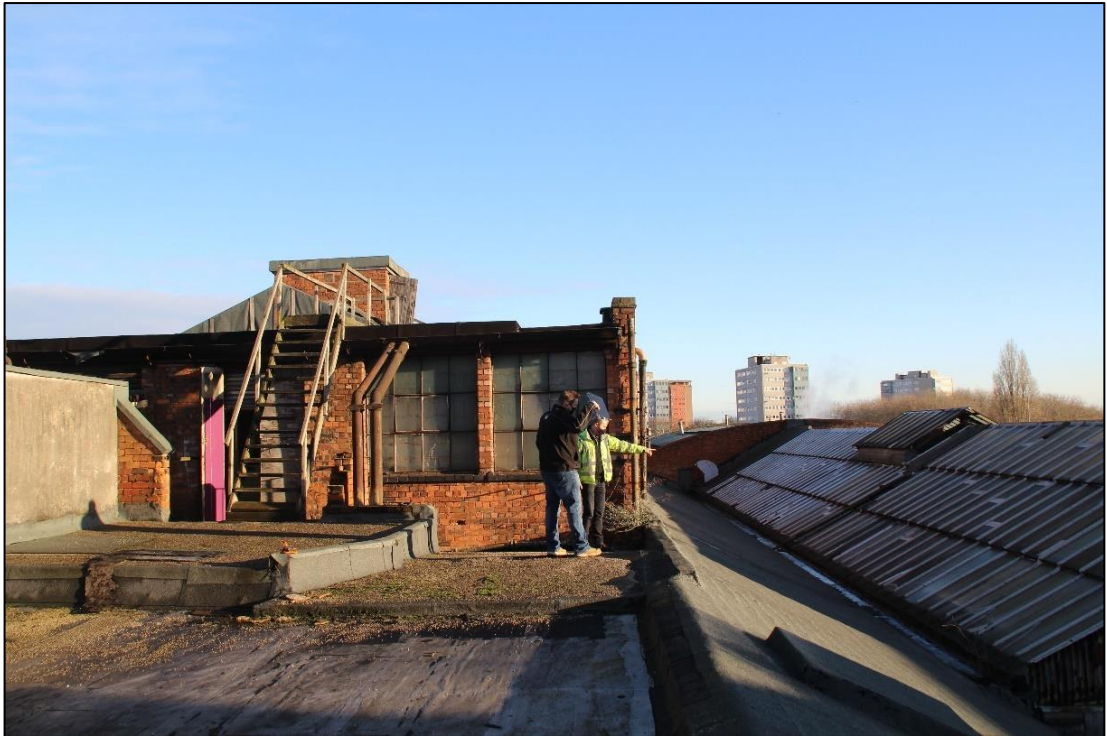
Photo 17 View looking east to the roofscape of Buildings 3 and 5
