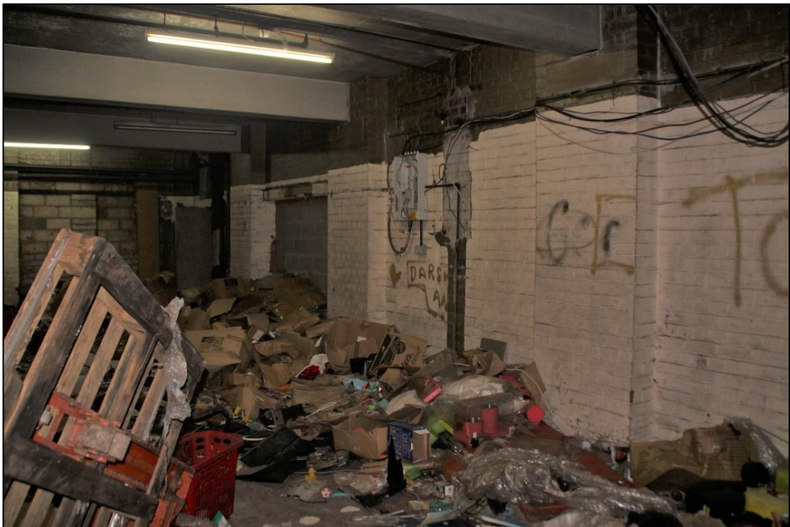
Photo 63 View of flank wall, Building 5
