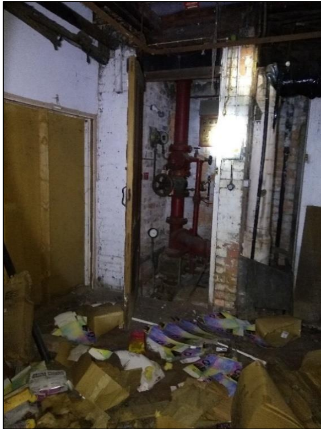
Photo 69 View of room with boiler pipes to the west of Building 5
