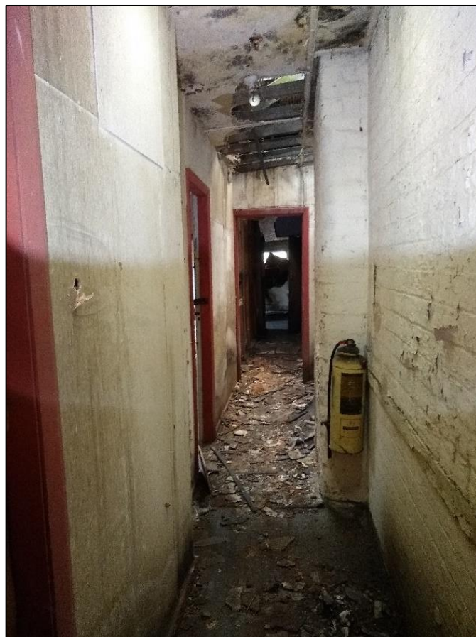
Photo108 View of the upper floor hallway in building C of Building 9
