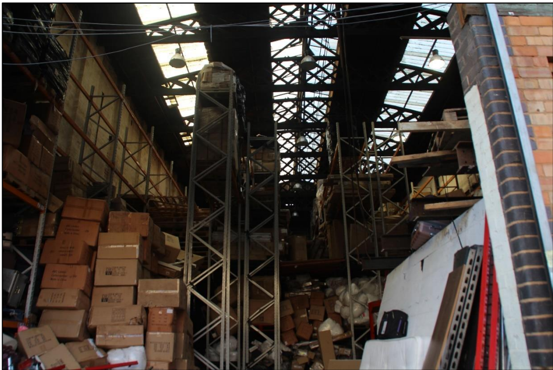
Photo 16 View of the Belfast roof truss of Building 2, seen from the entrance
