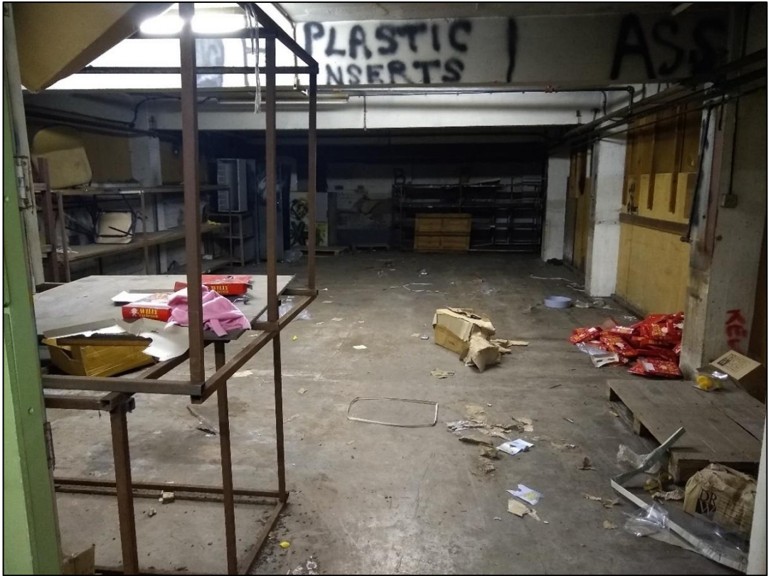
Photo 77 Basement floor of Building 6
