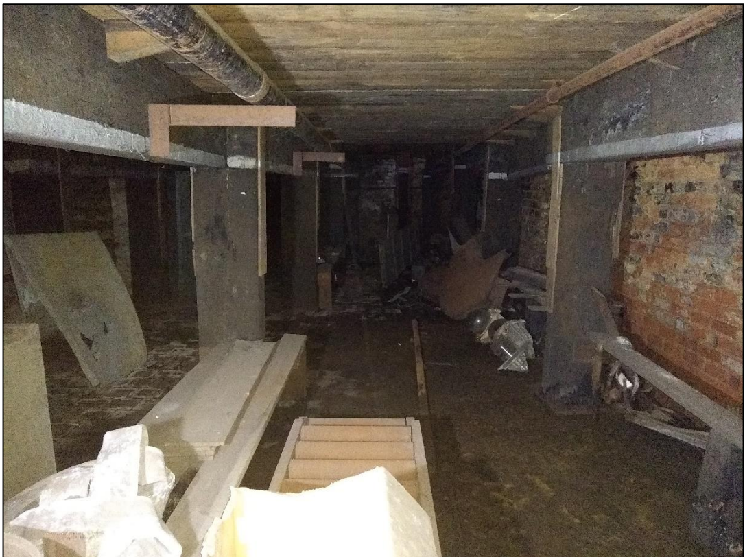
Photo 53 View of the basement of No.29 looking east
