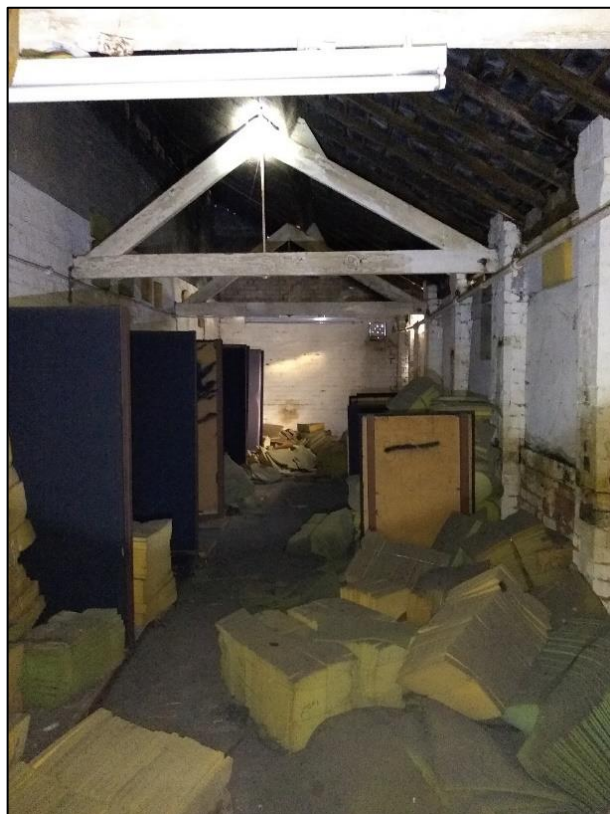
Photo 105 View of upper floor of linear range building A of Building 9
