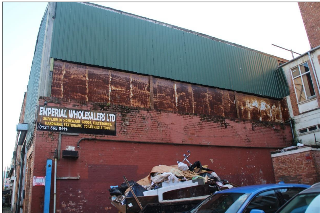
Photo 15 Southern (side) elevation of Building 2, looking north
