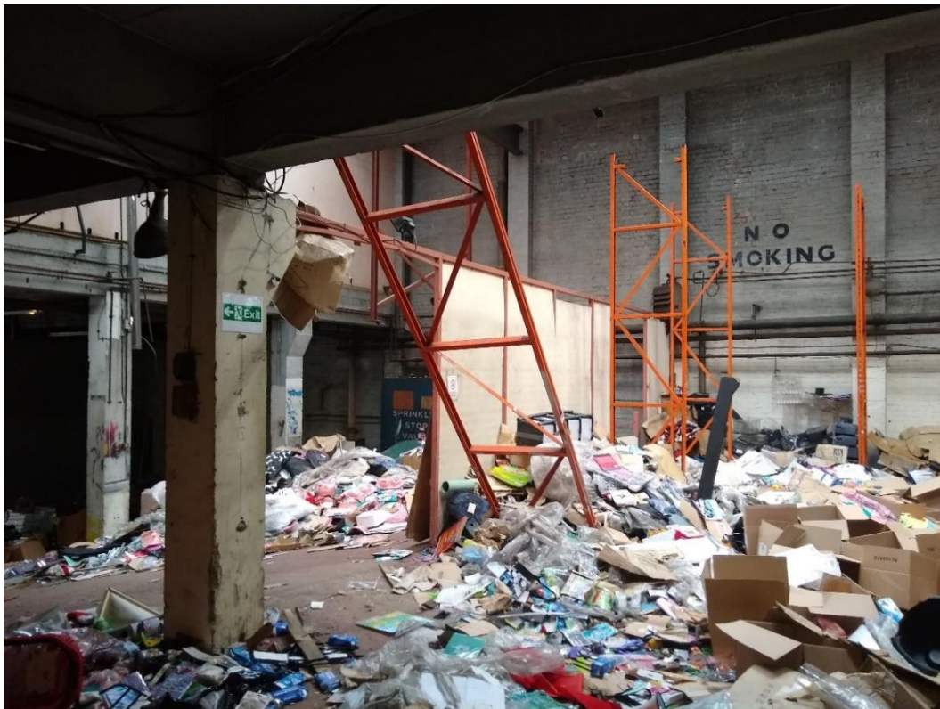
Photo 73 View of the main ground floor over the loading bay (to the left) in Building 6
