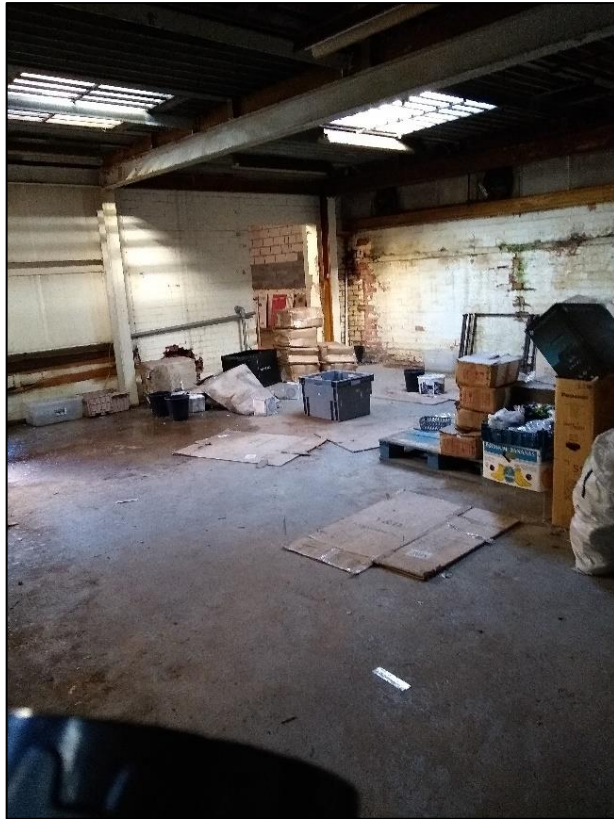
Photo 95 View of room in courtyard infill of Building 8
