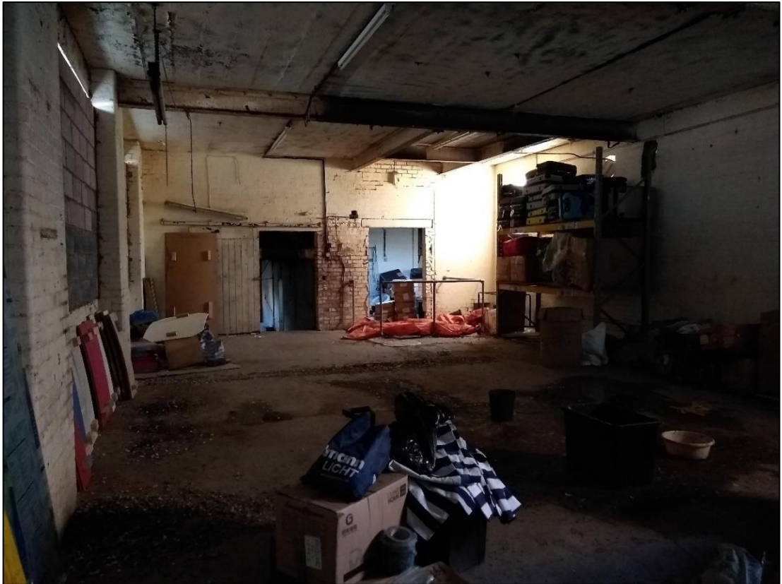
Photo 83 View of first floor of Building 7, looking south
