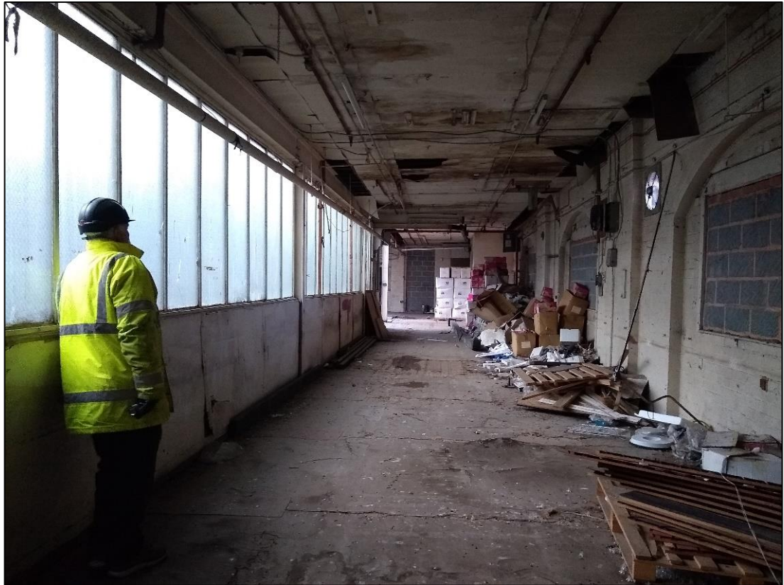
Photo 24 Second floor northern corridor in Building 3, looking west
