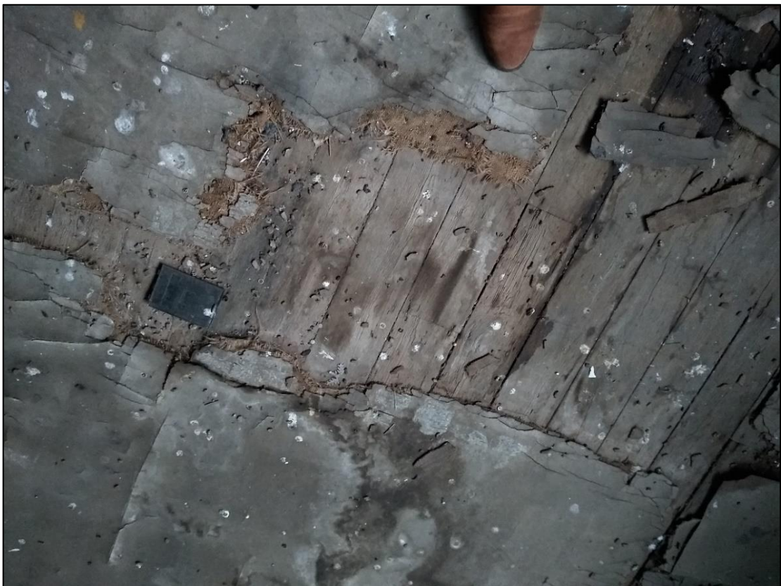
Photo 25 View of the timber and asphalt floor, second floor of Building 3
