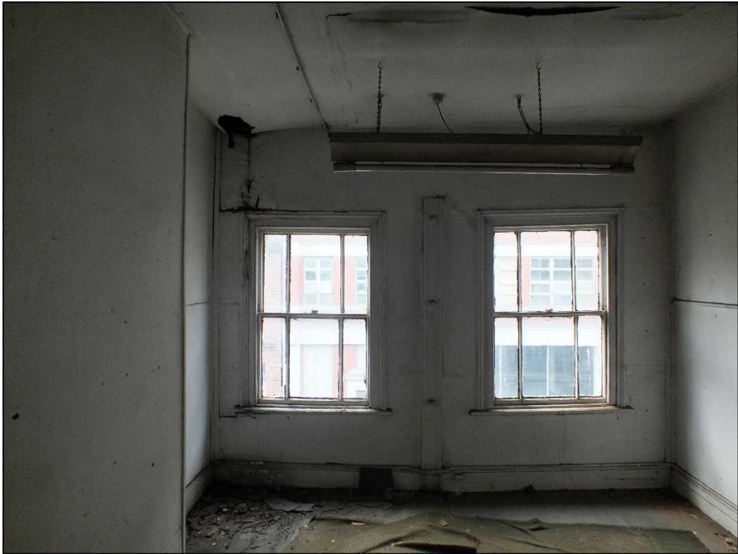
Photo 41 View of the windows overlooking Great Hampton Street, second floor No.28
