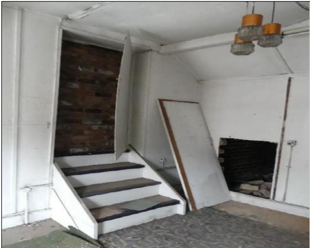
Photo 42 Internal stair, No.28 Great Hampton Street
