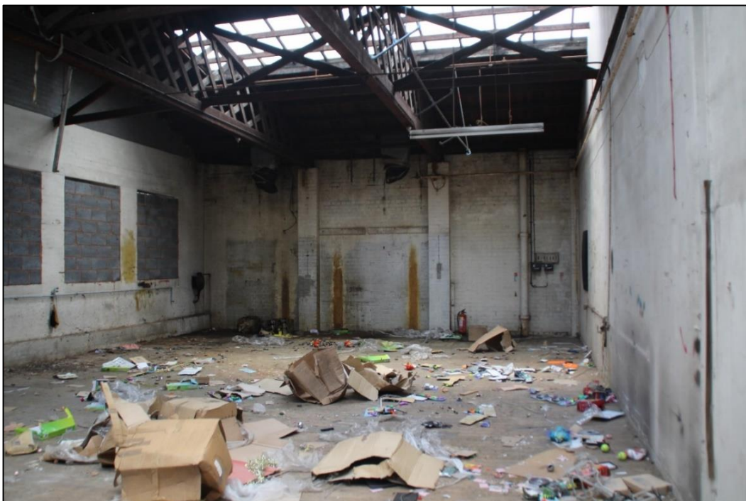
Photo 75 View of the upper floor in Building 6 over the loading bay
