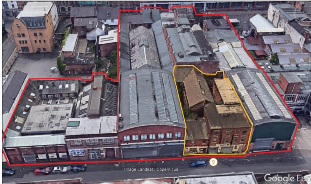
Fig.28 Aerial image of Building 9
