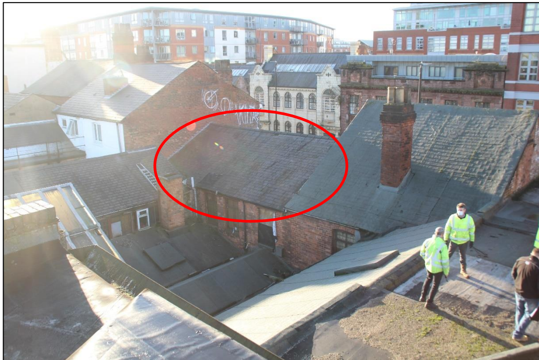
Photo 30 View of the roovescape of No.27 Great Hampton Street (circled)
