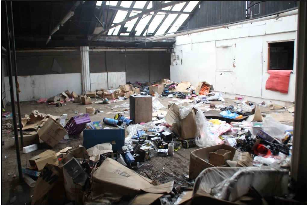
Photo 64 View of first floor in Building 5, looking west
