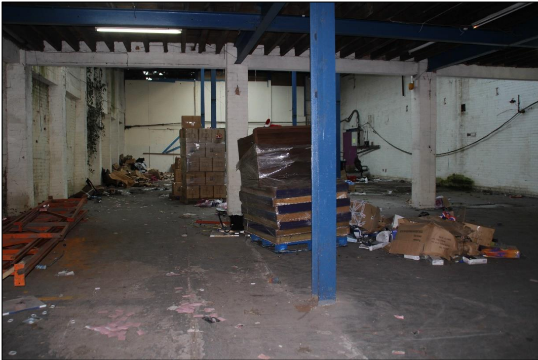
Photo 11: View looking east on the ground floor of Building 1
