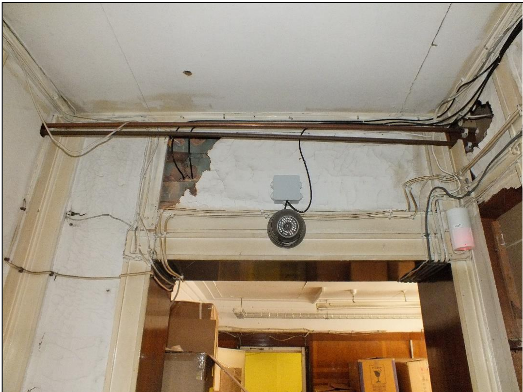
Photo 40 View of joinery detailing in No.28
