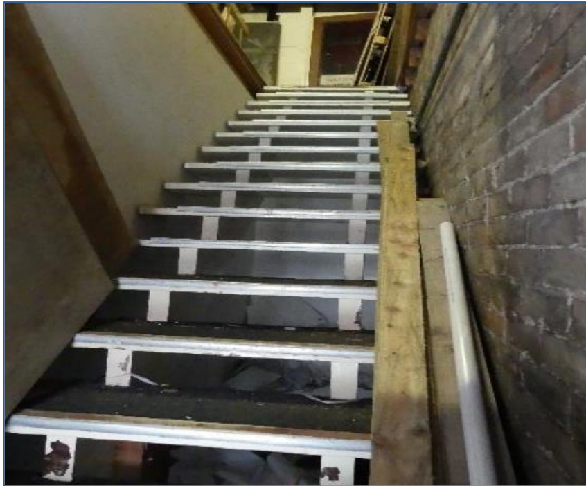
Photo 31 View up the staircase in No.27 Great Hampton Street
