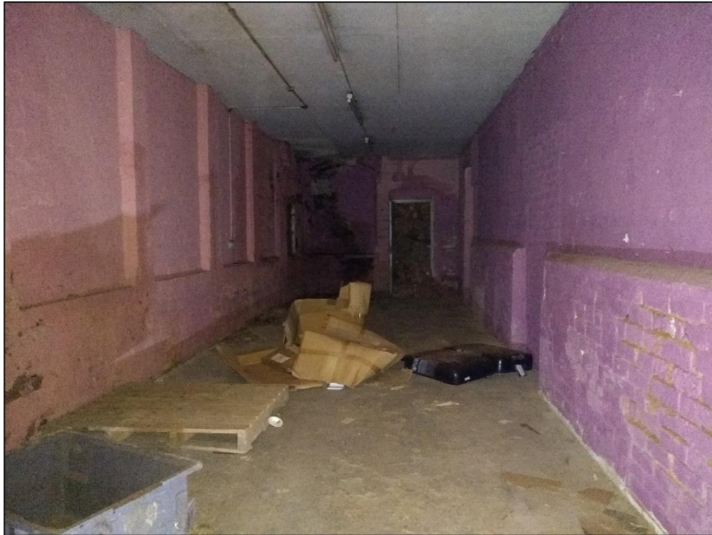
Photo 101 View of interior ground floor passageway, Building 9
