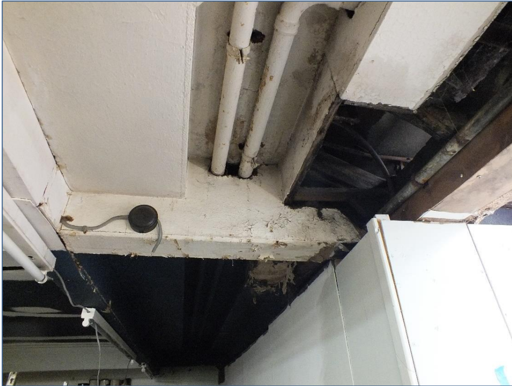
Photo 33 View internal details, No.27 Great Hampton Street
