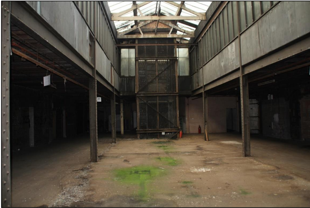
Photo 22 View looking west towards the lift shaft of Building 3
