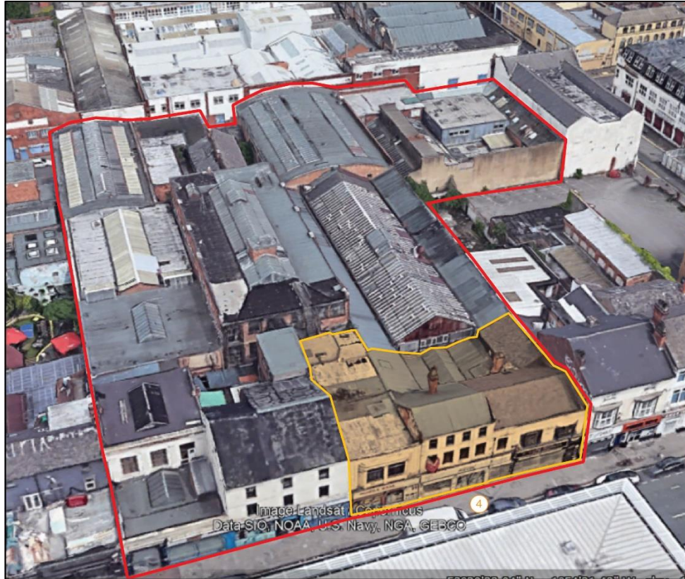
Fig.17 Aerial view of Building 4
