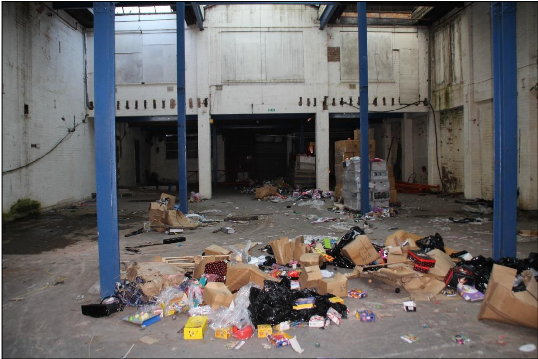
Photo 7: View looking west towards the mezzanine in Building 1
