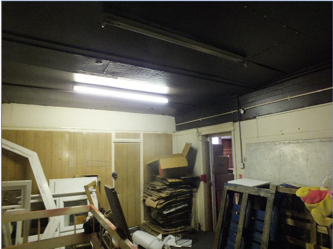
Photo 34 First floor room looking east towards Great Hampton Street
