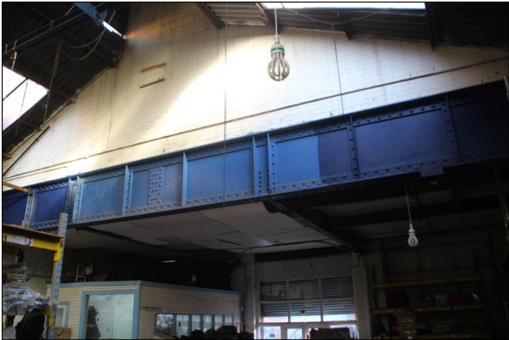
Photo 81 View of mezzanine structure from ground floor of Building 7
