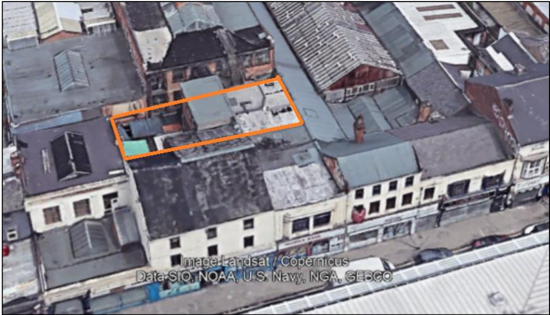
Fig.16 Detail of roof area adjacent to Building 3
