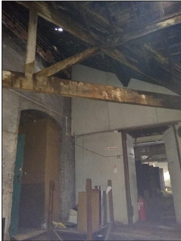
Photo 104 View of building A in rear range of Building 9
