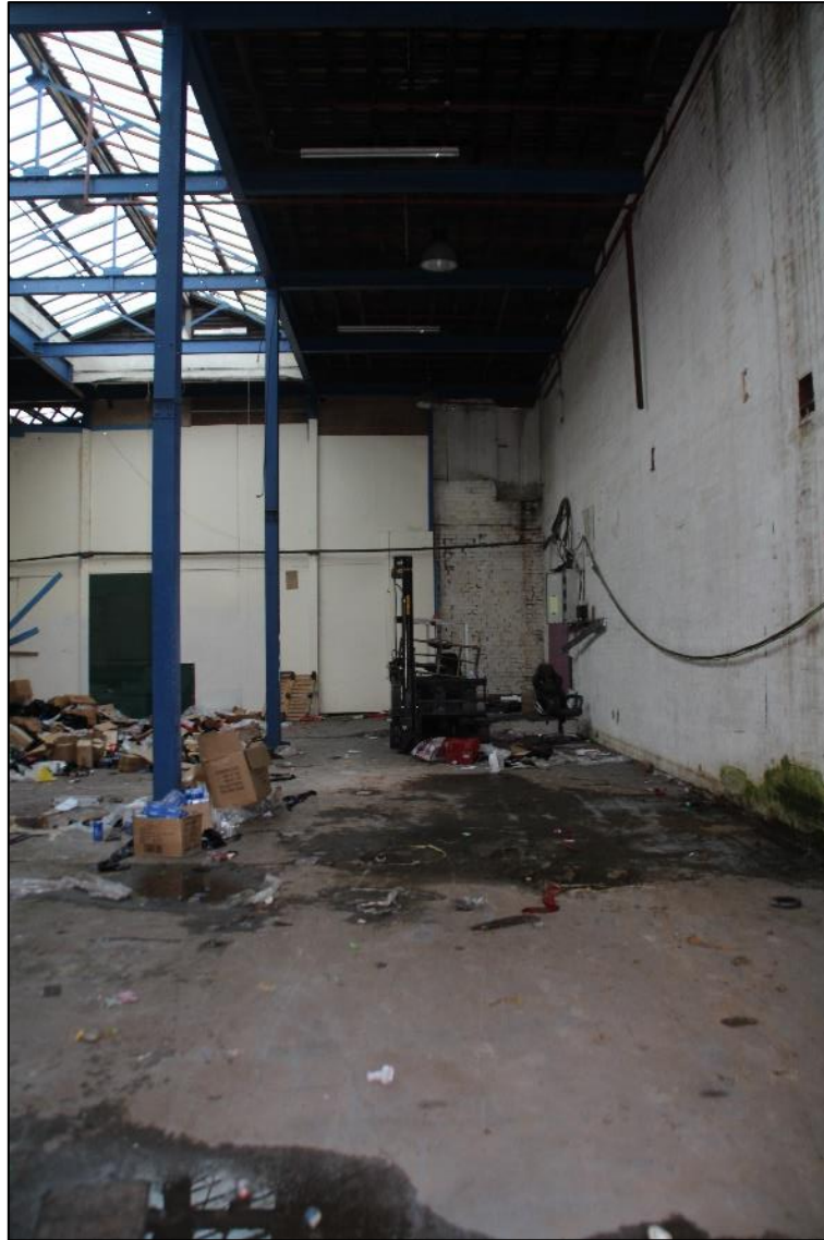
Photo 12: View looking east down the southern flank wall of Building 1
