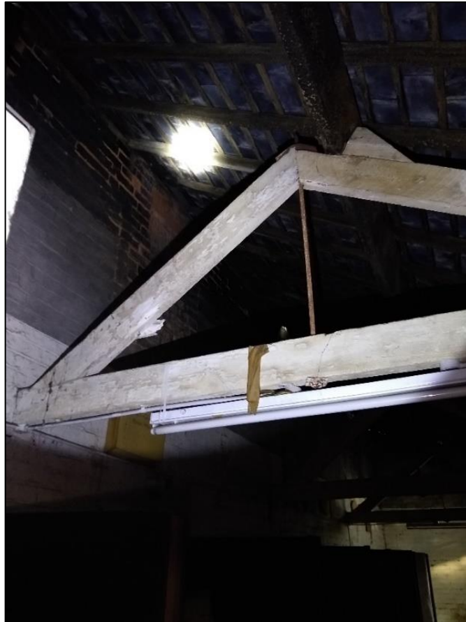
Photo 106 View of the roof truss in building A of Building 9
