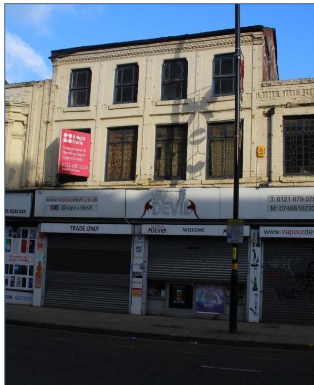
Photo 36 Front façade of No.28 Great Hampton Street
