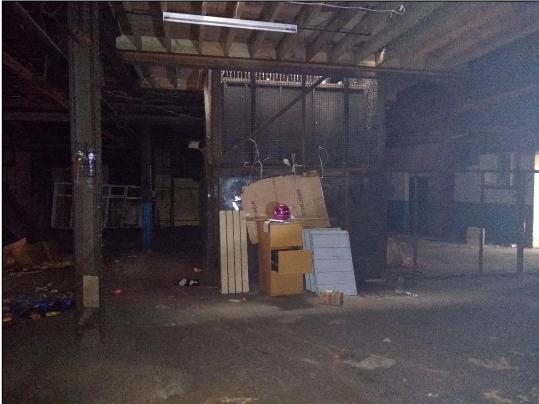
Photo 19 View looking west on the ground floor of Building 3
