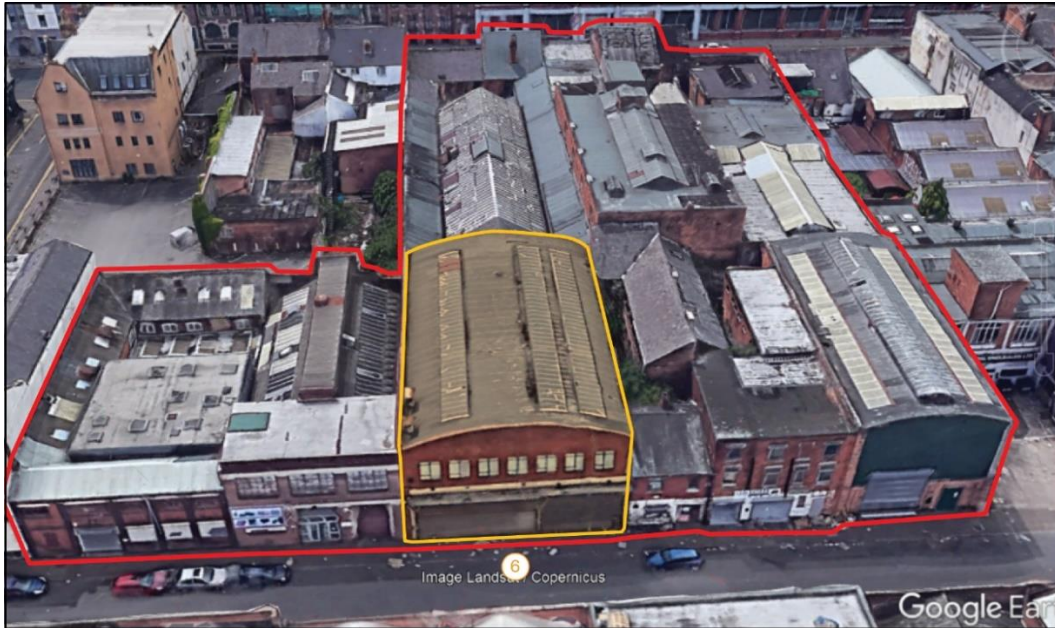
Fig.22 Aerial view of Building 6 viewed from Barr Street
