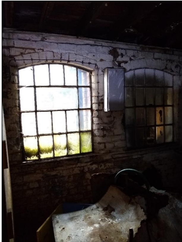
Photo 111 View of a window in building C of Building 9
