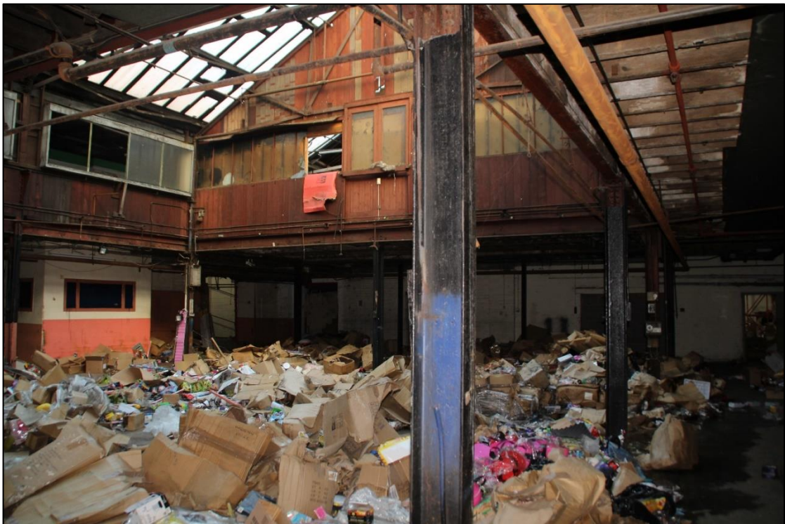
Photo 61 Internal view of Building 5, looking east
