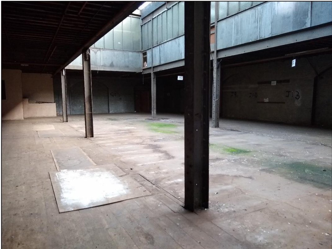
Photo 21 View looking east within the first floor of Building 3
