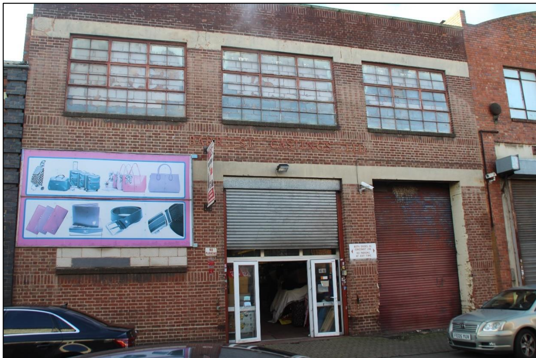
Photo 80 Barr Street frontage of Building 7
