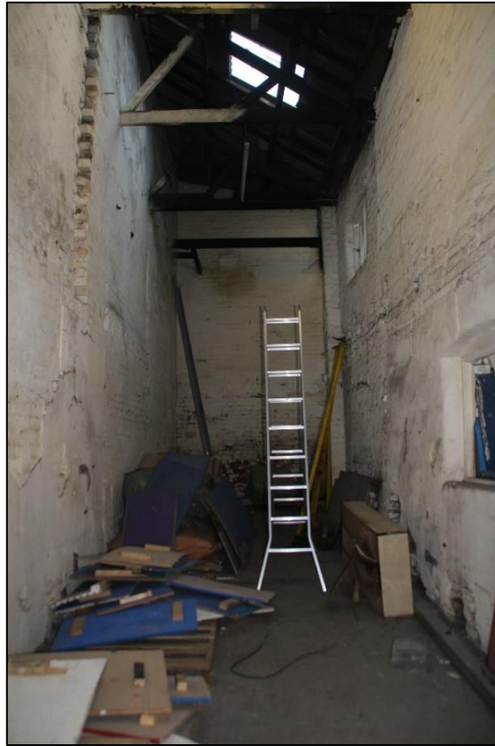
Photo 86 View of the southernmost linear former range in Building 8, looking west
