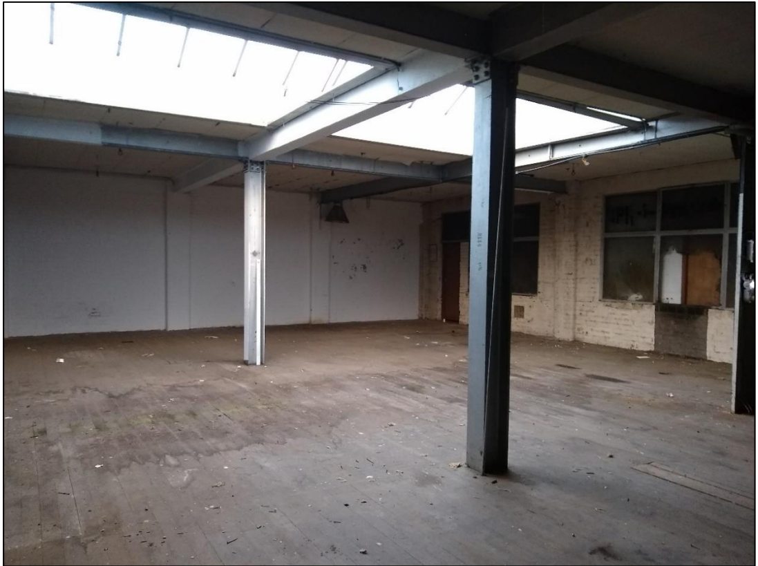
Photo 8: The first (mezzanine) floor of Building 1, looking north-east
