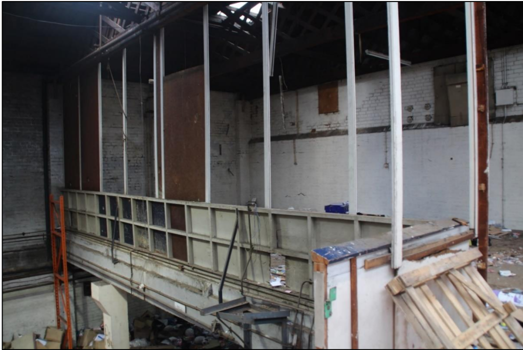
Photo 72 View of the mezzanine floor overlooking the loading bay in Building 6
