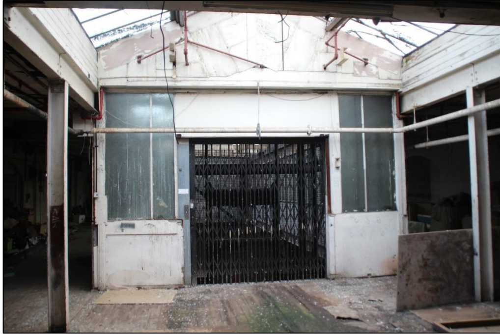
Photo 28 View of the lift in Building 3 on the second floor
