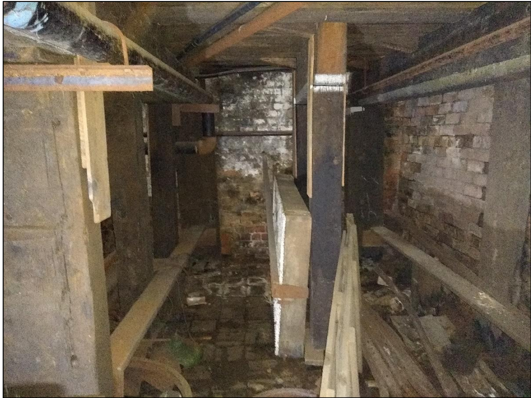
Photo 54 View of the basement on No.29 looking west
