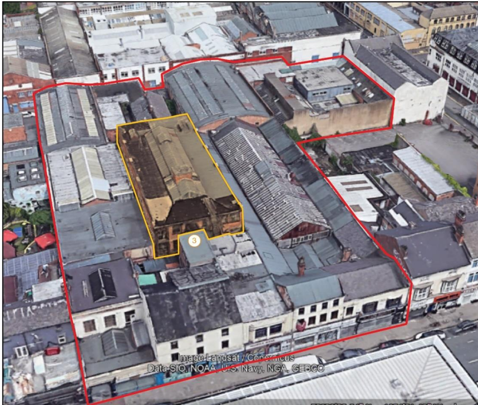
Fig.14 Aerial image showing location on Building 3
