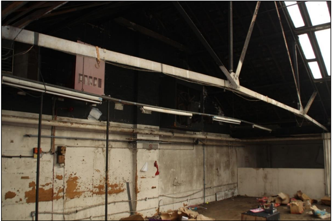
Photo 62 Internal view of roof truss on first floor of Building 5
