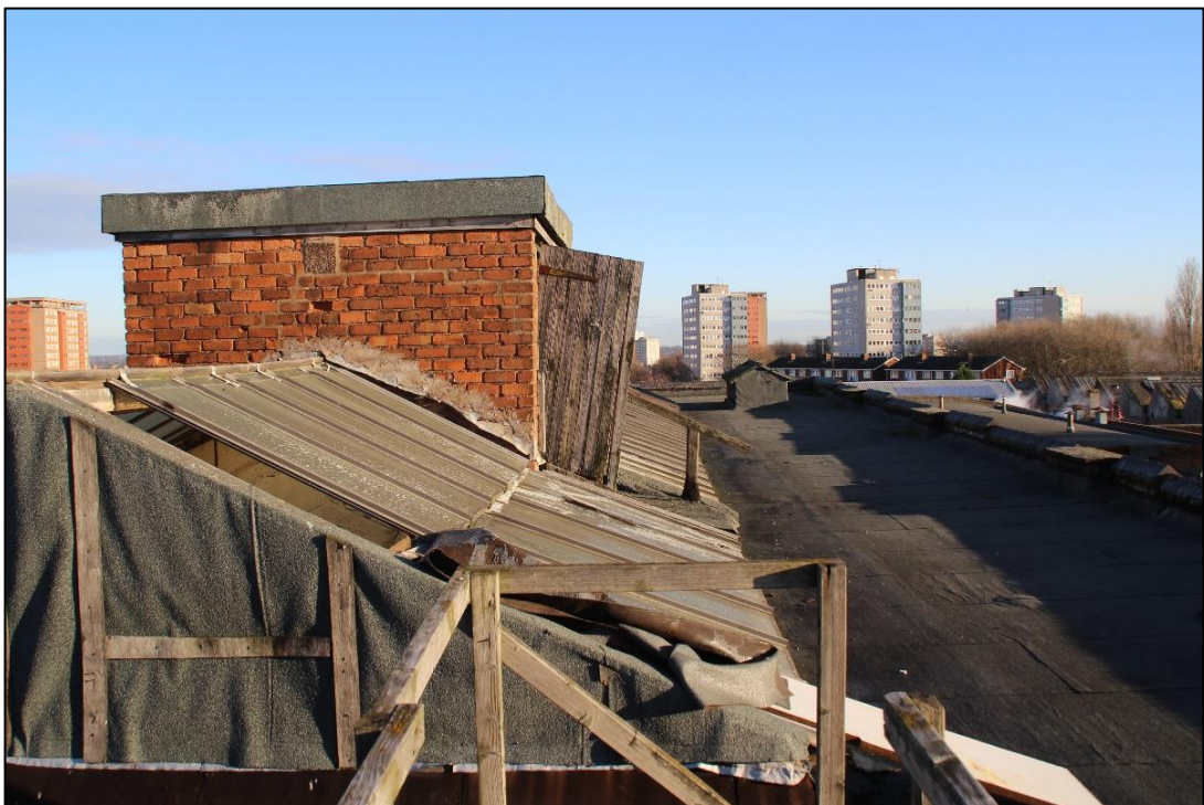
Photo18 Closer detail of the roof of Building 3
