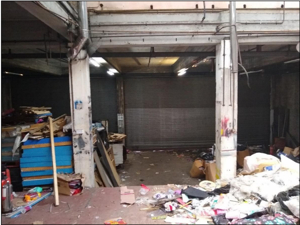
Photo 74 View looking east over the loading bay in Building 6
