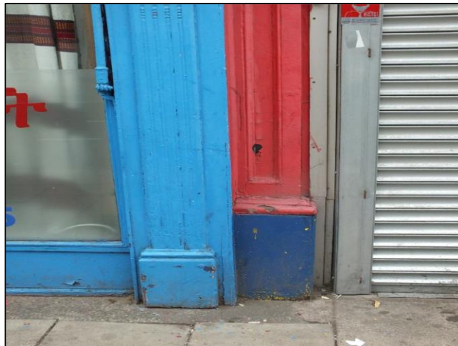
Photo 44 View of shopfront detail, No.29 Great Hampton Street
