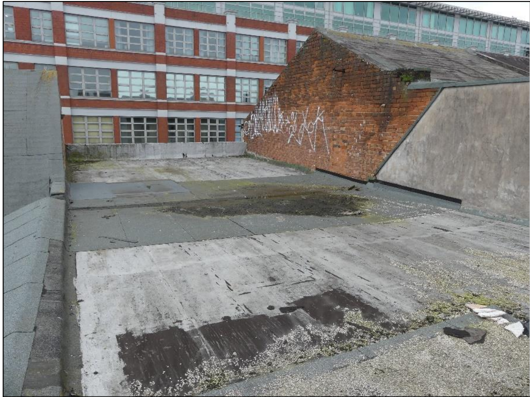
Photo 48 Flat roof of No.29 Great Hampton Street, looking east
