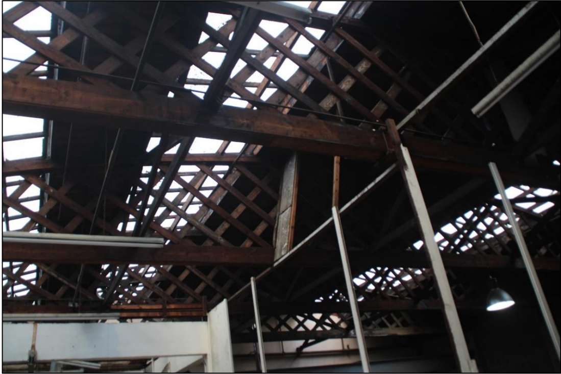
Photo 71 Internal view of the roof truss in Building 6
