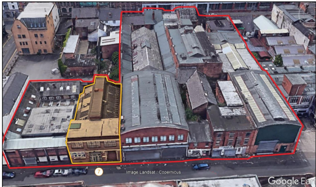
Fig.24 Aerial view of Building 7
