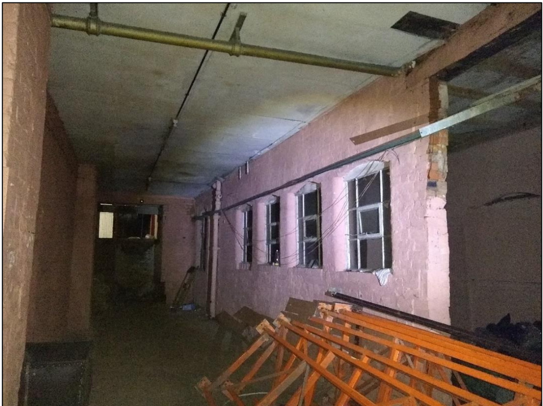
Photo 100 View of interior passageway, ground floor Building 9
