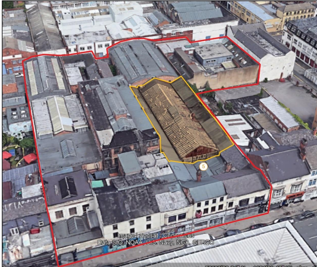
Fig.20 Aerial view of Building 5
