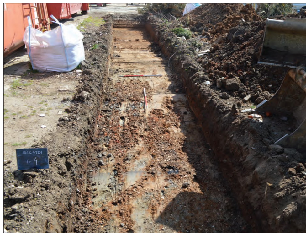
Trench 4, looking north-east (scales 1m)
