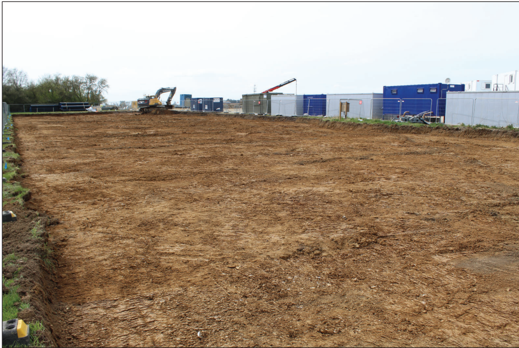
Area 1 after site strip, looking south-east
